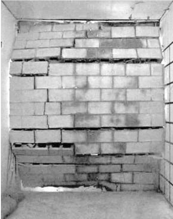
Figure 17.10 Example typical of the response expected from a CMU wall struck by a blast; at the time shown, the CMU is moving at several tens of feet per second (Photo courtesy of The Energetic Materials and Research Testing Center)
