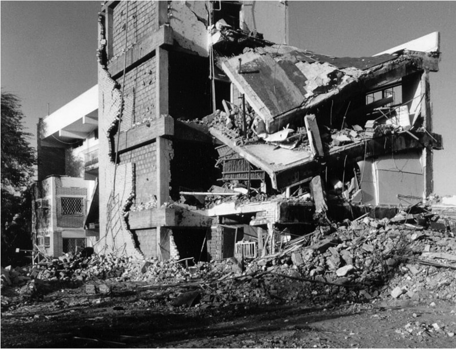
Figure 16.1 Failure of Building with Masonry Infill Walls
