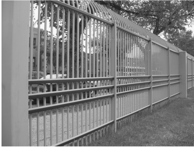
Figure 12.19 Anti-Climb Fence with Integrated Catch Cables
