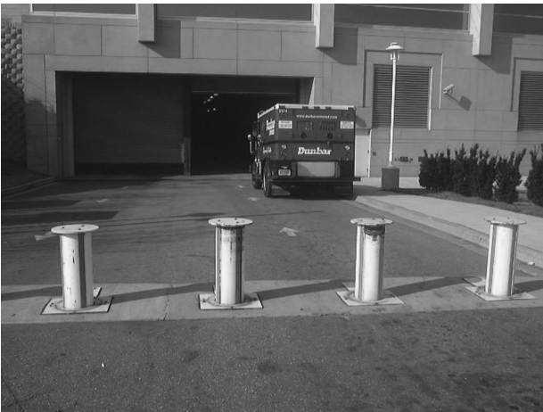
Figure 12.11 Operable (Pop-Up) Bollards
