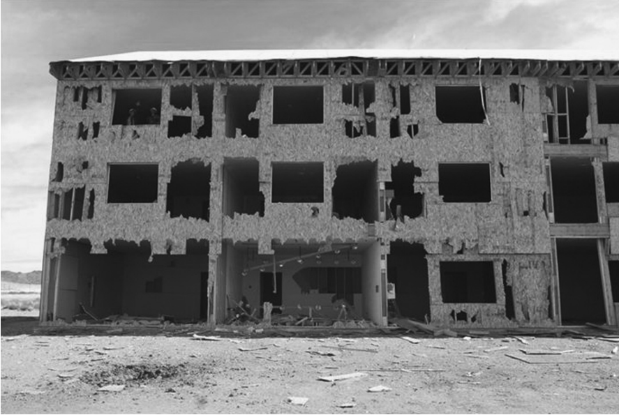
Figure 5.2 Full-Scale Building Testing
