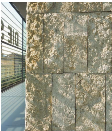
Fig. D5.2 Natural stone wall in the access corridor
