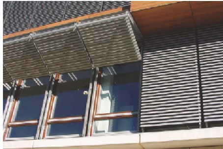
Fig. C1.33 Folding shutters for the Campeon office building in Munich. Architects: Maier Neuberger Projekte GmbH
