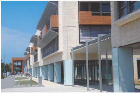
Fig. C1.33 Folding shutters for the Campeon office building in Munich. Architects: Maier Neuberger Projekte GmbH
