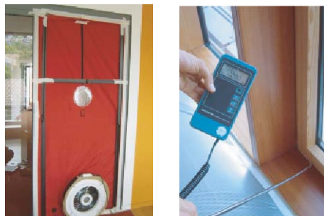
Fig. C3.1 Blower door, built into an ordinary door. Infiltration level reading did not show any leakage at window joints at a wooden façade.
