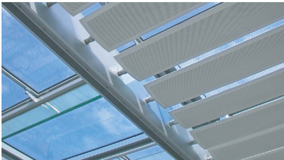
Fig. D5.4 The glass roof presents with an arrangements of multifunctional lamella with reflectance function toward the top.
