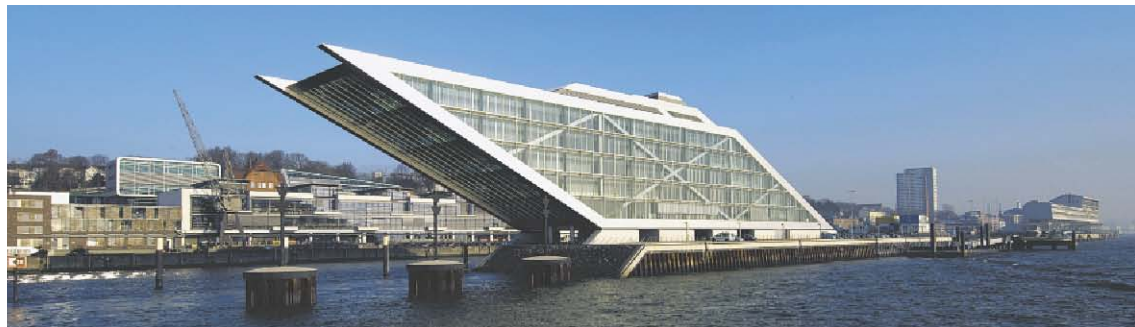
Fig. D1.1 Dockland Office Building, Hamburg/Germany
