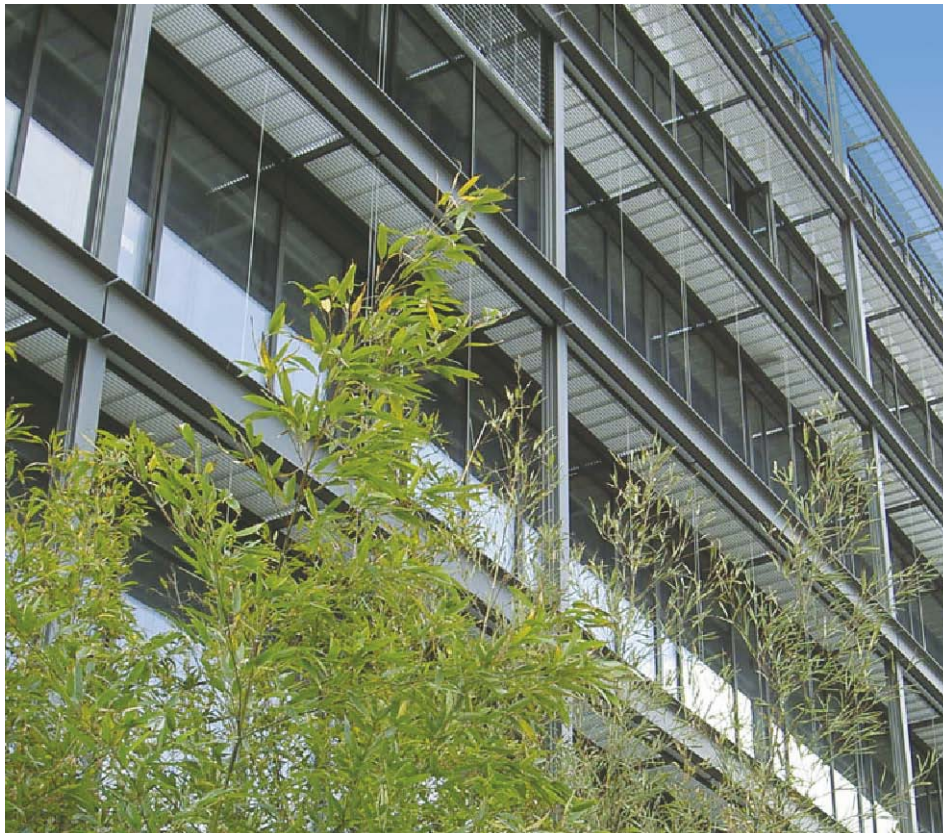
Fig. D3.2 The triple glazing for the building was designed especially and the frame elements were premium heat insulated
