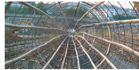
Fig. C2.31 Drilling pile during construction of a building. By layering the pile with pipelines, an energy pile for heating and cooling may be created.
