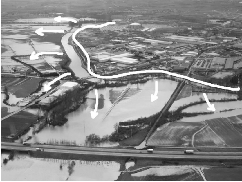
Figure 7.3 Multiple projects for ecological regeneration and hydraulic adaptation have been implemented over the last few years. The city of Vitoria-Gasteiz is situated over a huge underground aquifer, and the adequate management of the water has been of great importance for recognizing the “tangible” values of the greenbelt. Credit: CEA.
