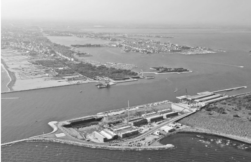
Figure 6.2 The Chioggia, one of the three inlets that connect the Venetian Lagoon and the Adriatic Sea. In the foreground, the temporary gate housing caisson prefabrication site and the double lock for fishing boats and emergency vessels. In the background, Chioggia. Credit: Ministry of Infrastructure and Transport—Magistrato alle Acque (Venice Water Authority), concessionary Consorzio Venezia Nuova image archive.
