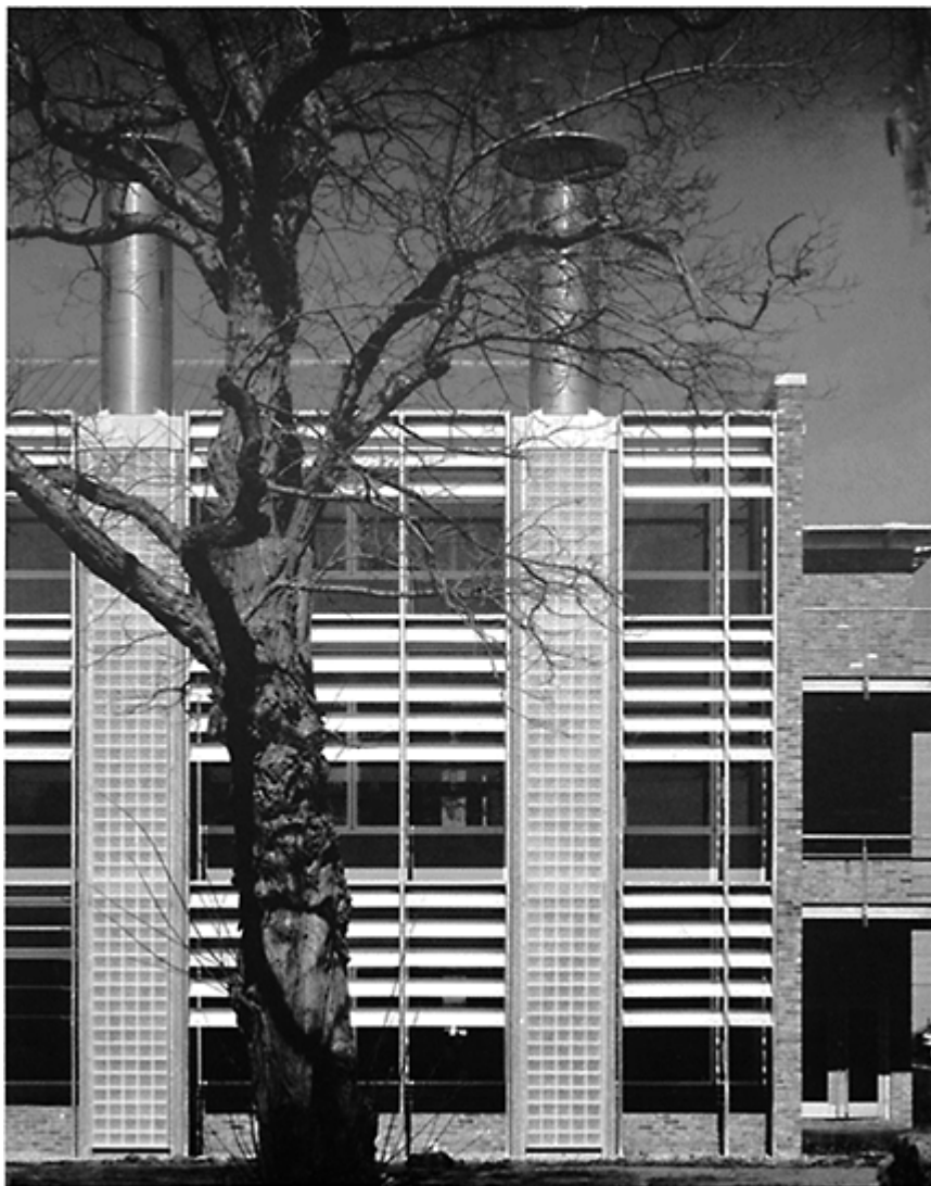
11.1 Detail of south facade showing relationship between ventilation stacks and solar shading. The Environmental Building, BRE, Garston. Architects: Feilden Clegg.
