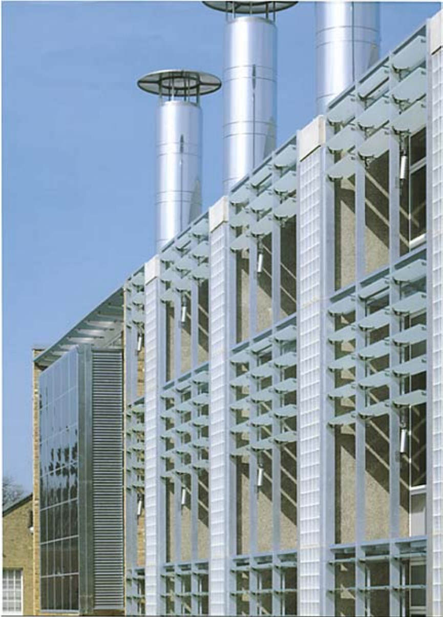
Atrium, Anglia Polytechnic University. Architects: ECD Architects.
