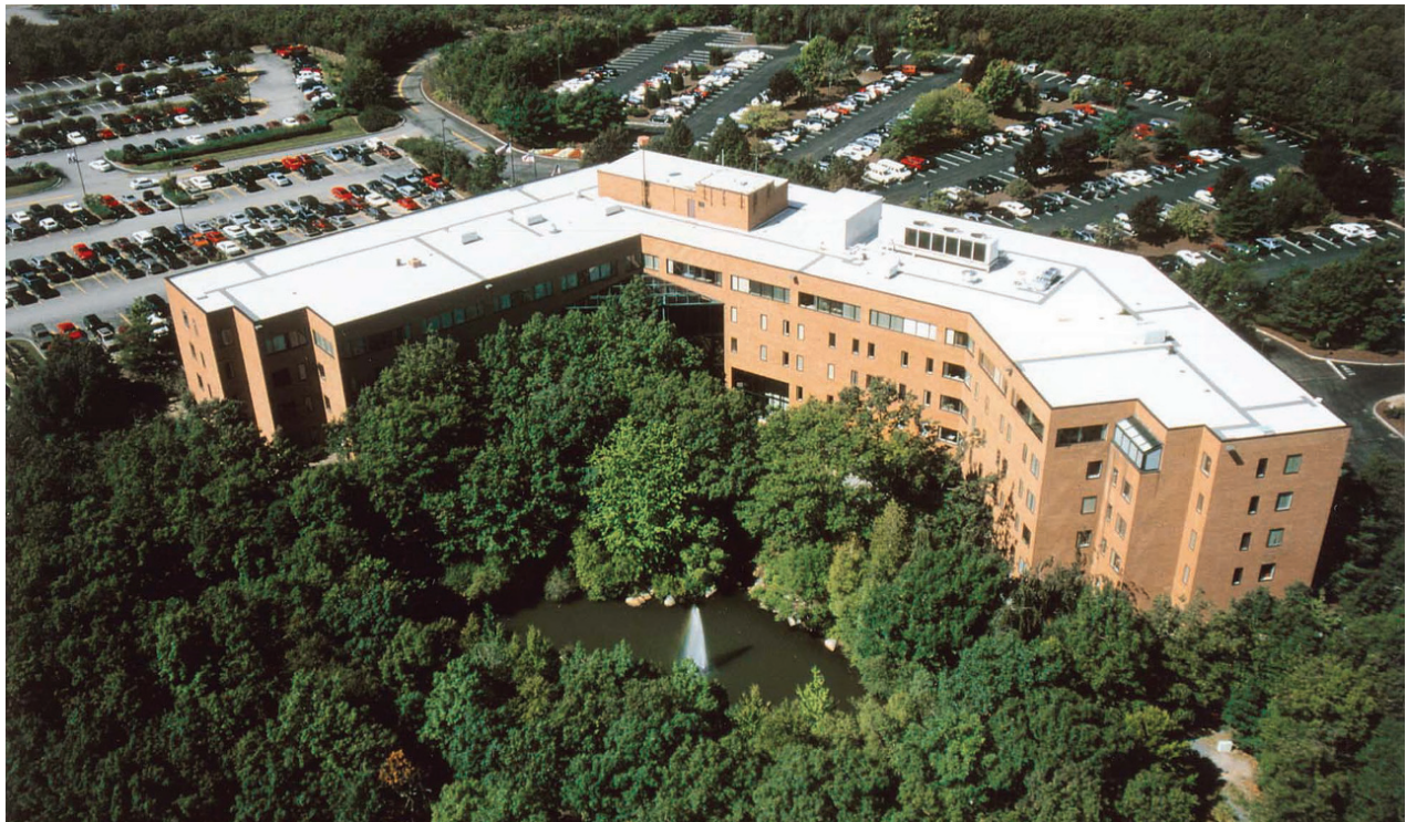
The National Fire Protection Association Headquarters in Quincy, MA, features a Sarnafil EnergySmart Roof®. (Photo courtesy of Sarnafil.)
