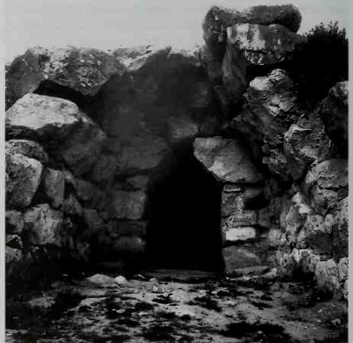
64. Tiryns, citadel, late thirteenth century, chamber in the thickness of the east wall
