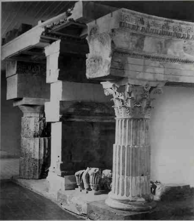
215. Epidauros, tholos, after 370, truncated reconstruction from within
