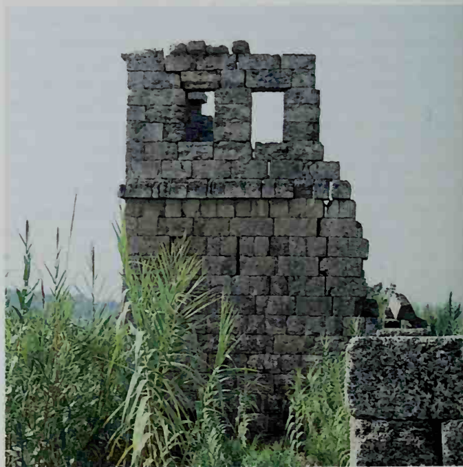
296. Perge, tower of city wall, probably third century
