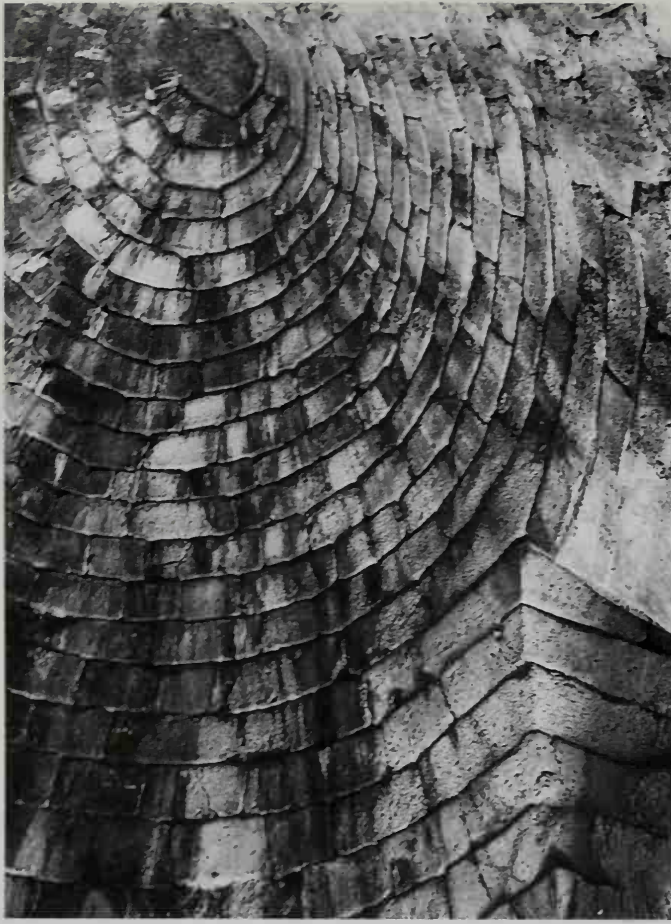
58. Mycenae, 'Treasury of Atreus', c. 1300–1250, vault from cap-stone to lintel
