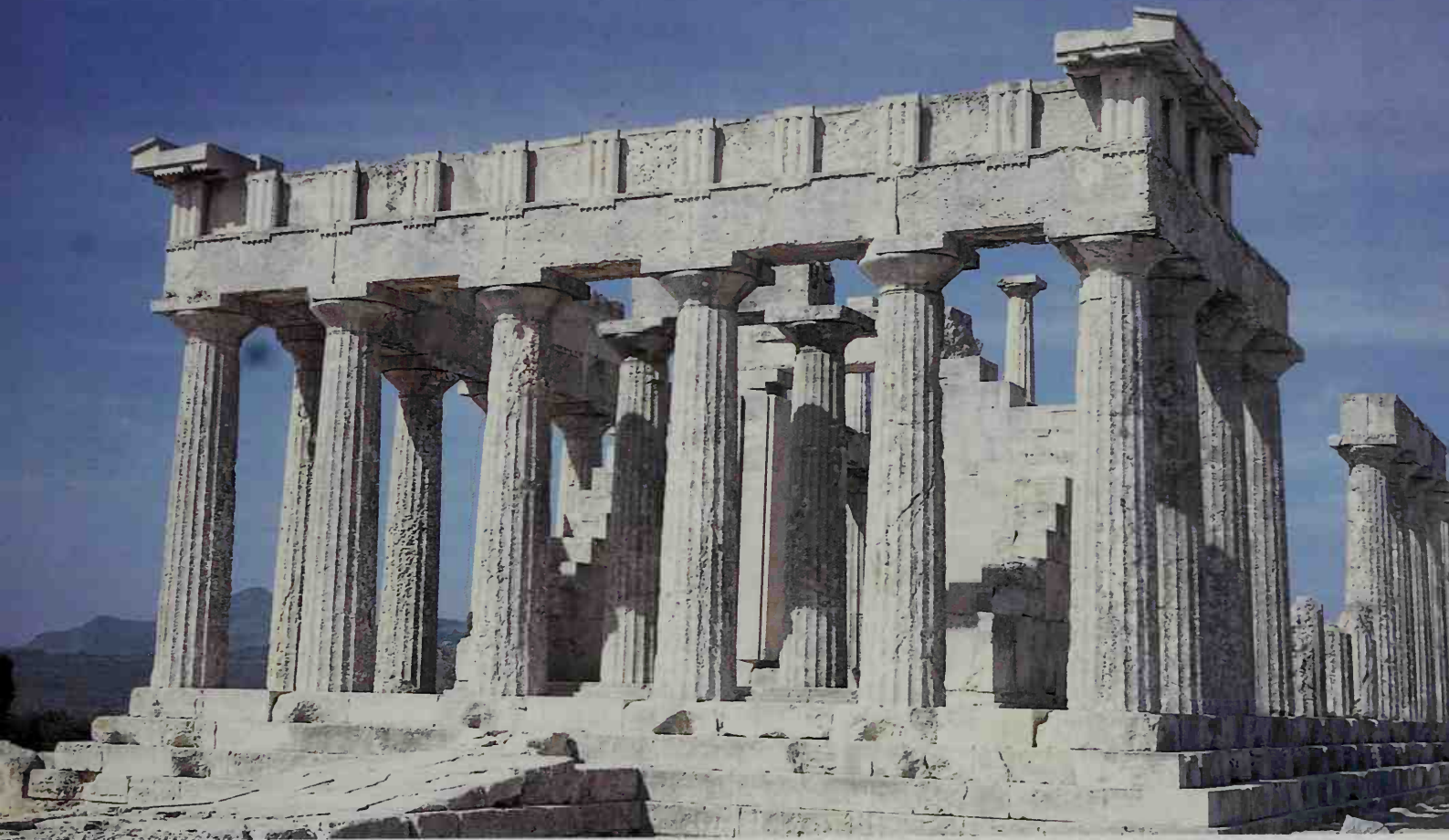
146 and 147. Aigina, temple of Aphaia, early fifth century, east end ( above ) and plan ( below )
