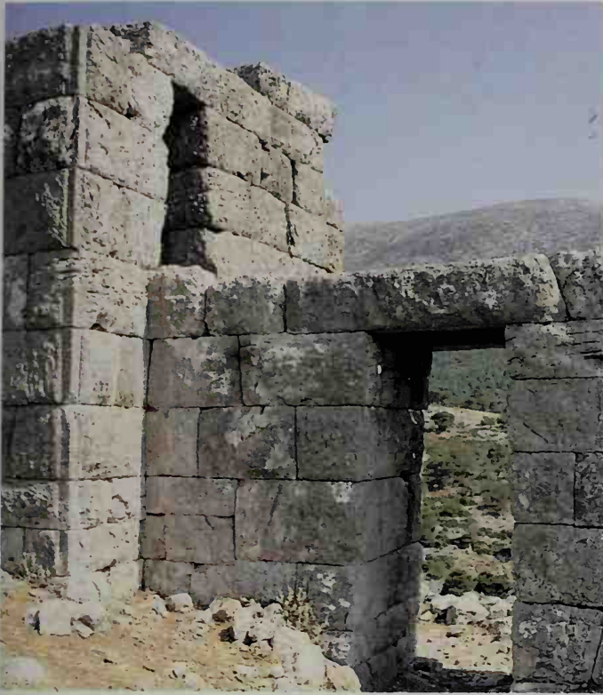
278. 'Eleutherai', Attic frontier fort, fourth century, wall-walk and tower
