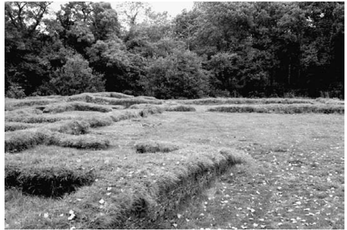
PLATE 265 Penhallam Manor: foundations of hall range to camera block from the kitchen
