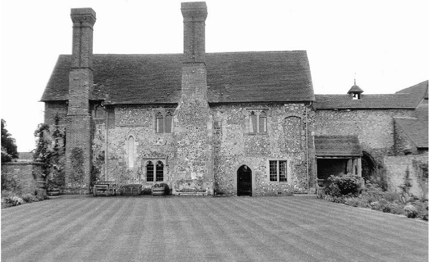
PLATE 170 Swanborough Manor: hall range from the north
