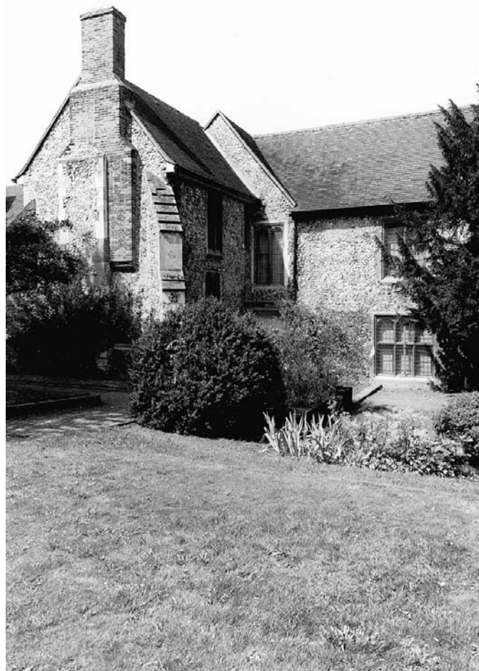
PLATE 159 Orpington 'Priory': camera and upper chamber blocks from the east
