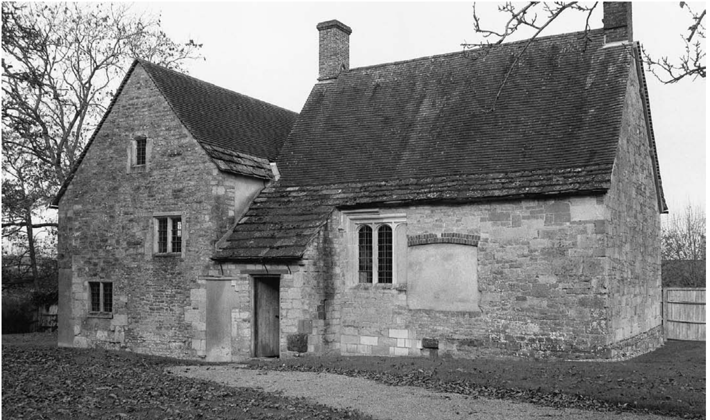
PLATE 236 Fiddleford Manor: hall and chamber unit from the south
