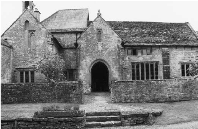
PLATE 277 Stoke Sub Hamdon Priory: hall range from the forecourt
