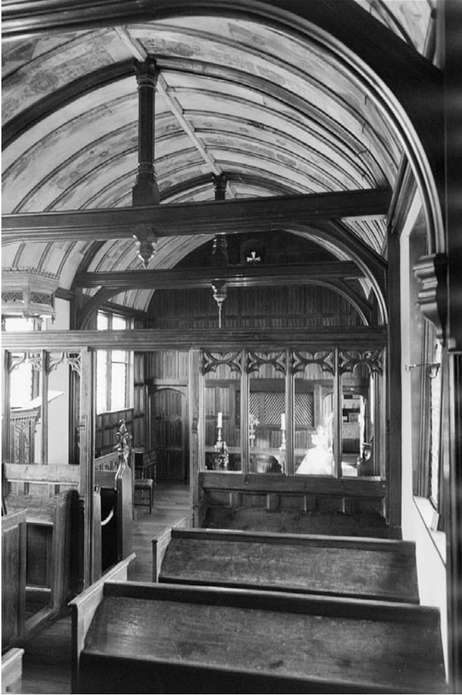
PLATE 149 Ightham Mote: eighteenth-century chapel conversion from guest lodging
