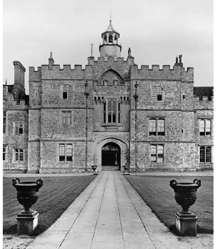
PLATE 150 Knole: Bourchier's Gatehouse from Green Court
