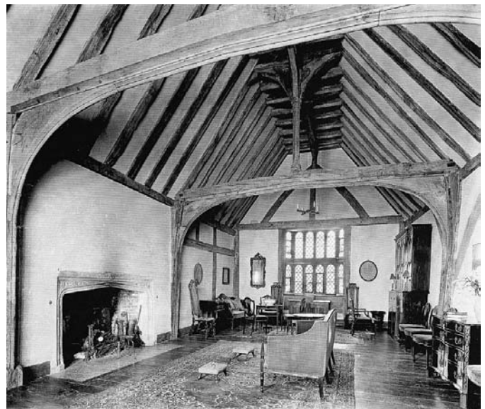
PLATE 139 Great Dixter: first-floor chamber of upper cross wing
