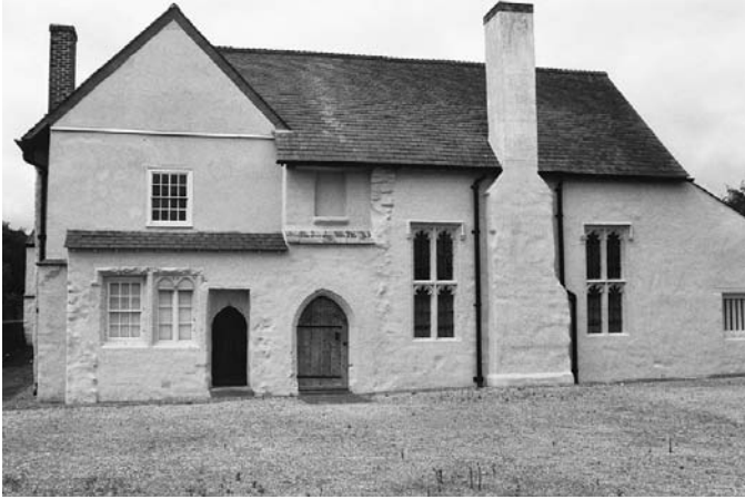
PLATE 210 Bowhill: hall range and parlour from the east
