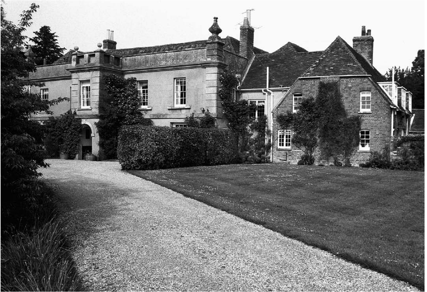
PLATE 182 Wonston Old House: from the south-west
