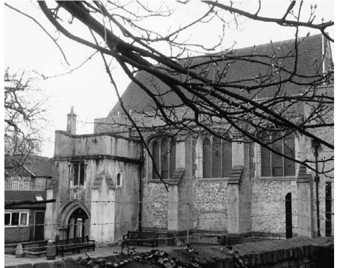
PLATE 133 Croydon Palace: hall from the north-west
