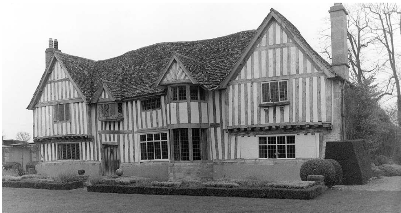
PLATE 84 Yelford Manor: from the south-west
