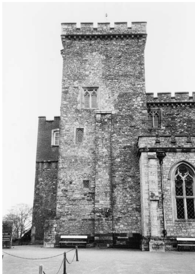
PLATE 267 Powderham Castle: north-west tower from present entry court
