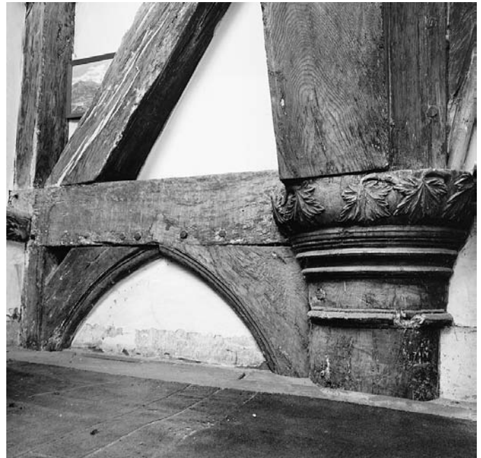
PLATE 157 Nurstead Court: hall aisle column and capital
