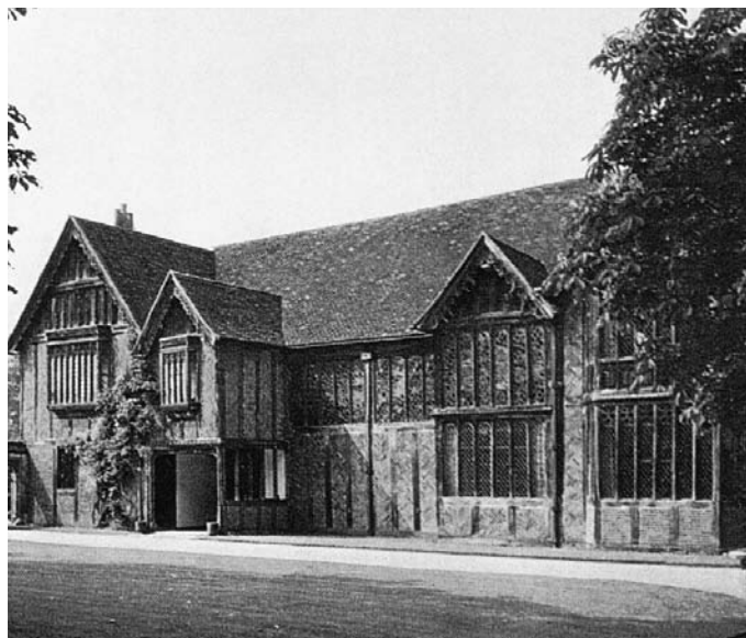
PLATE 54 Ockwells Manor: entrance front from the outer court
