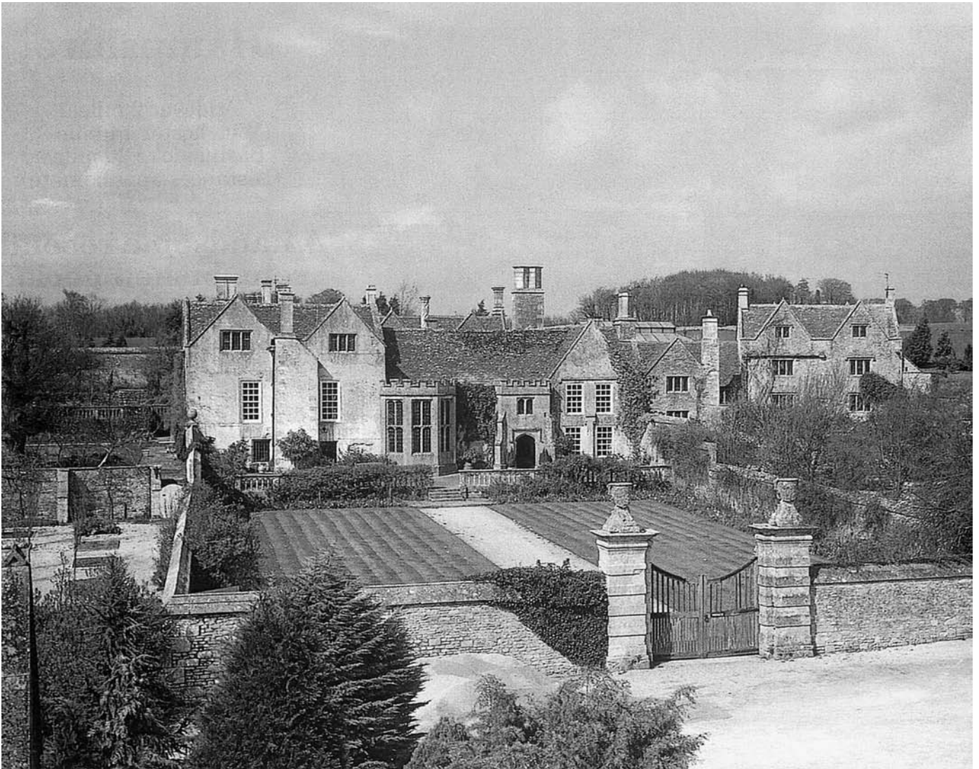
PLATE 208 Hazelbury Manor: from the south
