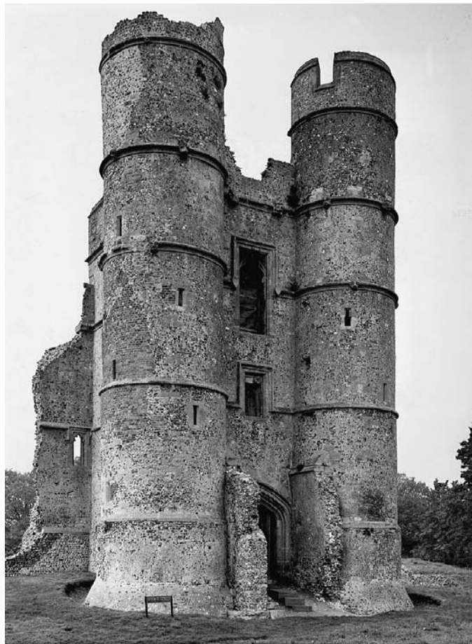
PLATE 34 Donnington Castle: gatehouse from the south-east
