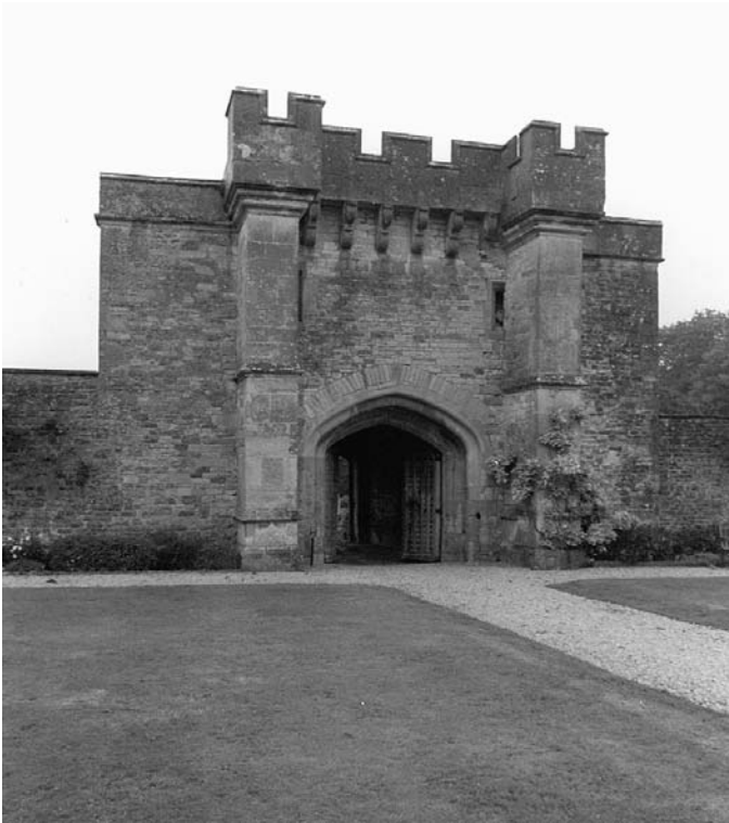
PLATE 198 Newton St Loe Manor: Lord Botreaux's entry gate (early fifteenth century)
