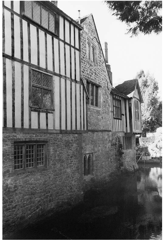
PLATE 148 Ightham Mote: from north-east showing stone chapel block, garderobe chute of additional residential block, and post-medieval framed additions
