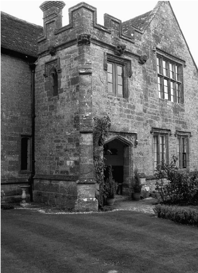
PLATE 186 Childhay Manor: hall porch
