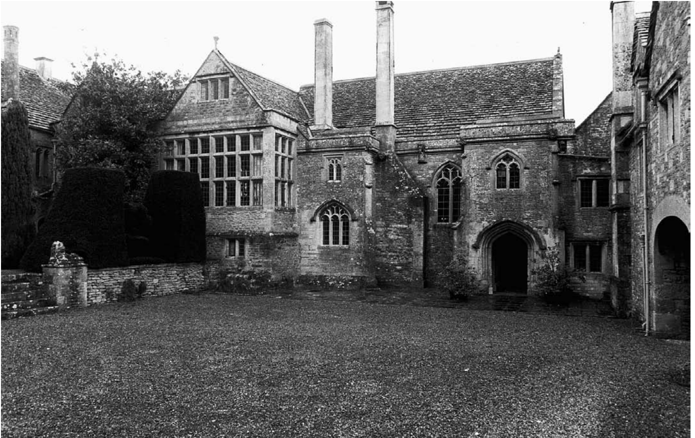
PLATE 276 South Wraxall Manor: hall range from inner court
