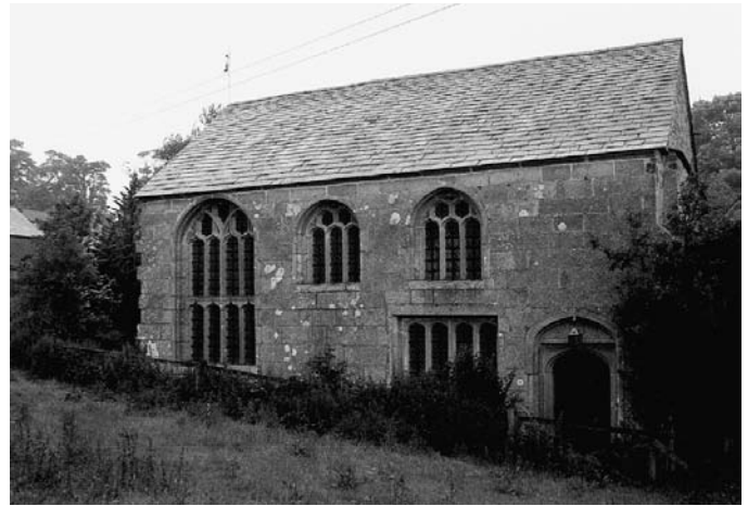
PLATE 284 Trecarrell Manor: hall from the south
