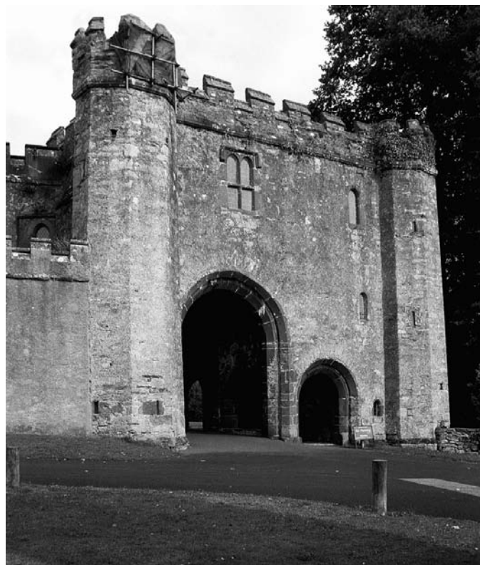
PLATE 283 Torre Abbey: inner gate
