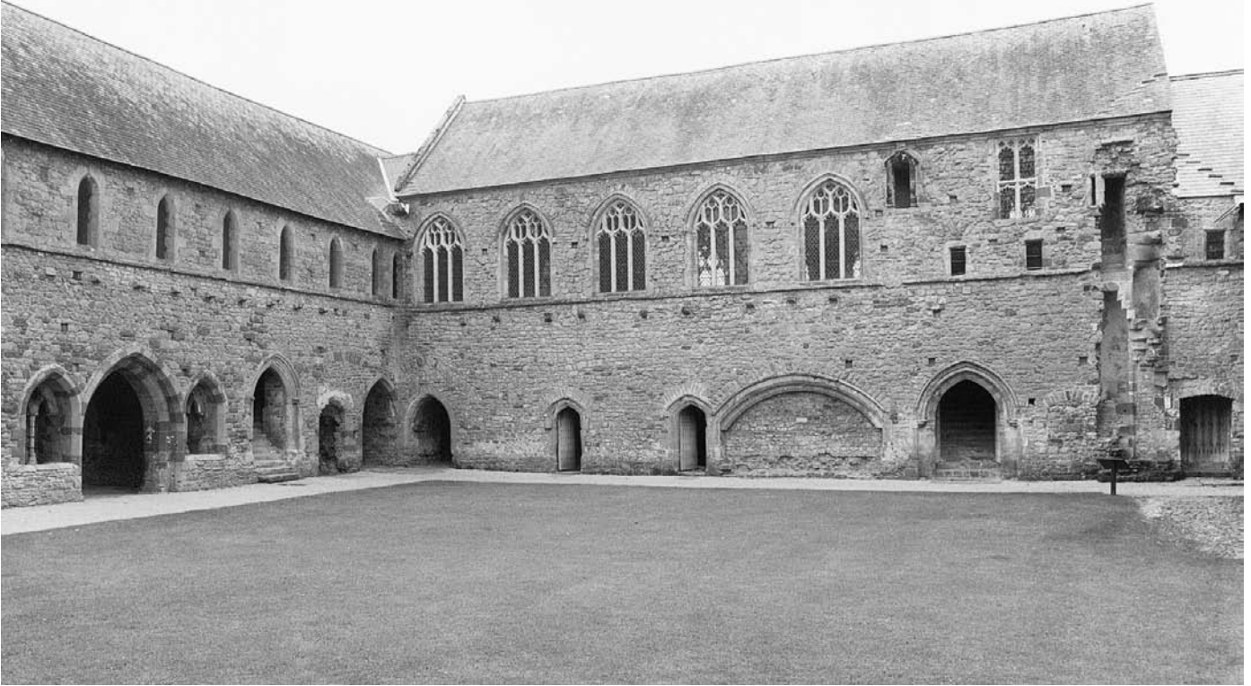
PLATE 218 Cleeve Abbey: dining hall with lodgings below from the cloister, dormitory range
