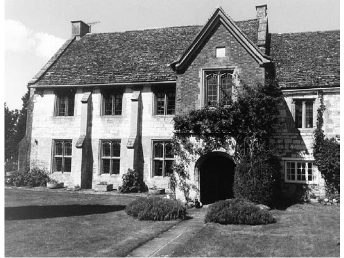
PLATE 18 Ashbury Manor: entry frontage
