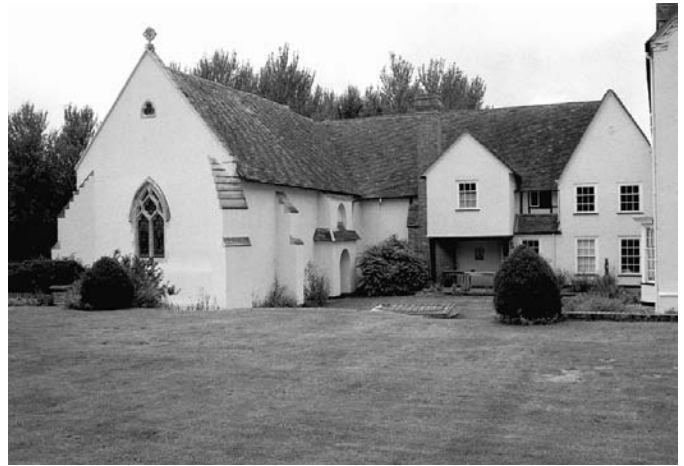
PLATE 3 East Hendred, Hendred House: rear frontage with chapel
