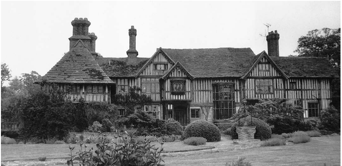
PLATE 132 Crowhurst Place: from the north-west
