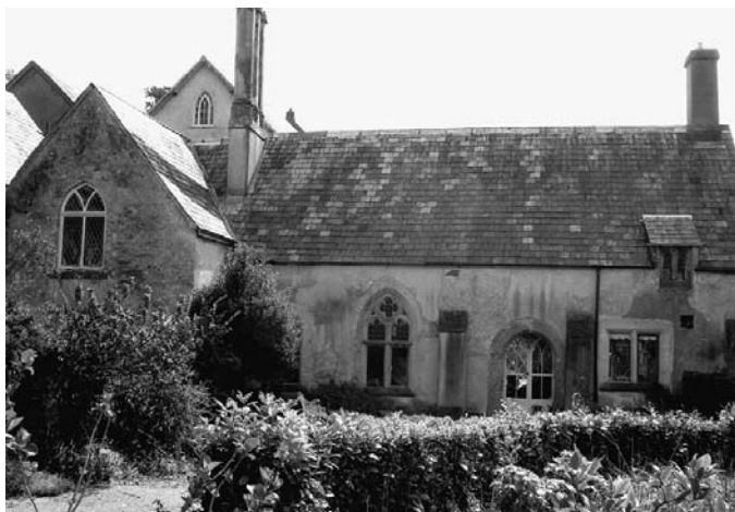
PLATE 251 Lustleigh Old Hall: hall and solar wing from the west
