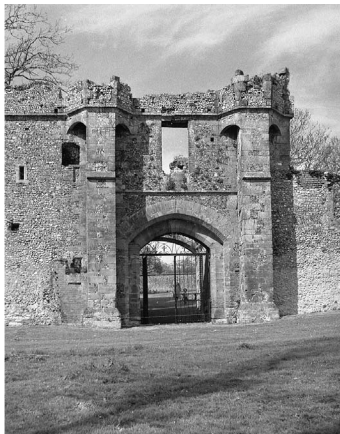
PLATE 140 Halnaker House: gatehouse from the south
