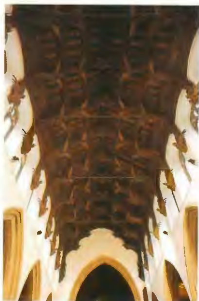
March, St. Wendreda parish church Nave and hammerbeam roof, ca. 1500
