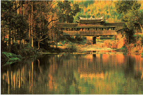
Fig. 8.19 The Yongqing Bridge in Sankui Town. The bridge was constructed in the second year (1797) of the Qing Dynasty Emperor Jiaqing’s reign, and it is a wooden outstretched-arm-style langqiao . It measures 33 m in length and 4.5 m in width and is at a height of eight meters above the water. With a total of twelve rooms, the bridge provides villagers with activity spaces. Source Photograph by Xianjun Zhou, provided by Wenzhou Tourism Bureau
