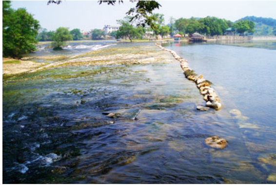
Fig. 8.47 One section of the stone dike of the Lingqu Canal, composed of the large and small balances. In total, the dike measures 500 m in length. Source Photograph by Yingruo Jin, provided by Yaogen Peng
