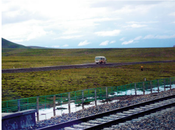
Fig. 6.42 Wildlife corridors flank the railroad tracks, an effort to prevent local animals from crossing the tracks. Source Photograph by Ye Shen
