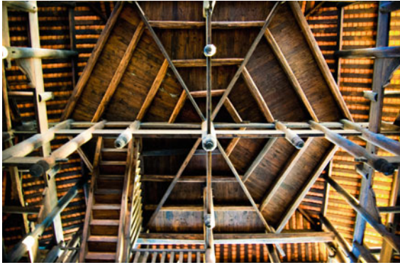
Fig. 8.27 Another pavilion on the bridge has a hexagonal ceiling structure. Source Photograph by Heng Yang, provided by Yi Liu
