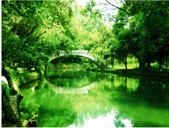
Fig. 8.44 This section of the Lingqu Canal was built with an embankment, where trees grow densely along the riverbanks. Source Photograph by Lida Fu, provided by Ming Jiang
