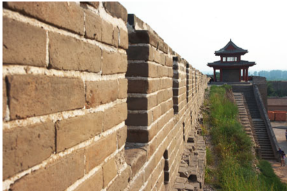
Fig. 5.25 The main body of the city wall was made from tamped earth; critical elements, such as the crenellations, were surfaced with brick. The city wall is crenellated with square corners that extend out over the city wall's four corners and outer edge. Source Photograph by Fan Yin
