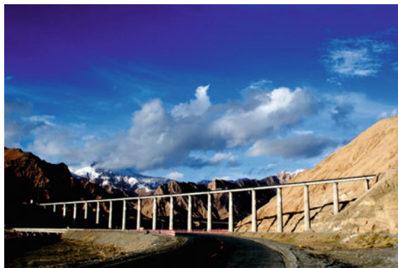
Fig. 6.48 This section of the Qinghai-Tibet railway crosses a large valley by way of the Sancha River Bridge. There are a number of diverse geological environments along the railway. One bridge, over 690 m in length and 54 m above the bottom of the valley, was a massive construction project of the tallest railroad bridge along the Qinghai-Tibet Railway. Source Photograph by Zhiguo Zheng, provided by Jiali Zhou
