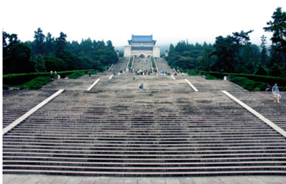
Fig. 6.5 The procession path to the mausoleum is 375 m in length and 40 m in width and serves as the complex's central axis. When walking up the stairs, people may feel as if they're gradually drawing closer to Sun Yat-sen's soul and spirit. From the Stele Pavilion to Sacrificial Hall, there are eight flights of steps, with a landing platform after each flight. There are 392 steps, which is a metaphor for the nearly three hundred and ninety-two million people in the Chinese population at that time. Source Photograph by Mu Yuan, provided by Piyan Jiang
