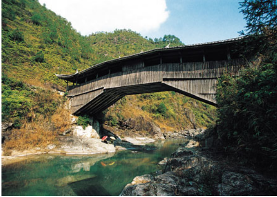
Fig. 8.9 The Santiao Bridge is the oldest existing wooden-arch-style langqiao in Taishun County. The bridge was first built during the Song Dynasty Shaoxing period (1131–1162) and later rebuilt during the Qing Dynasty Emperor Daoguang’s reign (1821–1850). Stretching across the Hengxi Creek, the bridge measures 32 m in length, 3.96 m in width and 9.55 m in height. Source Photograph by Xianjun Zhou, provided by Wenzhou Tourism Bureau
