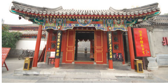
Fig. 5.32 The entrance to Huguang Guild Hall. Located to the southwest of the Hufang Bridge outside the Xuanwu Gate, the hall is adjacent to a street to the north and a canal to the east and south. Source Photograph by Fan Yin
