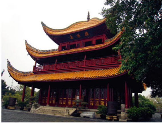
Fig. 3.20 Close view of the facade of the Yueyang Tower, which faces Dongting Lake. Helmet-style roofs were not commonly used in ancient Chinese architecture; the Yueyang Tower is one of a few examples of the style. The 12 upturned eaves, graceful and nimble, contrast the prismatic form of the tower's body. Source Photograph by Yuyu Wang. Note Upturned eave is a type of eave in traditional Chinese architecture that builds the eaves upturned with special treatment.
