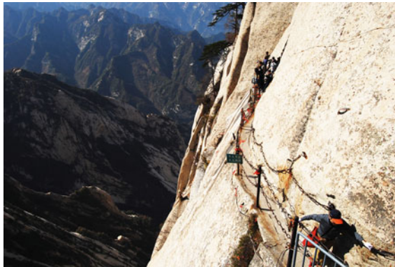
Fig. 6.12 The upper section of the Changkong Trail is 20 m in length and 7 m in width and was hewed out of a vertical mountain to connect the stone archway at the Nantian Gate with the western side of the Chaoyuan Cave. Source Photograph by Xinting Zhou, provided by Chunjiang Wu
