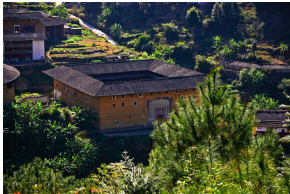
Fig. 9.8 The Chuxi earthen buildings in Yongding County, Fujian. The building in the photo has a simple structure and a square floor plan. This type of earthen building is widely found in Yongding, where there are more square buildings than circular ones. Source Photograph by Bihu Wu
