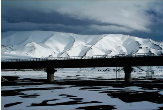
Fig. 6.52 In the unstable permafrost zone, the railroad runs above the ground on a viaduct that isolates the tracks from the volatile surface below. Source Photograph by Zhiguo Zheng, provided by Jiali Zhou
