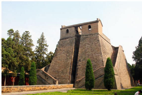
Fig. 2.27 Built in 1276, the Gaocheng Astronomical Observatory in Dengfeng is currently the oldest observatory in China. Source Photograph by Bihu Wu
