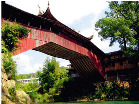
Fig. 8.9 The Santiao Bridge is the oldest existing wooden-arch-style langqiao in Taishun County. The bridge was first built during the Song Dynasty Shaoxing period (1131–1162) and later rebuilt during the Qing Dynasty Emperor Daoguang’s reign (1821–1850). Stretching across the Hengxi Creek, the bridge measures 32 m in length, 3.96 m in width and 9.55 m in height. Source Photograph by Xianjun Zhou, provided by Wenzhou Tourism Bureau
