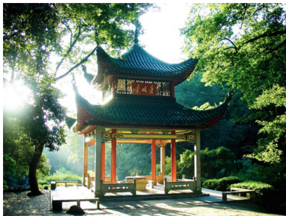
Fig. 5.7 The pavilion is covered with green glazed tiles. An outer square of four granite columns and an inner square of four wood columns that are coated in red lacquer support the structure. Source Photograph by Lixin Jian, provided by Xiaobing Zhang
