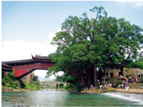
Fig. 8.18 The Beijian Bridge in Xiaqiao Village, Sixi Town. The bridge is topped with upturned eaves, and a pavilion rises in the center of it. Red siding boards protect the arch skeleton and beam-column. Source Photograph by Xinmin Huang
