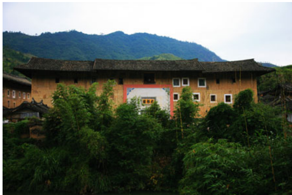
Fig. 9.9 The Guangyu Building in Yongding County, Fujian. The Guangyu Building, built in 1775, has three stories and total 102 rooms. It is the oldest and best-preserved earthen building in Hongkeng Village. Source Photograph by Wenkui Wang, provided by Lin Yan
