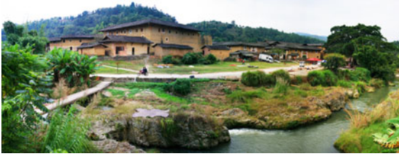
Fig. 9.14 An earthen building complex in Yongding County, Fujian. The complex does not stand out from its surrounding environment due to the use of loess as the major material in the construction. The thick exterior walls support the building’s weight and provide protection from intruders. The walls also create a microclimate of constant humidity and temperature. Source Photograph by Wenkui Wang, provided by Lin Yan
