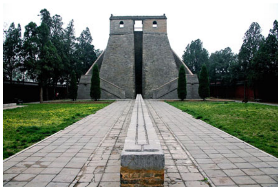
Fig. 2.33 Northern facade of the Gaocheng Astronomical Observatory platform structure and the heaven-measuring ruler. There is a groove in the middle of the northern wall and a stone tablet called “the heaven-measuring ruler” under the northern wall, perpendicular to the groove. This photograph also illustrates that the heaven-measuring ruler is built of bluestone over a brick foundation. On it, the draining groove in the north and the twin channels were designed to connect to the pouring groove. Source Photograph by Songtao Gong, provided by Jun Hu
