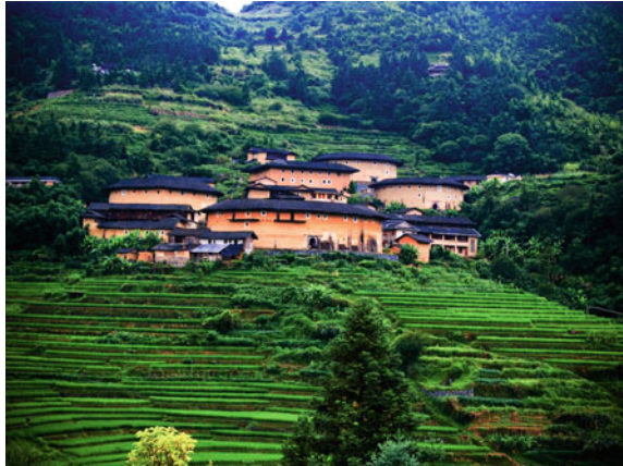
Fig. 9.16 Earthen buildings built into the mountains. Few openings in the exterior walls occur only in the upper sections of the walls. The buildings resemble fortresses in the mountain and are easy to hold but difficult to attack. Source Photograph by Mu Yuan, provided by Piyan Jiang
