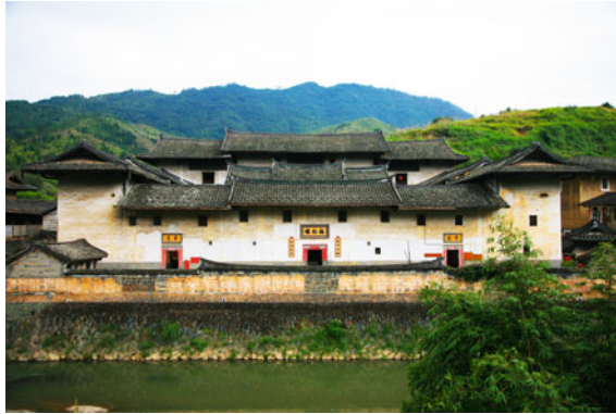
Fig. 9.12 The Fuyu Building in Yongding County, Fujian. The Fuyu Building, built in 1880, is a mansion-like earthen building along a central axis. The back of it is higher than the front, and two side rooms complete the courtyard enclosure. This layout utilizes height variance to establish a distinct hierarchical order. There are three gates in front of the building. The main building is separated from the side rooms by inner doors. The entire building complex consists of three sub-complexes. Source Photograph by Wenkui Wang, provided by Lin Yan
