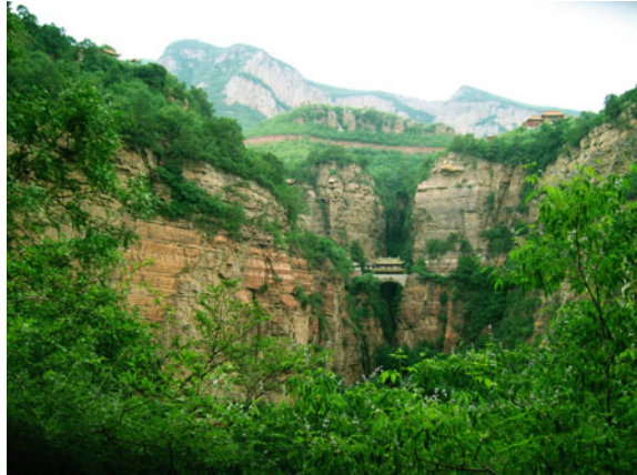
Fig. 8.1 Bridge-Tower Hall hangs in the chasm between two cliffs on Mount Cangyan, a mountain in Jingxing County, Hebei Province. The Pteroceltis that grows on the stone causes the mountain to appear as if composed of dark green stone. Source Photograph by Xiangnan Zhang, provided by Ming Jiang
