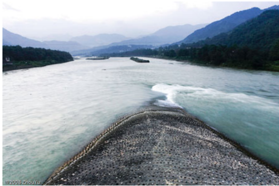
Fig. 8.36 View of the Dujiangyan Irrigation System from the Qinyan Tower. The Fish Mouth Levee divides the Min River into inner and outer branches. As shown in the photograph, the waterway in the foreground is the outer branch, and the waterway in the background is the inner branch. Source Photograph by Mu Yuan, provided by Piyan Jiang
