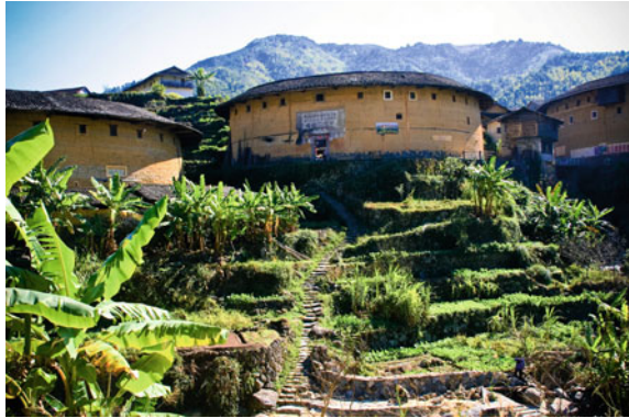
Fig. 9.7 A circular earthen building in Yongding County, Fujian. Usually, the first and second floors of an earthen building do not have windows, but the windows of the third and fourth floors can open. Source Photograph by Bihu Wu
