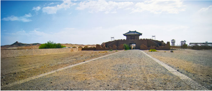
Fig. 3.5 From the secondary exit of the Yangguan Pass Museum, the fire beacon can be seen in the distance. Source Photograph by Fang Wang
