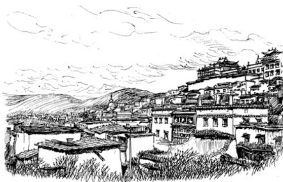
Fig. 2.8 Side view of the Ganden Sumtseling Monastery. The huge Sumtseling Monastery is built on a slope. Each level of buildings is stacked upon the previous level. Source Drawing by Kun Gao
