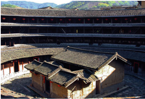
Fig. 9.15 The Chuxi earthen building in Yongding County, Fujian. This earthen building has three rings. The first ring has four stories, whereas the other two have only one story. Important ceremonies, such as weddings and funerals, are held in the ancestor’s hall at the center of the complex. Kitchens and storage rooms are located on the first and second stories; the third and fourth stories contain the residence. Source Photograph by Bihu Wu
