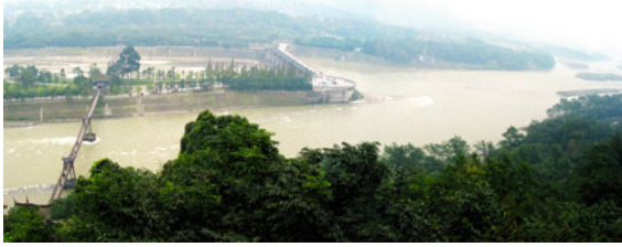
Fig. 8.36 View of the Dujiangyan Irrigation System from the Qinyan Tower. The Fish Mouth Levee divides the Min River into inner and outer branches. As shown in the photograph, the waterway in the foreground is the outer branch, and the waterway in the background is the inner branch. Source Photograph by Mu Yuan, provided by Piyan Jiang
