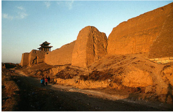
Fig. 5.24 The fortress wall of Cockcrow Postal Town, tamped with soil and gravel, is well preserved to this day. Source Photograph by Zhi Ou, provided by Ming Jiang
