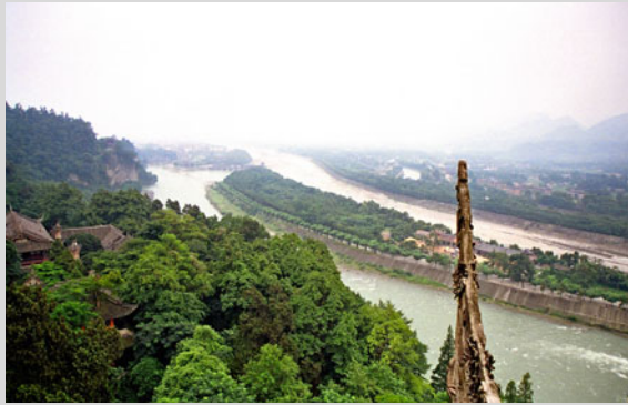
Fig. 8.35 The Dujiangyan Irrigation System from the Qinyan Tower. In this image, water flows downstream toward the Fish Mouth Levee, which divides the river into two branches. On the left is the inner branch and concave bank; on the right is the outer branch and convex bank. Source Photograph by Lu Fan
