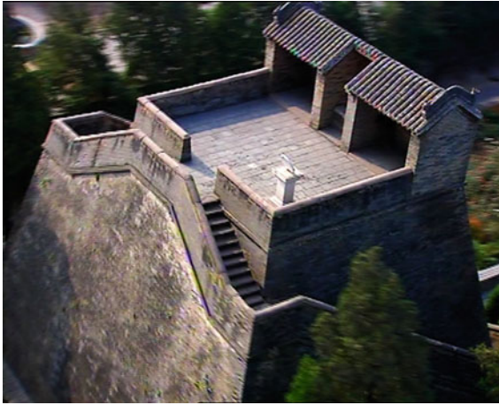
Fig. 2.35 Viewing the observatory from the south, two small rooms that were used for storing observation equipment are visible on the east and west sides of the platform. Source Photograph by Songtao Gong, provided by Jun Hu
