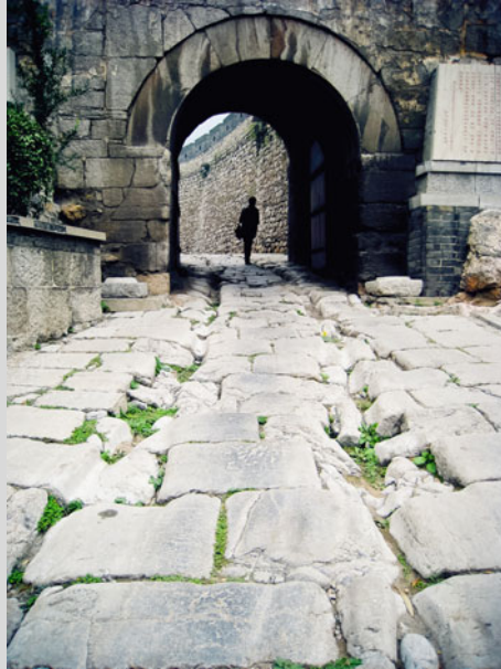
Fig. 9.28 Located on the west side of the Taihang Mountains, the Guguan Pass is a critical transportation node through which one could reach the other side of the mountain. Ruts in the stone road illustrate the long history and heavy use of the postal road. Source Photograph by Fang Wang
