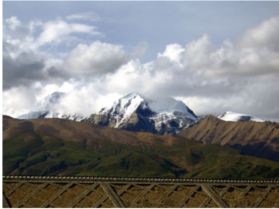
Fig. 6.46 A section of the railroad in the territory of Dangxiong, Lhasa, Tibet. This photograph was taken in August 2005, before the completion of the railroad, with Mount Nyainqentanglha in the background. Source Photograph by Wangmu
