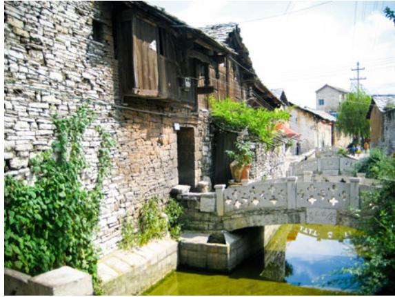
Fig. 9.22 Tianlong Tunpu Village. The omnipresent stone buildings are ostensibly simple, but retain an aroma of Jiangnan in concealing details. Source Photograph by Xinmin Huang
