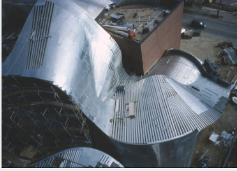
Gehry Partners, Peter B Lewis Building, Weatherhead School of Management, Case Western Reserve University, Cleveland, Ohio, 2002
