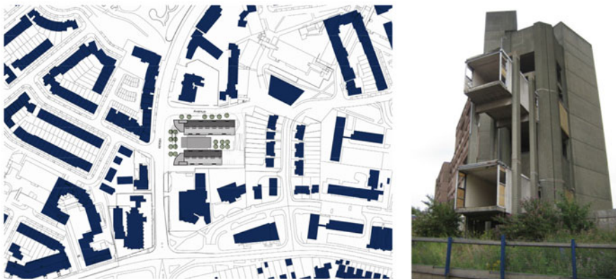
Site plan for the Hillside Hub/Remains of the flying bridges connecting one of the 1970s precast concrete slab blocks
