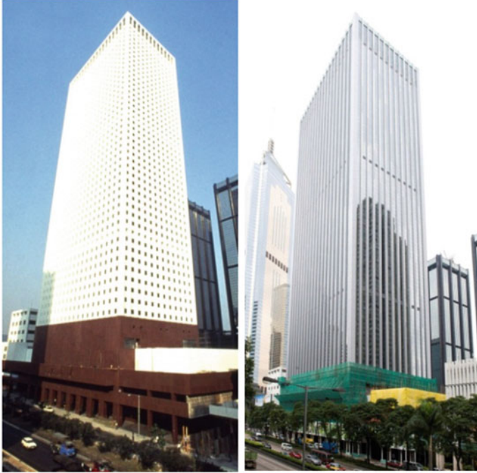
Fig. 6 China Resources Building green retrofit is the first building renovation project in Hong Kong that achieved LEED® Core and Shell Gold rating. Key features include reusing the existing structural frame, adopting high-performance façade, increasing indoor ventilation rate and upgrading the electrical and mechanical equipment ( left and right: building before and after renovation ) (©Arup)
