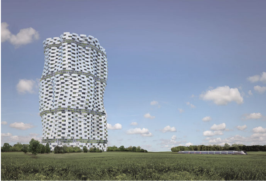
Fig. 7 The Vertical Village contains four giant continuous public double-rings with a combined length of one kilometre, which are located not—as usual—on the lowest level, but rather spread out through the entire height of the structure, creating heterogeneous city structures (Image by Gramazio Kohler Architects, Zurich)
