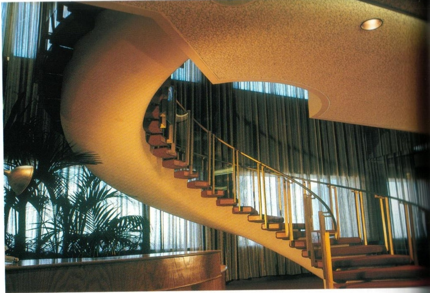
Spiral stair at the law offices of Lewis and Roca—plasticity of form is natural to reinforced concrete.
