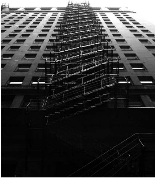
Fig. 8: Façade as Exit-Architecture: A typical fire escape, New York.
