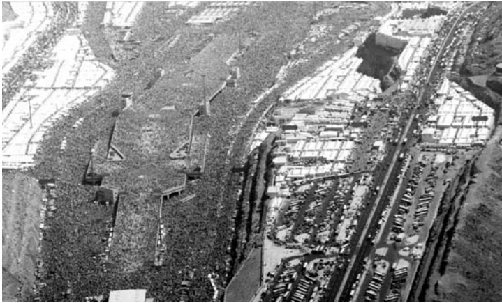
Fig. 18: The world's most dangerous work of architecture: The first Jamarat Bridge, constructed 1975, demolished in 2006.
