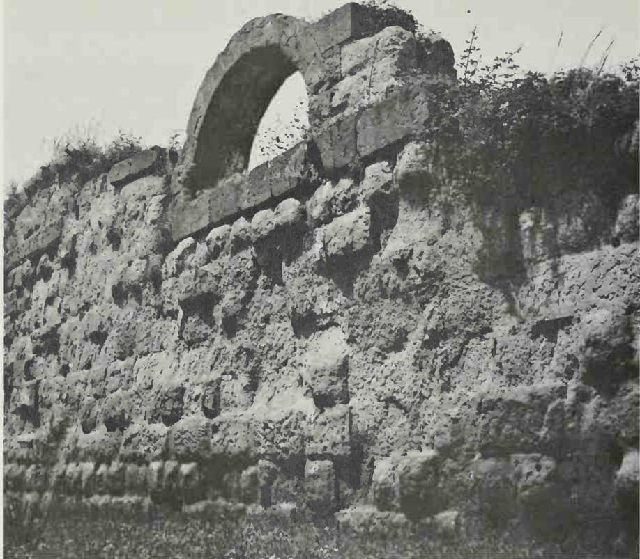
170. Rome, 'Servian Wall' at the Aventine, begun 378 B.C., rebuilt with an arch for catapults in 87 B.C.
