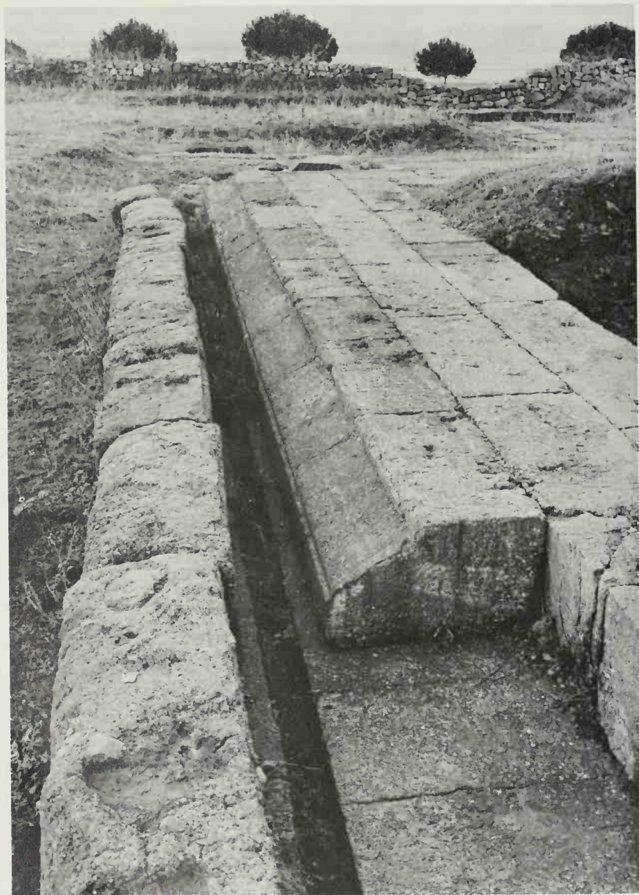
46. Gabii, temple, late third century B.C., podium with benches for statues along the sides and back
