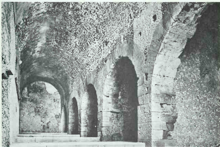
182. Ferentinum (Ferentino), Via Latina, market hall, c. 100 B.C.
