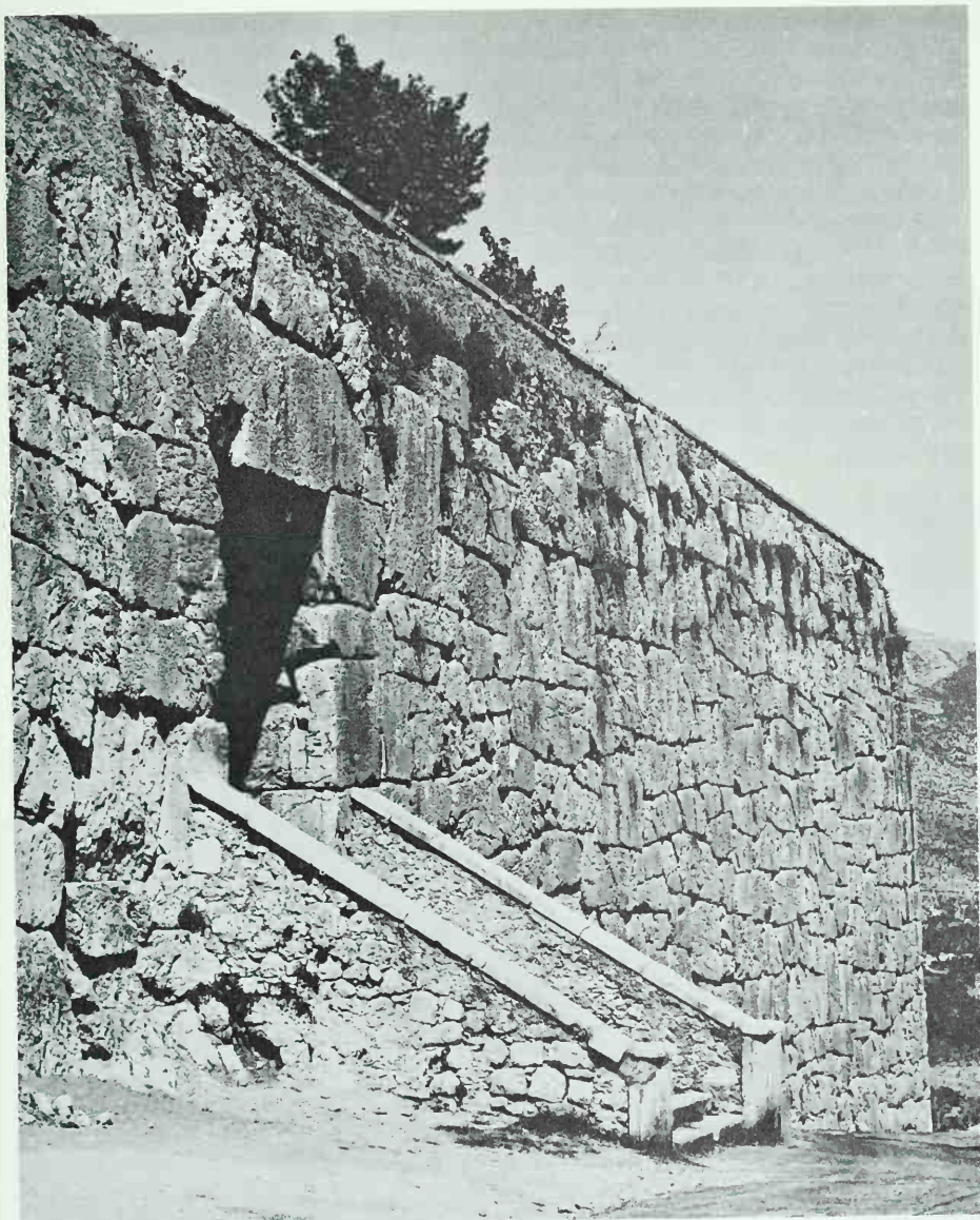
115. Alatrium (Alatri), terrace wall, third century B.C.
