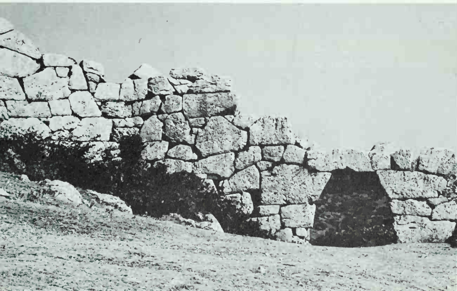
110. Signia (Segni), gate in the wall, fourth century B.C. (?)
