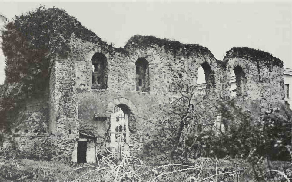
137. Rome, Porticus Aemilia, begun 193 and restored 174 B.C.(?), before the modern buildings on the site, showing the alternating arches on the first and second floors
