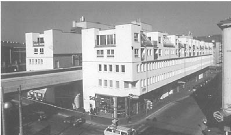
Residential and office development (enclosing a subway terminal track for turnback operation), Vienna (1997) © Harald Schoenfellinger, Vienna. Photo Celeste M. Williams and Dietmar E. Froehlich
