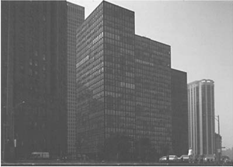
860–880 Lake Shore Drive Apartments (1948–51), designed by Ludwig Mies van der Rohe, Chicago
