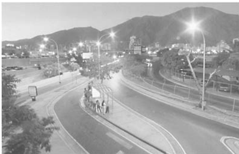
Overview of Section of Avenida Bolívar, Caracas, Venezuela (1996)
