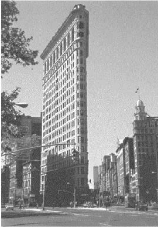
D.H.Burnham and Company, Flatiron Building, 1900–03, New York
