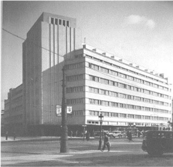
The ARO (Asigurarea Româneasca) Building, Bucharest, Romania, designed by Horia Creanga (1931)
