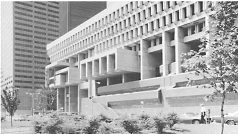
Boston City Hall, designed by Kallmann, McKinnell and Knowles (1968)
