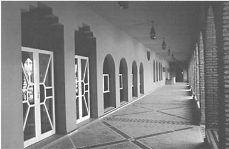
Regional Military Hospital (1982), Marrakesh, designed by Charles Boccaro
