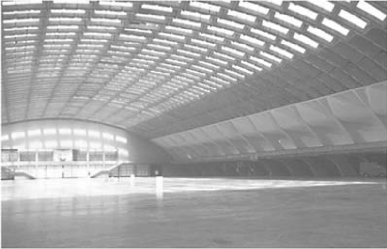
Exhibition Hall, Turin, Italy, interior longitudinal view, designed by Pier Luigi Nervi (1949)
