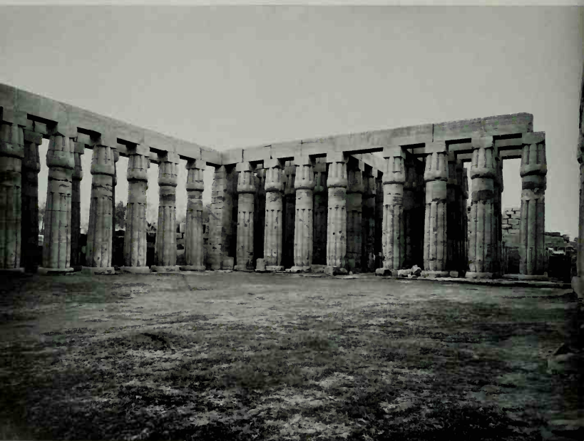
160 Luxor, Temple of Amon-Mut-Khons. The great court of King Amenophis III and porch of the temple house, seen from the north
