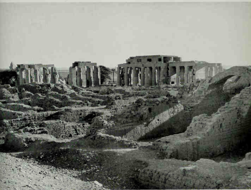
233 Thebes. Funerary temple of King Ramesses II, seen from the north. In the foreground the ruins of the store-rooms
