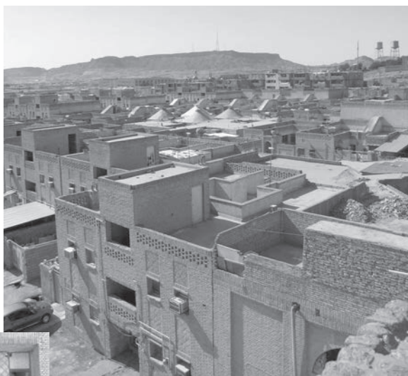
Figure 4.15 Parapet walls surround the rooftops of Shūshtar New Town and provide shade for interior courtyards. Courtesy of Aga Khan Trust for Culture, Geneva
