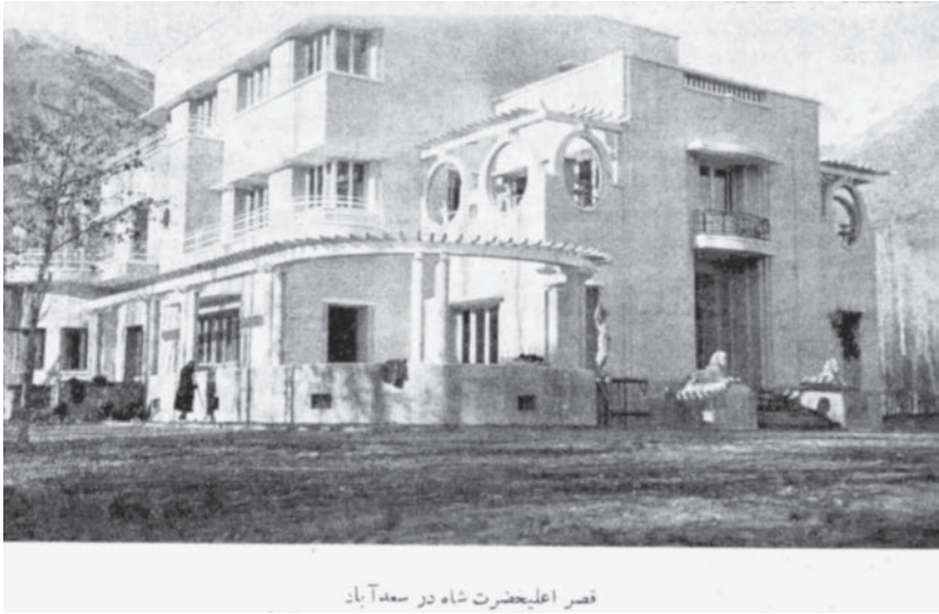
Figure 2.10 View of a palace built by Vartan Hovansian in the Sa'd ābād Royal Complex, Ārshūtiqt (Architect), Murdād/Shahrīvar 1325/ August/September 1946, vol. 1, no. 3, p. 4. Courtesy of the Library of the Parliament of the Islamic Republic of Iran, Tehran
