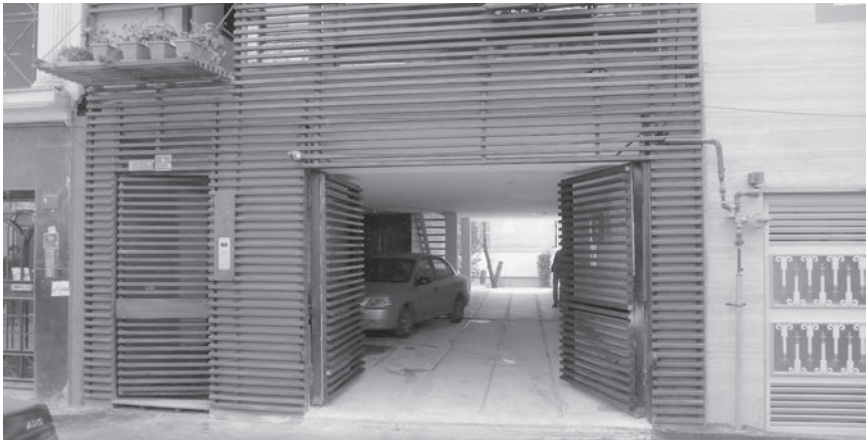
Figure 6.2 Dowlat II Residential Complex by Alireza Shirafati of Arsh Design Studio, 2007. View of the façade with opened wooden lattice screens. Photographs by Arsh Design Studio. Courtesy of Aga Khan Trust for Culture, Geneva
