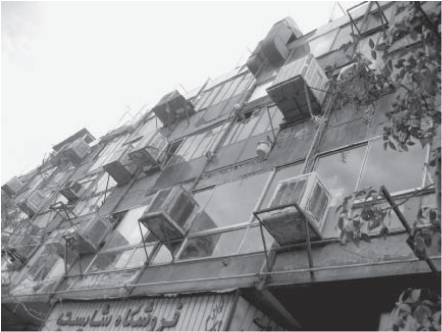
Figure 0.2 Building façade in central Tehran, furnished with suspended air conditioners. Photograph by the author, 2007
