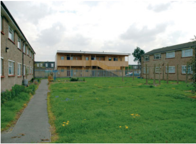
The new block on Adelaide Road has been shoehorned into a small space overlooking one of the unloved public green spaces that are scattered throughout the estate. The echoes of Adelaide Court are clear, but care in the site planning is missing, with the stairs to the upper level abutting a harsh metal fence.
