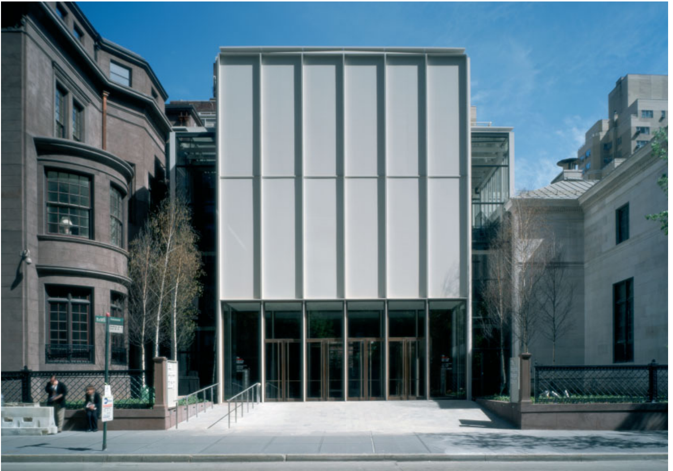
Piano's new Madison Avenue facade of the Morgan Library complex juxtaposes a rectangular white-painted steel box to the articulated stone facades of the older Morgan buildings on either side, offering a sharp contrast between old and new. The addition, however, is visible only as the visitor approaches. From just a block away, only the historic buildings can be seen.
