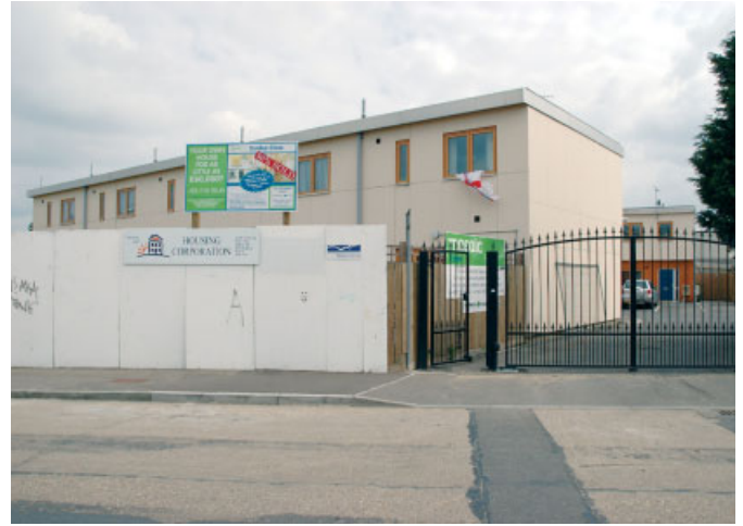
The assisted self-build scheme of 2003 was to help young people into their first homes. The scheme was 100 per cent rental with no equity for the residents. Having gained planning approval for the remaining sites, the end-user base has changed, along with the quality. These units are now being presented as a shared-ownership scheme by the housing association.
