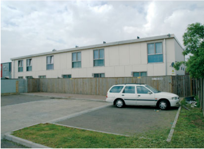
The original finish to the building was unpainted grey cement board, with individual variations that would have become more explicit with weathering. The housing association has taken the unfortunate decision to paint over this boarding, not only adding to the maintenance costs of the building, but actually making it stand out from its neighbours more than was previously the case.
