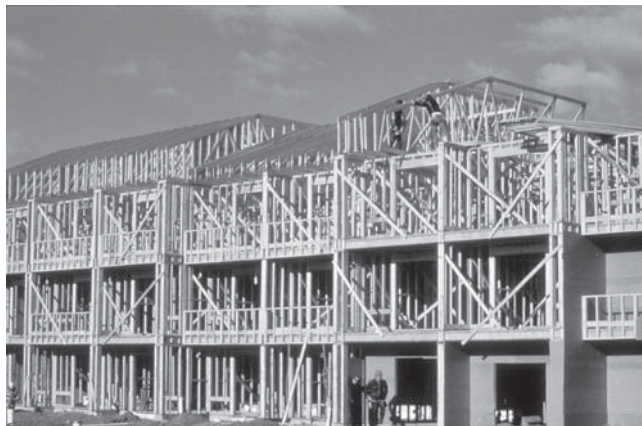
Figure 1.1 Multi-story wood-frame buildings. (Photo Courtesy of Southern Pine Council)
