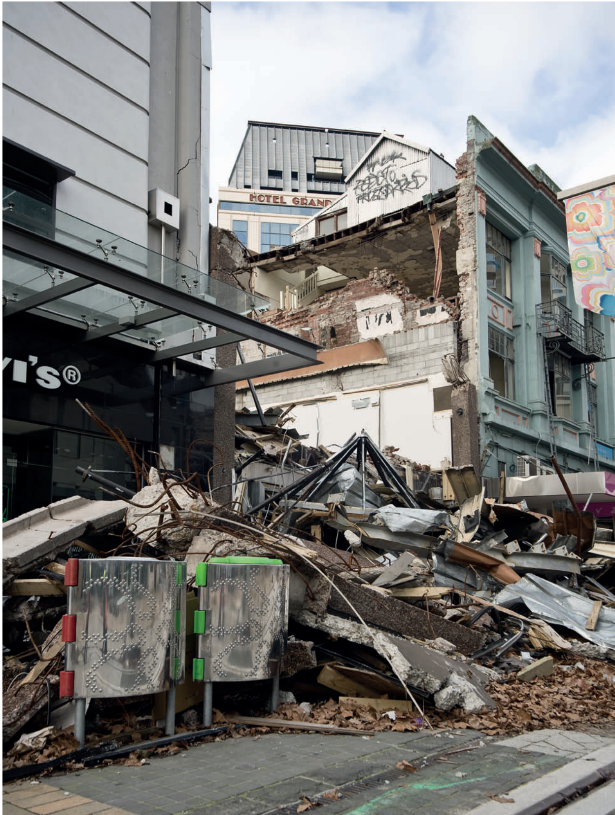
Figure 2.11 Christchurch, NZ: after the earthquake. Christchurch High Street – by the city mall: before the 2011 earthquake this was the site of an innovative primary school, Discovery 1, located in underused space above a department store and its sister secondary school, Unlimited Paenga Tawhiti, also located above a nearby block of shops
