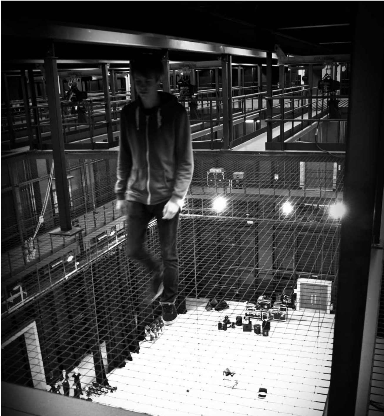
Figure 6.8 Backstage Centre, Purfleet, UK: tension wire grid above the sound stage
