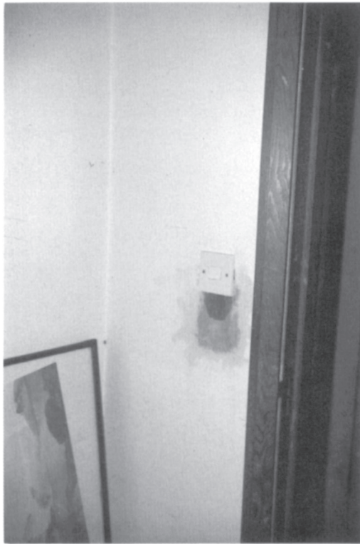
Plate 23. Remedial wood preservation problems. If some organic solvent formulations are applied too generously, solvent vapours are absorbed by PVC cables, causing bleeding of the plasticizer which can stain ceilings and walls but also cause arcing and short circuits.
