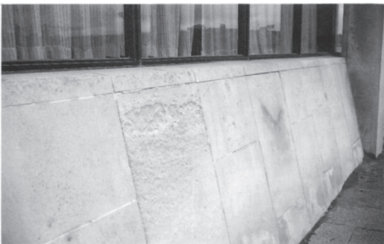
Plate 4. Portland limestone erosion in Blackpool. Erosion of isolated cladding panels was due to pore size variation; the durable panels were predominantly macroporous but the eroded panels were microporous.
