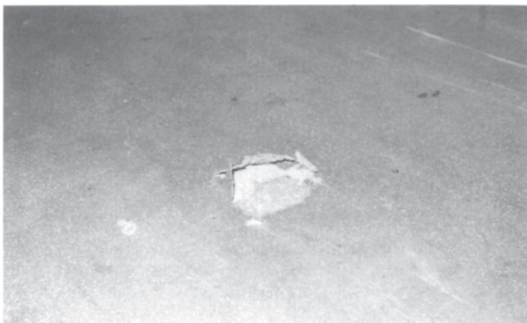
Plate 38. Paint deterioration in a marine environment. The electrophoretic acrylic coating on these new aluminium window frames was damaged by alkali attack; sea spray reacted with the lime in the adjacent new rendering to form sodium hydroxide.
