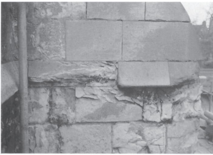
Plate 5. Stone incompatibility at Lincoln Cathedral. The stone repair was very durable but also very porous, allowing rainwater to accumulate on the original stone beneath and cause frost spalling during freezing conditions. Similar fracture and erosion damage can be caused by absorption of limestone washings by a sandstone, or even magnesian limestone washings by a calcareous limestone.
