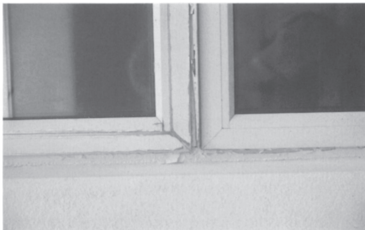
Plate 37. Render fractures. The fractures in this render are caused by sulphate attack expansion of the cement in the mortar of the supporting brickwork; the bricks were known to contain excessive sulphate and sulphate resisting cement was specified but not used.
