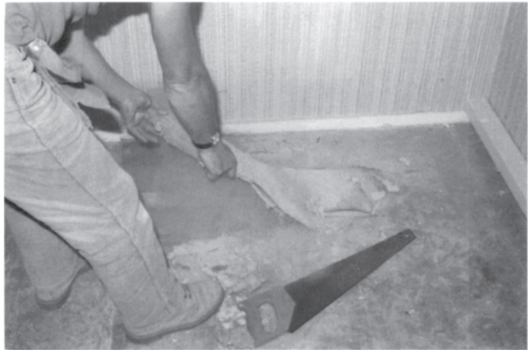
Plate 11. Powder Post beetle damage to a plywood floor. Powder Post Lyctus beetle attacks only fresh sapwood of certain hardwoods but it can cause complete destruction.
