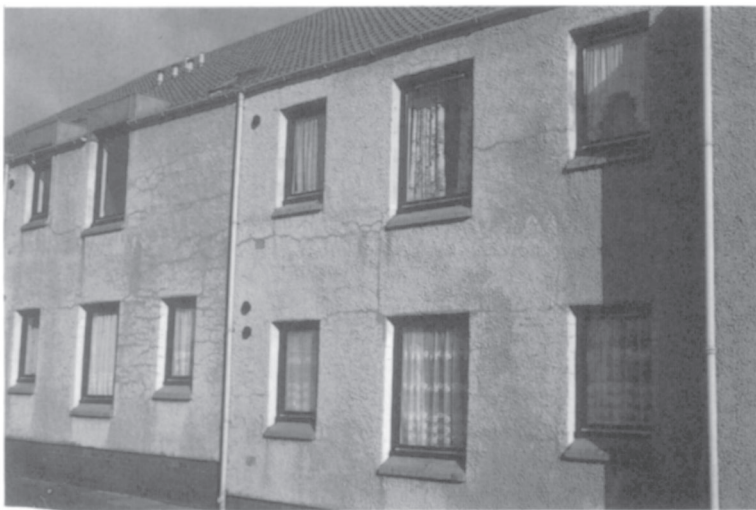
Plate 37. Render fractures. The fractures in this render are caused by sulphate attack expansion of the cement in the mortar of the supporting brickwork; the bricks were known to contain excessive sulphate and sulphate resisting cement was specified but not used.
