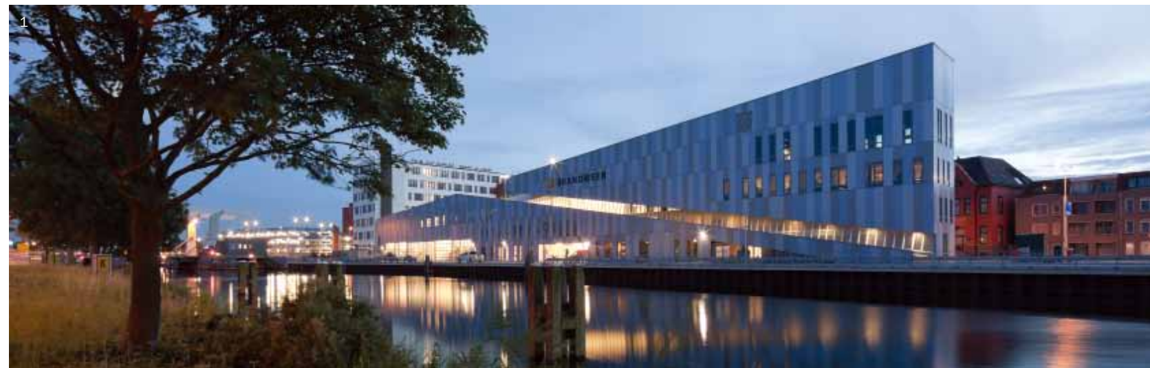
2, 3. The visible strong slanting line on the front and back of the building forms the access ramp for the parking on the roof
