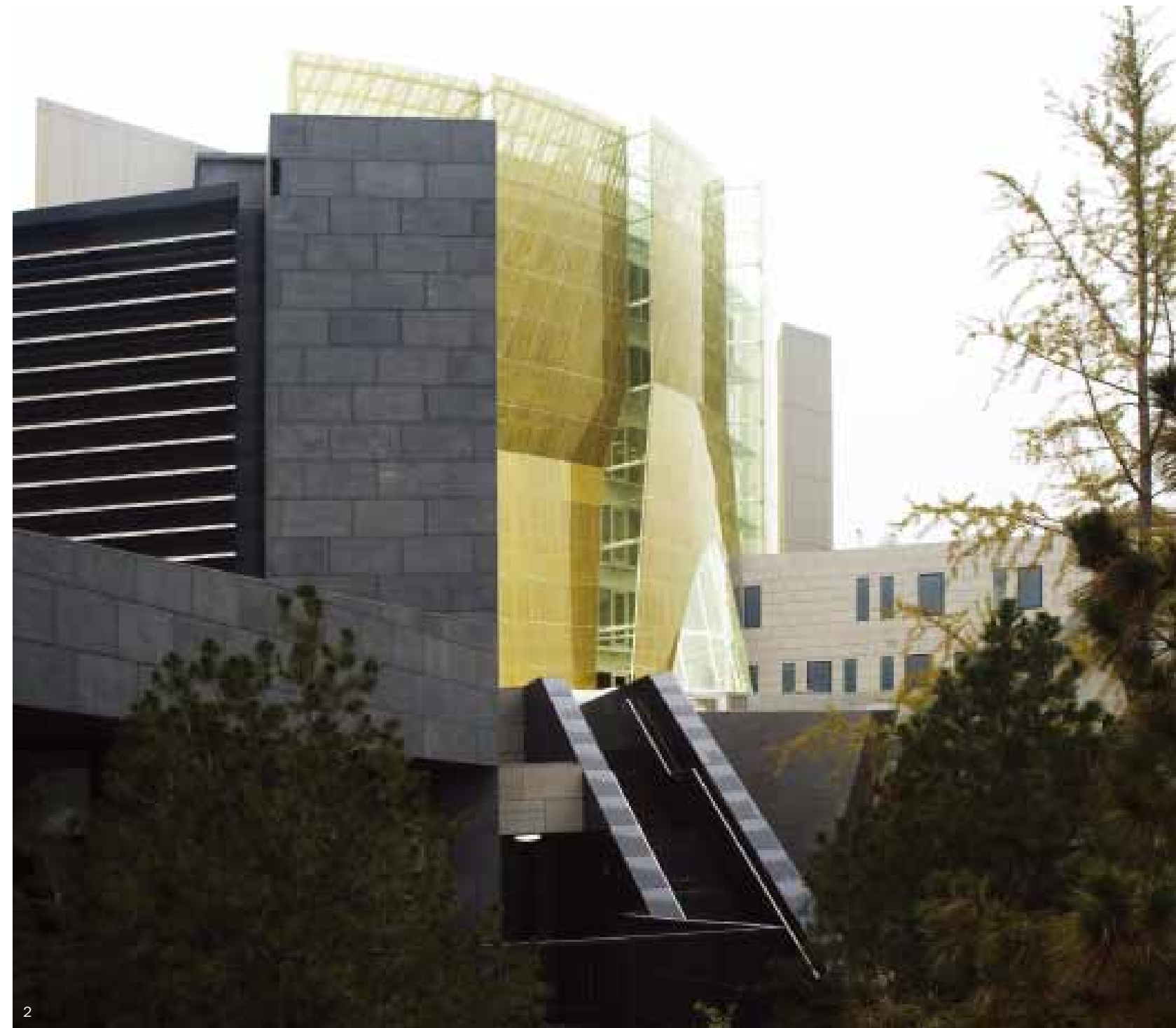
1. Details of the west façade of the building 2. The stone was chosen to save the energy
