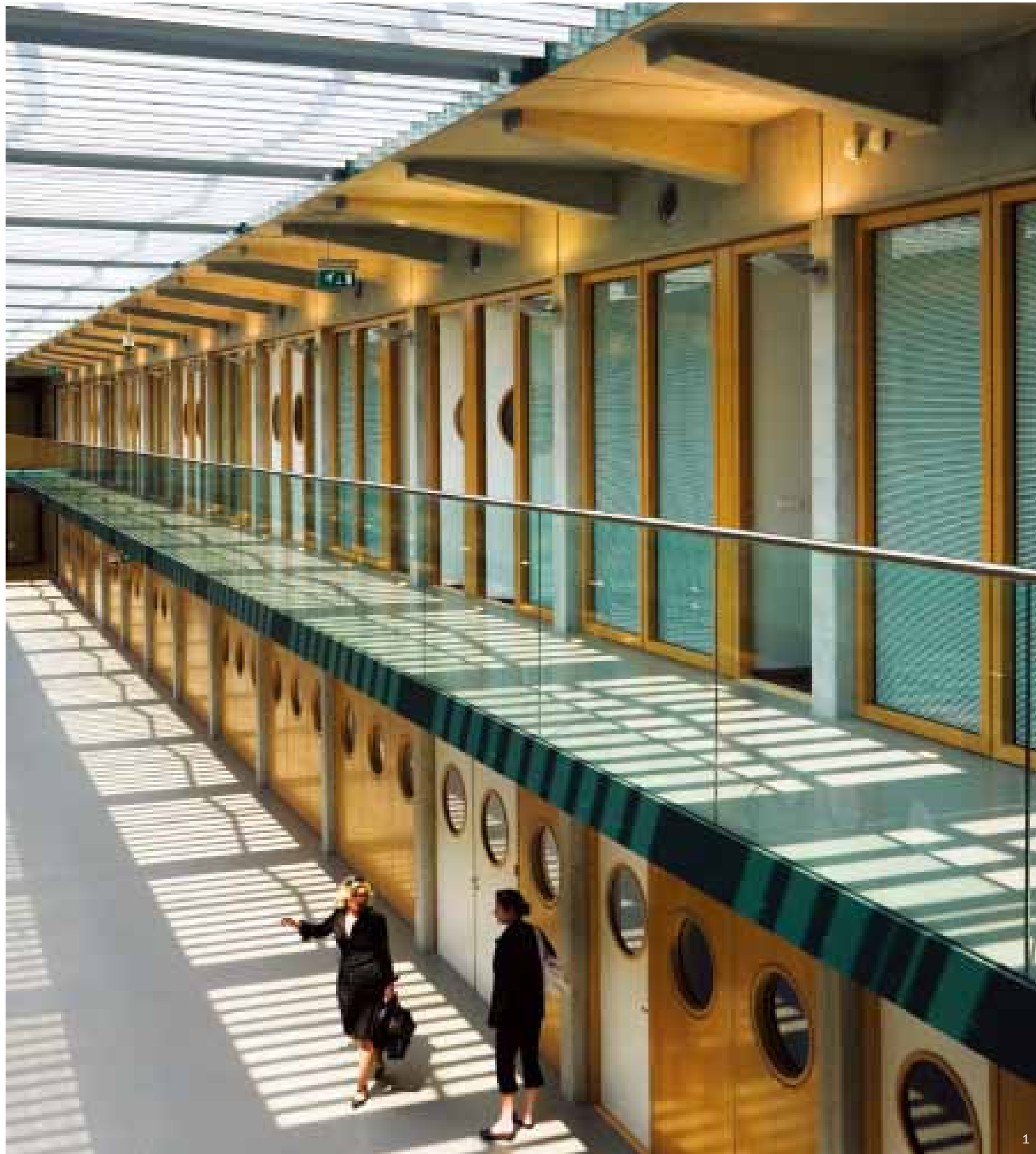
1. Two floors and a central 'street' are interconnected by means of double-height atriums 2, 3. The structure of the multi-purpose building comprises a prefab concrete frame of two floor elements, i.e. columns and beams
