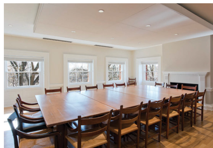
Below. A typical teaching space in McDowell, this classroom features a brick fireplace and a new dropped ceiling with Decoustics acoustical tiles.
