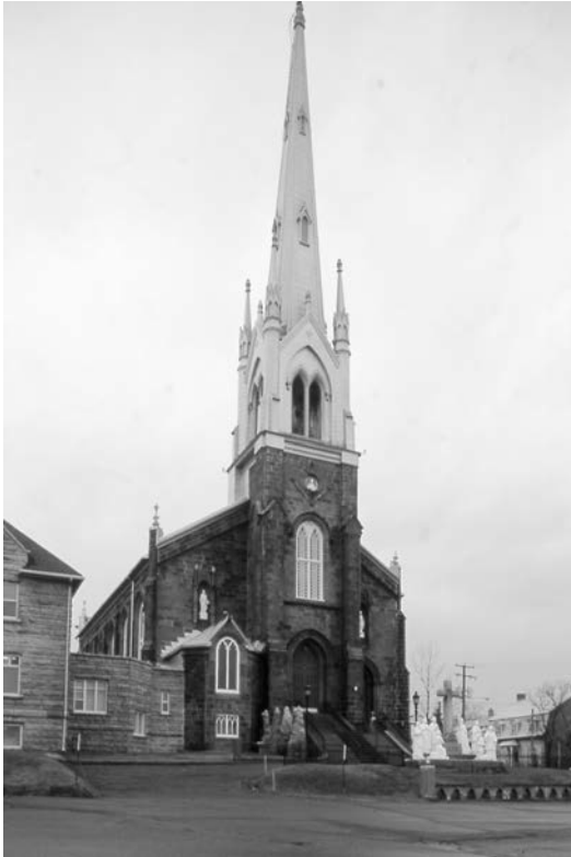
Fig. 2.8 Roman Catholic Church of Saint Michel, Sillery, Quebec.
