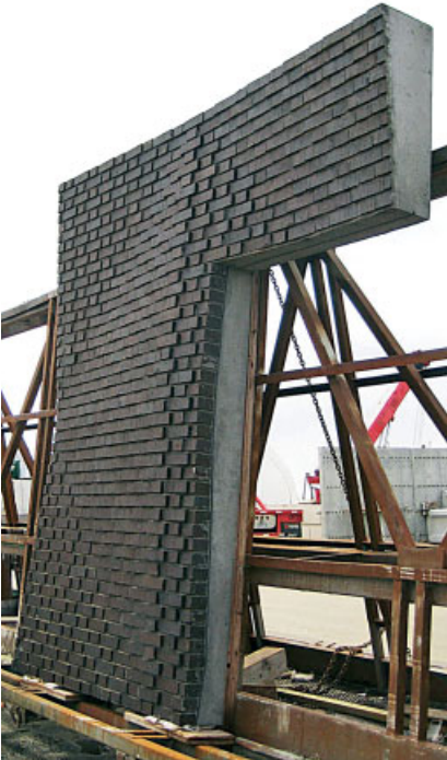
A typical panel cures in the yard prior to shipment. The back-up concrete is tinted to the desired colour of the mortar joints. The architects chose to expose this concrete at the window returns as well. Three typical panels come together to form a window opening, and matching concrete sills were cast separately and placed in the field.
