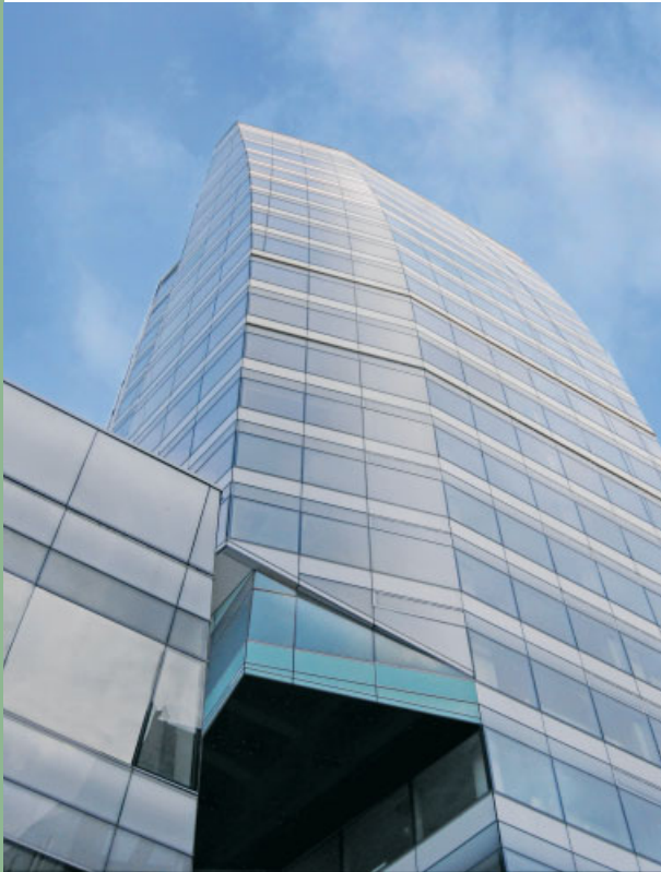
The gently twisted clear-glass and fritted tower of the Cooper Square Hotel tilts slightly as it rises, creating an intriguing presence on the skyline and providing larger rooms on higher floors where the views are unobstructed.
