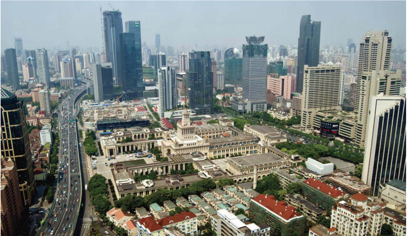
Fig. 5.13. ▲ Center: Shanghai Exhibition Center from East; right mid-ground: John Portman Associates, Shanghai Center, Shanghai, 1984–1990; left: elevated eight-lane thoroughway over Yan'an Road, mid-section, 1998–1999. Photo by author.
