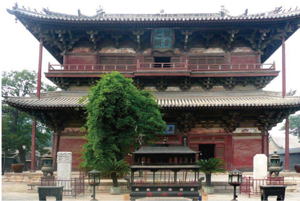
Fig. 1.18. Guanyin Pavilion, Dule Monastery, Ji county, Hebei, 984. Photo by author.
