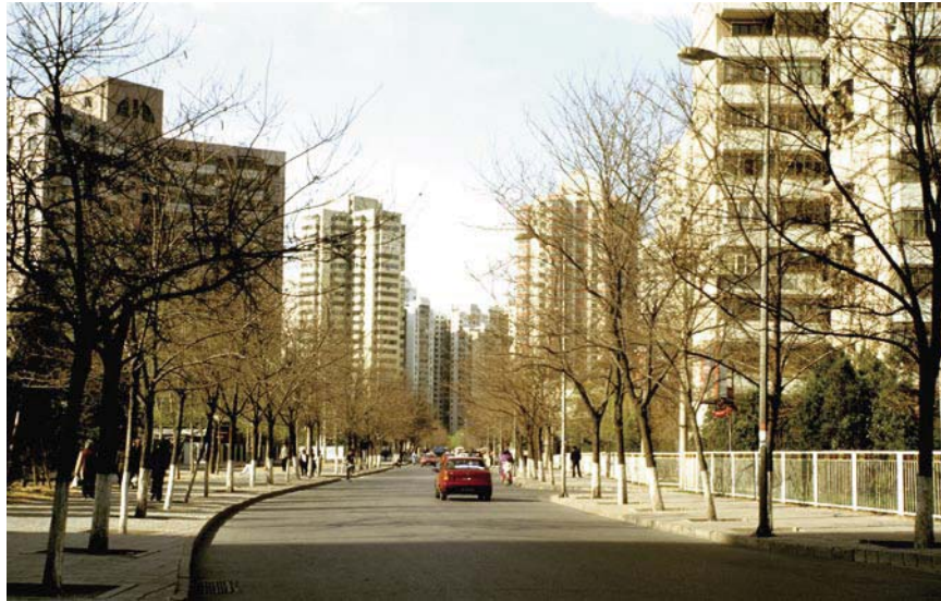
Fig. 15.6. Fangzhuang, one of the earliest large housing developments in Beijing, late 1980s. Photo by author.
