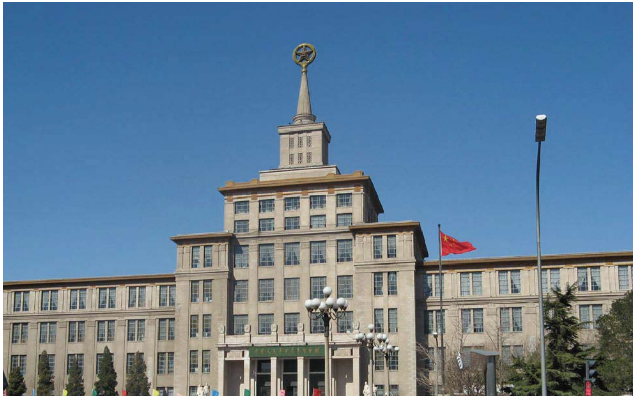
Fig. 5.7. ▼ Ouyang Can, Wu Guozhen, and others, Beijing Building Design Institute, Chinese People's Revolutionary Military Museum, Beijing, 1958–1959. Photo by author.
