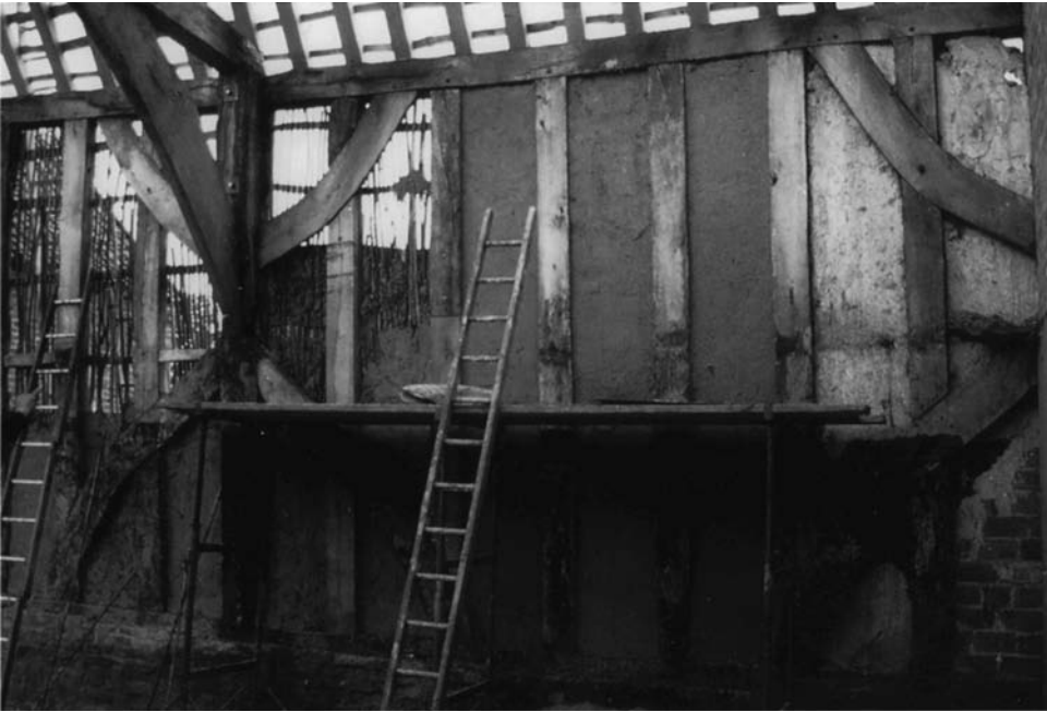
Fig. 3.21 Construction of new wattle-and-daub panels.
