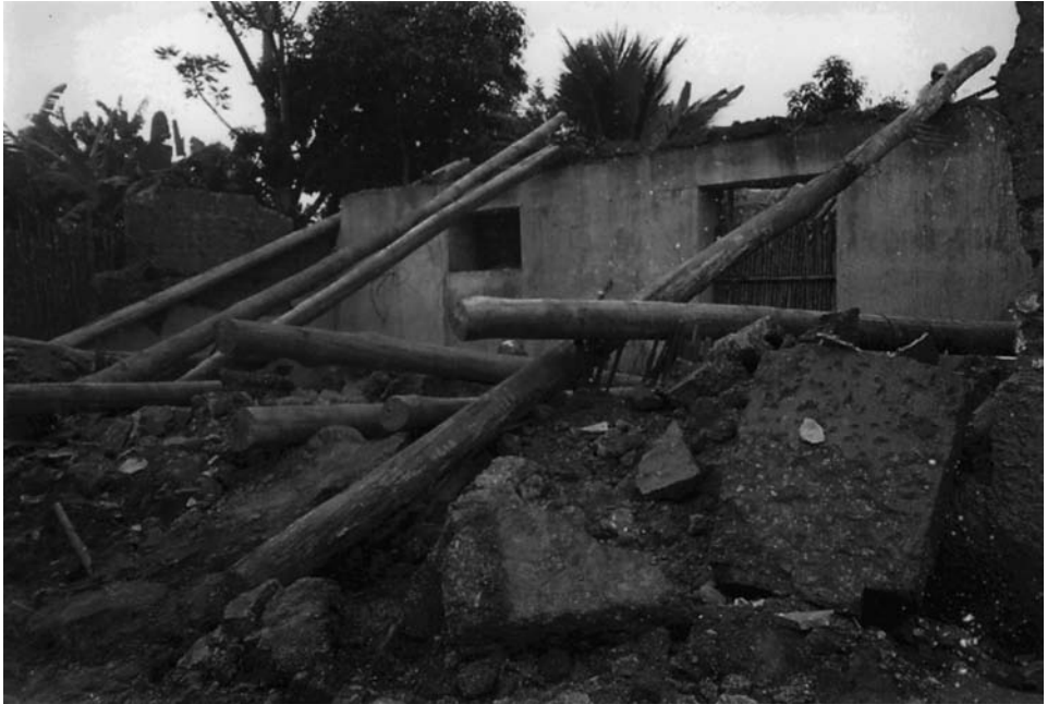
Fig. 6.1 Tapial house in Soritor. (Courtesy of Practical Action.)
