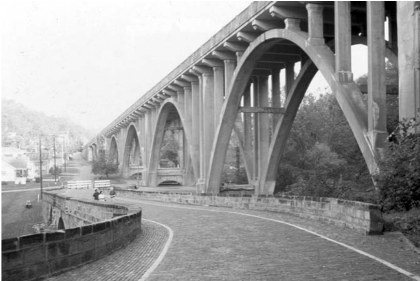
Fig. 3.22 The graceful four-arch US Route 40 concrete viaduct of the mid-1930s in Belmont County, Ohio overshadowing the Blaine Hill ‘S’ Bridge built as part of the national road project in 1828.
