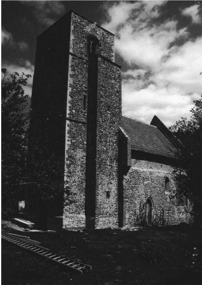
Fig. 6.20 Completion of phase two works.
