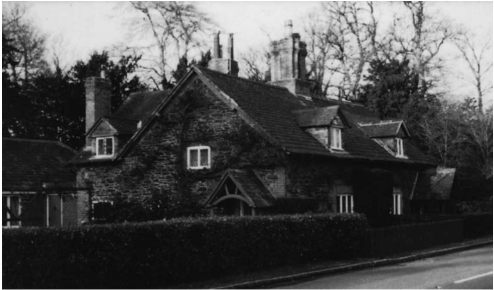
Fig. 3.15 The igneous and metamorphic rocks of the Charnwood Forest area of Leicestershire have provided granite and slate for a number of local buildings.
