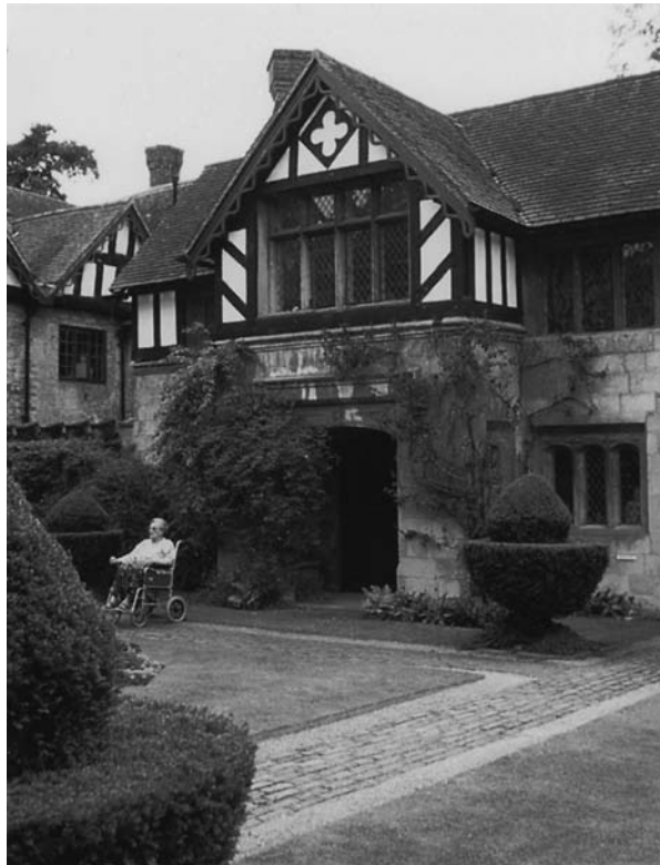
Fig. 3.2 The service wing of Baddesley Clinton, Warwickshire was designed and built in 1890, and blends in well with the medieval manor house despite being built of concrete blocks and sham timber framing (Norman, 1998, p. 12).
