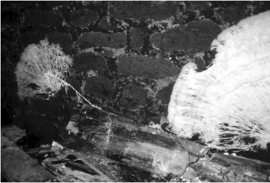
Fig. 4.20 Mycelium of wet rot ( Fibroporia vaillantii ) (Photograph by Hutton + Rostron).
