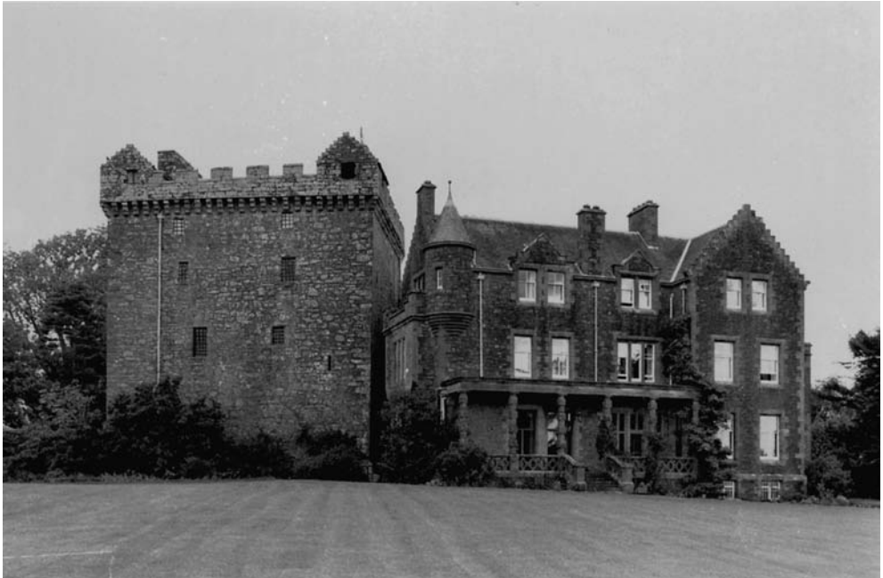
Fig. 2.4 Comlongon Castle, Dumfries, Scotland. The massive fourteenth-century tower house, built at a time when defence was a principal functional requirement in the border region of Scotland, compares to the late nineteenth-century mansion house designed largely for appearance and comfort.
