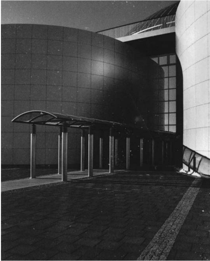
Fig. 7.1 Perlan (The Pearl), Öskjuhlíó, Reykjavík, Iceland. Hot-water storage tanks for the district heating system form the basis for a winter garden, restaurant, meeting room and viewing platform. The dome consists of reflective glass panels on a hollow steel frame carrying hot or cold water to regulate the temperature inside.
