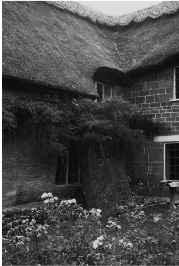
Fig. 3.6 Local materials used together in a traditional manner, creating an important sense of time and place.
