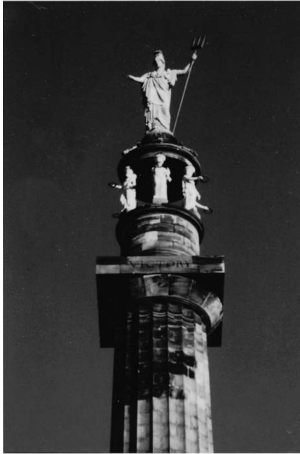
Fig. 3.27 Nelson's Monument, Great Yarmouth, Norfolk (1817–19). The figure of Britannia and the six caryatids around the open drum are constructed of glass-reinforced plastic and replaced original figures of Coade stone. The figures are formed in jointed sections over galvanised mild-steel armatures and support frames, with a concrete filling and etched surface finish.
