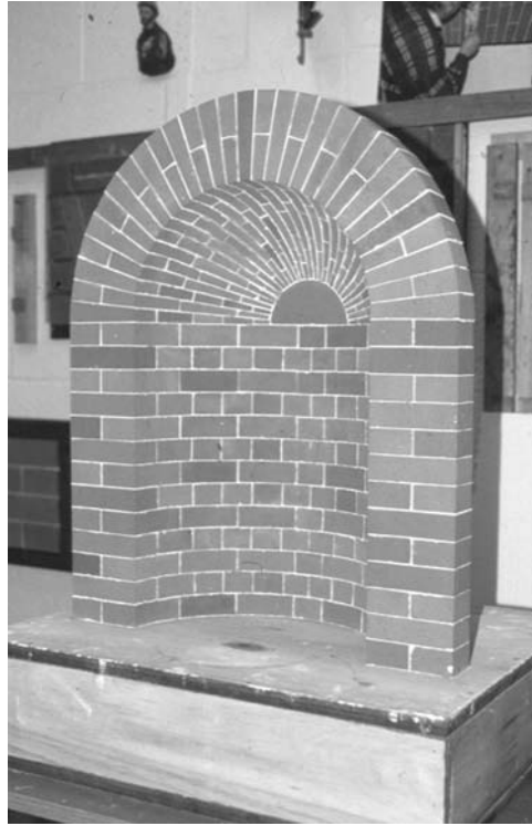
Fig. 6.26 Gauged brick niche constructed by Gerard Lynch in the manner of an apprentice ‘masterpiece’ as part of his doctoral programme. This scaled piece was constructed using six smaller bricks that were individually cut and shaped from one original oversized TLB orange rubbing brick that was produced in the 1950s.
