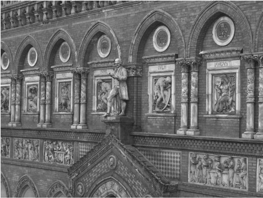
Fig. 3.17 The frontage to the Wedgwood Memorial Institute in Burslem, Staffordshire, was designed following a competition based on the use of decorative ceramics. The chosen scheme was by Robert Edgar and John Lockwood Kipling, which proposed a polychromatic design of decorated brickwork, tiles, terracotta mouldings and panels, mosaic, and Della Robbia ware. Terracotta panels show the months of the year, with mosaic signs of the zodiac above, and bas-relief panels depict the processes of the pottery industry. The building was completed in 1873, when a terracotta statue of Josiah Wedgwood was fixed above the entrance.
