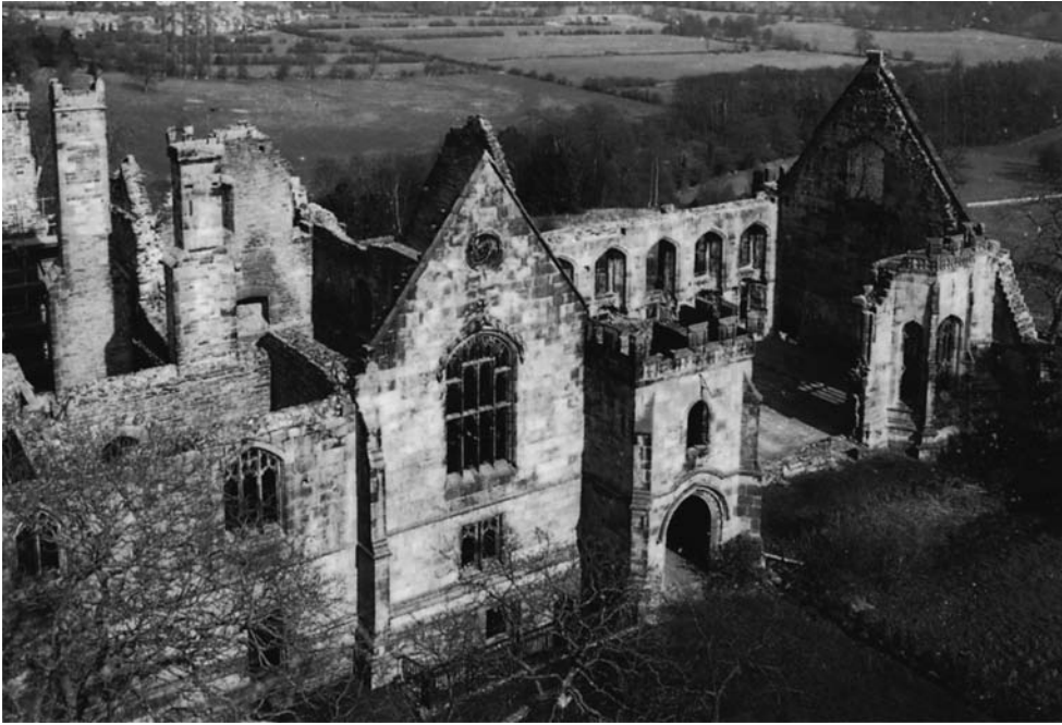
Fig. 5.10 Exposed wall heads and internal surfaces of Wingfield Manor, Derbyshire. Built in the mid-fifteenth century, this country mansion has been unoccupied since the 1770s.
