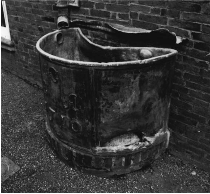
Fig. 7.10 Damage caused to an eighteenth-century lead cistern in an attempt to drain the water and remove from the site.
