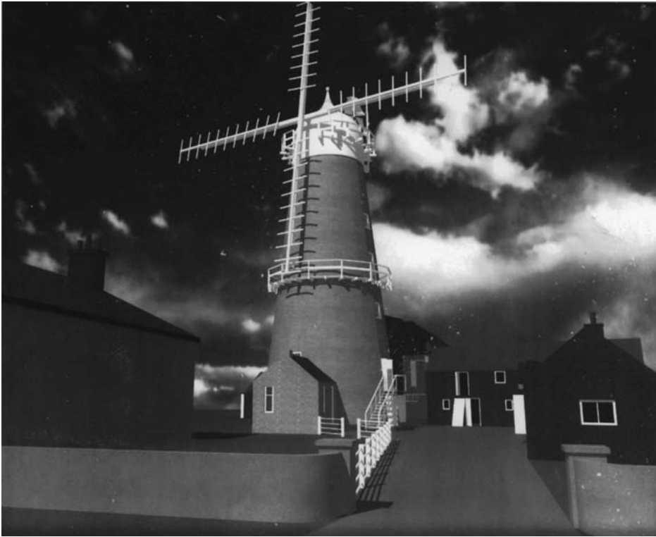
Fig. 3.33 CAD-based modelling and video animation used to record and interpret Denver cornmill, Norfolk in advance of proposed restoration. (Courtesy of Rob Ashton/UKgeomatics.)
