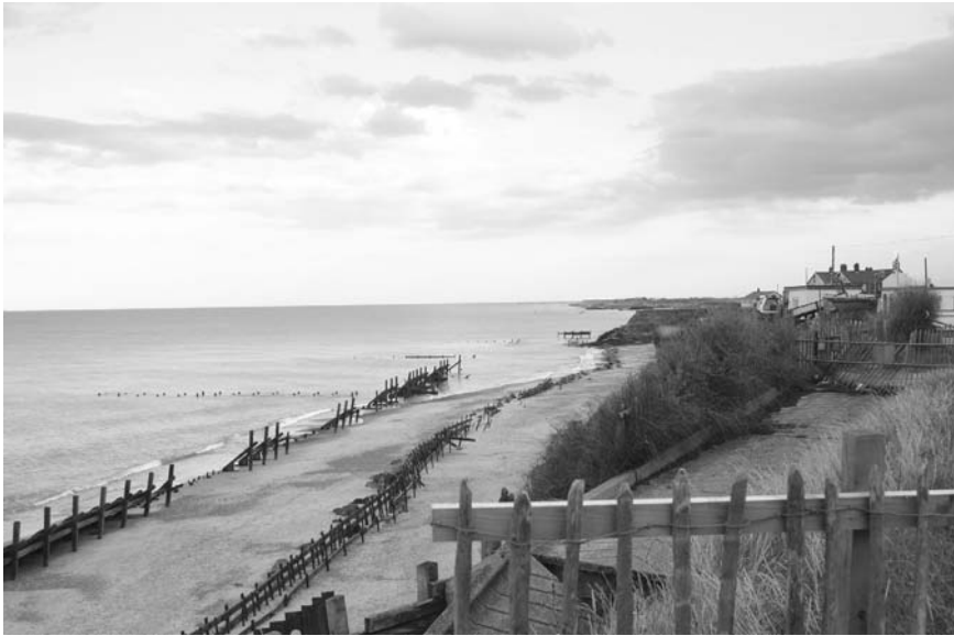
Fig. 6.27 Significant coastal erosion with unsustainable sea defences and preferred policy of unabated erosion leading to loss of heritage assets.
