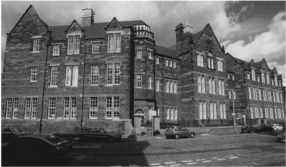
Fig. 6.14 Norton Park exterior. (Courtesy of Burnett Pollock Associates.)
