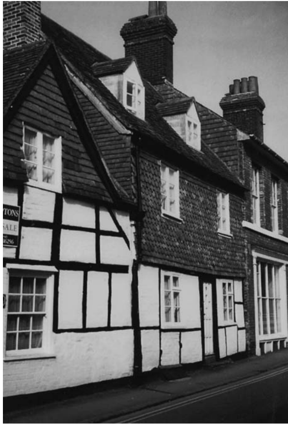
Fig. 3.18 Brick chimney stacks, plain roof tiles and ornamental tile hanging combine with timber framing in Marlborough, Wiltshire to illustrate the influence of changing tastes and fashions.
