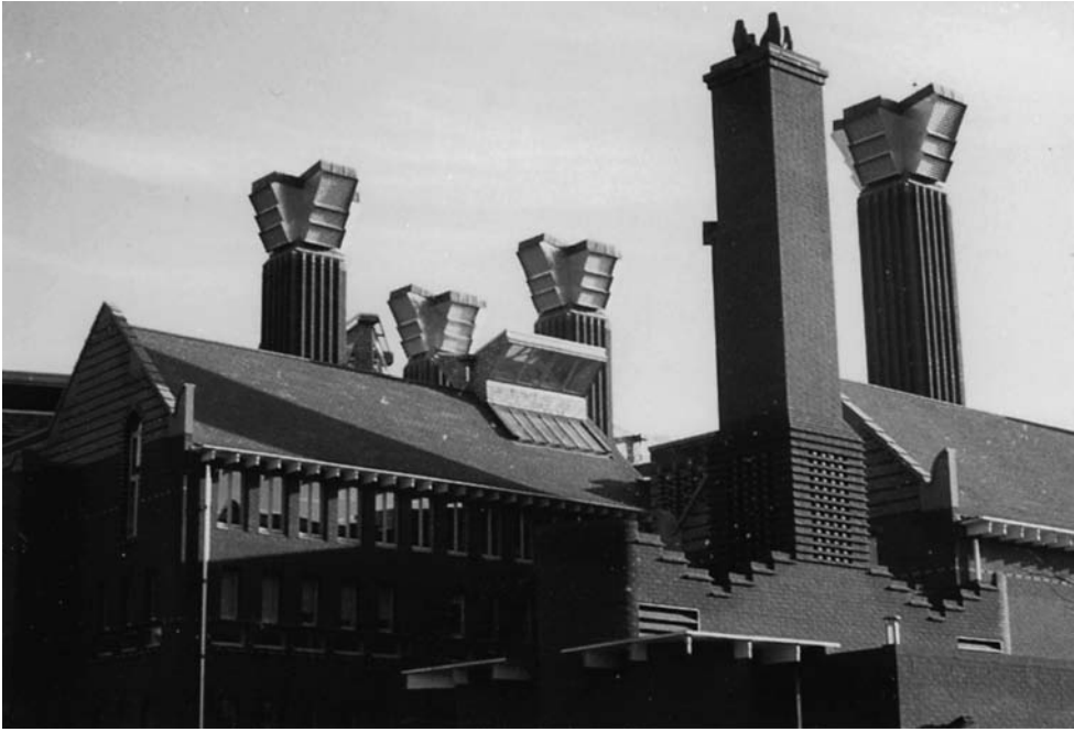
Fig. 3.31 Queen's Building, De Montfort University, Leicester. The design strategy for this low-energy, naturally ventilated building allows it to function without the use of air conditioning, despite high internal heat gains in lecture theatres and computer laboratories. Ventilation for the auditoria relies on the stack effect of warm air rising and being replaced by cold air at low level.
