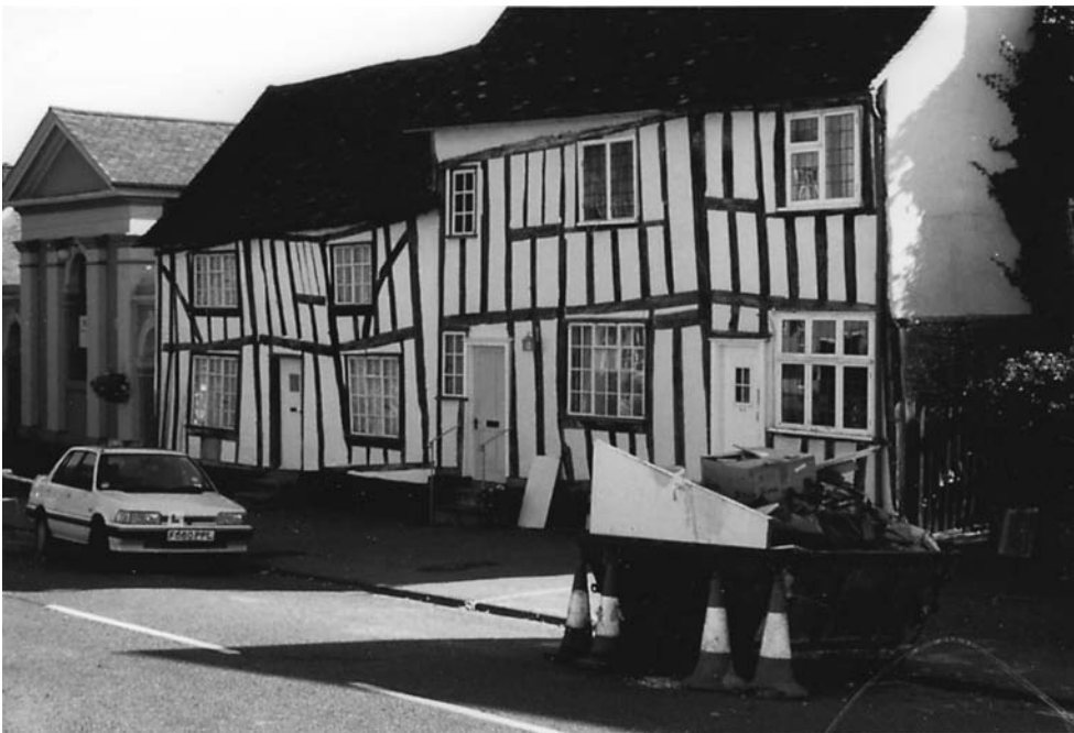
Fig. 5.20 Distortion exhibited by timber-framed buildings in Lavenham, Suffolk.
