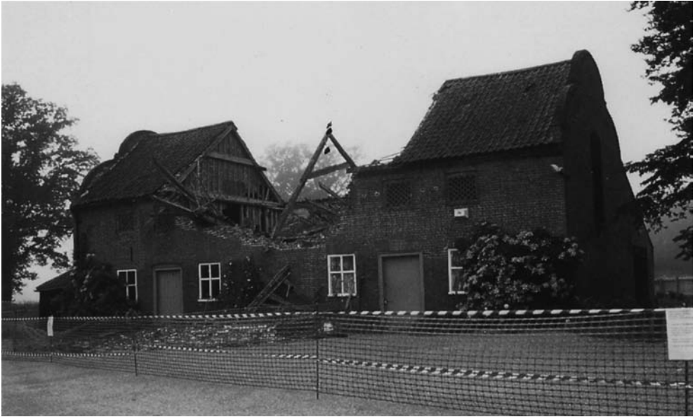
Fig. 4.7 Damage caused by lightning at Blickling, Norfolk in June 1993.
