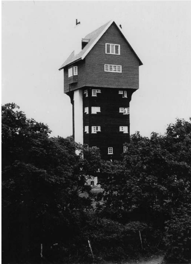
Fig. 2.7 The House-in-the-Clouds, Thorpeness, Suffolk. This combination water tower and house was built in 1923 as part of the Thorpeness village development. The five-storey steel box-frame tower and oversailing two-storey superstructure, which contains the water tank, are clad with weatherboarding.
