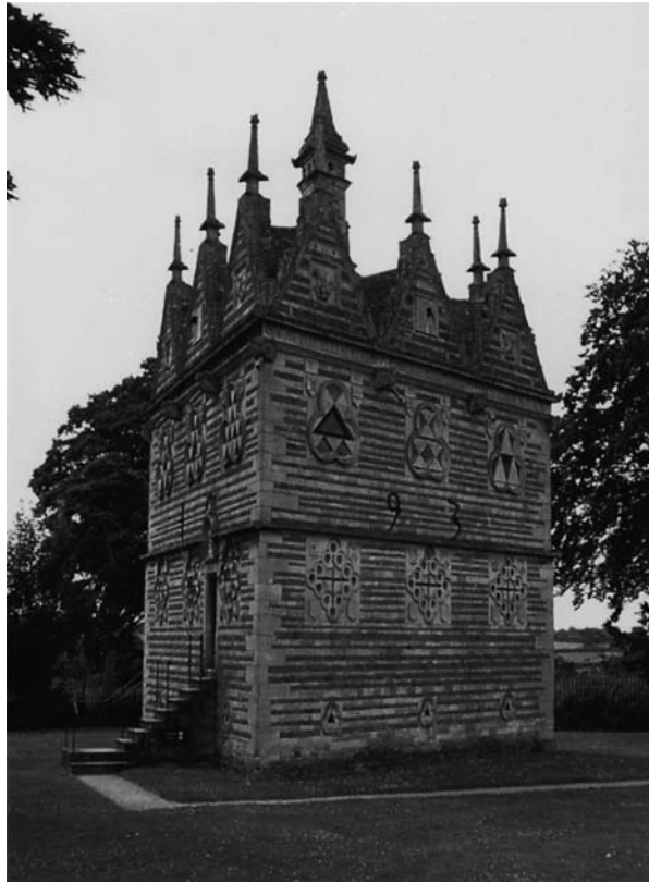
Fig. 2.3 Rushton Triangular Lodge, Northamptonshire. In plan, this building is an equilateral triangle, with three storeys having three windows on each side and on each floor. Each side has three gables, rising to three tapering pinnacles. At the intersection of the roof is a three-sided chimney stack. Below the gables is a frieze with a continuous inscription carried round the three sides, each side (33 ft long) bearing 33 letters. The Lodge, built by Sir Thomas Tresham in 1593–97, is symbolic of the Holy Trinity and linked to the doctrine of the Mass, and contains allusion to both religious literature and personal imagery (Isham, 1995).
