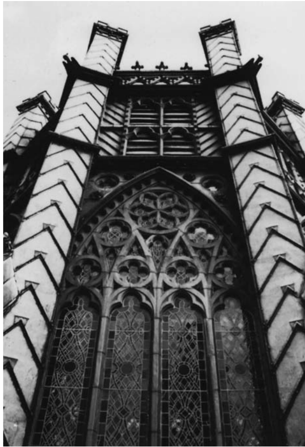
Fig. 3.26 Milled lead used on the lantern to the octagon at Ely Cathedral, Cambridgeshire.
