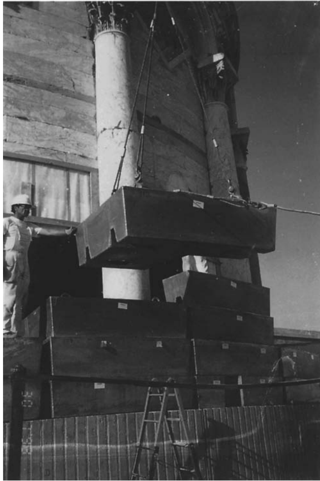
Fig. 6.11 Construction of north counterweight. (Photograph by John Burland.)
