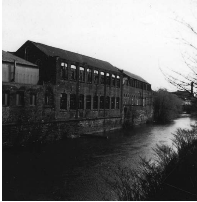
Fig. 5.11 Redundant industrial buildings on River Don in Sheffield.
