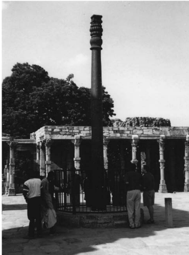
Fig. 3.24 The fifth-century pillar at the Qutab Minar complex in Delhi, India is made of an extremely pure iron and remains virtually free from corrosion. (Photograph by John Stanley.)
