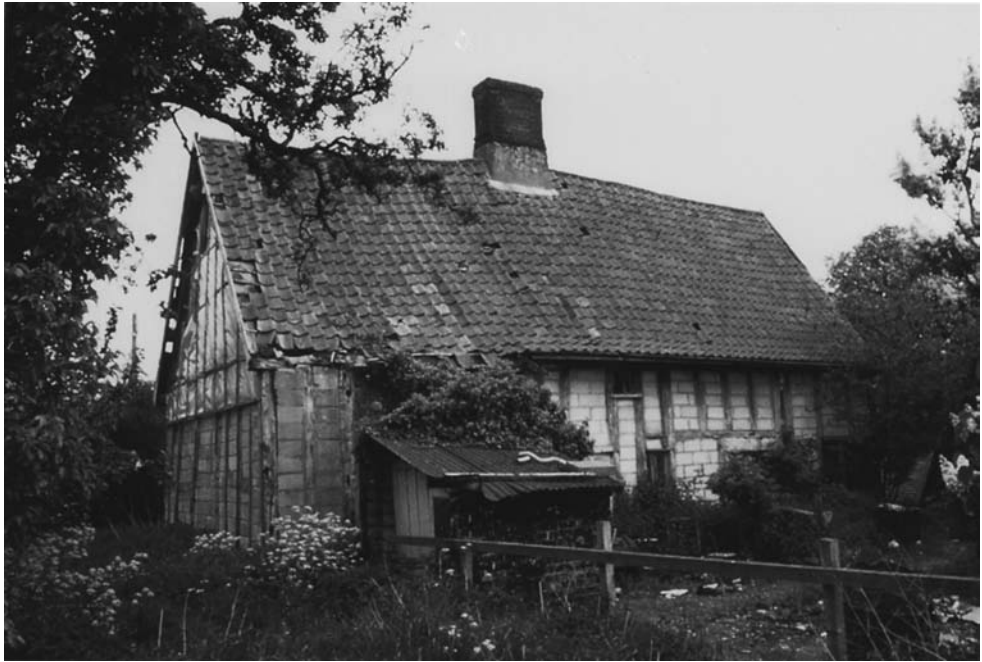
Fig. 3.8 Early timber-framed buildings made use of many small trees, typically oak, for both framing and finishing. In his work on the British countryside, Oliver Rackham (1986, p. 87) has calculated that some 330 oak trees were used in the construction of a fifteenth-century Suffolk farmhouse, half of the trees being less than 9 inches in diameter. These timbers, and others of greater size, might have been transported around the country, and made ready close to the location of the proposed building.
