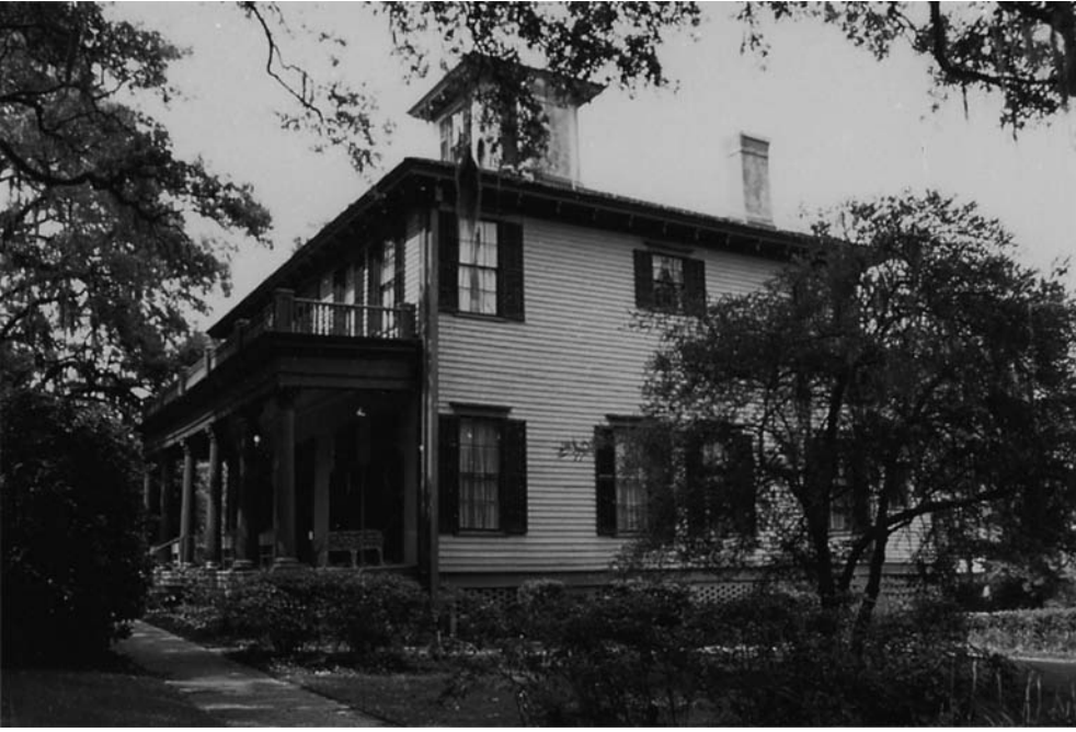
Fig. 3.28 Brokaw-McDougall House, Tallahassee, Florida. Built in c. 1856–60, this house was designed to provide a comfortable internal environment with its veranda, shuttered windows, overhanging eaves, cupola and tall ceilings. The internal arrangement, with shaded windows and the cupola positioned over the stairway, provided ventilation throughout the house before the advent of air conditioning.
