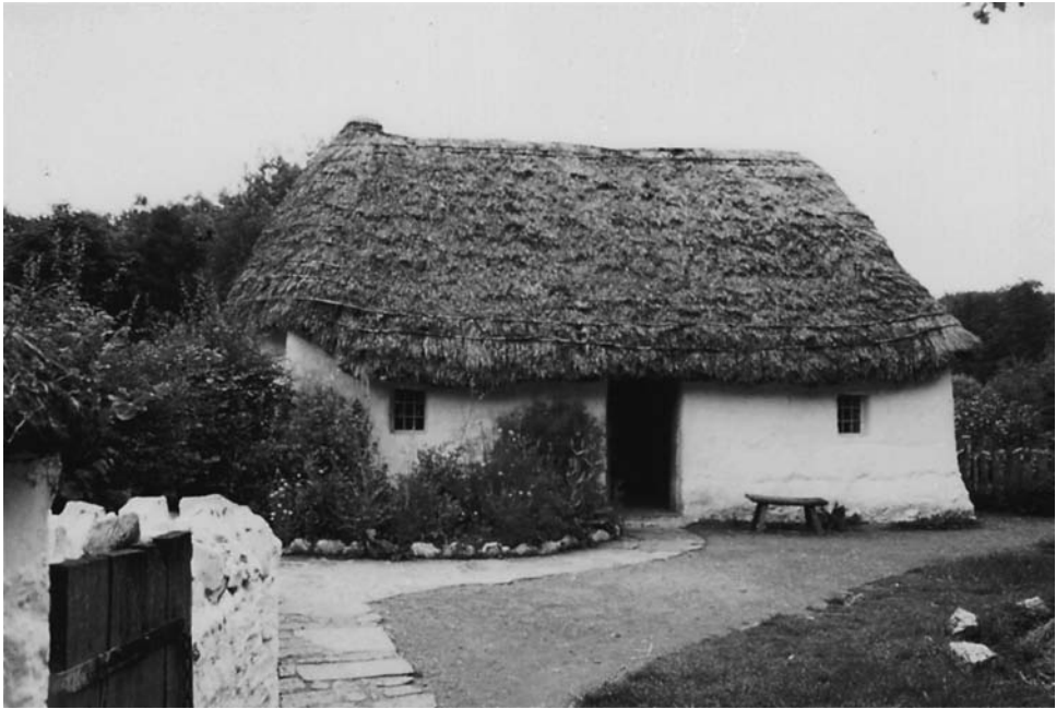
(a) Appearance of the cottage.
