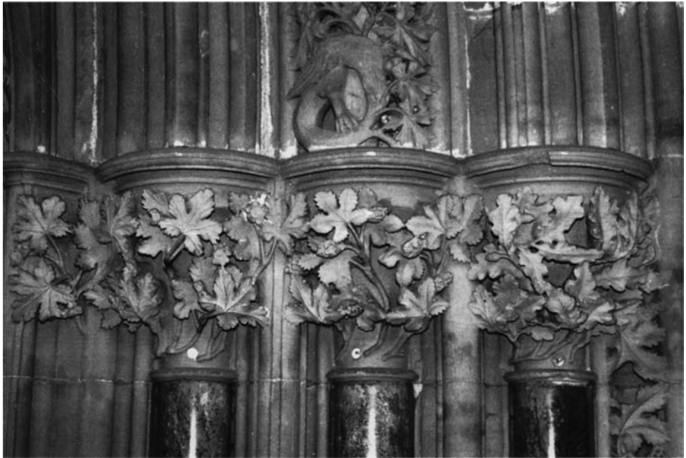
Fig. 2.9 The carved stone foliage and Purbeck marble shafts to the doorway into the Chapter House at Southwell Minster, Nottinghamshire (c. 1290) display a new artistic realism for the period in combination with conventional architectural elements. (By kind permission of the Provost and Chapter of Southwell Minster.)
