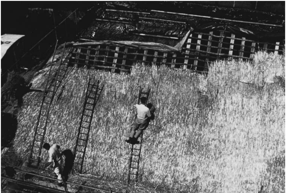
Fig. 3.13 Long-straw thatching in progress using specifically grown materials to avoid deterioration caused by chemical fertiliser residues.
