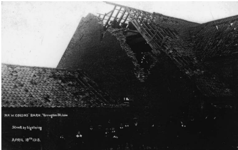
Fig. 5.3 Postcard showing damage caused by lightning at Grove Farm, Terrington St John, Norfolk in April 1913. (Courtesy of Mr and Mrs C. Cousins.)
