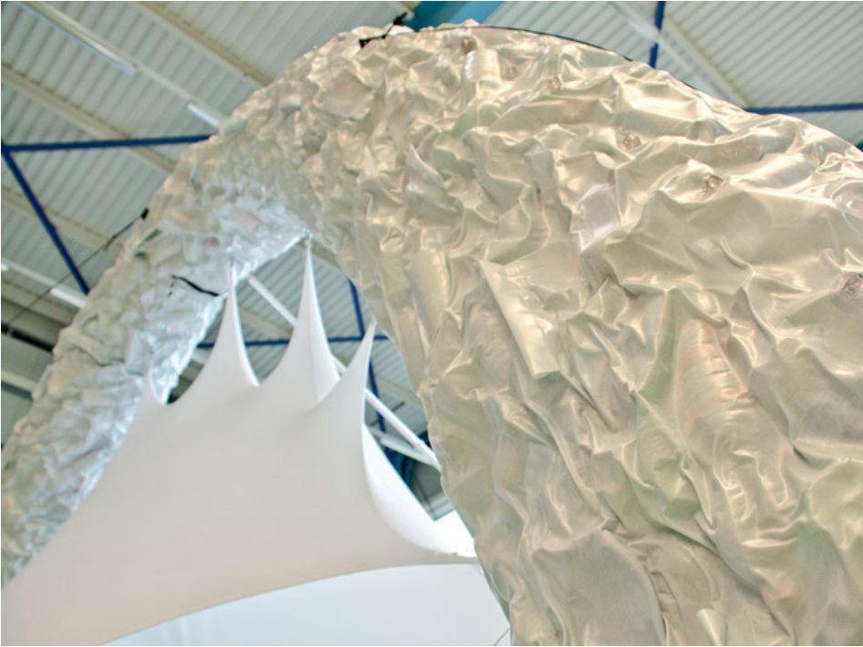
8 The Airless arch system can be constructed out of various foil types, addressing different functional and aesthetic properties.
