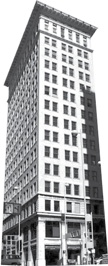
1903: Ingalls Building, Cincinnati, Ohio, Elzner & Anderson. First reinforced concrete high-rise building.
