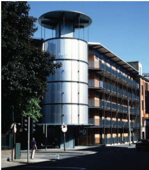
**Figure 2.45** Murray Grove: pioneered prefabrication.
