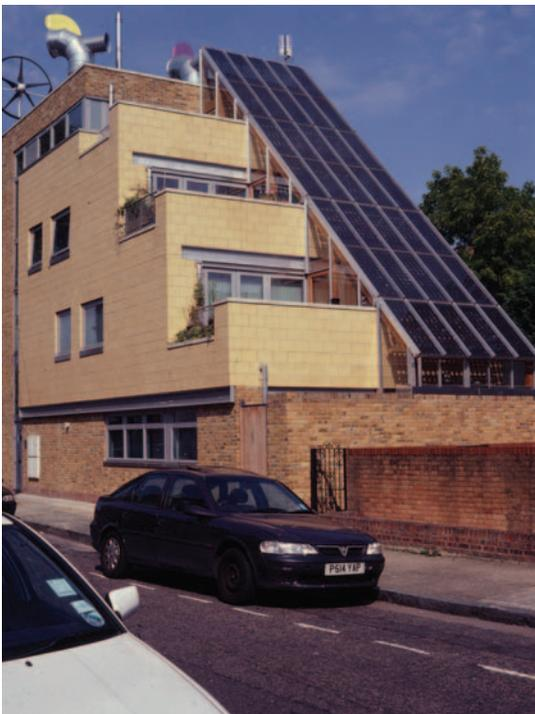
**Figure 2.106** BowZED zero carbon housing.
