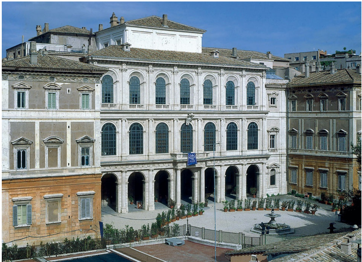
4.26 Carlo Maderno with Gianlorenzo Bernini and Francesco Borromini, Palazzo Barberini, entry façade, Rome, 1628–33.
