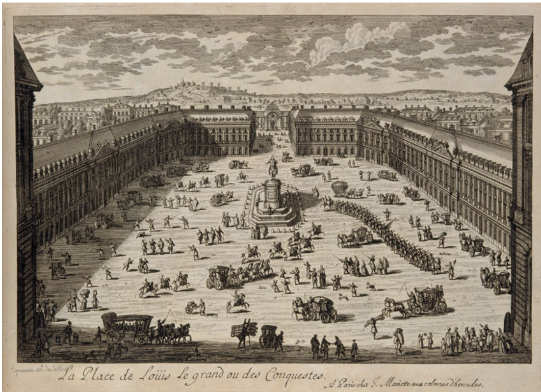
10.3 Jules Hardouin-Mansart , Place Louis-le-Grand (Place Vendôme), Paris, begun 1699. Etching by Pérelle, mid seventeenth century. Château de Versailles.
