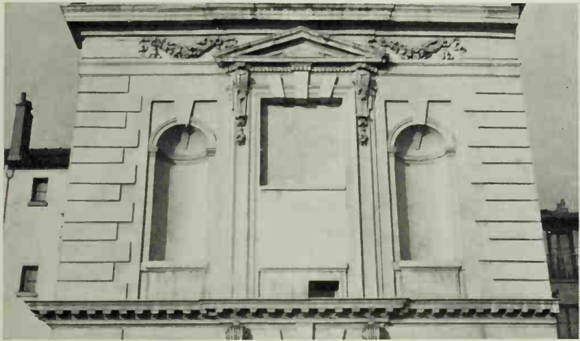
(A) and (B) François Mansart: Château of Berny, Seine. Begun before 1624
