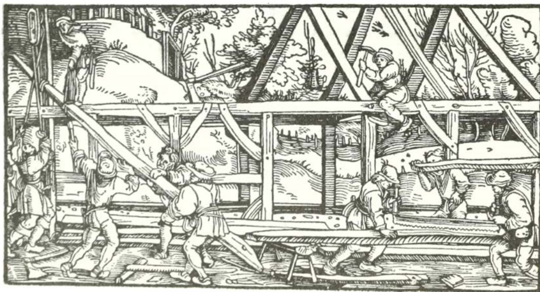
Building a timber-framed house. German woodcut, 16th century.
