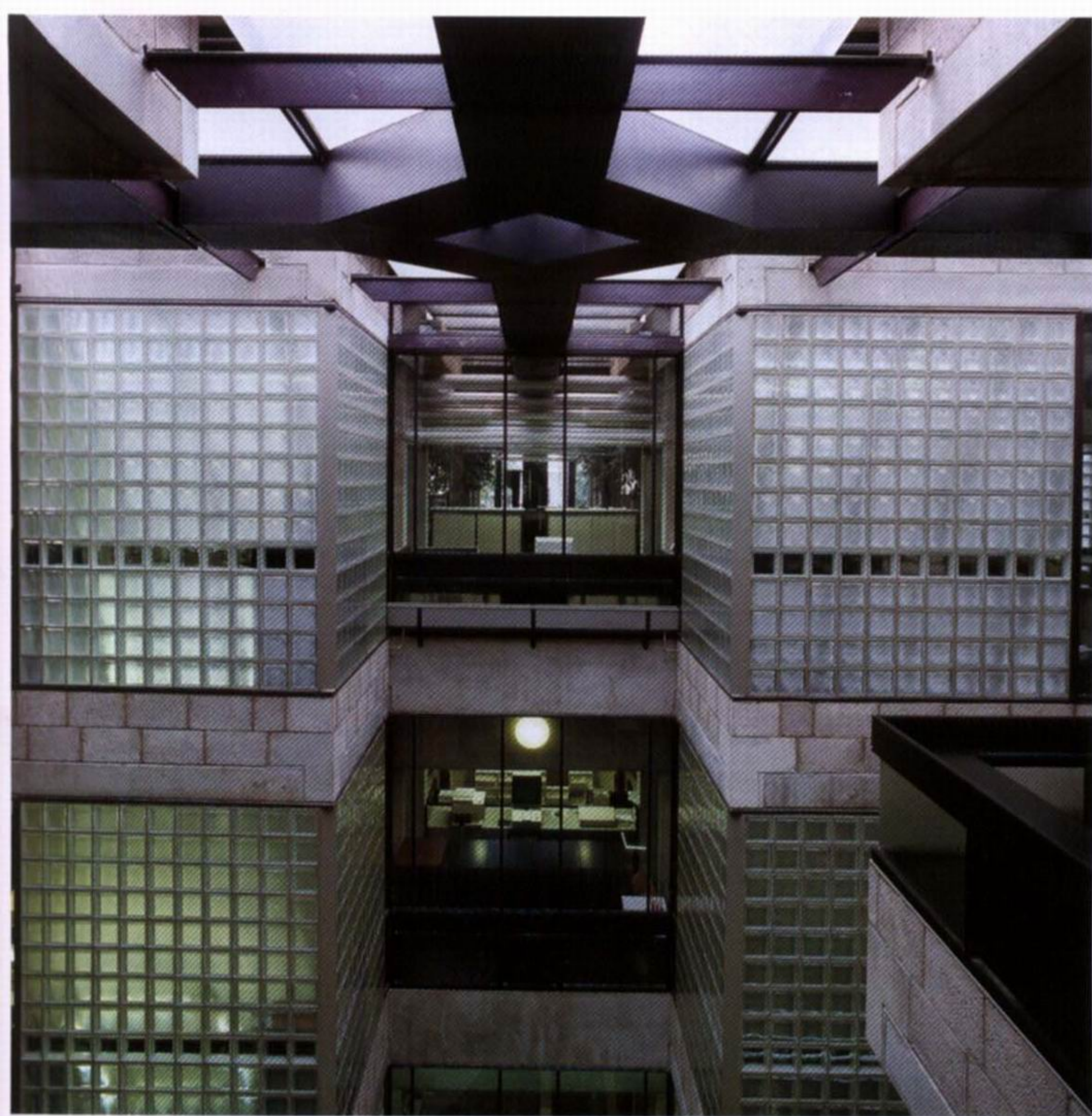
(Above) Internal light well and (right) staircase
