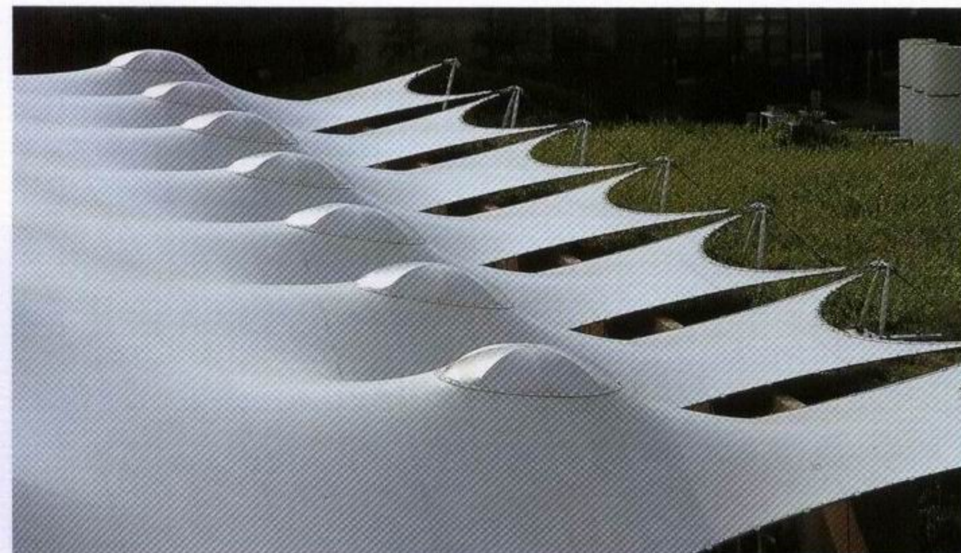
(Left) The translucent fibreglass membrane coated with teflon, seen from above and below
