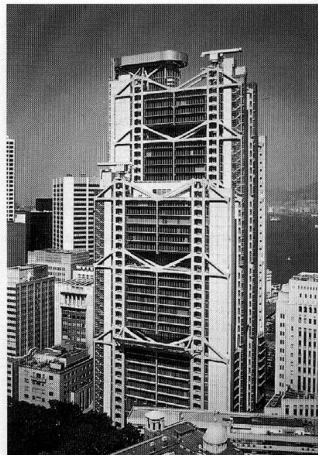
Foster Associates, Hong Kong and Shanghai Bank
