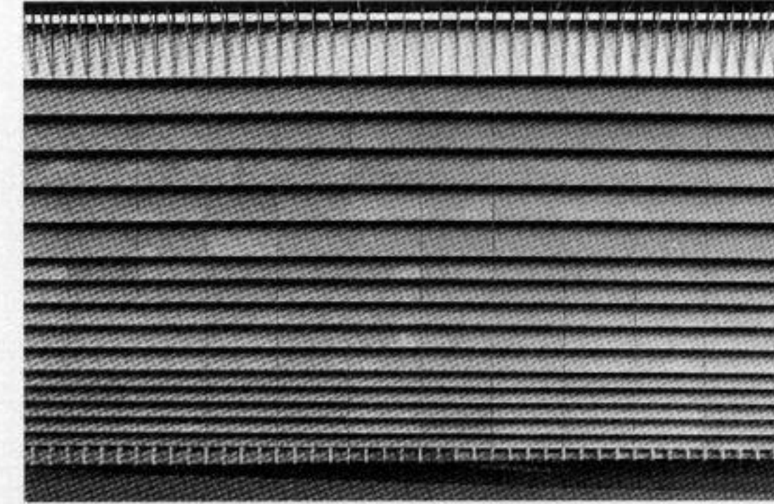
Jacques Herzog and Pierre de Meuron, Ricola Storage Building, Laufen, Switzerland (1986–87)
