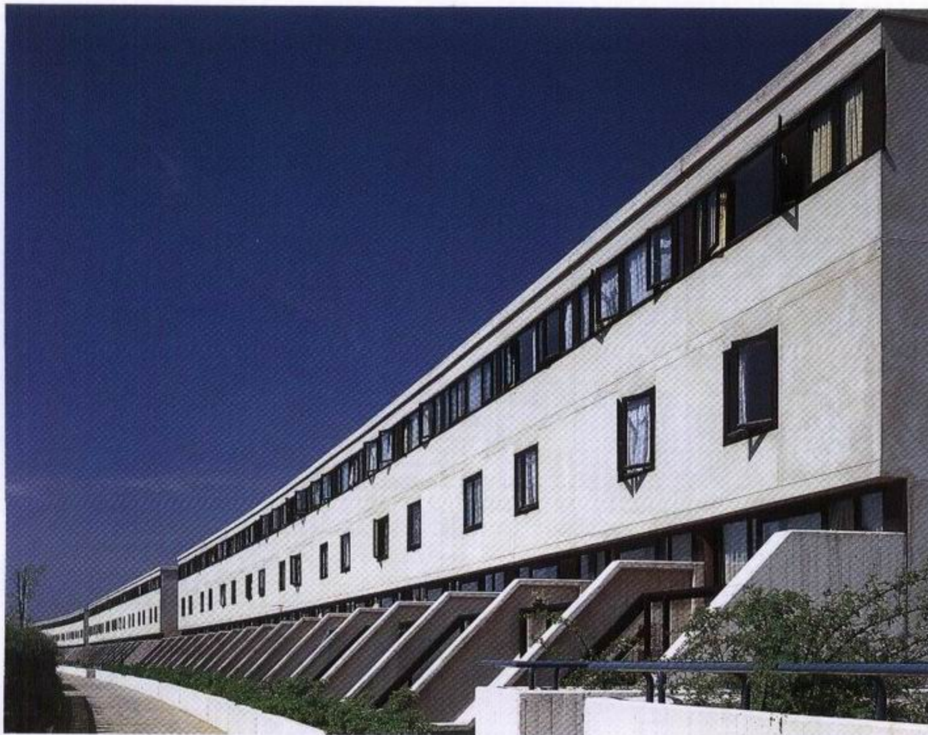
Two views of the pedestrian streets of the Alexandra Road housing project
