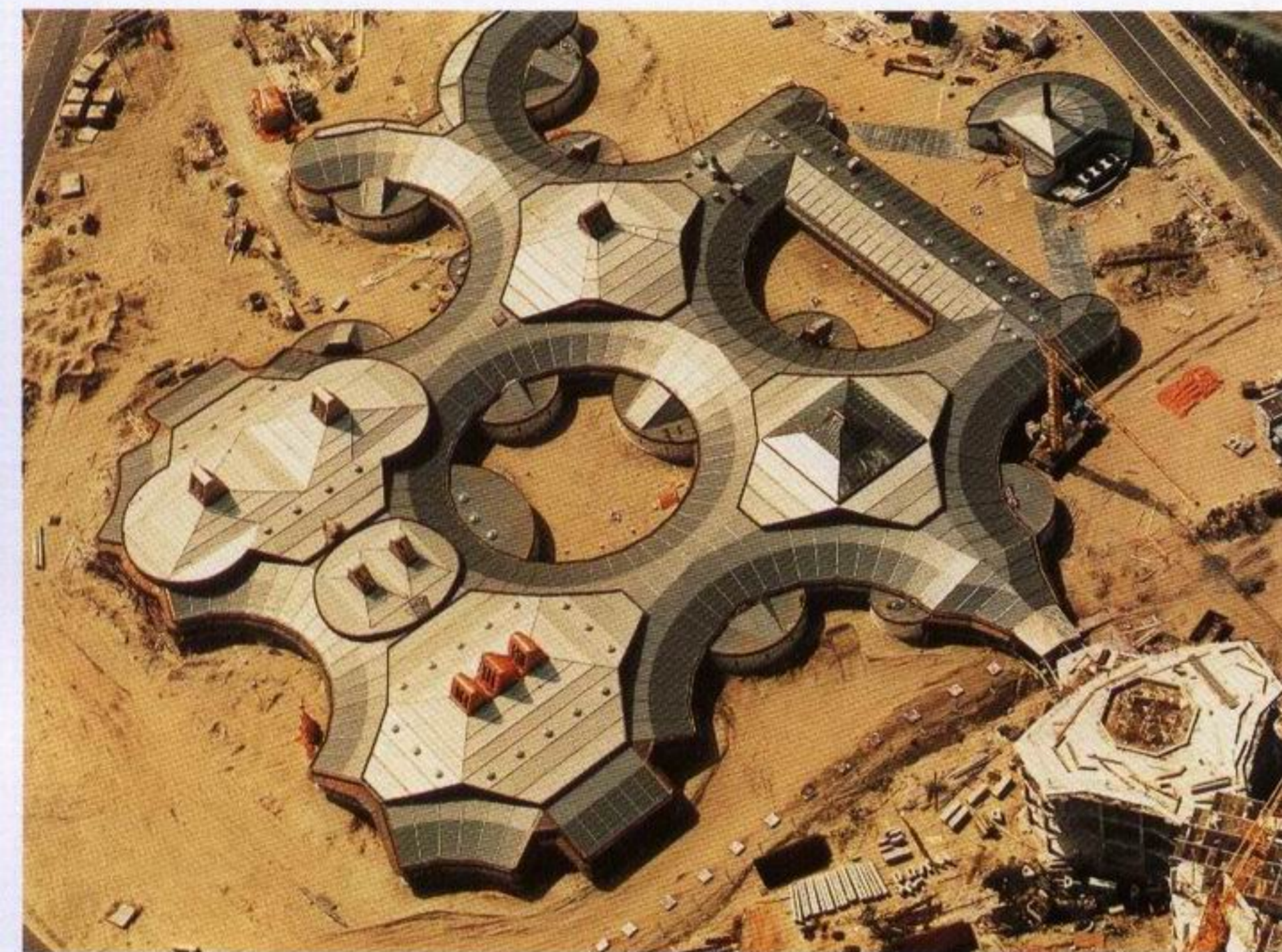
(Left) Aerial view
