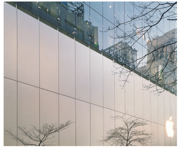
Bohlin Cywinski Jackson, Apple Store, Tokyo, 2003. Stainless steel panels in a precise rectangular grid are broken only by the company logo, which is subtly integrated into the design. Because they are bead blasted and thus slightly reflective, the panels appear to change color with the weather, ranging from cool gray to warm green/gray.
