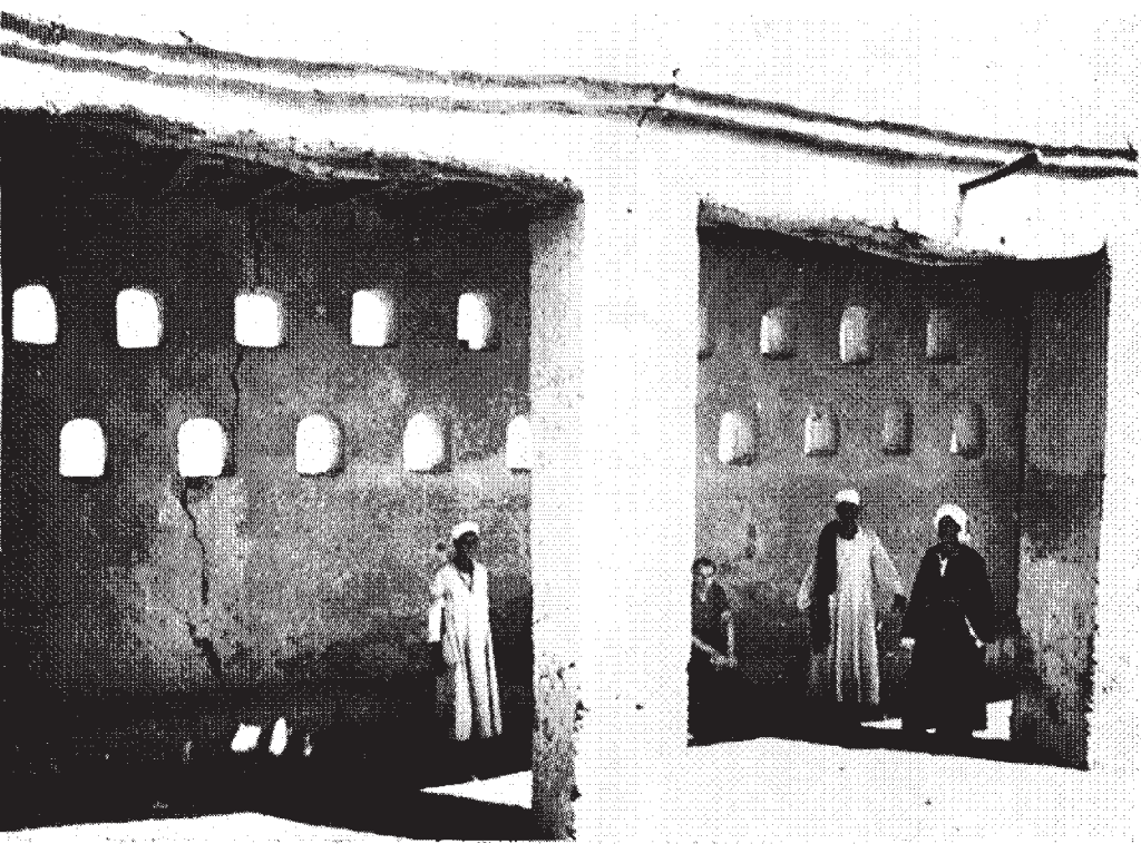
48. Loggia wall with openings to the windward side
