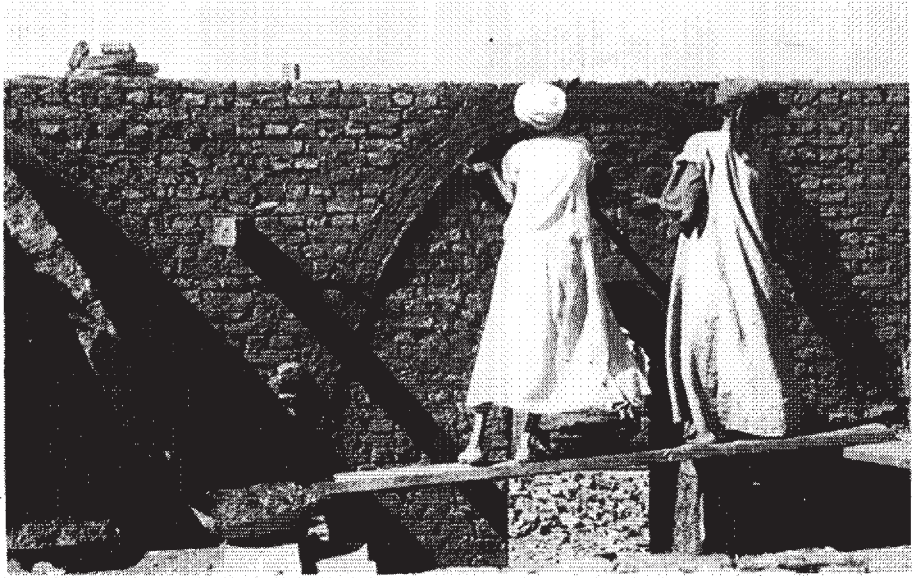
8. Trimming plaster with an adze
