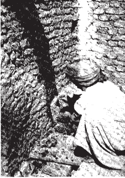
9. The first brick is laid against the end wall
