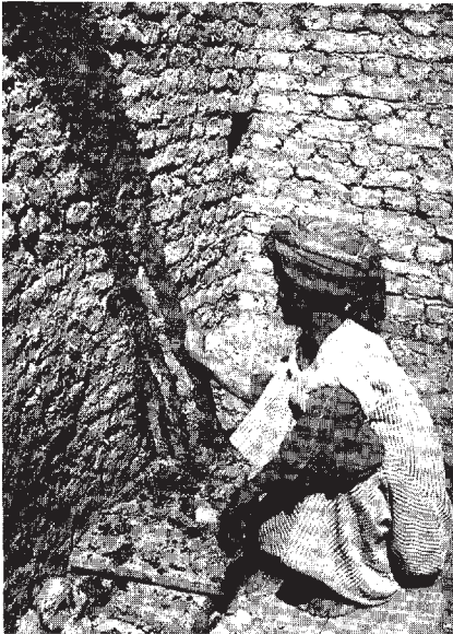
13. More mud is laid against the third course
