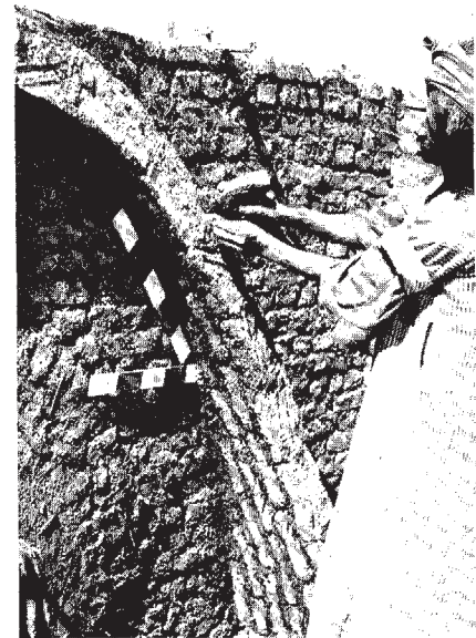
16. The first inclined ring is completed
