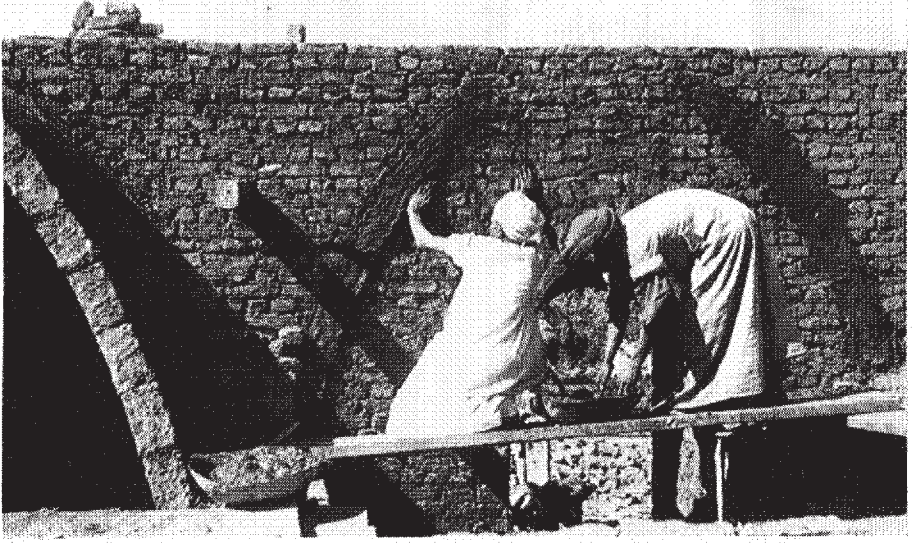
7. Masons outline a parabola on the end wall with mud plaster
