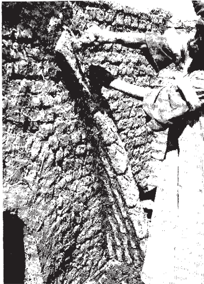
15. The fifth course is completed
