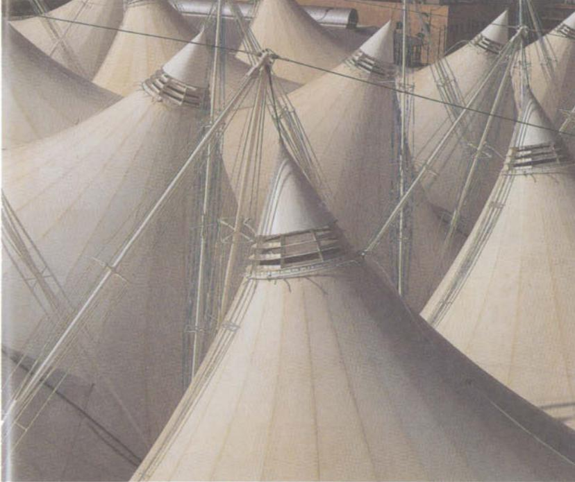
Fig. 17. (c) On top of each conical structure is a warm air exhaust opening combined with an evaporative cooling system to create an evaporative tower.
