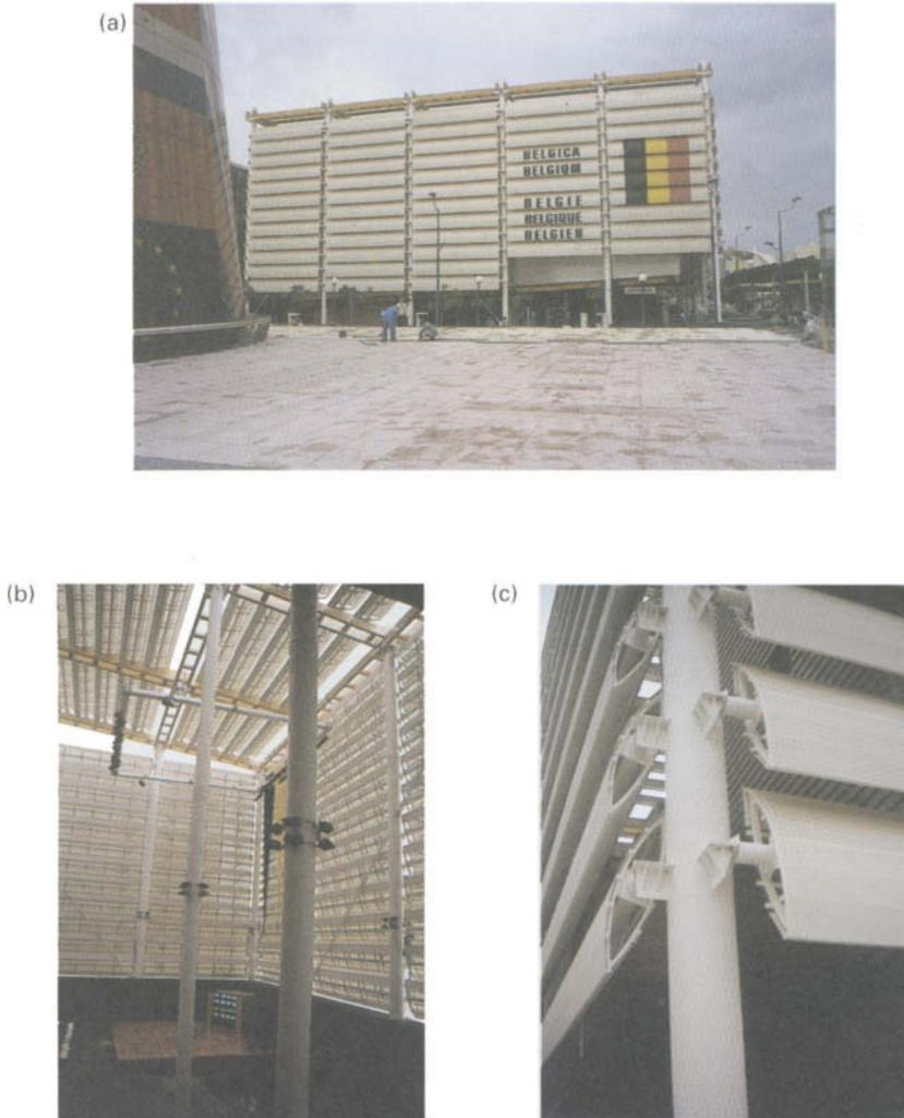
Fig. 8. *Belgian Pavillion, Seville, Spain* (Driesen–Meersman–Thomaes). (a) The Belgian pavilion may be considered as a large courtyard, on the outside protected from the sun by a system of screens. (b) A column structure based on a  $10 \times 10$  m module supports the surrounding sun screen system and the exhibition building, the containers, sheds, balcony, staircase and walkways. (c) Sun-protecting fabric wings on front walls.
