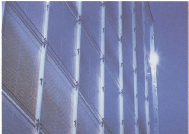
Fig. 3. *Business Promotion Centre, Duisburg, Germany (Sir Norman Foster and Partners)*. (a) The seven-storey Business Promotion Centre is a landmark building which hopes to regenerate business and promote growth in the Ruhr area. (c) The triple layered cladding system uses computer controlled blinds.
