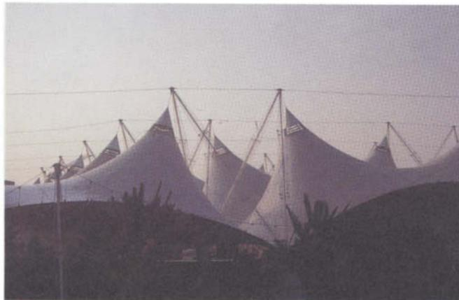
Fig. 17. *El Palenque*, exhibition structure, Expo '92, Seville, Spain (J. M. De La Prada Poole). (a) The Palenque is an area of 8000 m<sup>2</sup> including a space for shows with capacity for 1500 spectators, together with other areas for restaurants and shops. (b) The white PVC covering (13% transmissivity) has a controlled irrigation system to avoid the overheating of the external side and the re-irradiation to the spaces below.
