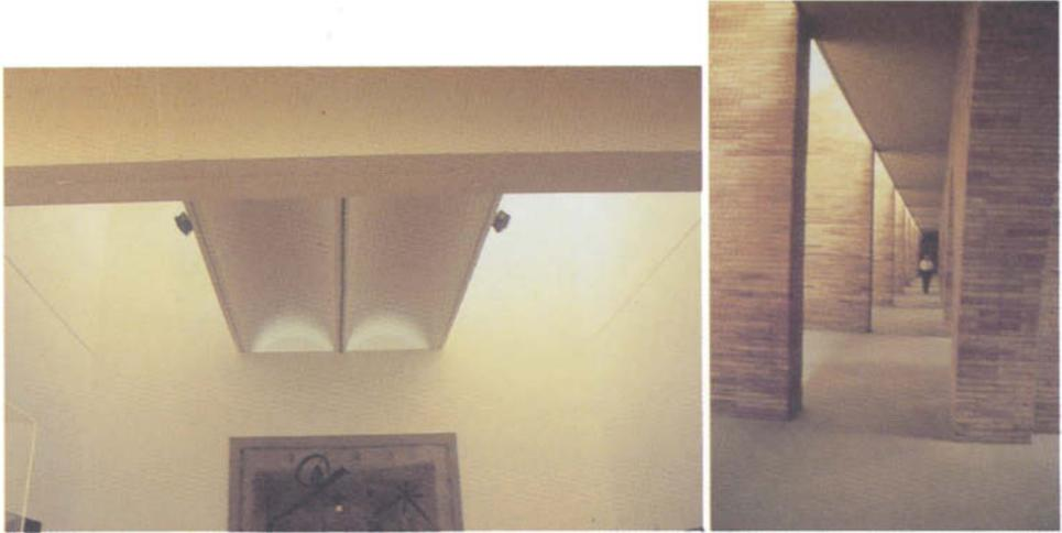
Fig. 16. Photograph of an interior with 'hidden light', showing the light but not the opening.
