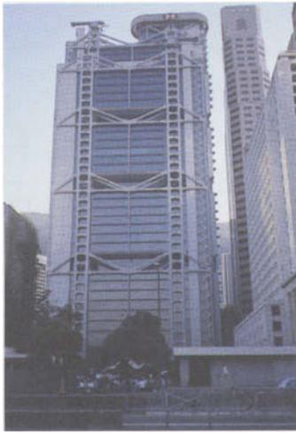
Fig. 11. *Hong Kong Shanghai Bank, Hong Kong* (Foster Associates). The suspension structure in asymmetrical trusses: the “short” part of the hanger holding up the service modules and escape stairs; the “long” part holding up the central floor spans. The vaste banking hall atrium where natural lighting is increased by a sophisticated array of movable mirrors powered by a computer-controlled electric motor.
