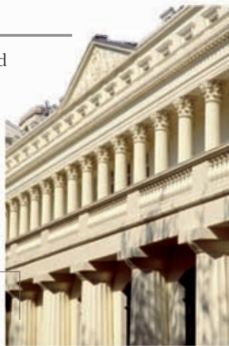
Cast-iron Doric columns
