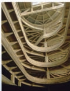
FACTORY INTERIOR, SHOWING HELICAL RAMP
