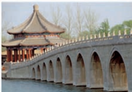
BRIDGE OVER KUNMING LAKE
