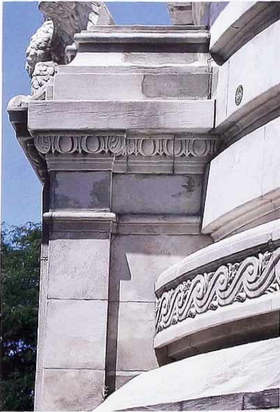
OM-63 Bottom right: Vitruvian scroll; upper left: egg-and-dart molding. Fascia above and below ornamented molding
