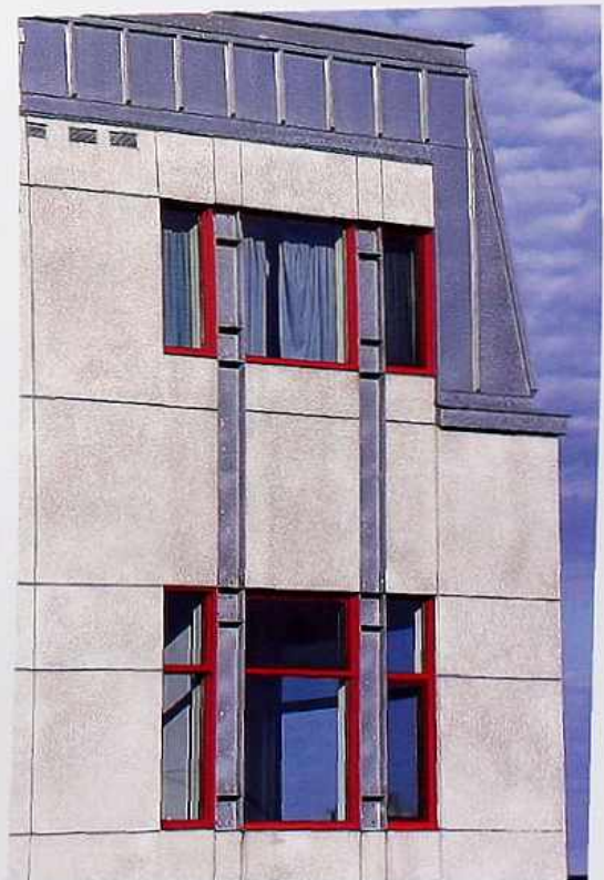
WI-157 Metal design in spandrels connecting upper and lower windows
