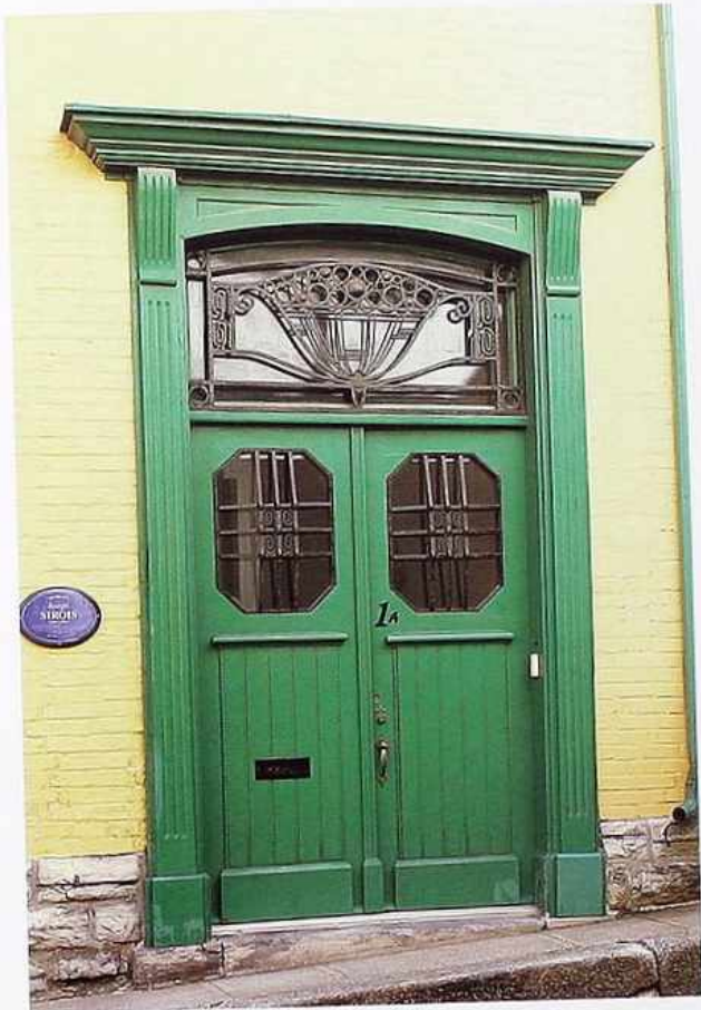
DW-69 Paneled double doors with octagonal lights with leaded glass transom in cambered arch; letter slot; fluted pilasters; crown molding
