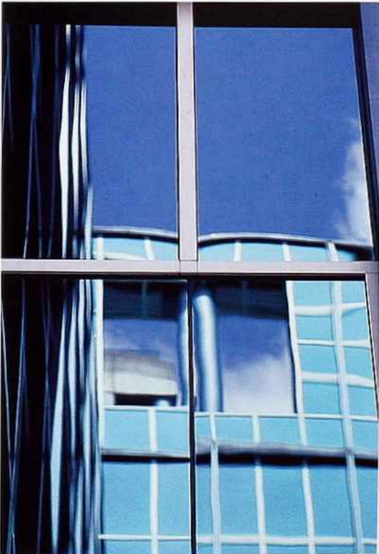
WI-7 Stainless steel muntins, modern commercial building
