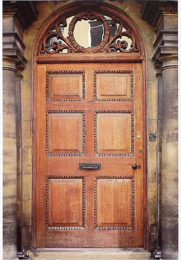
DW-17 Six-panel wood door with raised panels, carved molding, and half-round transom light
