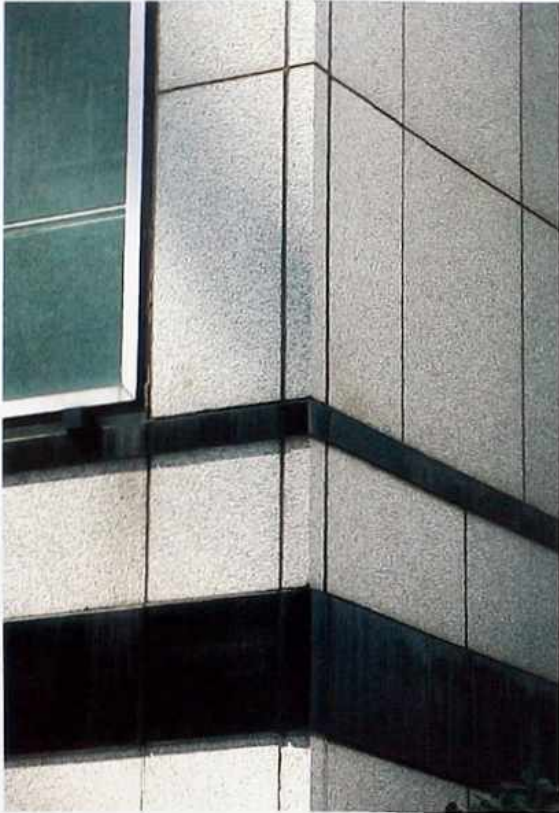
WA-131 Outside corner of granite veneer with raked joints; belt courses at window and jetty, modern commercial building
