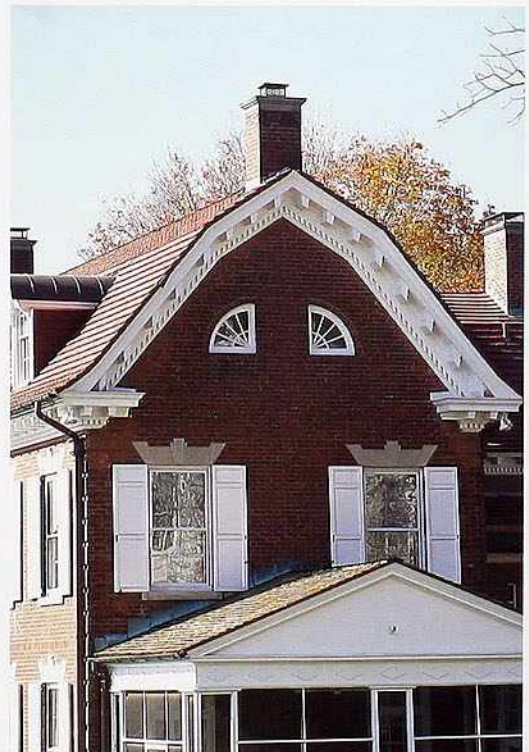
CR-129 Flared gambrel, soffit with modillions
