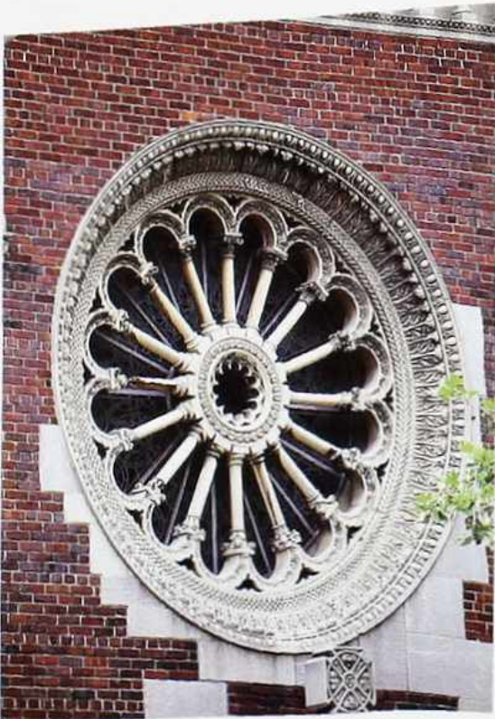
WI-67 Rose window with stone tracery
