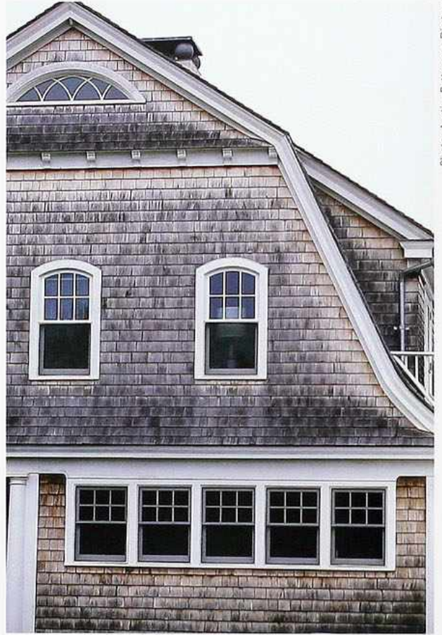
WI-49 Top to bottom: arched gable window; arched six-over-one double-hung windows; six-over-one double-hung windows, traditional shingle house
