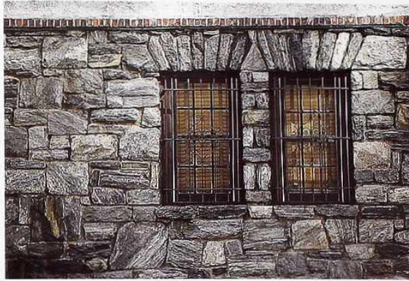
WI-129 Windows with jack arches in roughly squared random stone wall
