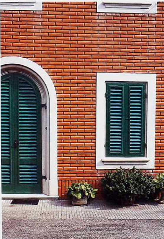
WA-177 Modern variation of Roman brick in running bond with tinted mortar and soldier base course; louvered shutters on door and window
