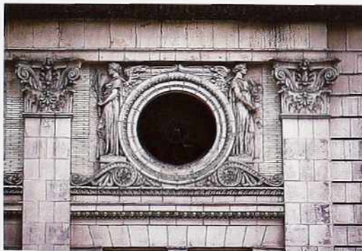
OM-51 Stone relief frieze over entry: bull's-eye window framed by draped figures, scroll motifs, and Composite capitals on flat pilasters
