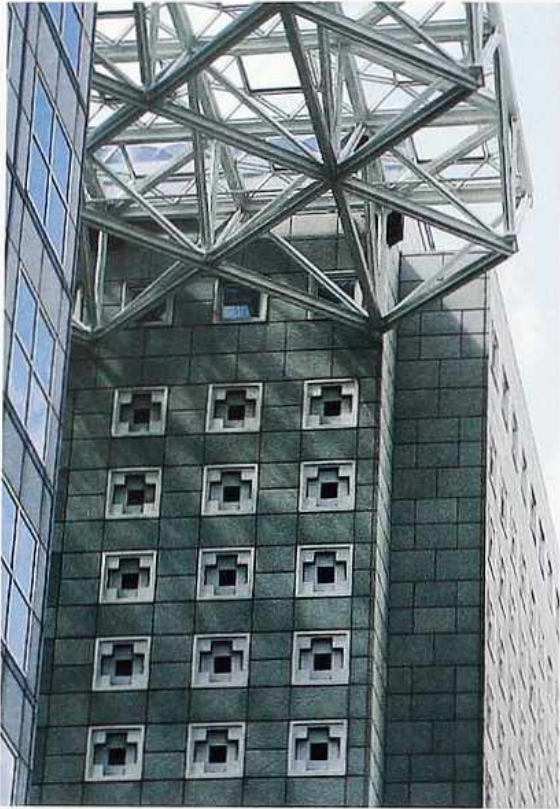
WA-138 Granite veneer with contrasting granite window inserts surmounted by space frame, modern commercial building
