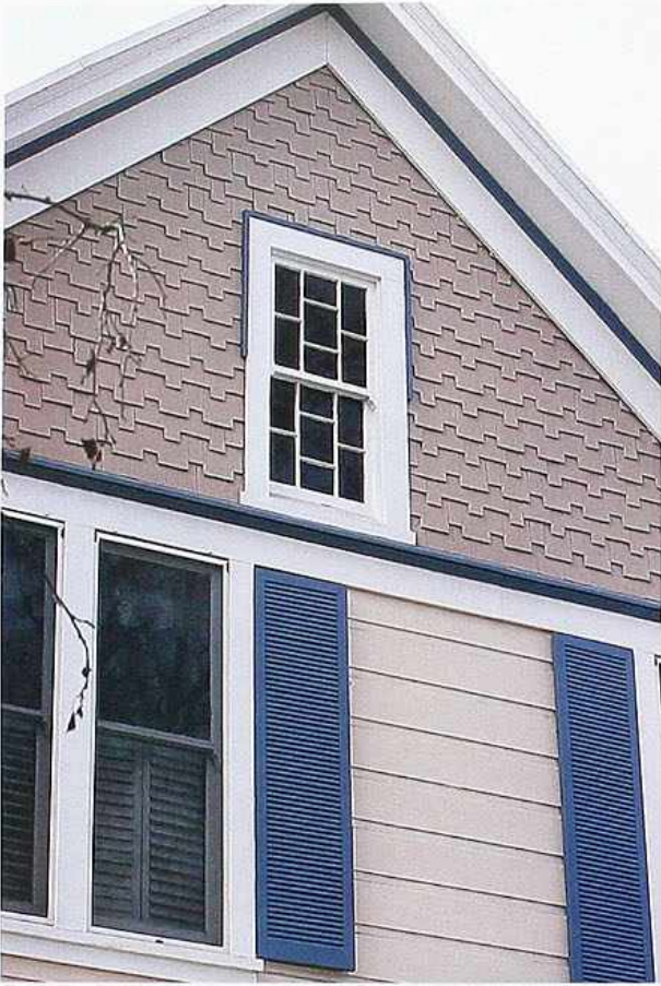
WI-48 Double-hung windows: seven-over-seven decorative lights; one-over-one with shutters
