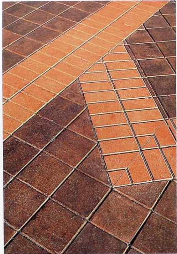
FP-82 Pre-cast concrete pavers; double soldier course in straight-joint-course field; flexible paving, urban public space
