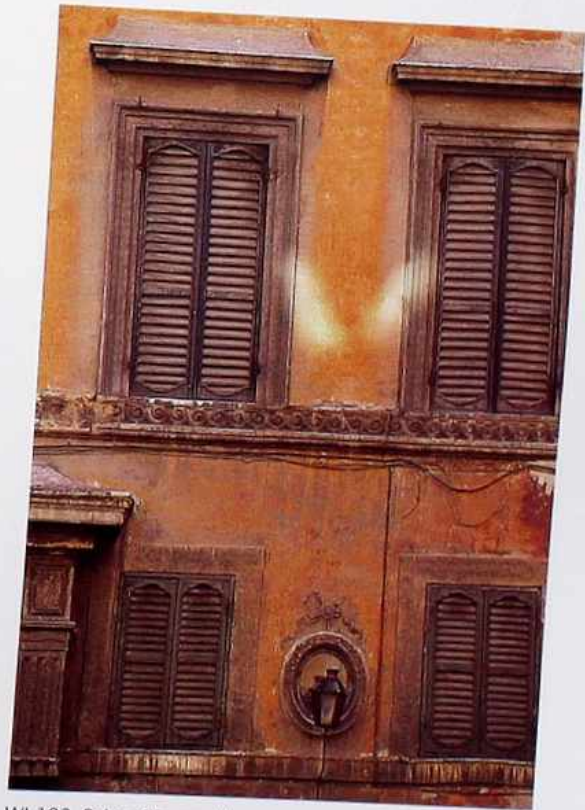
WI-182 Pairs of framed louvered shutters
