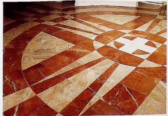
FP-16 Marble parquet in circular radiating design in foyer
