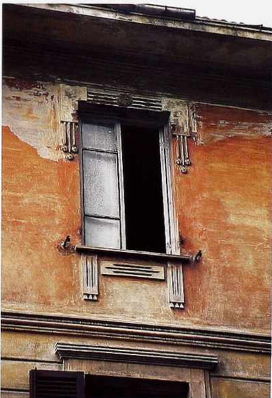
WI-36 Double-casement window in stucco wall
