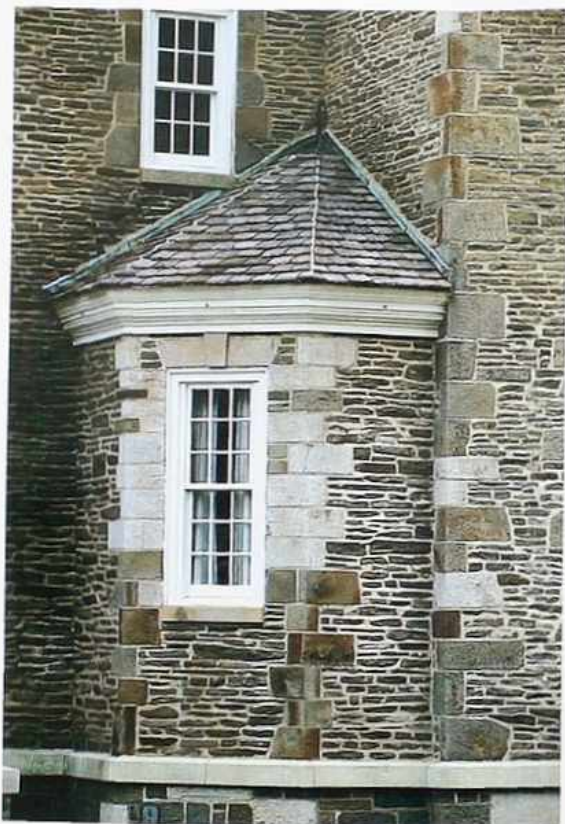
WA-106 Inside-corner turret in coursed rubble with dimension-stone quoins on outside corners and around window
