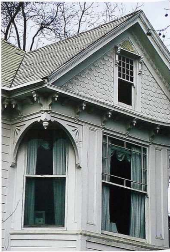
WI-51 Double-hung windows: one-over-one (left); sixteen-over-one (gable); one-over-one decorative-lights (right), 19th-c. clapboard house
