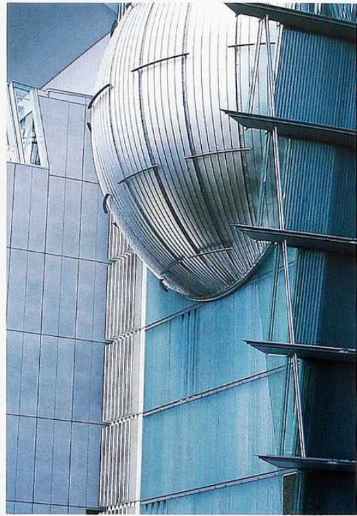
FA-27 Ovoid projection on facade made of custom fabricated metal panels, modern commercial building
