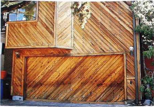
WA-51 Diagonal siding with flat edge trim and corner window, modern house
