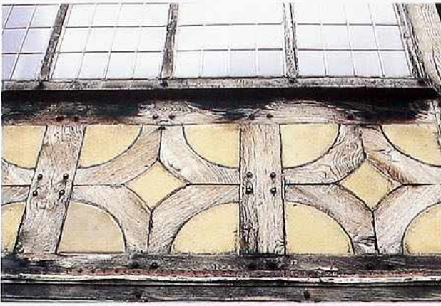
WA-273 Diamond-shaped panels on half-timbered and pegged construction
