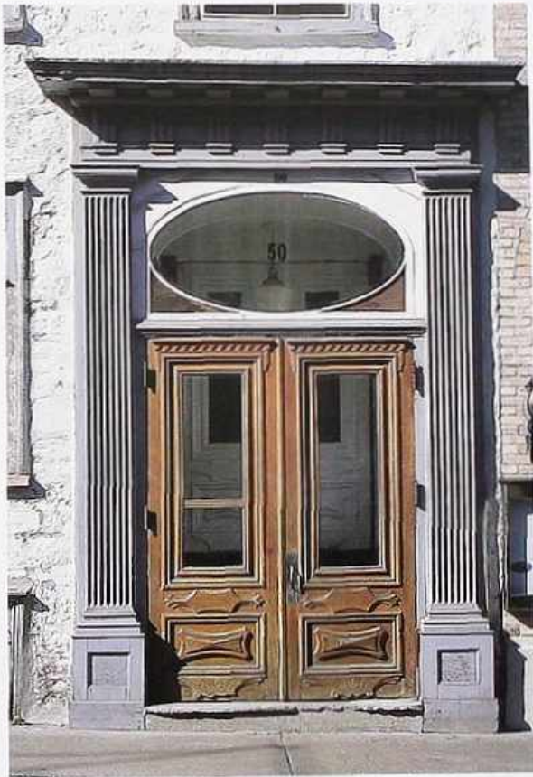
DW-62 Oval transom light over wood paneled doors with single lights; doorframe flanked by Doric pilasters and entablature, 19th-c. apartment house
