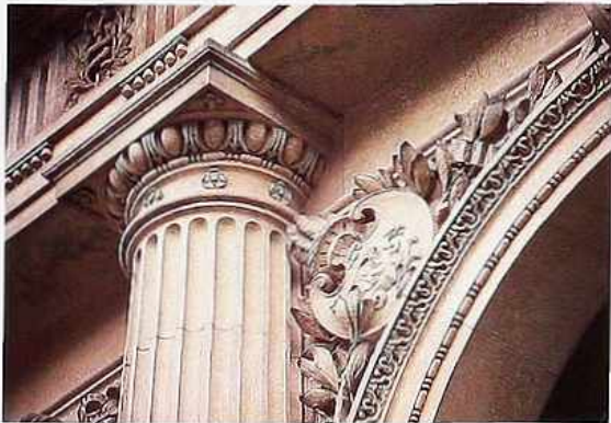
CP-3 Doric capital with Roman styling, egg-and-dart motif in echinus; rosettes on neck of engaged column
