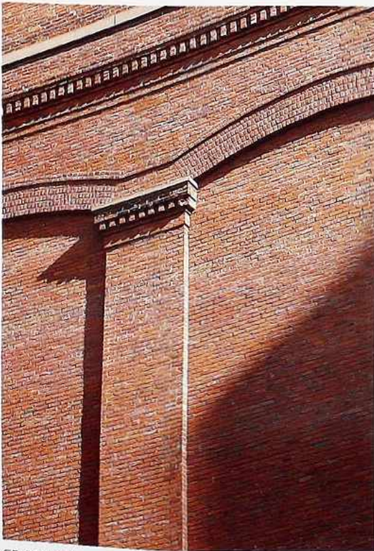
CP-90 Brick pilaster with dentil motif at the capital and blind cambered or very shallow segmental arch; dentilated molding above arch
