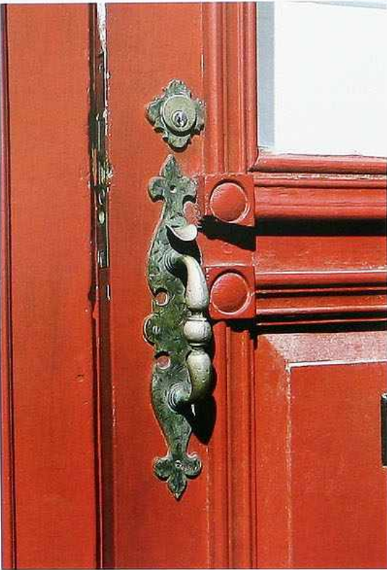
DW-121 Cast naturally patinated bronze door handle with latch and lock
