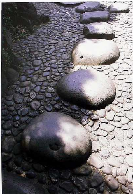
FP-43 Large round boulders surrounded by split natural stones, both set in concrete, garden path
