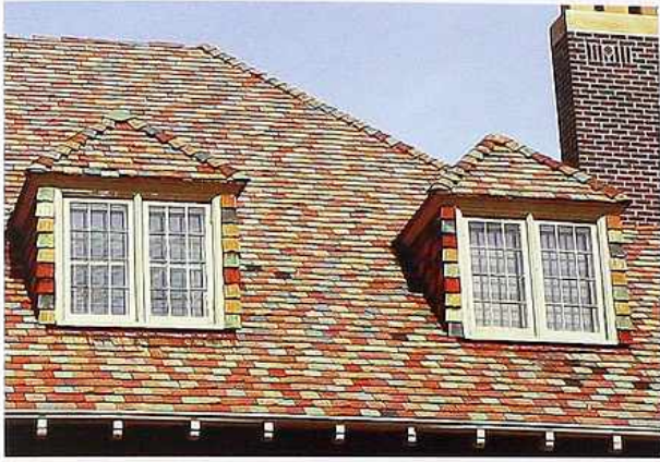
CR-49 Flat multicolored shingle tiles with hipped roof dormers, 20th-c. American house
