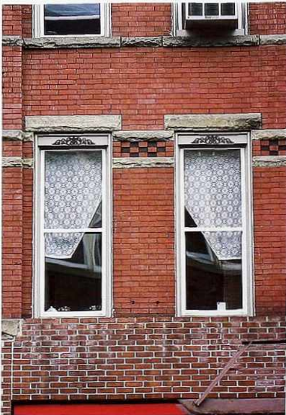
WI-124 Stone lintels and carved casing tops with stone and brickwork band around double-hung windows in brick wall
