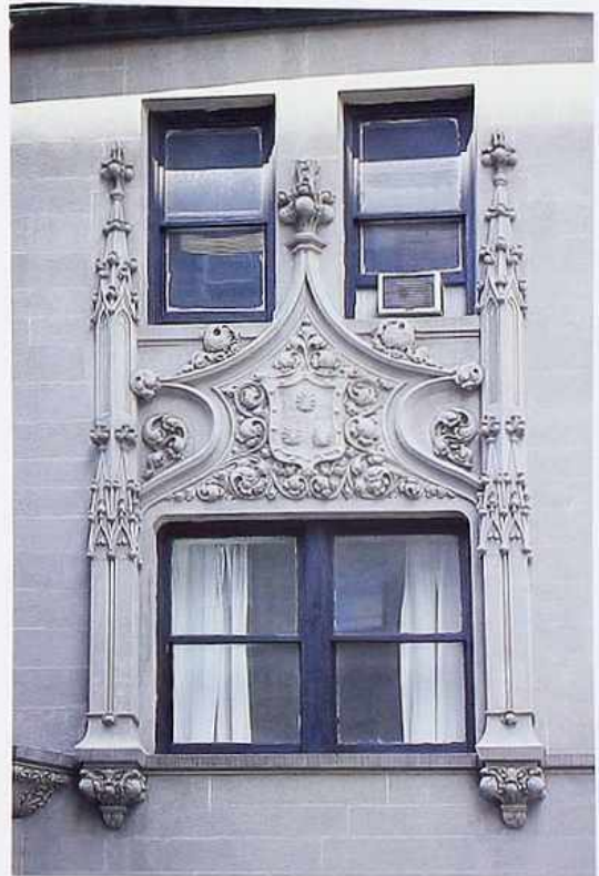
WI-137 Fanciful neo-Gothic spandrel with cartouche flanked by corbelled pilasters, apartment building
