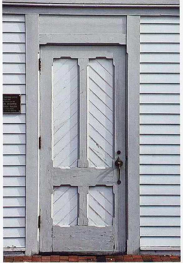
DW-10 Four diagonally planked panels, painted door with wrought-iron handle, clapboard house
