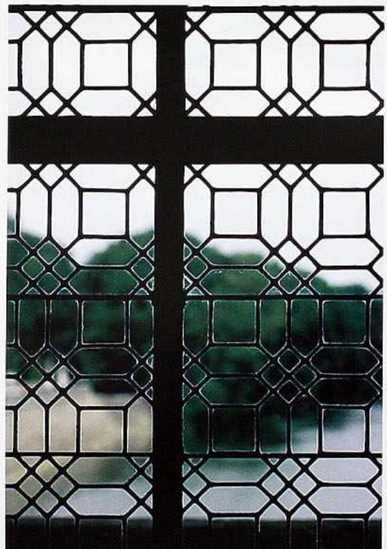
WI-4 Leaded glass with octagonal brass muntins in interlocking pattern
