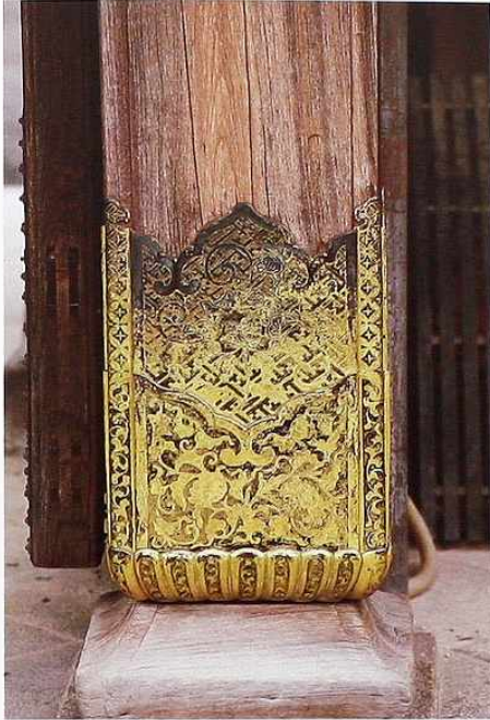
CP-54 Gilded relief ornamental metal sheath covering the base of a timber post
