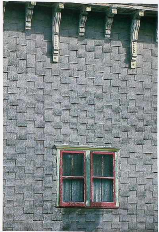
FA-54 Bituminous shingles in staggered course below bracketed cornice
