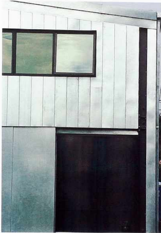
FA-7 Metal-clad modern house. Top: adjacent vertical strips; strip window; bottom: flush panels (left); contrasting metal entry (right)
