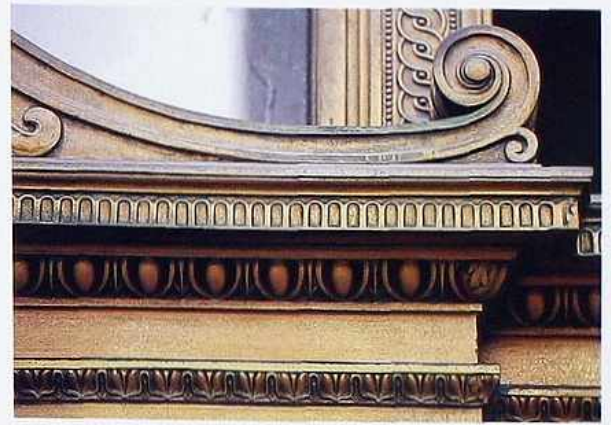
OM-5 Volute on bronze scrolled pediment. Molding, top to bottom: corona with band ornament; egg-and-dart ovolo; tongue-and-dart cyma reversa
