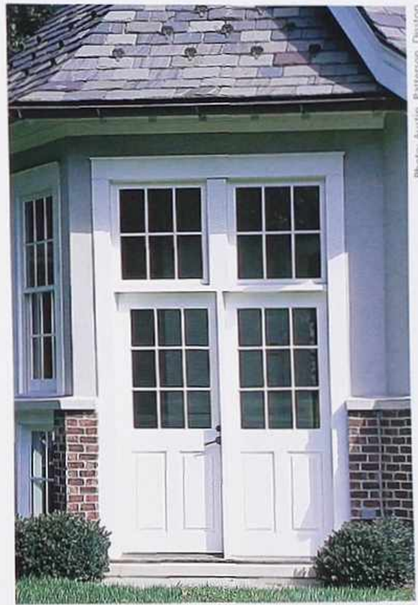
DW-63 Six-light double transom panels over nine-light painted wood double doors with center post, traditional house
