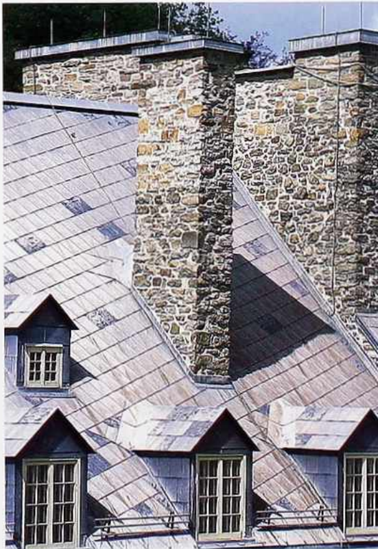
CR-153 Coursed-rubble chimney
