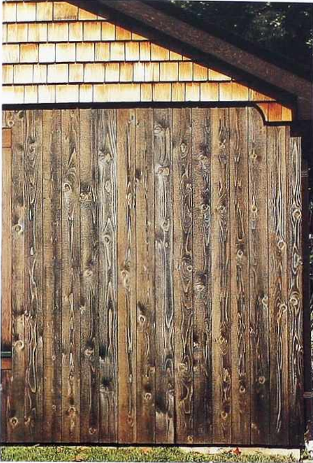
WA-15 Vertical board siding with new cedar shakes on gable, residential garage
