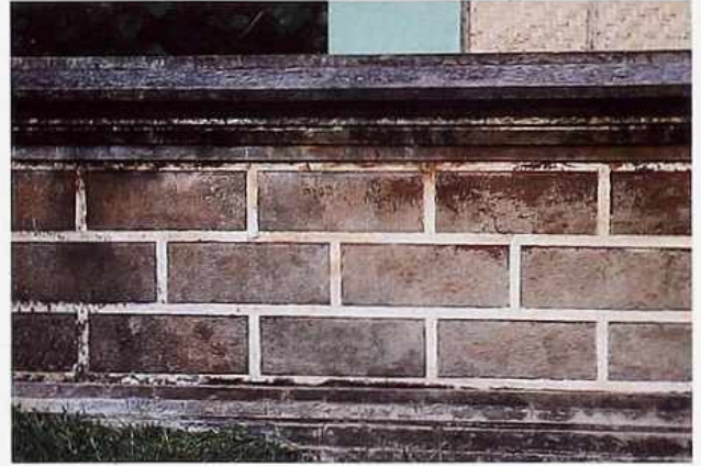
WA-224 Stucco finish applied in rectangular concrete framework imitating masonry in running bond
