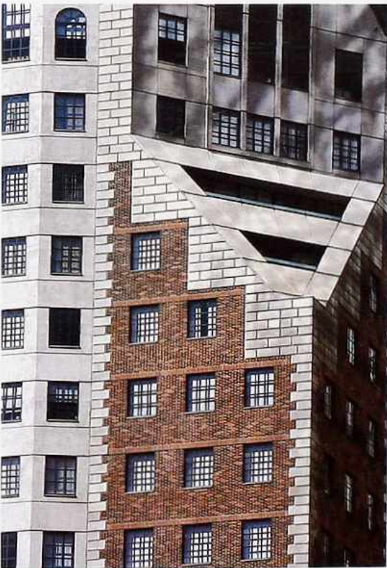
WA-304 Stone veneer and brick wing with stone-veneer quoins, modern commercial building
