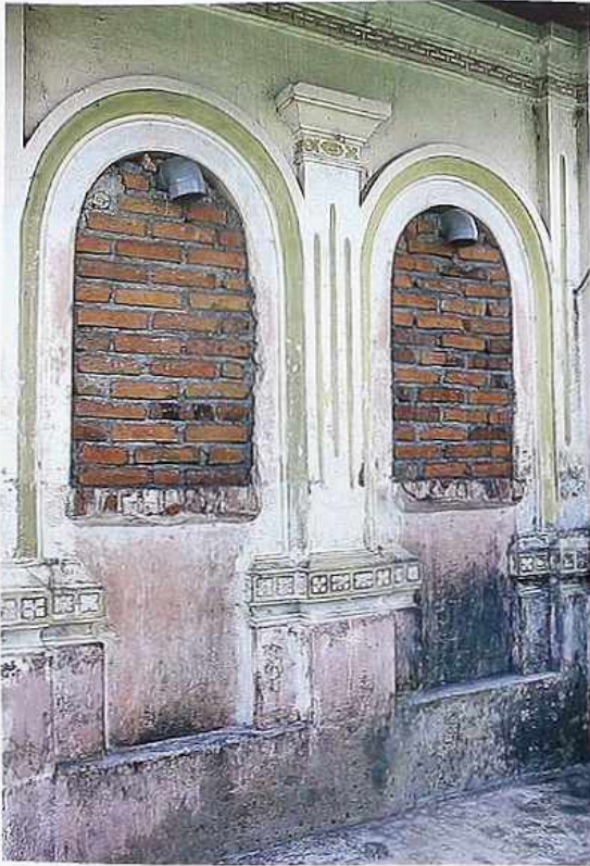
CP-88 Weathered painted pilasters in a blind arcade with semicircular arches
