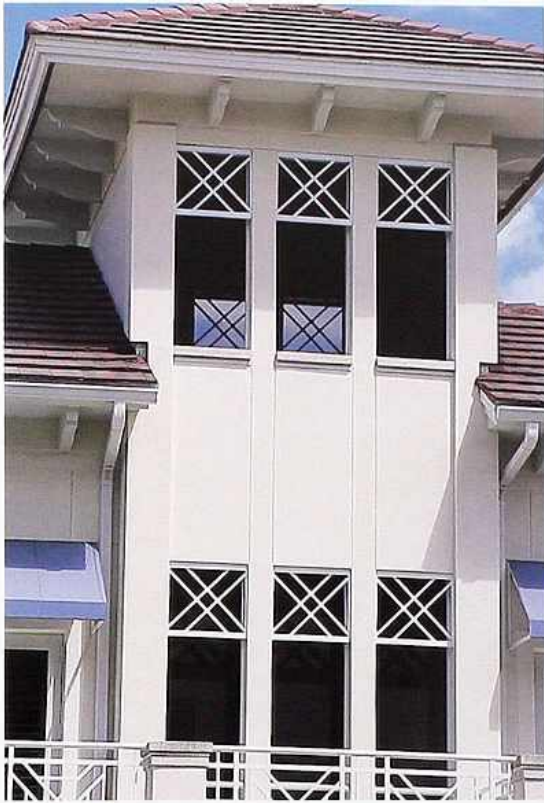
WI-69 Fixed windows with lattice in top lights, modern house
