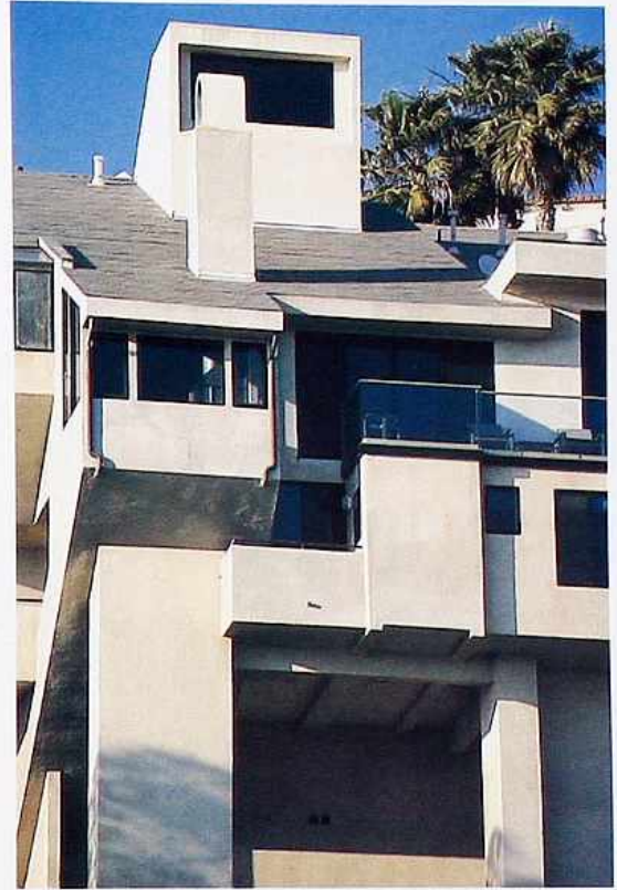
WA-245 Painted smooth stucco, modern house
