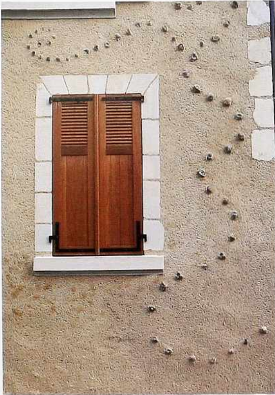
WA-230 Stucco with dimension-stone window and corner quins and natural stone insets in serpentine design; louvered shutters, house
