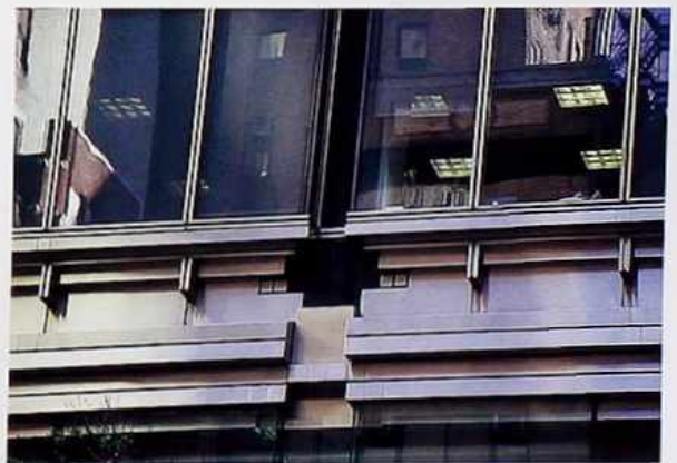
OM-78 Metal fascia bands suggesting a classical entablature, broken at the division between bays (detail of OM-75)
