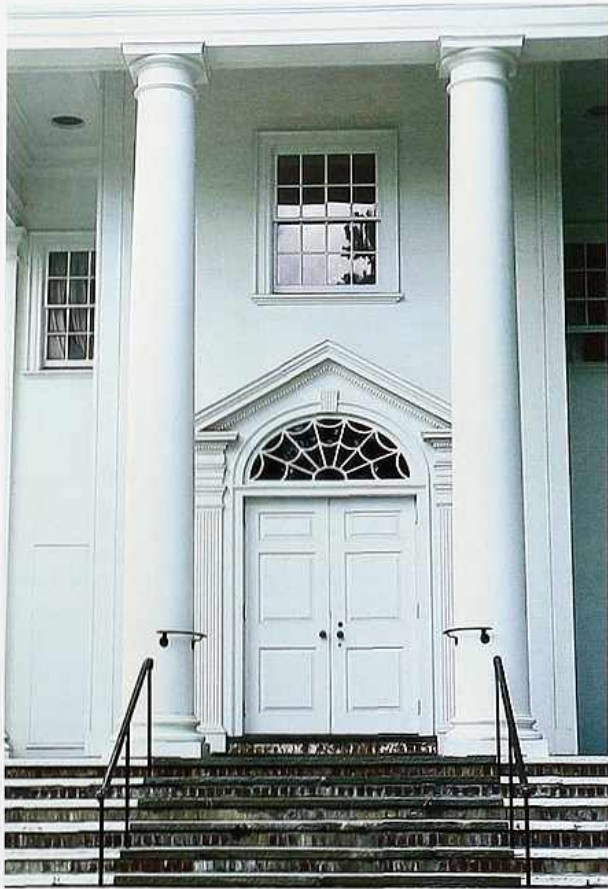
CP-73 Roman-style Doric columns with Attic base supporting portico; pedimented door
