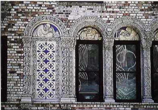
WI-144 Framed bas-relief tympanums and ornamented pilasters around windows; blind-arch window with glazed tile
