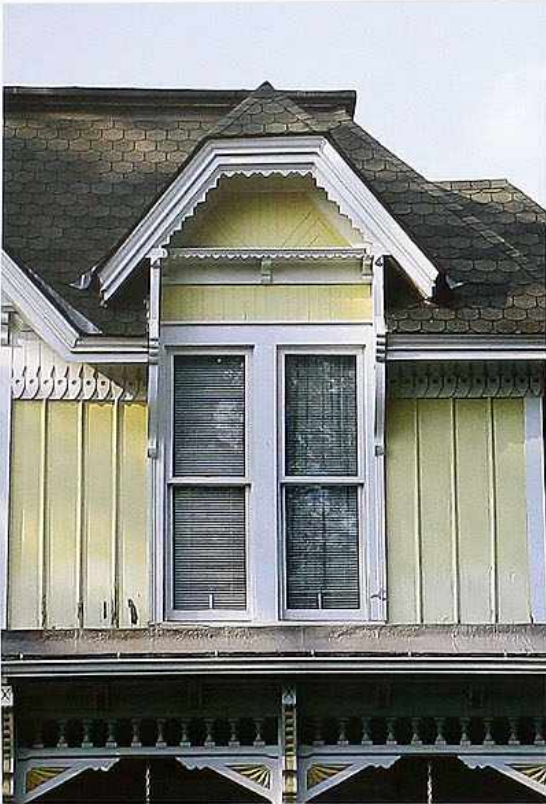
CR-76 Wall dormer with jerkinhead roof
