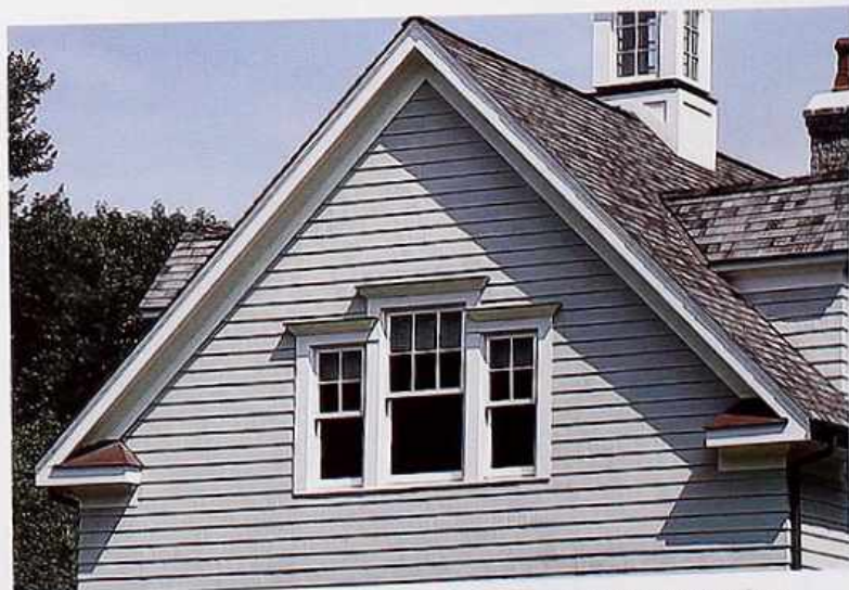
WI-117 Set of three gable wall double-hung windows; flat wood casings, with crown molding caps
