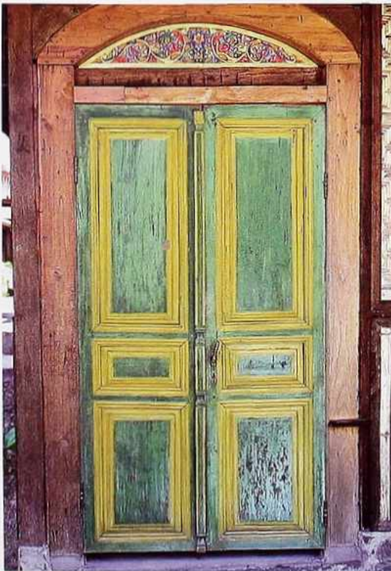
DW-39 Three-panel double doors with painted panels and painted carved ornament; segmental arch transom, Bali
