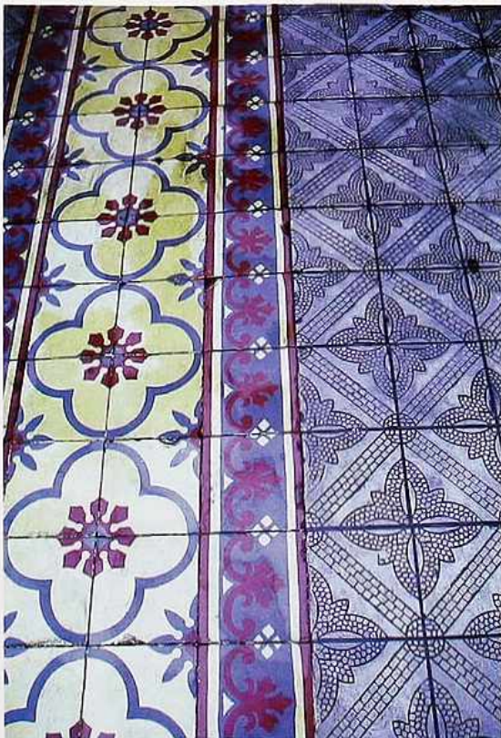
FP-105 Decorated glazed tile, straight-jointed, forming diaper patterns, and a running-repeat border
