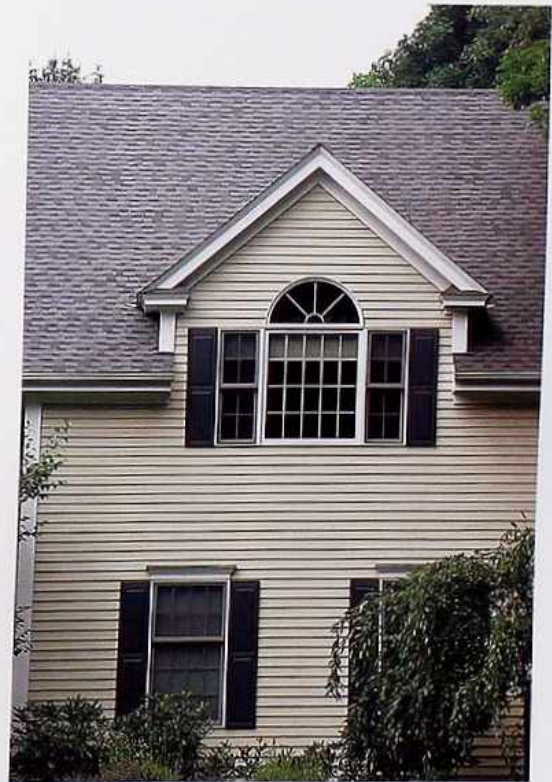
CR-92 Gabled wall dormer with Palladian window
