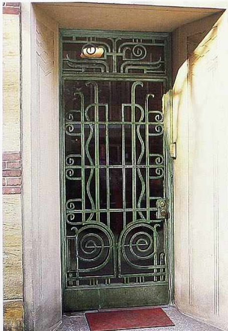
DW-114 Wrought-iron gate recessed in wall
