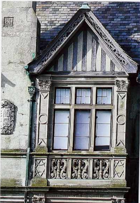
WI-138 Set of three dormer windows with stone casing flanked by pilasters in half-timber-style gable with engaged balustrade
