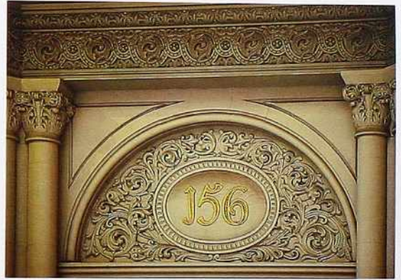
OM-25 Tympanum with foliated ornament, concave oval cartouche with gilded building number
