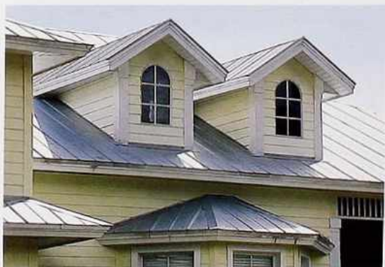
CR-103 Gable-roof dormers with deep eaves
