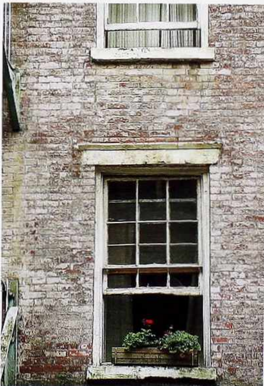
WI-46 Six-over-six double-hung window with stone lintel in weathered brick wall
