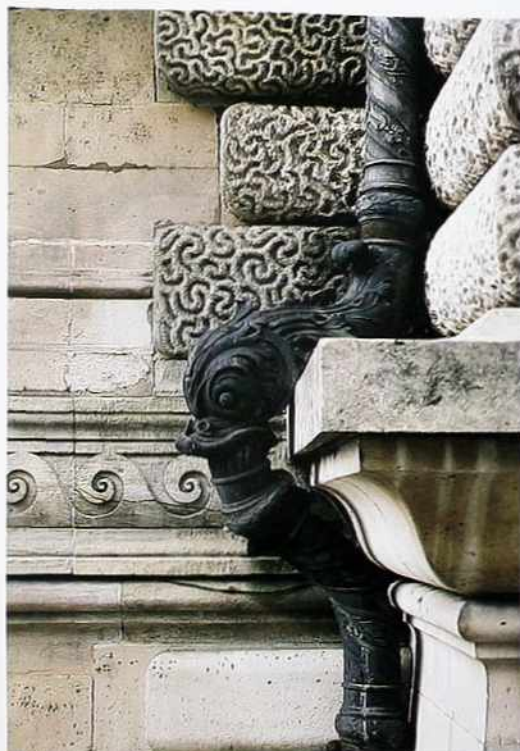
CR-158 Copper drainpipe and rainwater head
