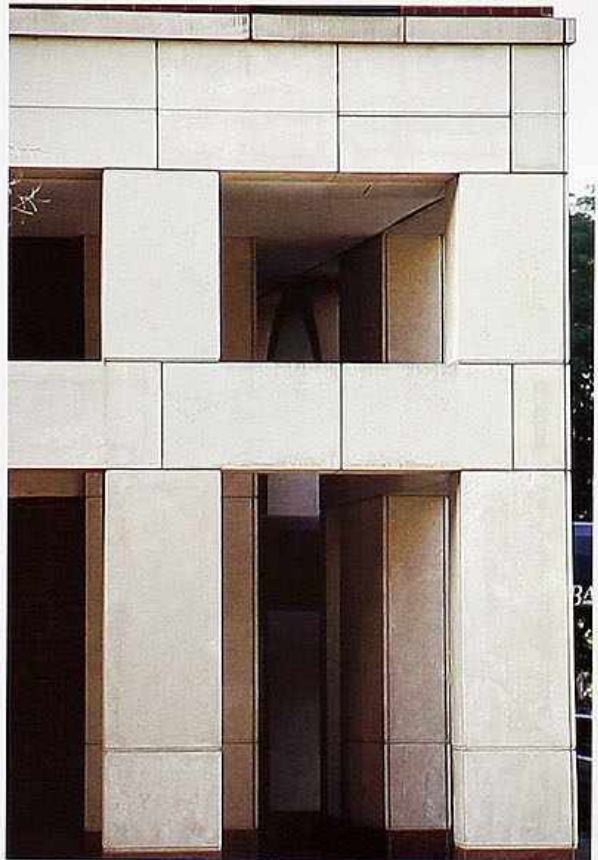
CP-133 Trabeated arcade (post-and-lintel construction), modern commercial building
