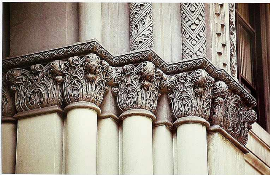
CP-20 Romanesque capitals on a series of pilasters and jamb-shafts in compound arch
