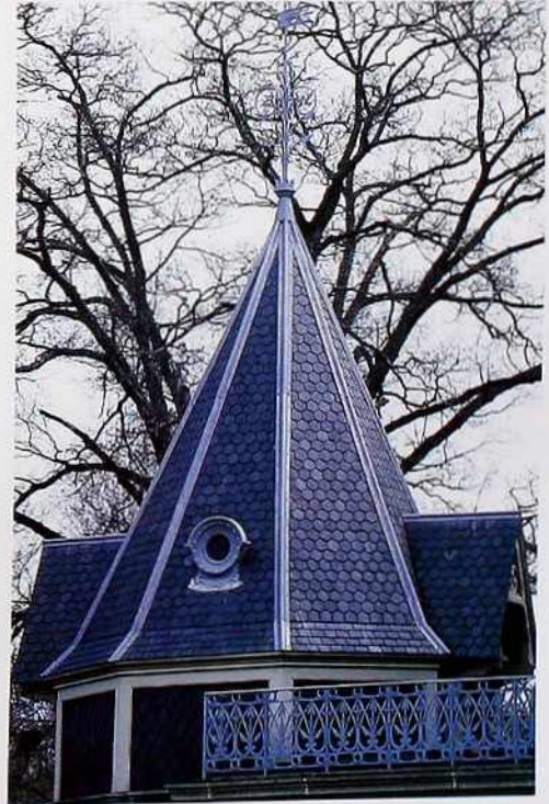
CR-133 Pyramidal octagonal roof on turret, cross-gable dormers
