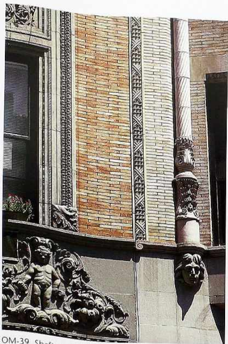
OM-39 Shaft on a mascarón bracket. At left, foliated sculptural panel with a cherub
