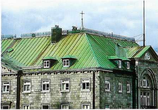
CR-115 Hipped, copper with standing seams; hipped-roof dormers (left) and pedimented wall dormer (right)
