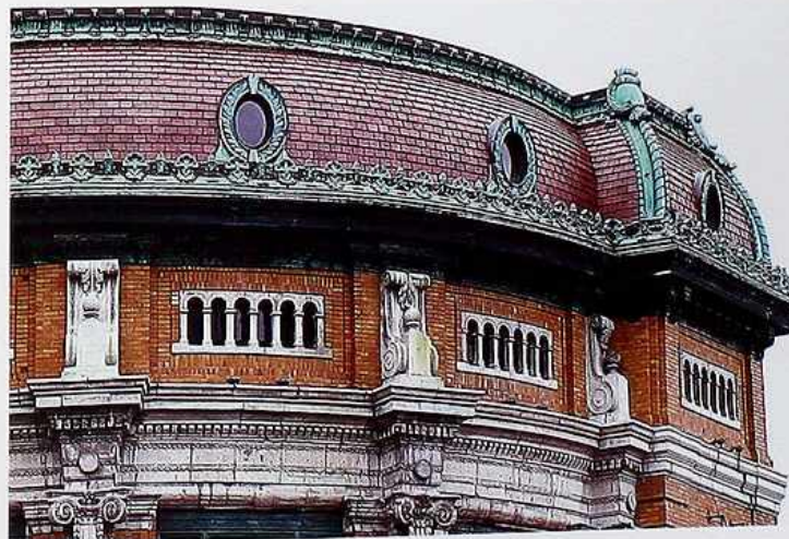
CR-53 Flat shingle tiles on convex curved roof with copper molding, 19th-c. mixed-use building
