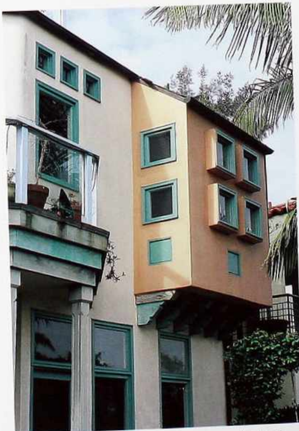
WI-92 Oriel with awning or fixed windows, shed roof, and corbels, modern apartment house
