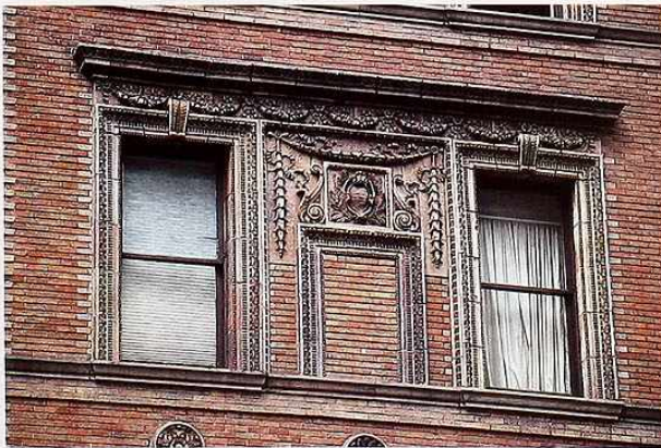
WI-128 Terracotta cornice with garlands around windows with terracotta casings; blind window under cartouche
