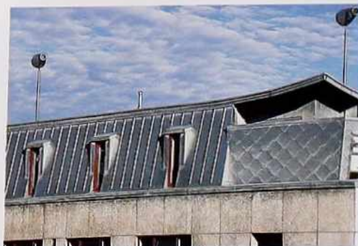
CR-104 Shed-roof dormers on gambrel roof
