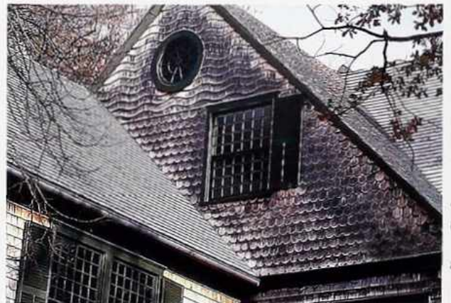
FA-50 Cut shingles on gable. Top: wave pattern around bull's-eye window; bottom: fish-scale pattern
