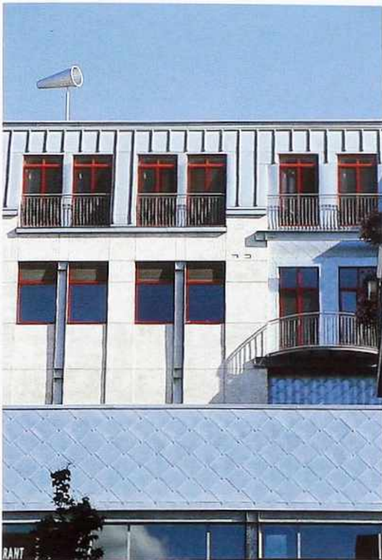
WA-302 Top to bottom: batten-seam metal cladding; cast concrete or stone; metal shingles; metal-framed glass, modern commercial building
