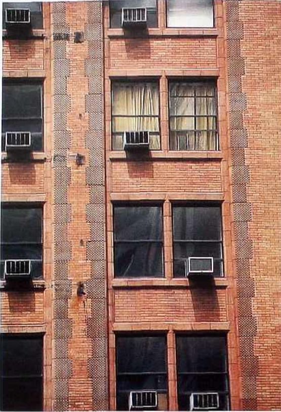
WA-197 Brick window-wall with recessed spandrels, brownstone window trim and quoins
