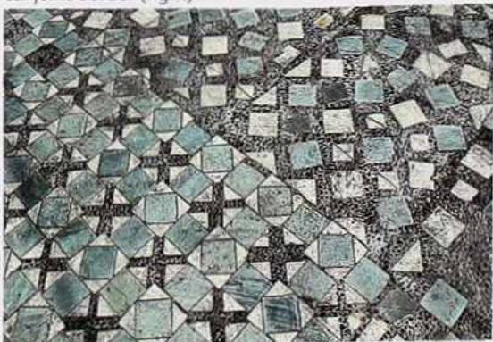
FP-101 Square and triangular ceramic tiles set in exposed-aggregate field in geometric and random patterns, entryway
