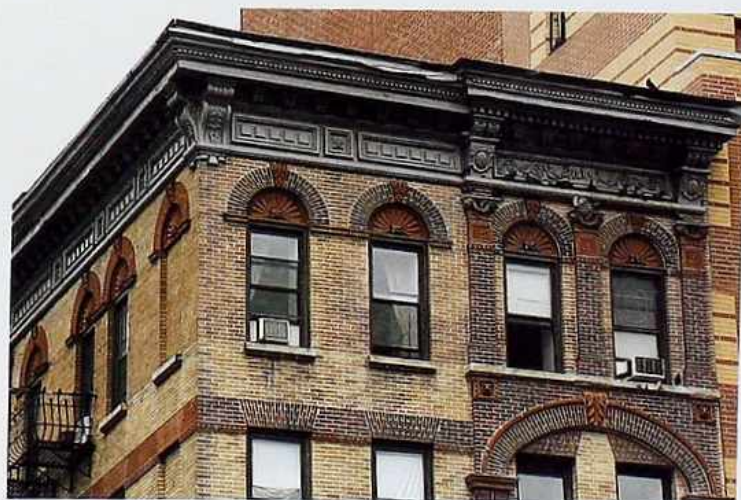
WA-188 Contrasting brick banding and pilasters; gauged-brick semicircular arches on upper windows, 19th-c. apartment house
