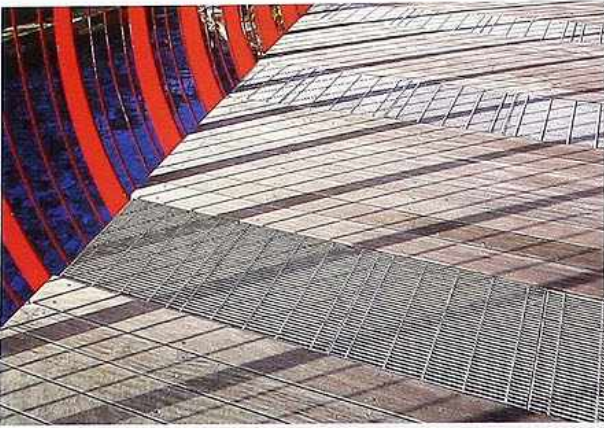
FP-8 Grooved weather-treated wood decking alternating with metal grates, urban public space
