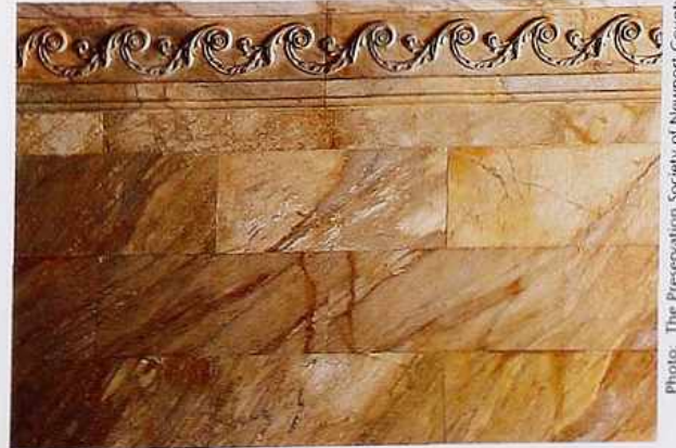
WA-71 Siena marble in running bond with Vitruvian scroll frieze on hallway wall
