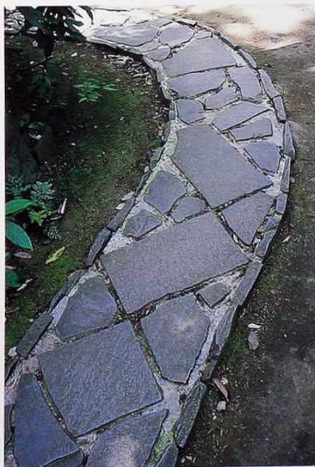
FP-50 Roughly squared paving stone in diamond pattern with border, garden path
