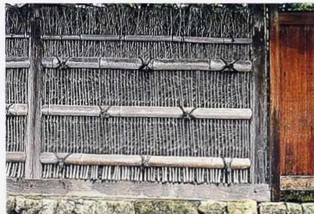
WA-12 Woven bamboo twigs tied to bamboo post and rails, garden fence
