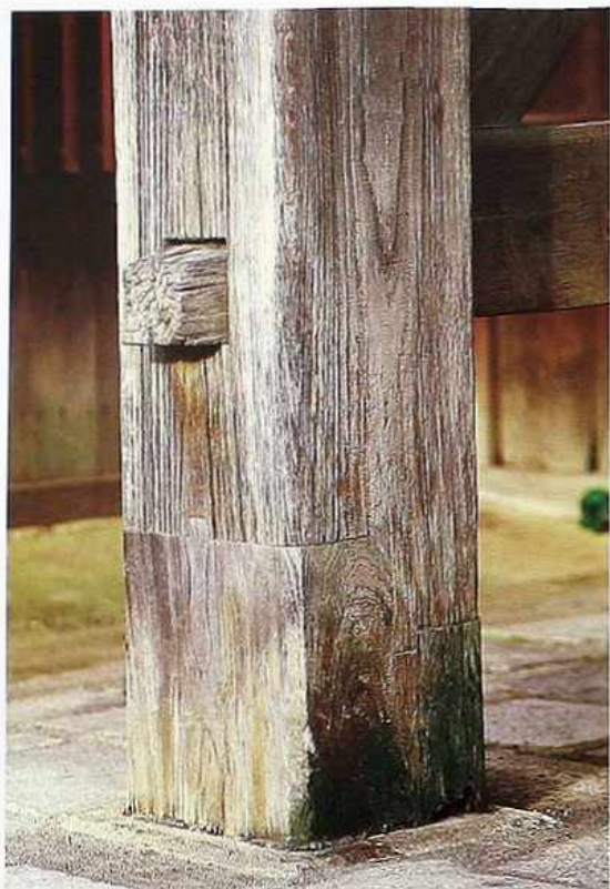
CP-105 Timber post with mortise-and-through-tenon joint
