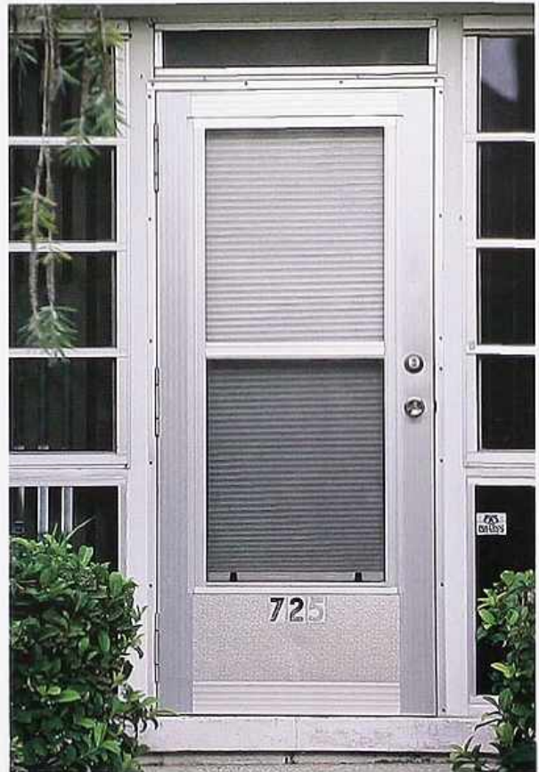
DW-59 Brushed aluminum door with two lights in metal frame with transom light, modern apartment house
