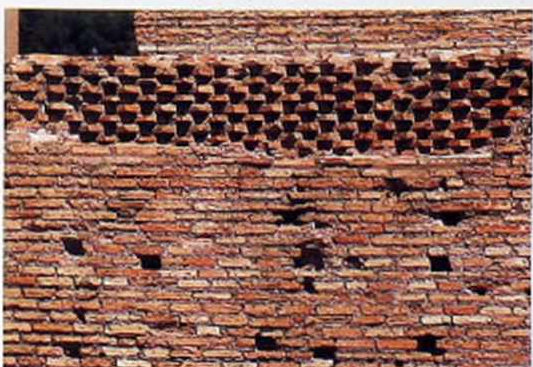
WA-163 Ancient Roman brick wall with structural dog-tooth course exposed by weathering of brick facing layer
