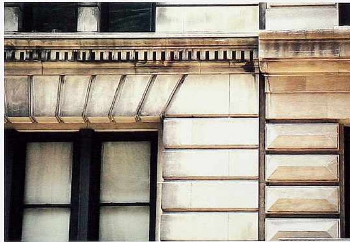
WA-87 Limestone walls. Left: bevel-cut stack bond with jack arch and dentil cornice; right: gem-cut stack bond
