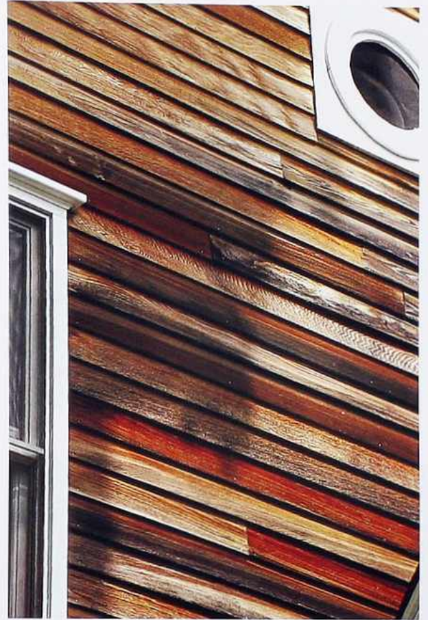
WA-16 Detail of unpainted clapboard and window casing
