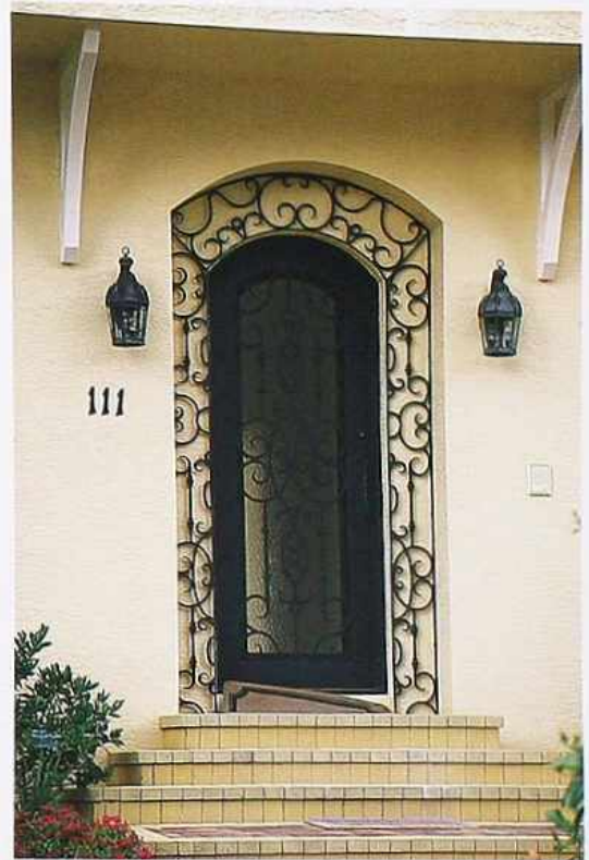
DW-91 Door hood over arched doorway framed with wrought-iron filigree band; metal door with grille over full glass, modern house
