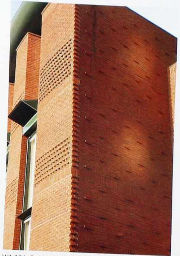
WA-194 Corner detail of custom bond with dog-tooth banding and diaper pattern of projecting stretchers, modern apartment house
