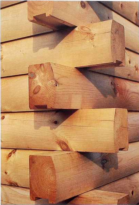
WA-5 Pine log house construction, corner detail
