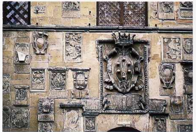
OM-31 Large cartouche surmounted by a crown, with molded frame with crossettes, surrounded by smaller cartouches of similar design
