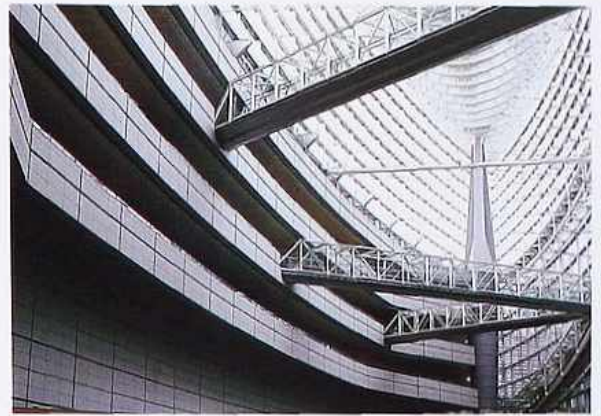
CR-17 Elliptical atrium of metal-framed glass with pedestrian bridges, modern commercial building
