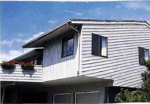
WA-53 Horizontal and vertical board siding with angled siding aligned to roof rake, modern house
