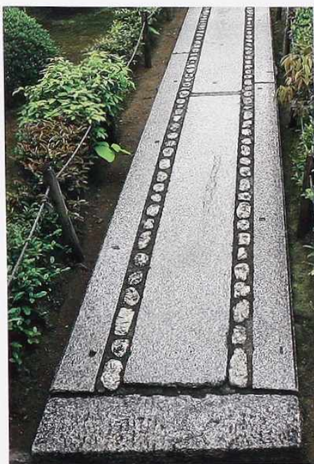
FP-48 Squared granite blocks with split-stone inset on garden path
