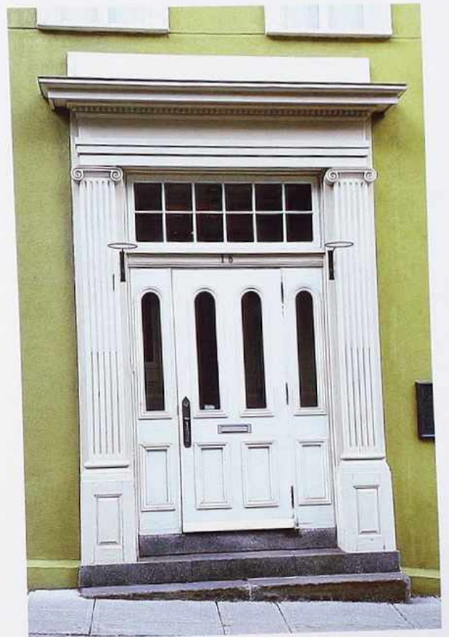
DW-70 Paneled double doors and side lights with lancet-shaped lights and twelve-light transom; letter slot; ionic-style pilasters and entablature
