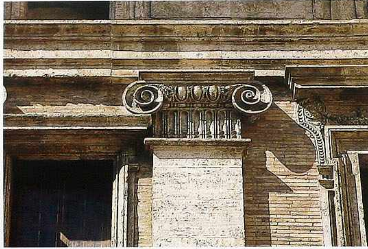
CP-25 Ionic capital with fluted necking on pilaster
