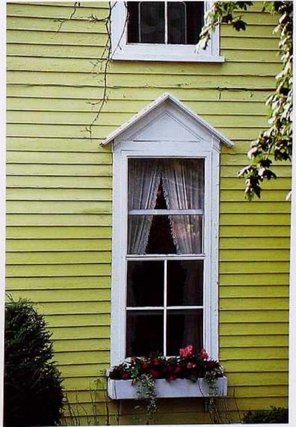
WI-110 Wood gable-shaped hood over double-hung window, American clapboard house
