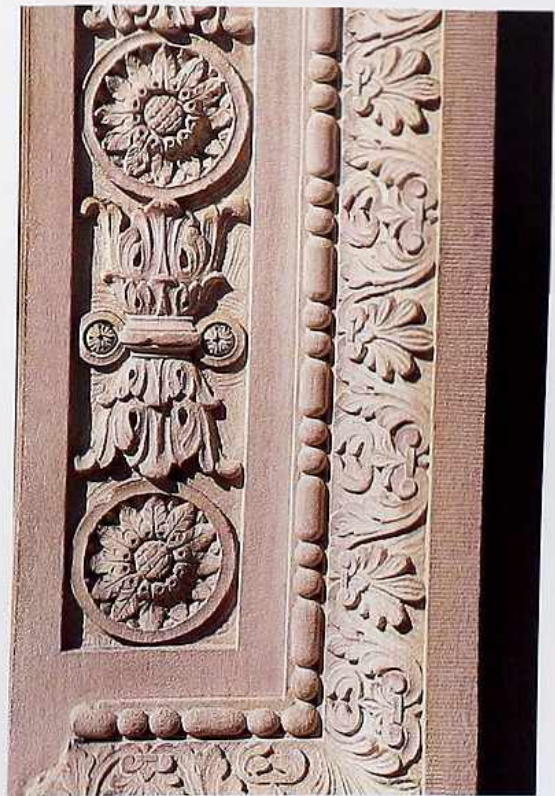
OM-66 Corner detail of enriched ovolo molding with trailing foliated pattern; bead-and-reel framing foliated design flanked by rosettes
