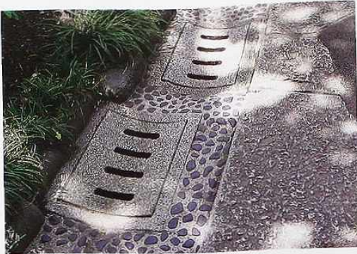
FP-113 Pre-cast exposed-aggregate drain grates in gutter beside a walkway, urban park
