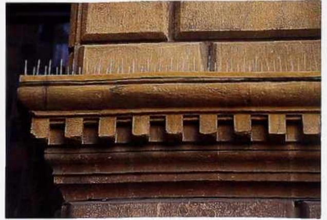
OM-70 Cornice. Top to bottom: plain ovolo molding, dentil band, plain cyma reversa, plain cyma recta
