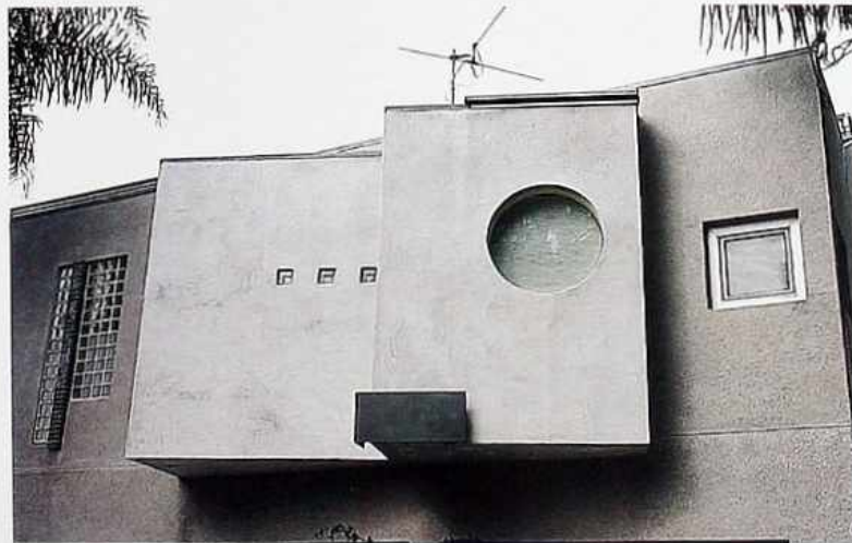
WA-216 Concrete projecting window, modern house
