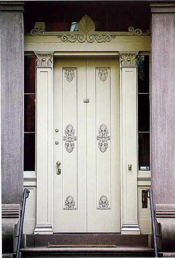
DW-9 Two panels with applied trim; pilaster doorframe with anthemion on lintel; transom light and side lights
