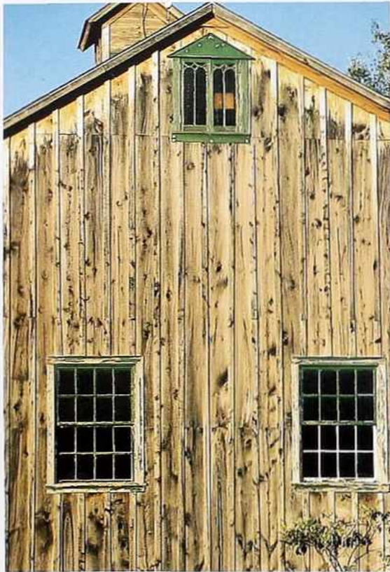
WA-28 Gable-end wall with unpainted board-and-batten siding and gable window
