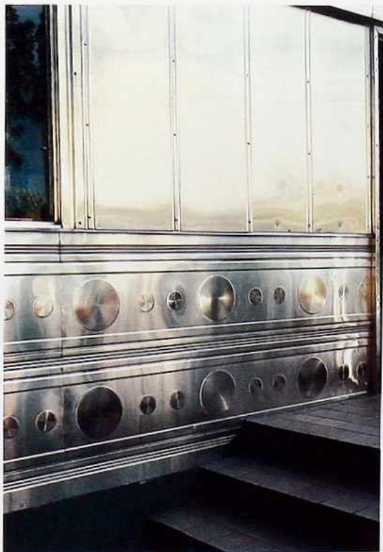
FA-9 Brushed stainless steel cladding with stamped ornamental moldings and exposed fasteners, American diner
