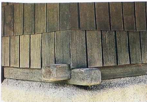
WA-9 Notched corner joint of square timber frame with painted cedar shakes on concrete foundation
