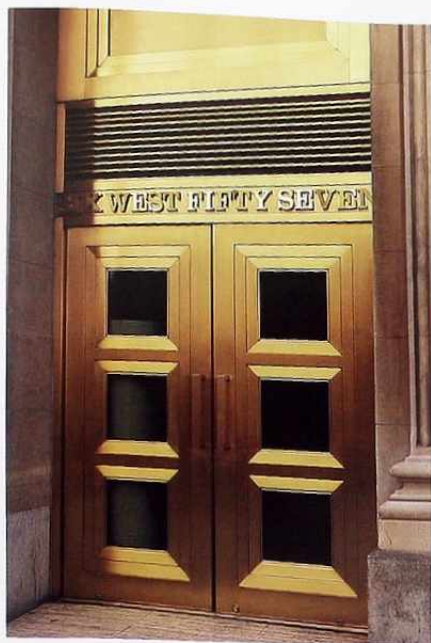
DW-45 Brass three-paneled double doors, panels with lights and framed with molding; louvered brass transom panel
