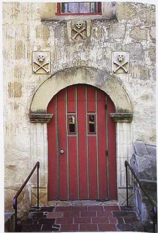
DW-77 Segmental arch with molded imposts over painted plank door; skull ornament in stucco surround, 19th-c. American Southwestern mission
