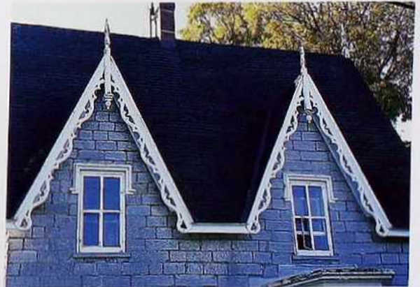
CR-85 Double wall dormers with gingerbread-style decorated bargeboard, 19th-c. American stone house
