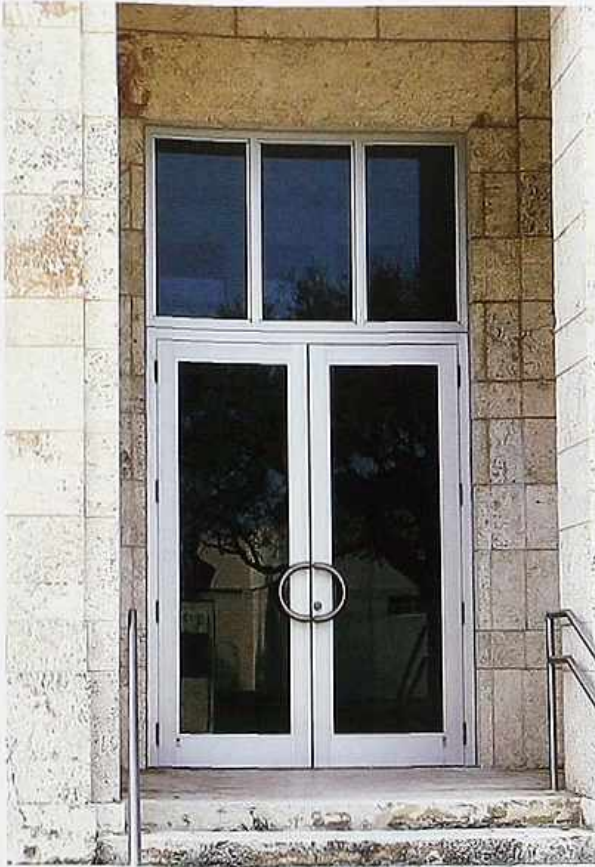
DW-58 Full glass double doors in stainless steel frame with three-light transom in recessed entryway; stone surround and steps, modern commercial building
