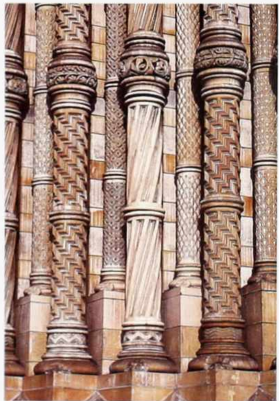
CP-68 Gothic-style jamb-shafts with annulets, varied shaft treatments: spiral fluting and stepped helical geometric pattern
