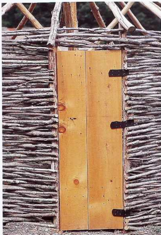
DW-24 Plain-sawn plank door with wrought-iron strap hinges; woven wood walls, 18th-c. corn crib
