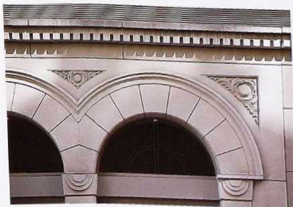
CP-142 Semicircular arches with voussoirs and archivolt, carved spandrel, and dentilated molding
