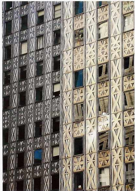
FA-14 Curtain wall; spandrel panels with dimensional geometric pattern, modern commercial building
