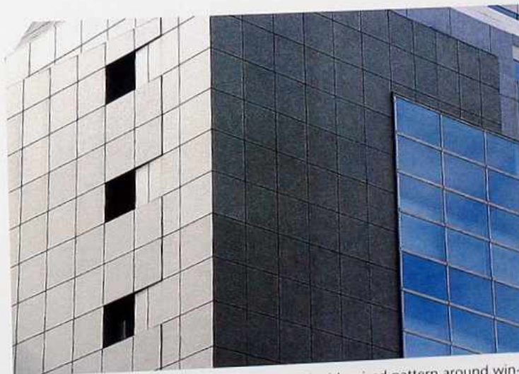
WA-137 Honed-granite veneer in stack bond with raised pattern around windows, modern commercial building
