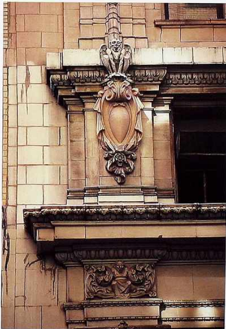
OM-45 Cartouche surmounted by antic. Enriched molding, top to bottom: foliated cyma reversa; foliated cyma recta; egg-and-dart ovolo; tongue-and-dart; bead-and-reel
