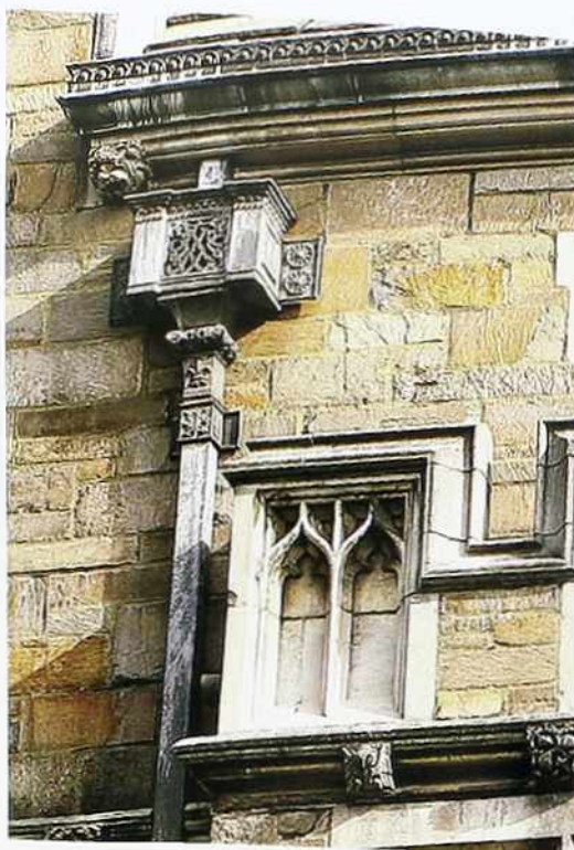
CR-156 Metal decorated gutter, rainwater head, and drainpipe
