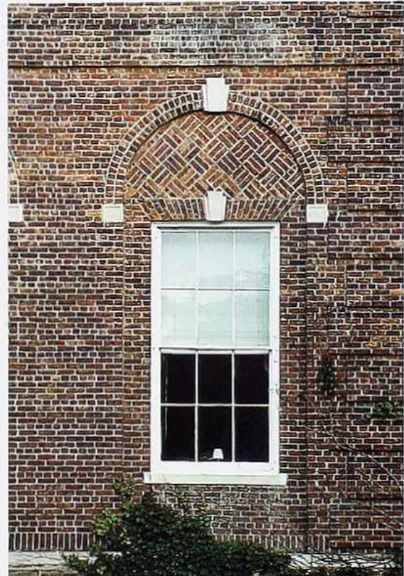
WA-178 Common bond with fourth-course header, blind arch of diagonal basket-weave over window, and raised quoin corners
