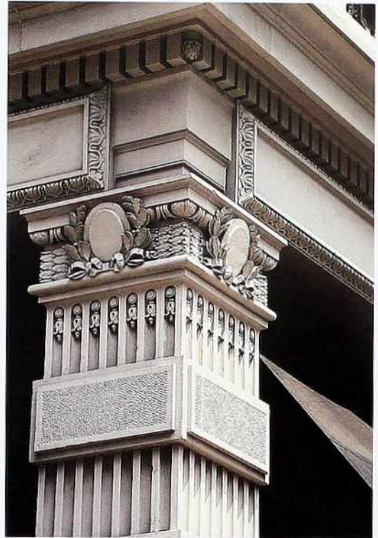
OM-106 Three-banded architrave, plain shallow soffit; raised panels surrounded by leaf-and-dart molding over architrave
