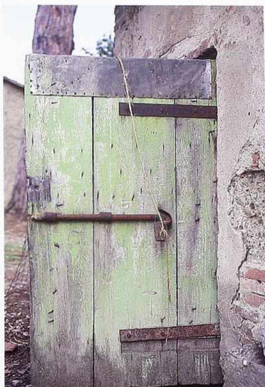
DW-33 Weathered painted wood-plank door with rustic iron strap hinges and latch, farm courtyard
