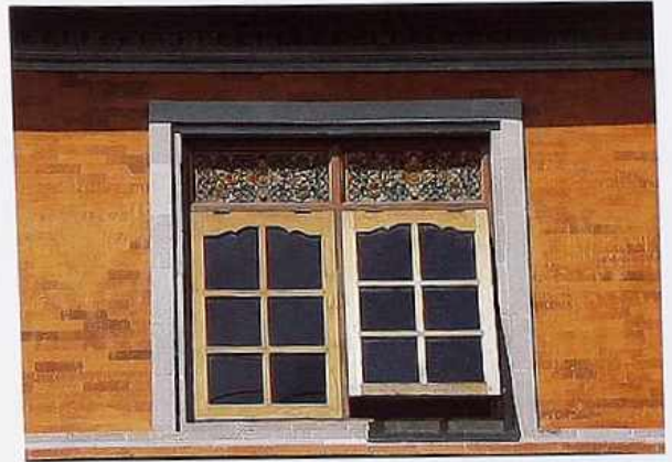
WI-26 Wood-framed awning windows with carved transom panel, Balinese house
