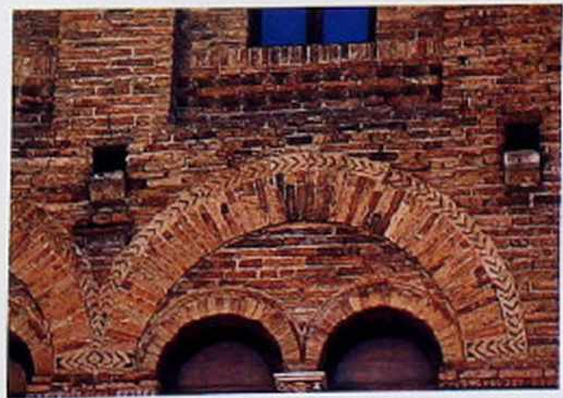
WA-164 Medieval arcade under relieving arch in gauged brick with chevron-decorated extrados and recessed spandrels
