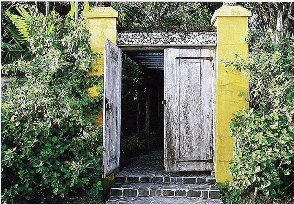
DW-109 Garden entrance with wood-paneled doors in a stucco wall
