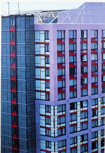
FA-131 Trabeated facade with multicolored infill and spandrel panels, modern commercial building
