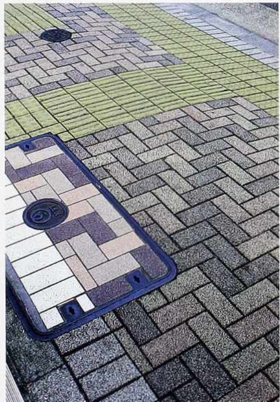
FP-84 Polychrome pre-cast concrete pavers in herringbone and banded patterns, urban street
