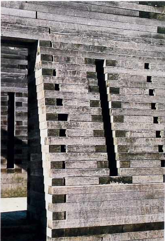
WA-49 Fortification-style battered wall with lapped-joint corners
