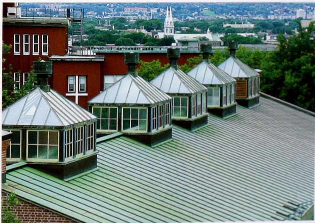
CR-36 Sheet metal with standing seams on gable roof and glazed monitors, modern commercial building
