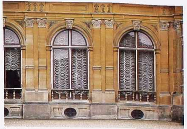
WI-99 Semicircular-arch transom lights over French doors in stone surround with keystones and pilasters, English house
