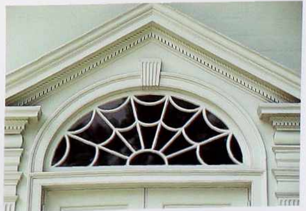
WI-103 Bat-wing fanlight under pediment
