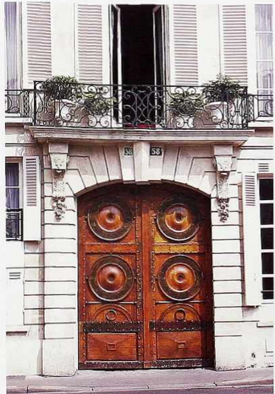
DW-75 Stone segmental arch with carved wood double doors; keystone and corbels supporting a balcony, Parisian apartment house
