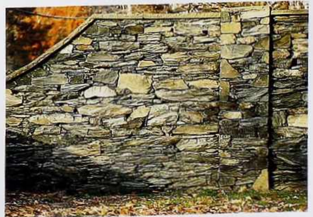
WA-81 Coursed rubble drywall with pilaster and flagstone coping
