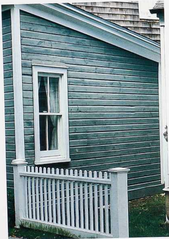
WA-38 Painted tongue-and-groove siding on shed-roofed house with corner board and rake trim
