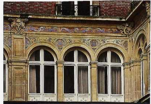
WI-143 Series of arches, pilasters, and polychrome terracotta or stone spandrels framing windows in stone casing, 19th-c. French mixed-use building
