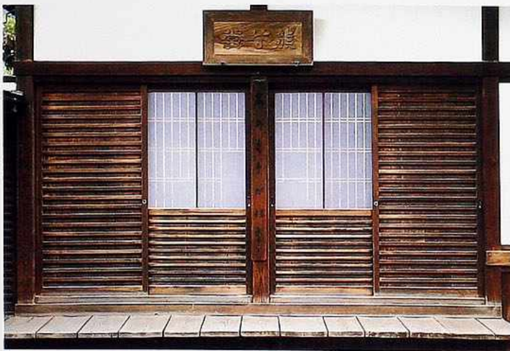
WA-46 Timber frame with infill of planks and battens with sliding doors and paper-covered windows
