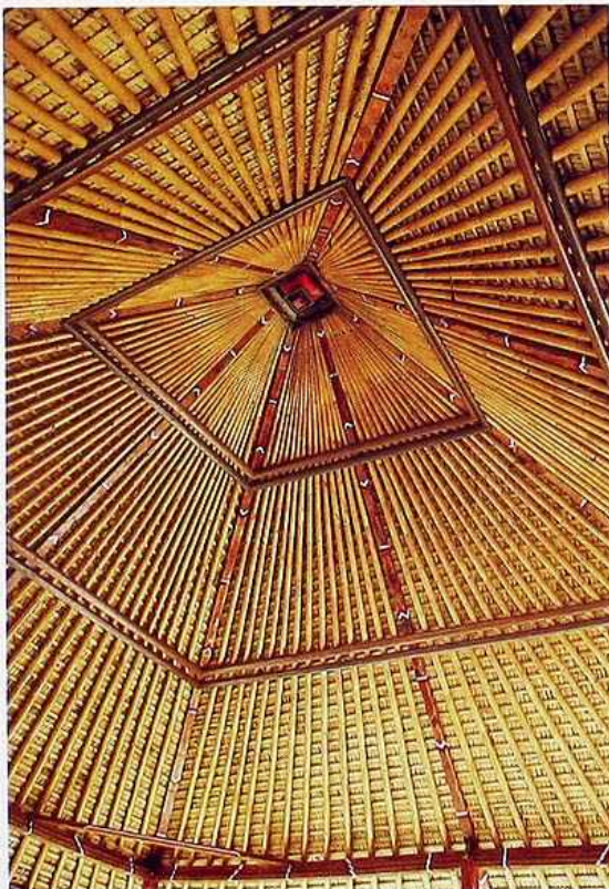
CR-3 Grass thatch roof showing connection between thatching and structure
