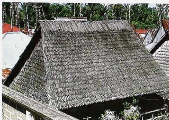
CR-66 Split bamboo shingles on gabled roof, Indonesian house
