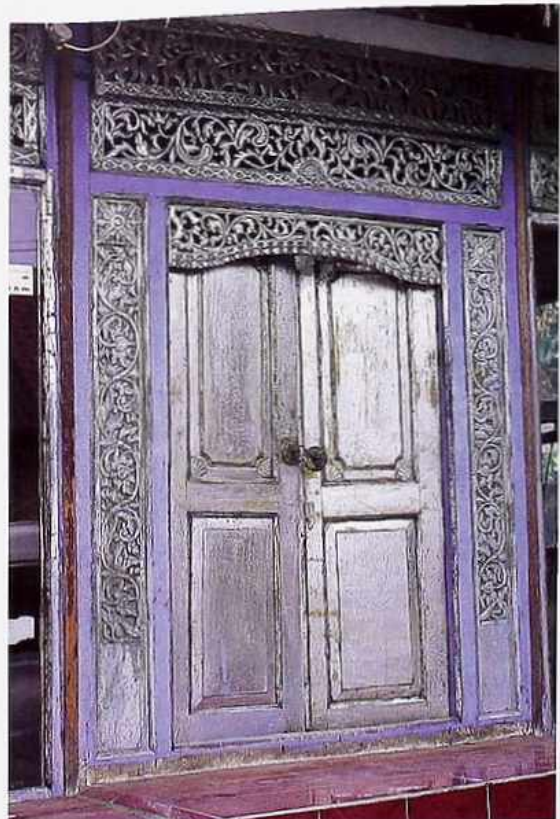
DW-40 Two-panel double doors with raised panels, carved side panels, and pierced carved transom, all with metallic paint
