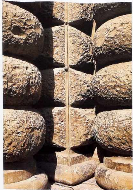
WA-90 Corner detail of rusticated stone pilaster between banded engaged columns
