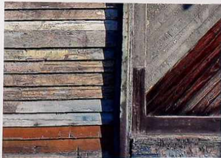
FA-101 Weathered painted clapboard and siding with diagonal board framed door
