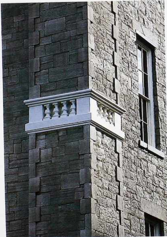
WA-99 Outside corner of split-faced, random ashlar with raised sand-finished quoins and engaged balustrade
