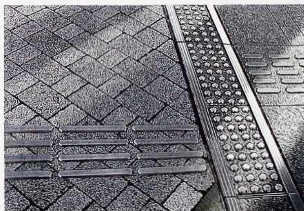
FP-109 Metal safety-paving brads and strips applied to granite pavers, urban public space
