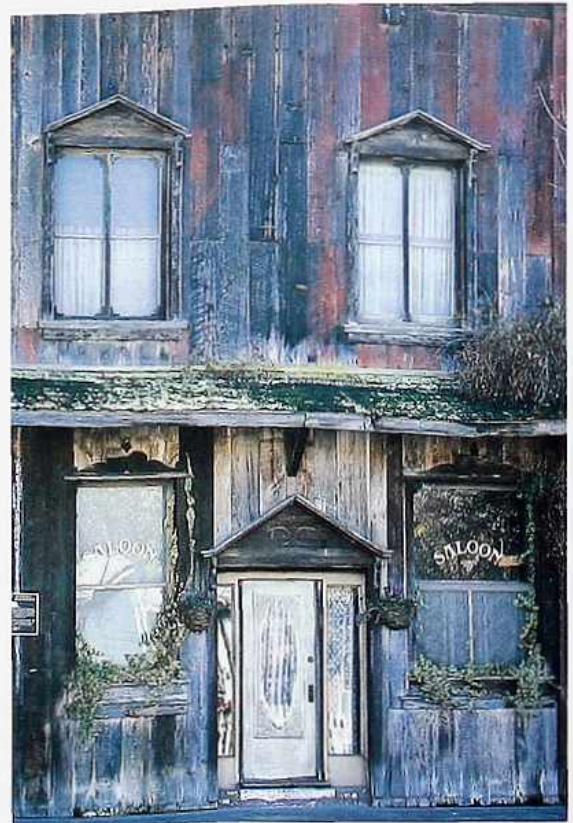
WA-31 Weathered flush vertical board siding with pediment-capped windows and door, American western saloon facade
