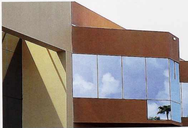
WI-165 Mirror-glass strip windows, modern commercial building
