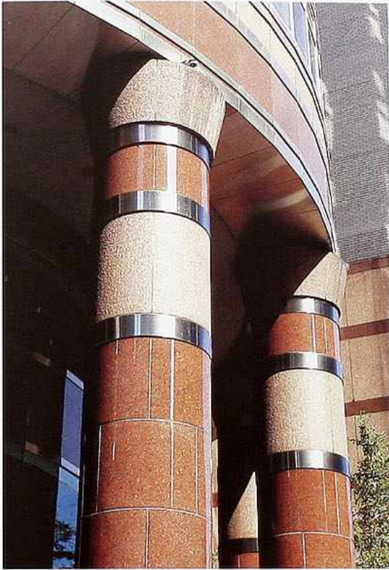
CP-126 Steel or concrete piers with polished stone and metal cladding, modern commercial building
