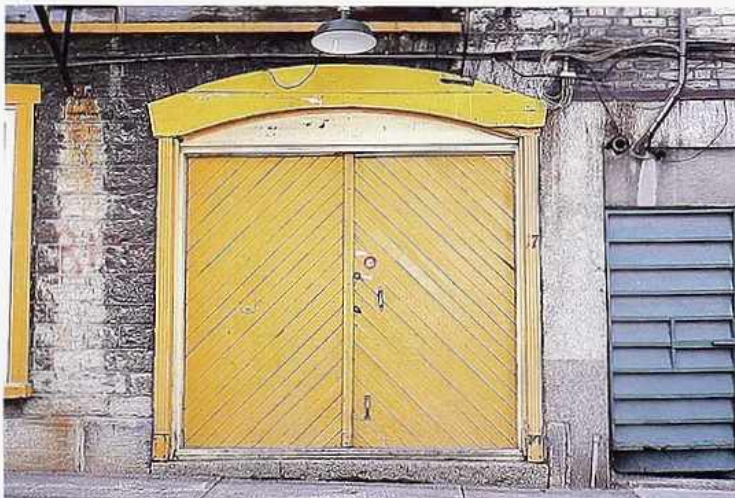
DW-32 Wood double garage doors with diagonal planking, in segmental arch
