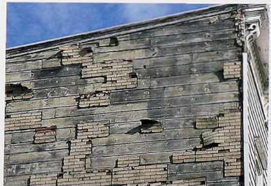
FA-56 Weathered bituminous shingles in faux brick pattern, exposed wood cladding
