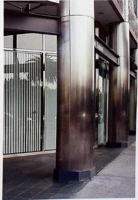
CP-129 Steel column with stainless-steel cladding supporting entry canopy, modern commercial building
