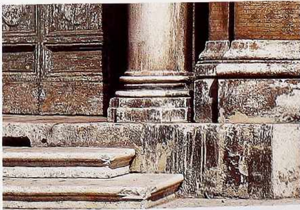
CP-39 Weathered marble column with Attic base on stepped octagonal plinth; right: brick pilaster on square marble base
