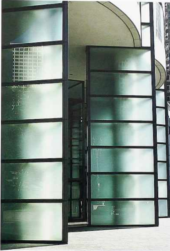
DW-97 Portico of metal-framed glass panels, modern commercial building
