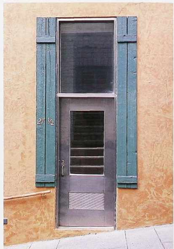
DW-61 Stainless steel door with single light and transom light; frame flanked by shutters, modern doorway in older urban building
