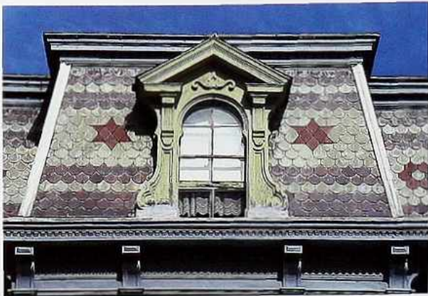
CR-62 Scalloped slate roofing in banded pattern with inset stars
