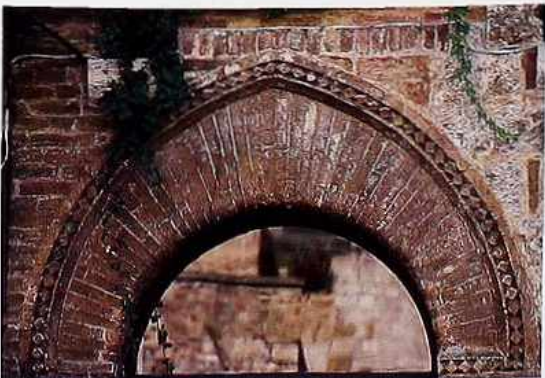
CP-154 Florentine arch (extrados and intrados not concentric), gauged brick. Extrados emphasized with a molding
