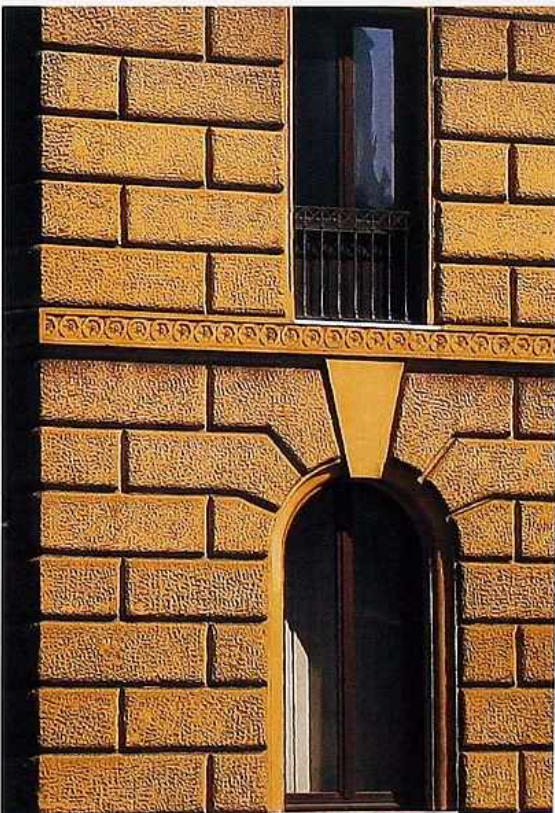
WA-112 Rusticated running bond with hand-tooled finish; sand-finish keystone; crossettes; carved ornamented belt course
