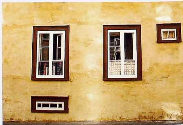
WA-242 Weathered undulating smooth stucco on painted wall with a variety of windows, urban house
