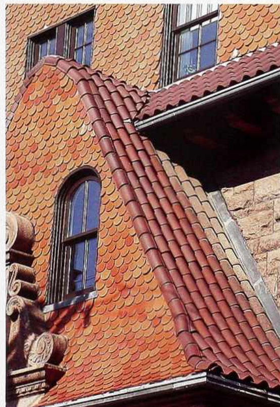
CR-57 Mission-tile roof with idiosyncratic gable and facade clad in scalloped tile shingles, 20th-c. American house
