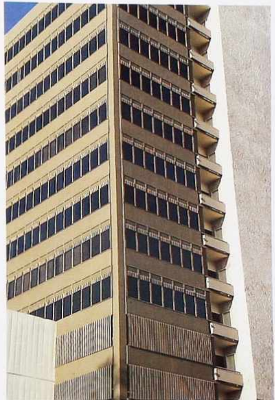
WA-303 Concrete building with metal trim
