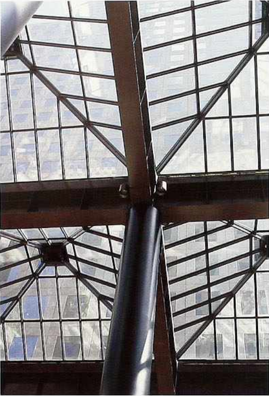
CP-112 Steel frame and tubular column; wide-flange beams supporting framed glass ceiling of modern commercial building
