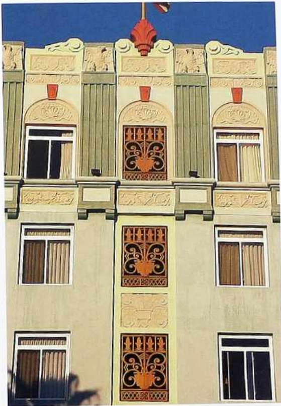
FA-124 Polychrome facade with low relief ornament in stucco and cast concrete, Art Deco hotel
