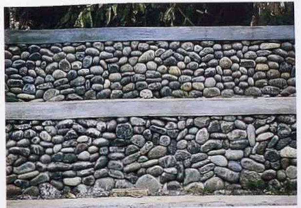
WA-79 Rubble walls of cobbles with wide squared stone step capping lower wall and coping on upper wall
