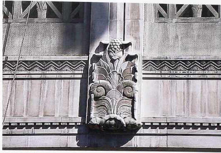
OM-13 Foliated ornament over doorway flanked by zig-zag (top) and dentilated (bottom) bands
