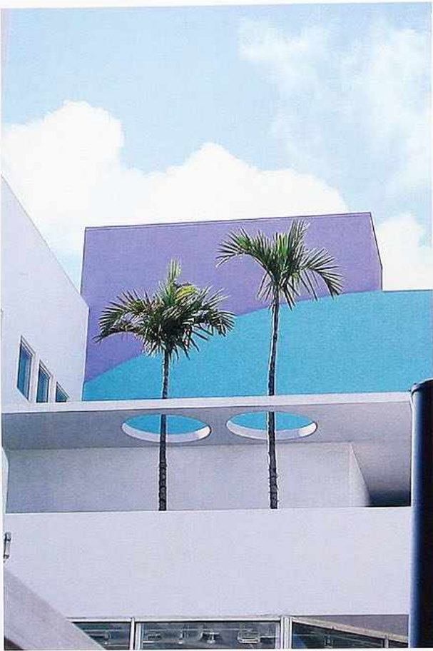
R-140 Flat, punctured roof with projecting eave and palm trees growing through concrete canopy
