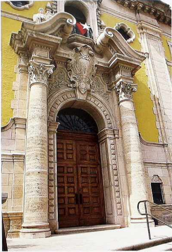
DW-72 Ornate arched entry with Corinthian capitals on engaged columns, fanlight, archivolt, cartouche keystone, and scrolled pediment
