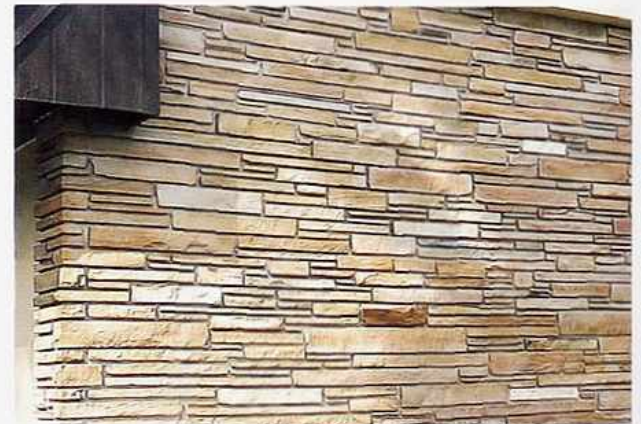
WA-65 Split- and rock-faced sandstone; shelf course, random ashlar with raked mortar
