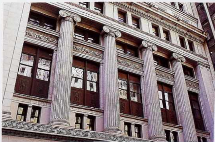
CP-104 Ionic engaged columns with entablature and festooned spandrels
