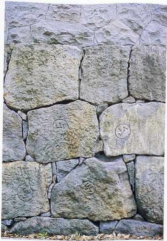
WA-73 Coursed rubble with gallets and rock-face cap
