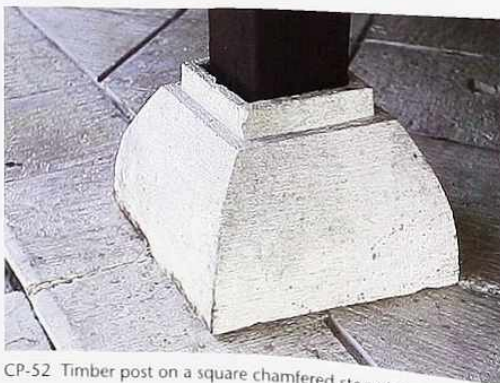
CP-52 Timber post on a square chamfered stone base
