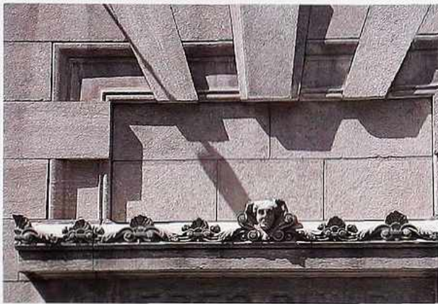
OM-59 Antefixes on cornice over a portal, the center one a mascarón
