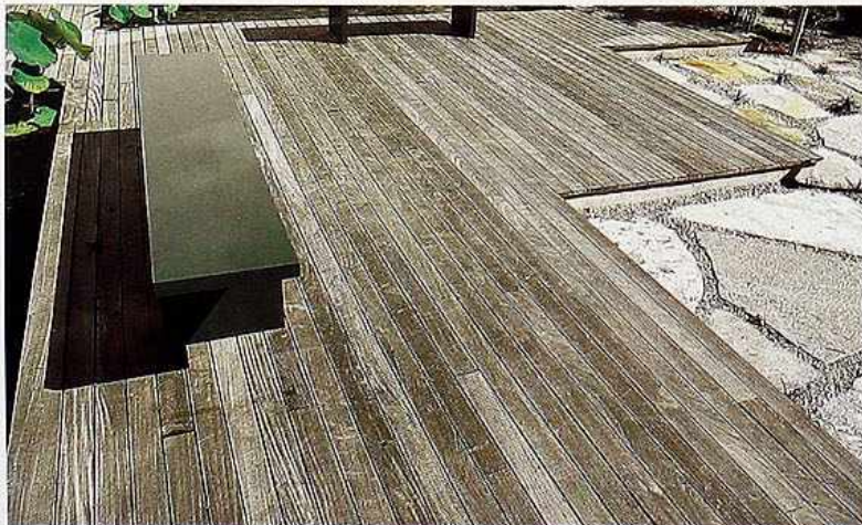
FP-12 Ipe-wood deck in flagstone walk; painted mahogany benches
