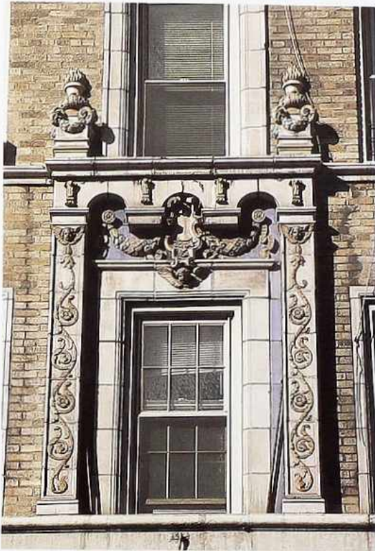
WI-136 Polychrome ornamented architectural terracotta frame around stone casings, apartment building
