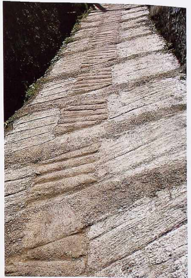
FP-79 Concrete textured to resemble rough wood planks, possibly cast-in-place, with texture produced by forming materials
