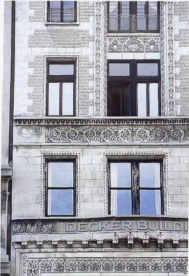
FA-112 Molded cornices and window surrounds with running ornament on multistory masonry facade
