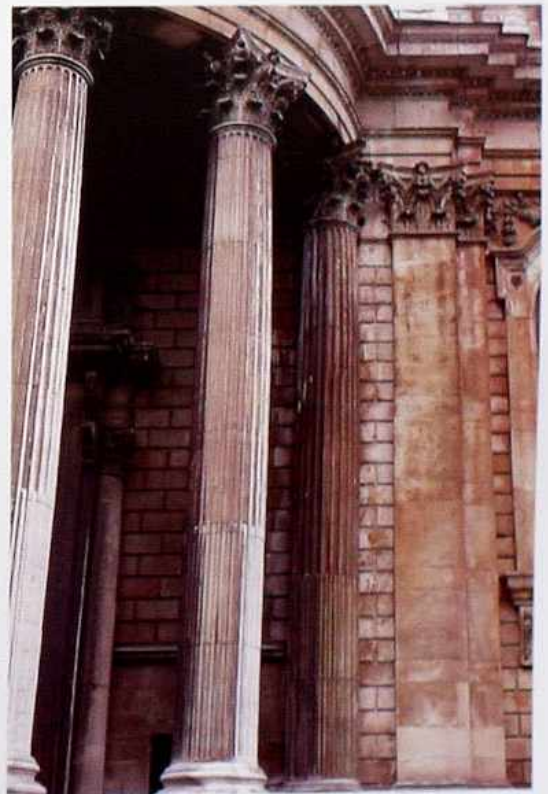
CP-72 Corinthian columns with partially fluted shafts next to flat pilasters
