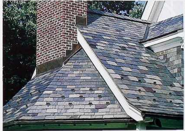
CR-61 Variegated Vermont slate roofing with snow guards
