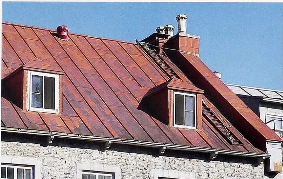
CR-39 Standing seams with hipped roof dormers
