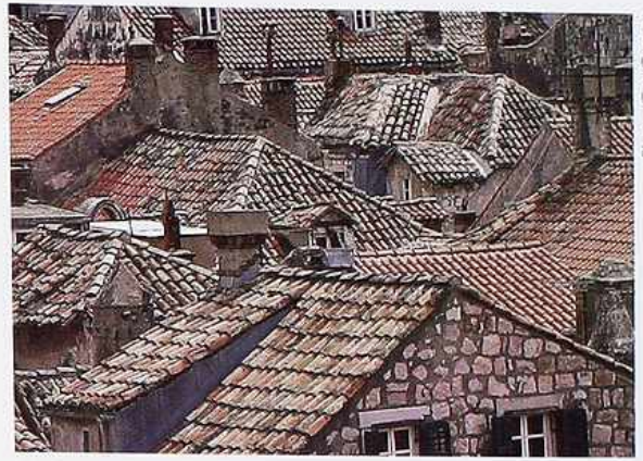
CR-50 Tile rooftops, Adriatic coastal village
