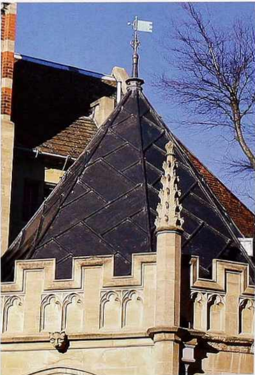
CR-132 Pyramidal metal roof
