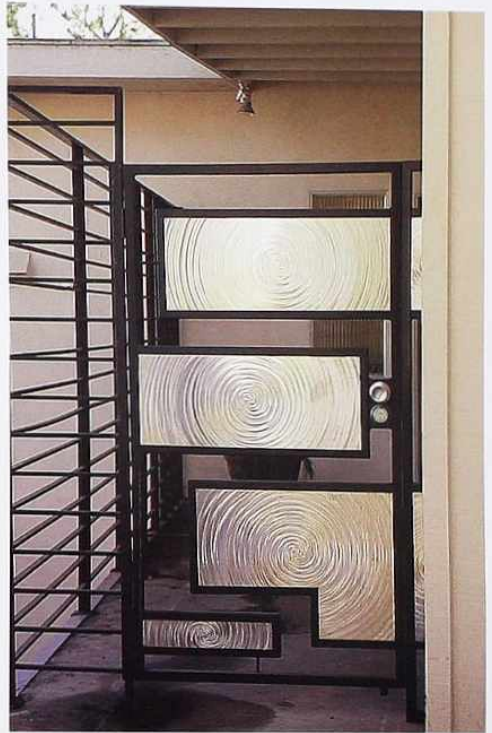
DW-119 Entry gate of framed metal panels with brushed directional pattern in open rectangular frame, modern house
