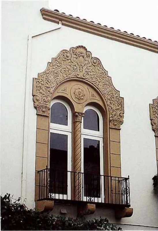
WI-150 Relief ornamental panel and pilasters around variation of Venetian-style window with balcony; 20th-c. apartment house
