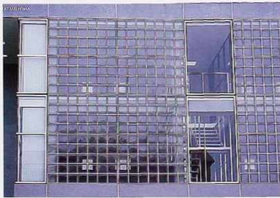
WI-21 Glass-block panels spanning two stories and flanked by fixed windows, modern commercial building
