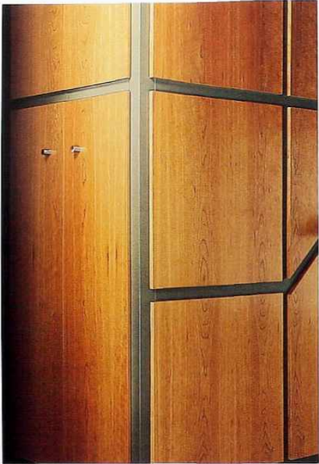
WA-1 Interior applied cherry-veneered panels with square finished edges on painted wood frame
