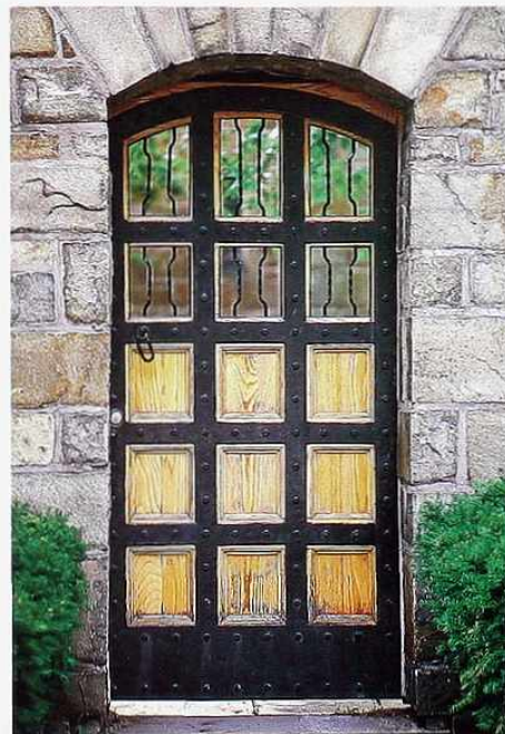
DW-4 Fifteen wood and open-grilled panels, studs on painted stiles and rails; segmental-arch doorway
