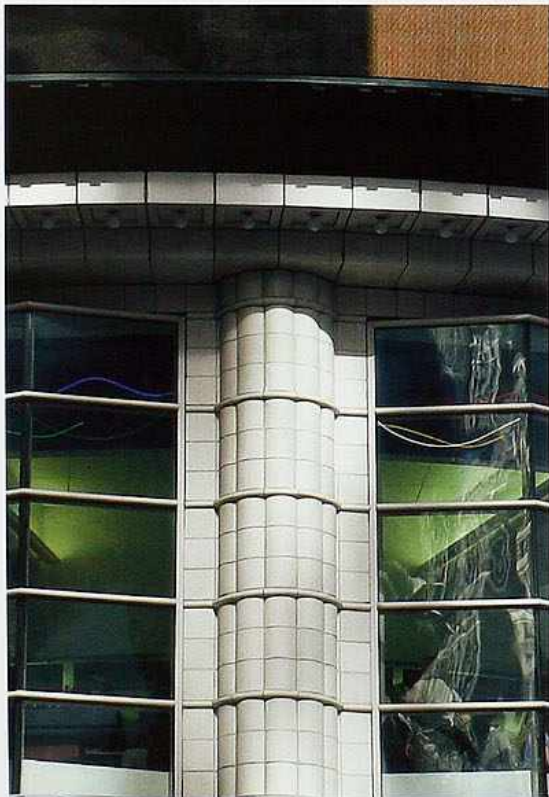
CP-98 Bundled pier on modern commercial building
