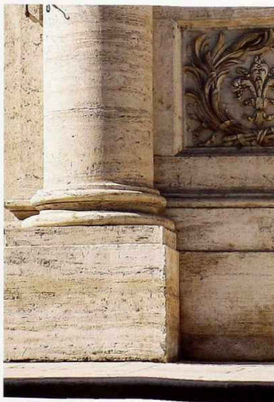
CP-44 Travertine column on Attic base on square stepped plinth
