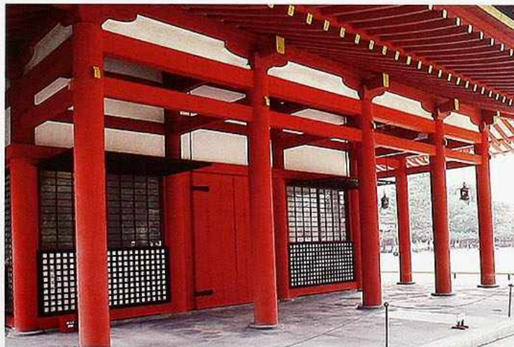
CP-140 Post-and-beam construction, Japanese temple
