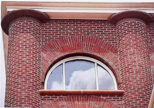
CP-102 Brick engaged columns flanking gauged-brick semi-circular arch windows
