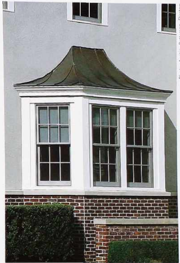
WI-77 Cant-bay window: six-over-six, double-hung, with wood casings, brick base, and flared standing-seam roof, traditional house
