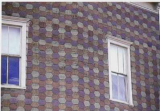
FA-57 Bituminous shingles in multicolored hexagonal pattern
