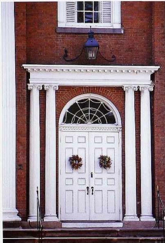
DW-74 Neoclassical entry with pairs of Ionic engaged columns supporting dentil entablature, eight-paneled double doors, bat-wing fanlight
