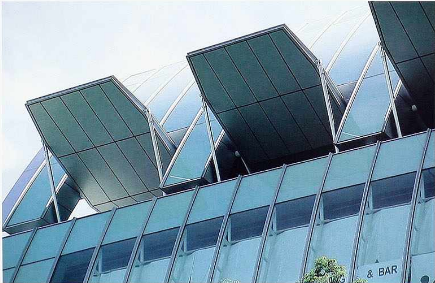
WI-204 Skylight shutters, modern commercial building
