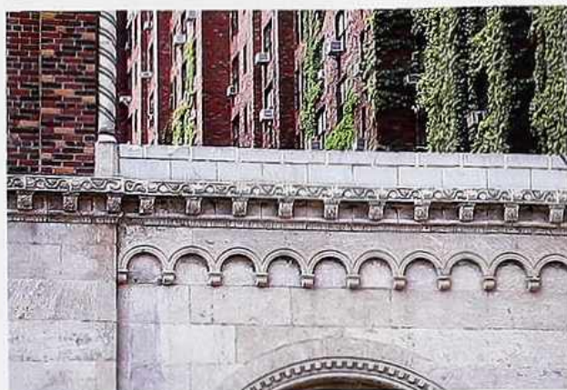
OM-88 Cornice. Top to bottom: serpentine band; modillion band; Gothic cornice. Dentilated archivol at bottom
