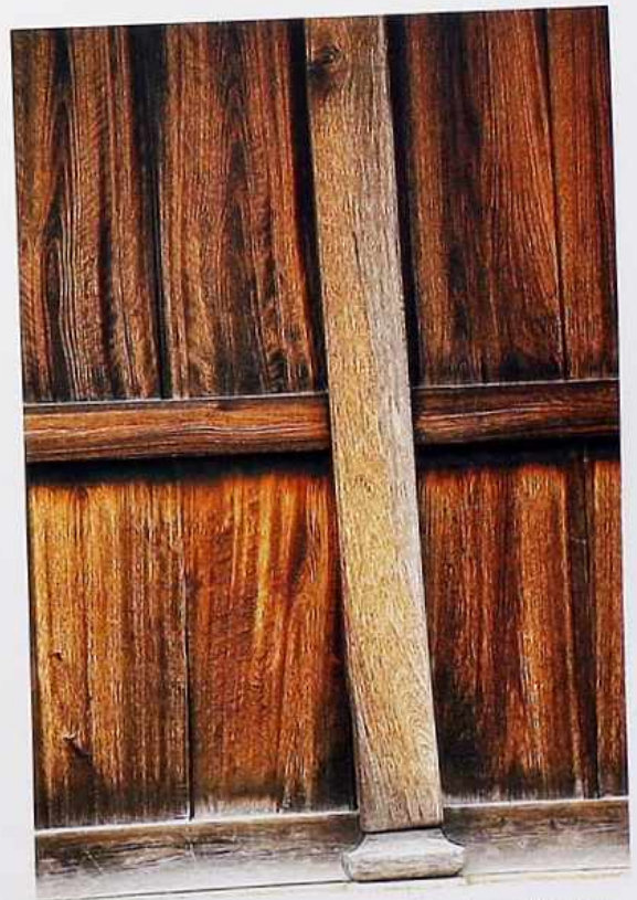
WA-43 Plain-sawn vertical planks with horizontal batten on shaped stone foundation; timber post with wood base
