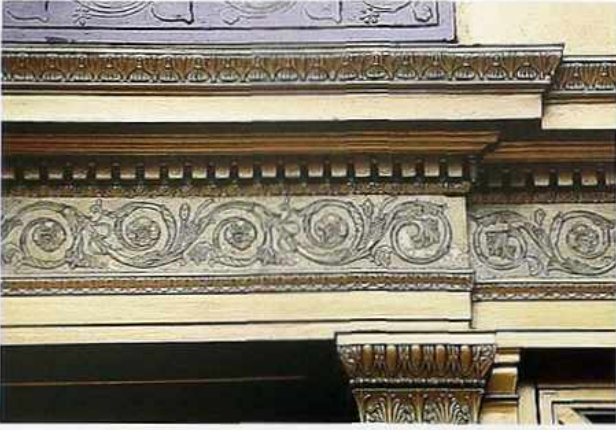
OM-67 Entablature. Top to bottom: leaf-and-dart, plain corona, cyma, dentil band, egg-and-dart molding, foliated frieze, modified tongue-and-dart cymatium. Capital: egg-and-dart echinus, bead-and-reel, anthemion cavetto
