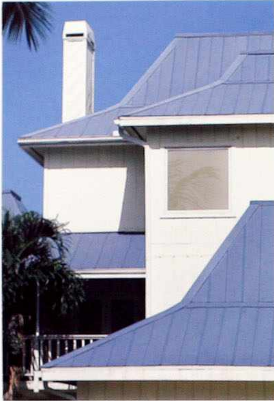
CR-30 Anodized aluminum or coated sheet steel with standing seams, variation of hipped roof, modern house
