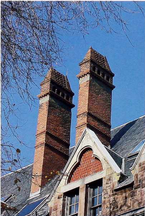
CR-145 Brick chimneys with hipped chimney hoods
