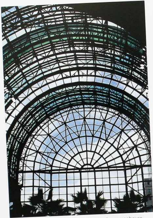
CP-176 Barrel-vaulted metal and glass modern greenhouse structure
