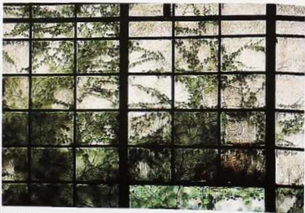
WI-13 Tinted and weathered glass, factory windows
