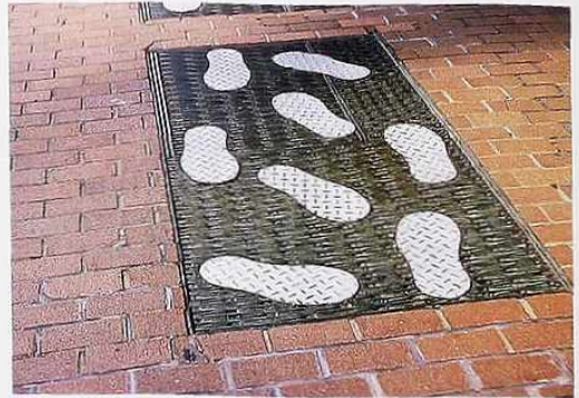
FP-116 Expanded-metal sidewalk grate with applied steel foot-prints
