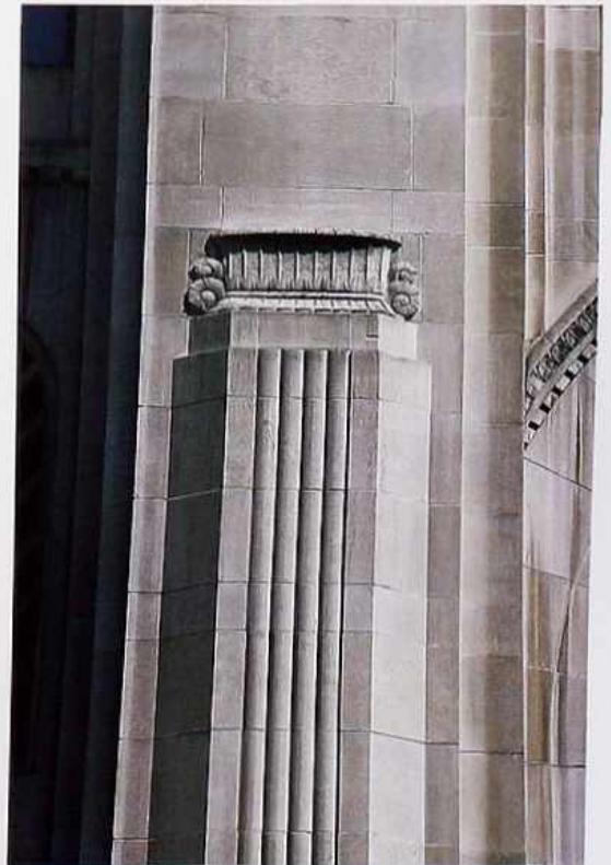
CP-87 Pilaster with trapezoidal profile, cabled, with a diminished capital resembling an Egyptian bell capital
