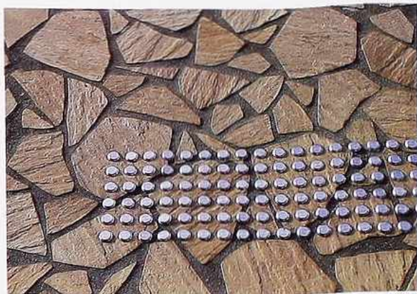
FP-108 Metal safety-paving brads on flagstone set in concrete, urban public space
