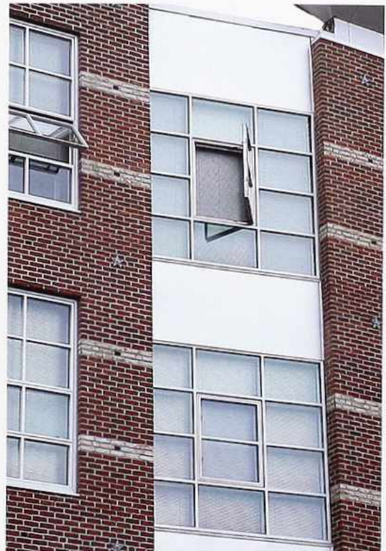
WI-39 Casement windows (center) and awning window (left) set in fixed lights; extruded aluminum mullions, modern apartment house
