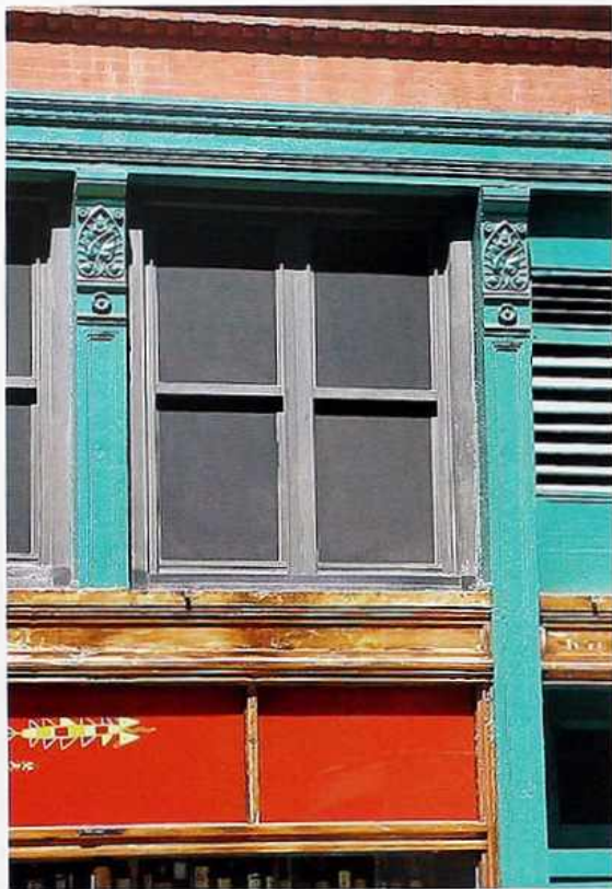
FA-75 Trabeated cast-iron facade painted in nontraditional colors
