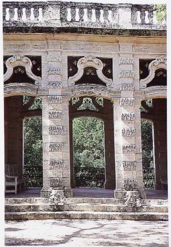
CP-135 Banded vermiculated coquina pilasters on square posts, garden arcade
