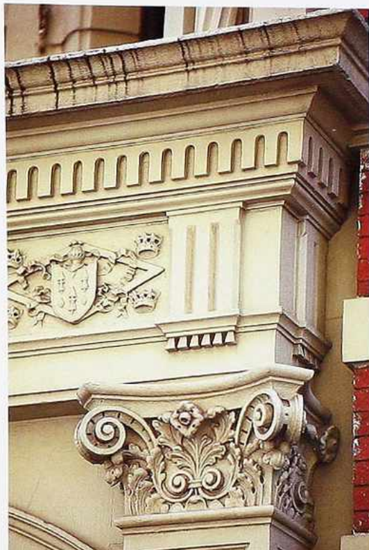
OM-102 Entablature with Doric features: triglyphs alternating with heraldic ornament in the frieze, quasi-dentil band, and soffit without mutules. Stylized Corinthian capital
