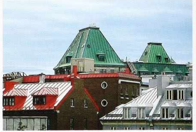
CR-116 Parapeted gable with hipped-roof dormers (left), hipped roof with hip dormers (right), and flared mansard with hip dormers (top), all sheet metal
