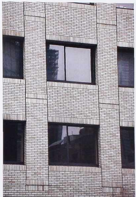
WA-180 Brick panels in running bond articulated by joints and soldier courses; soldier courses top and bottom of windows, modern commercial building
