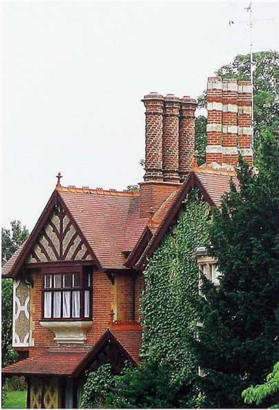
CR-143 Brick-pilaster chimneys: spiral (left); banded (right)
