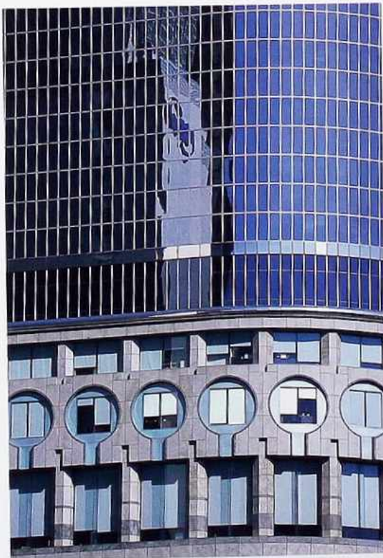
FA-126 Curving glass curtain wall above stone-veneer facade with expressed piers and keyhole window surrounds, modern commercial building
