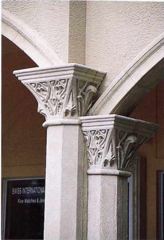
CP-14 Modern derivatives of Byzantine-style square capitals serving as impostes on octagonal shafts
