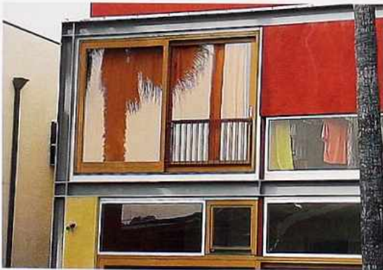
WI-40 Fully glazed wood sliding door, surrounded by fixed lights or awning windows, modern house
