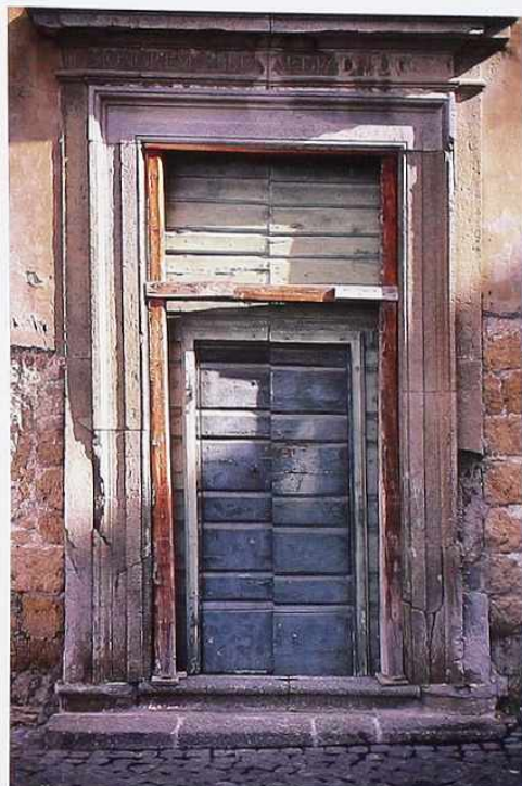
DW-105 Weathered entry with wood molding, transom panel, and painted paneled door
