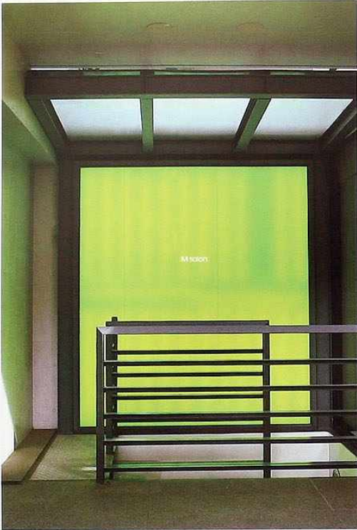
DW-101 Entry with large colored glass window and overhead lighted glass panels, modern commercial building
