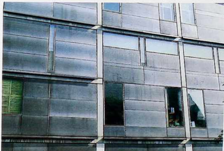
FA-25 Reinforced concrete frame with black acid-etched stainless steel panels and windows, modern institutional building
