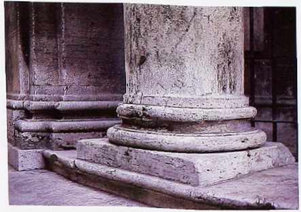
CP-36 Attic base of weathered travertine column on square plinth
