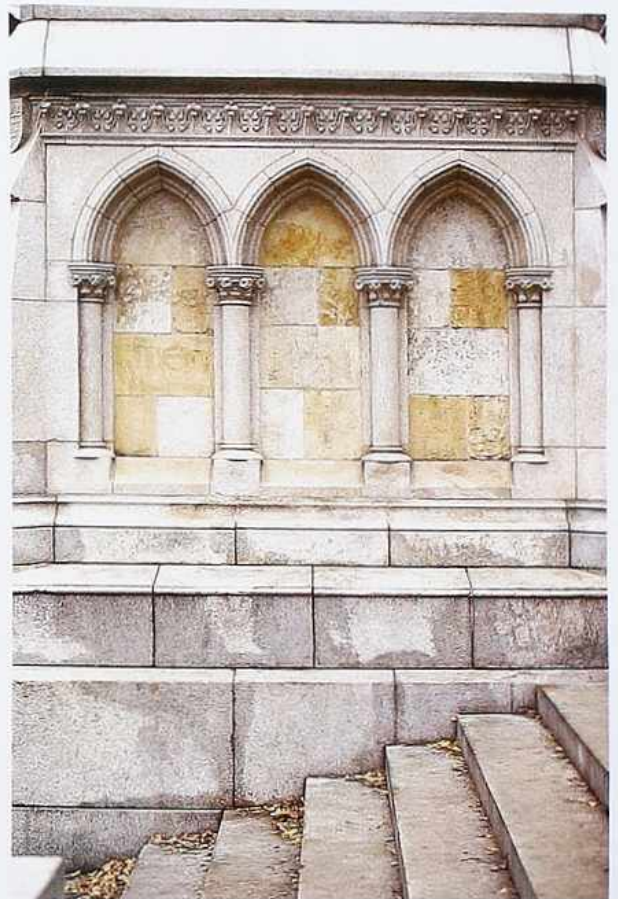
WA-121 Staircase wall in coursed ashlar with Gothic blind arches and engaged columns
