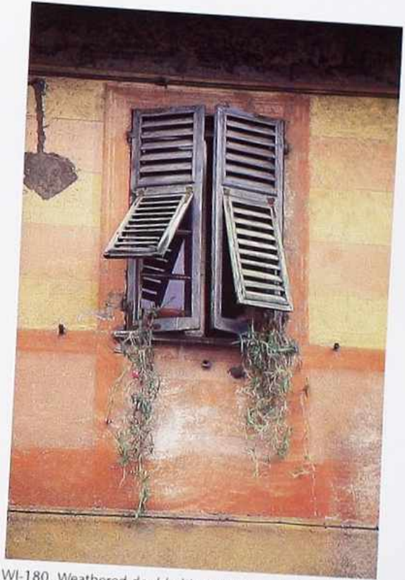
WI-180 Weathered double-hinged louvered shutters
