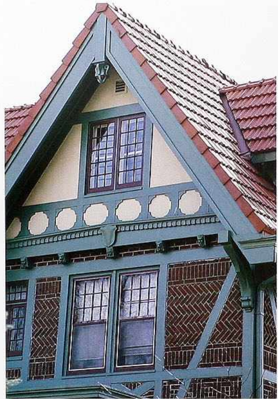
CR-77 Half-timber-style gable wall with tile roof, 20th-c. American house
