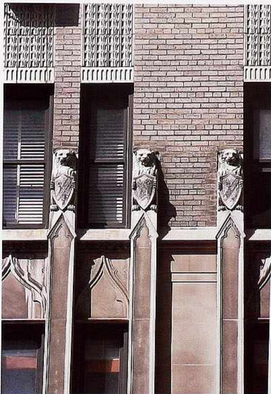
FA-117 Neo-Gothic ornamental features with ornamental spandrels in brick facade
