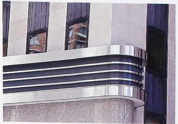
OM-74 Metal fascia bands suggesting molding, modern building facade
