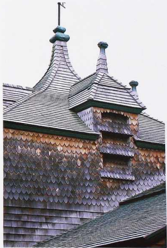
FA-44 Weathered sawn shingles in fish-scale pattern on ogee roof
