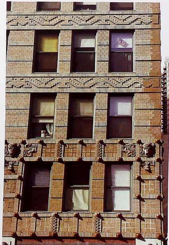
FA-118 Brick facade with stone or cast rams-head-and-snake ornaments and running geometric ornament in spandrel bands
