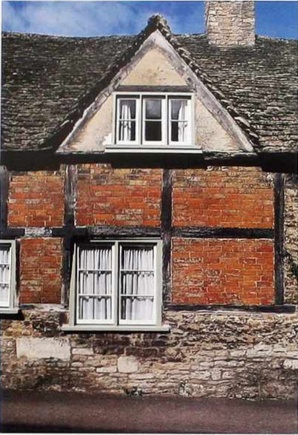
WA-282 Half-timber with brick infill; fieldstone first story, 16th- or 17th-c. English house
