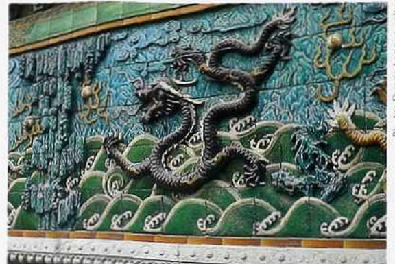
FA-62 Glazed polychrome relief tiles with dragon design on exterior wall
