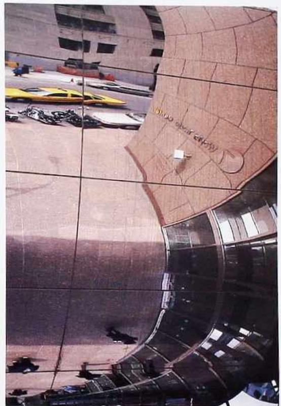
FA-8 Flush curved mirror-finished stainless steel cladding, modern commercial building
