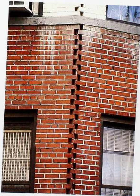
WA-195 Corner detail of common bond, sixth-course header, with dog's-tooth corner
