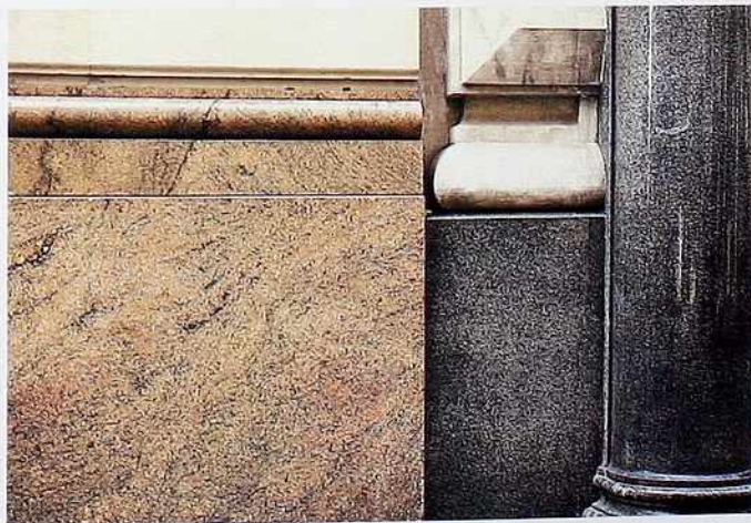
WA-88 Polished granite and marble. Left to right: granite-vener base with bead molding; granite plinth with marble ovolo molding on base; polished granite engaged column
