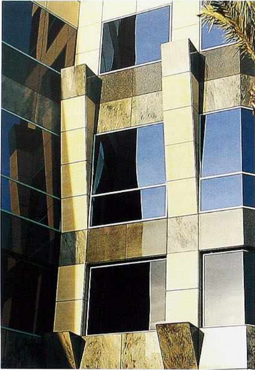
WA-145 Polished veneer in polychrome bands with pilaster strips, modern commercial building
