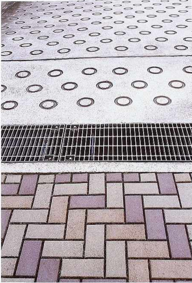
FP-78 Top to bottom: circle diaper pattern stamped in concrete; metal grate drain cover; pre-cast polychrome concrete pavers in herringbone pattern
