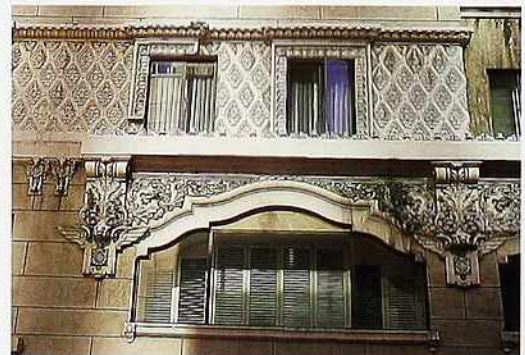
WI-145 Assortment of moldings and ornament around square casement windows over profiled fixed window
