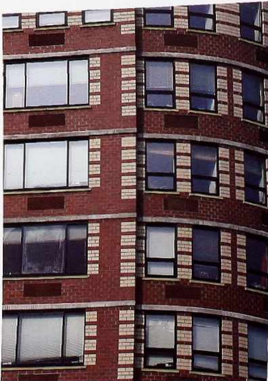
WI-156 Repetitive fenestration of picture windows with side lights and double-hung windows (right) with brick quoins, modern commercial building
