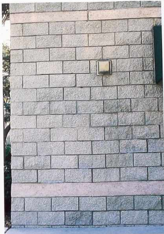
WA-226 Split-face concrete block in running bond with pink banding, modern commercial building
