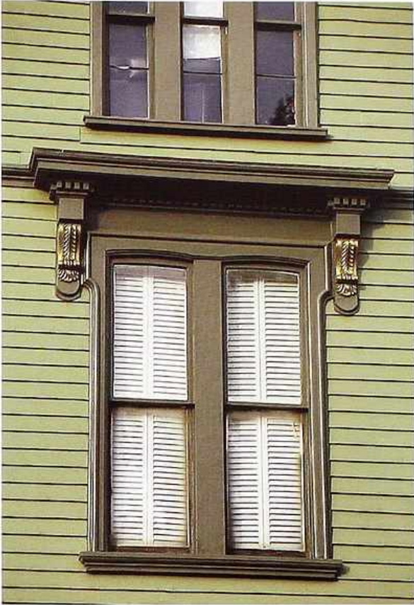
WI-107 Flat wood casing with crossettes around one-over-one double-hung windows; hood supported by brackets, American clapboard house
