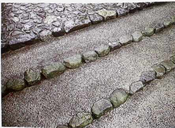
FP-76 Pea-sized gravel aggregate inset with rows of rocks and bordered by small split, polished fieldstone set in concrete
