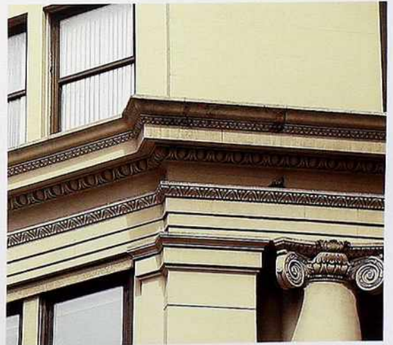
OM-85 Top to bottom: heart-and-dart ogee, egg-and-dart ovolo moldings, plain frieze, leaf-and-dart moldings
