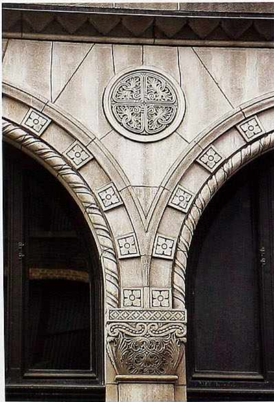
CP-148 Arcade of semicircular arches, rope molding in intrados, square panel rosettes, and quatrefoil medallion in spandrel
