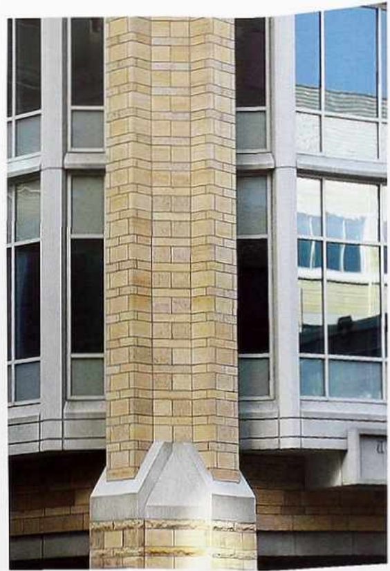
CP-81 Compound corner pier, modern commercial building
