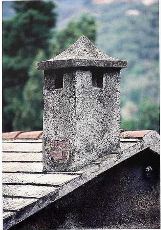
CR-148 Stucco-over-brick chimney with pyramidal hood
