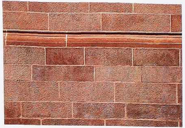
WA-67 Hammered-finish brownstone in coursed ashlar with flush mortar joints and water-table course
