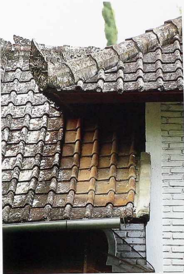
CR-40 Weathered terracotta pantile with antefix at end of ridge tiles on hip, Balinese house
