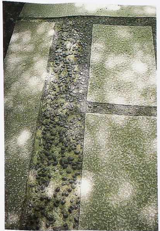
FP-69 Pre-cast paving blocks of light-colored exposed aggregate in a field of dark-colored exposed aggregate
