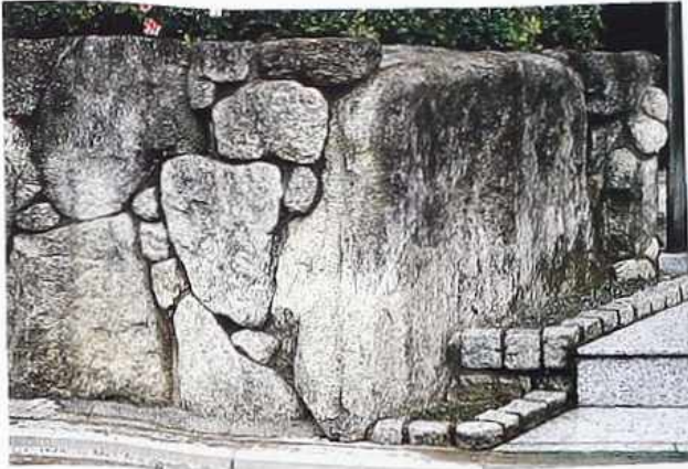
WA-76 Massive rubble with gallets, garden wall
