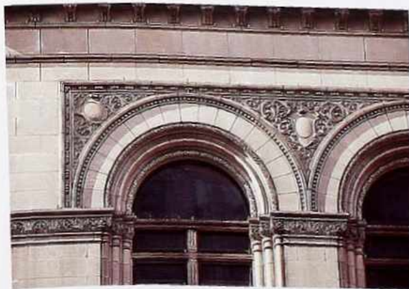
CP-144 Arcade of semicircular compound arches; spandrels with cartouches and foliated ornament
