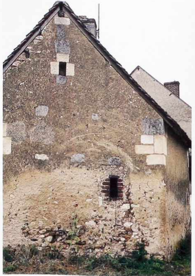
WA-249 Large-aggregate stucco with cobbles and quoins on weathered gable-end wall, farm building
