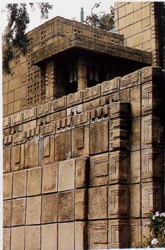
WA-229 Custom concrete blocks with screen wall (top), residential entryway
