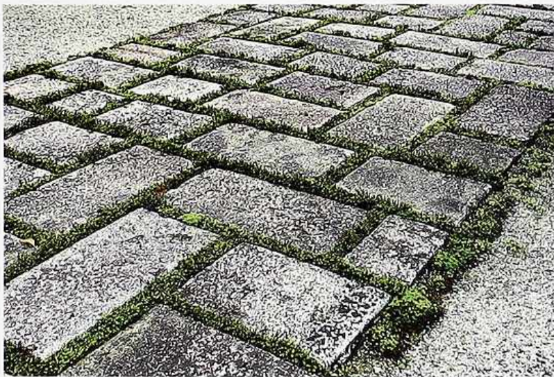
FP-29 Roughly squared paving stone in random-ashlar pattern with moss on sidewalk
