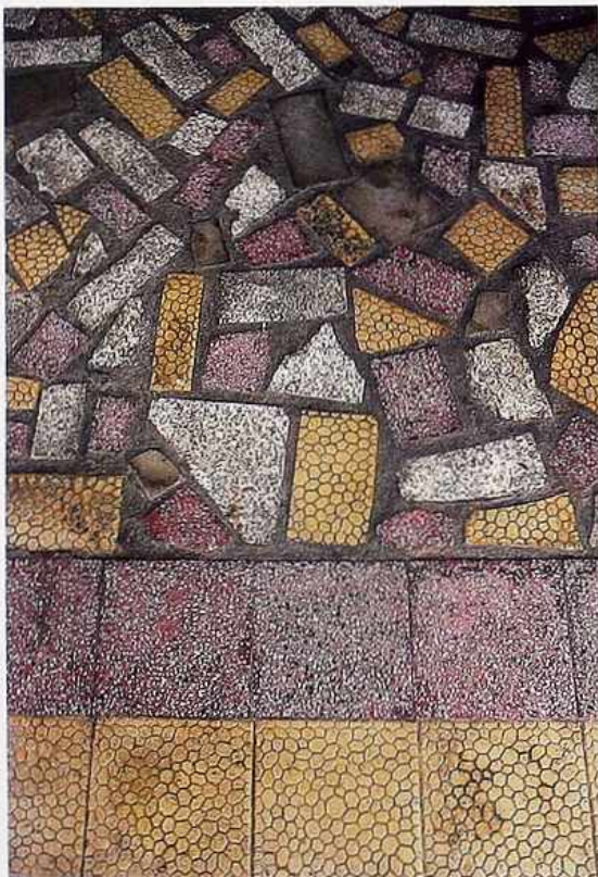
FP-83 Polychrome pre-cast concrete textured pavers: mosaic area (top) bordered by straight-joint border, urban public space
