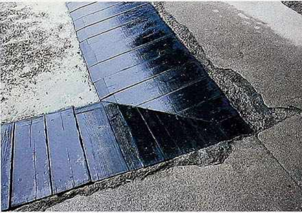
FP-10 Wood planks with concrete surround, courtyard walkway
