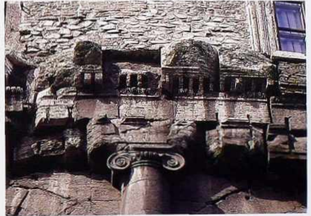
OM-95 Weathered Ionic entablature with remains of a dentil band and an egg-and-dart ovolo molding below it
