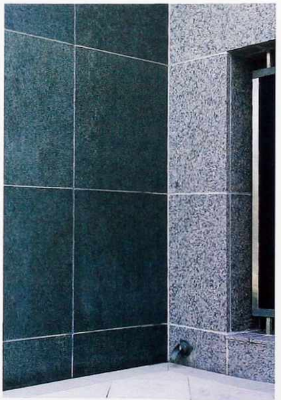
WA-134 Inside corner of honed-granite veneer in stack bond with grouted joints and window reveal, modern commercial building
