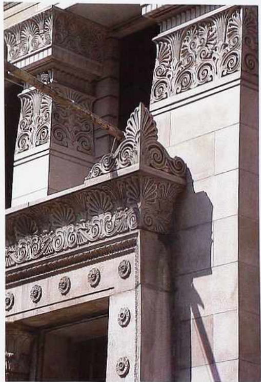
OM-54 Door surround with rosettes; cavetto cornice with anthemion motif and antefix at corner; pier capped by anthemion
