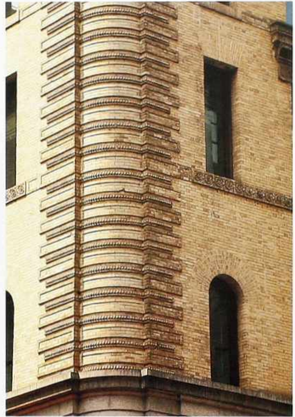
WA-190 Curved corner banded with courses of stretcher bricks and sculpted brick or architectural terracotta
