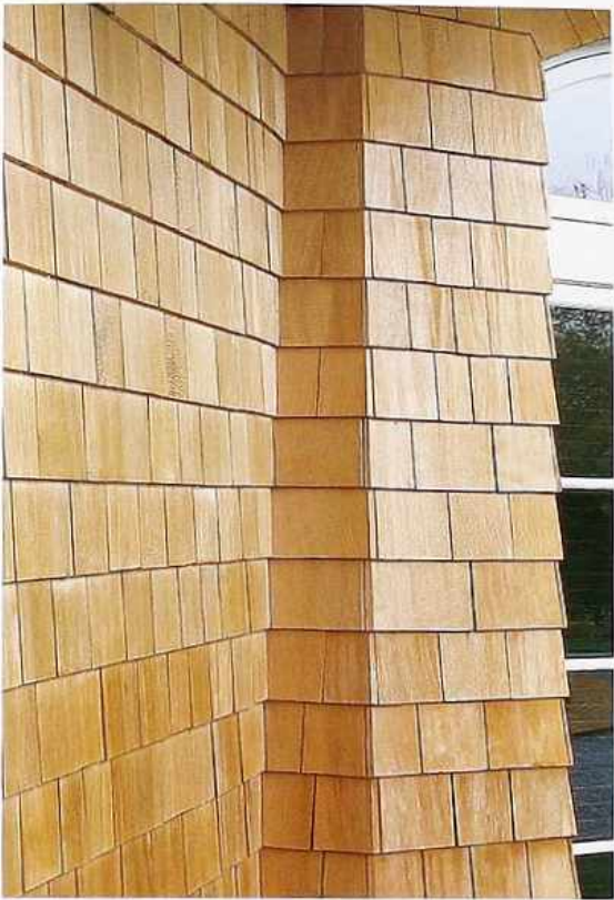
FA-43 New Alaskan yellow cedar shakes in common coursing, corner detail
