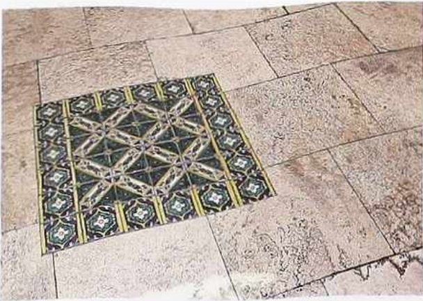
FP-91 Decorated glazed ceramic tiles surrounded by stone in running bond, commercial entry
