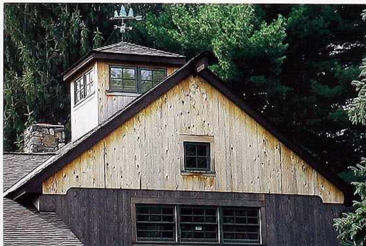
CR-88 Gable-end wall with new flush board siding above weathered siding; glazed monitor with pyramidal roof
