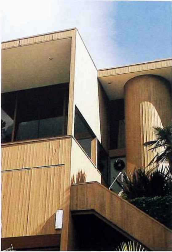
WA-47 Flush board siding on flat and curved surfaces, modern house
