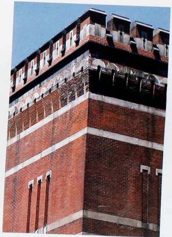
WA-196 Corner detail of Romanesque-style brick building with stone banding, parapet roof with crenellation
