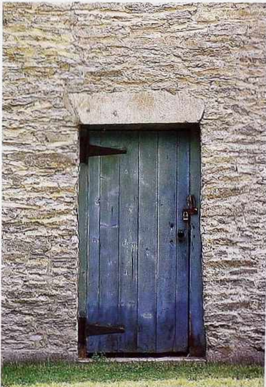
DW-43 Weathered painted wood batten door with iron strap hinges
