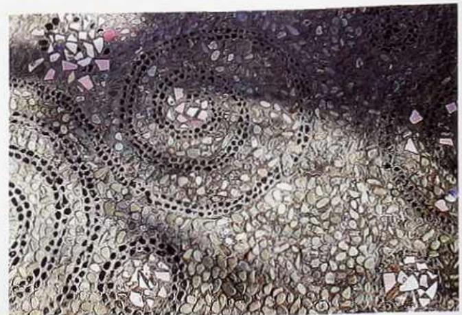
FP-77 Serpentine design of polychrome pebbles in exposed aggregate
