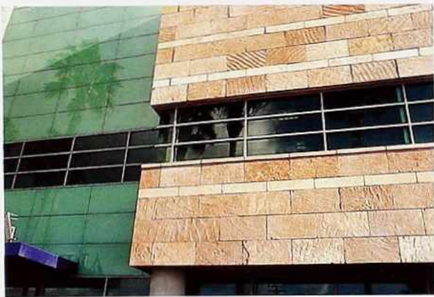
WA-299 Split-face sandstone veneer next to colored-glass or plexiglass-clad wing, modern commercial building
