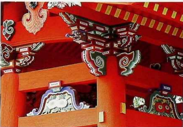
CP-120 Post-and-beam construction with polychrome ornamental brackets, Japanese temple
