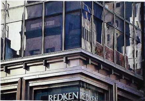
OM-75 Corner detail of metal fascia bands suggesting a classical entablature, the continuation of mullions suggesting a modillion band
