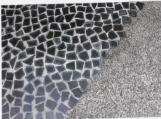
FP-74 Pea-sized gravel aggregate (right) next to randomly shaped and placed tile
