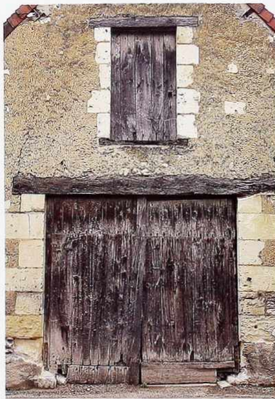
DW-26 Weathered plank doors under rough-hewn timber lintel; rustic stone and stucco qable wall of barn and hayloft
