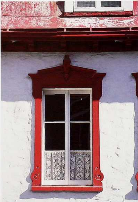
WI-113 Profiled flat casing around double-casement window
