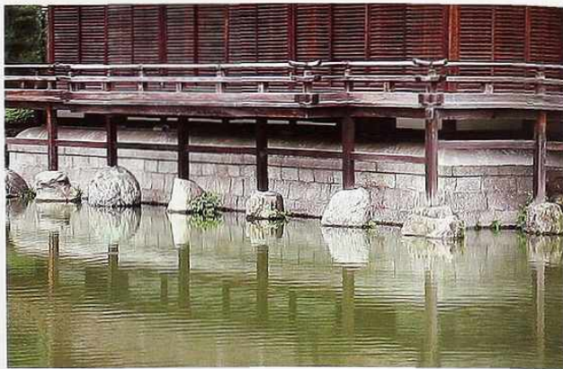
CP-53 Natural boulders supporting timber posts under deck of pavilion in Japanese garden pond
