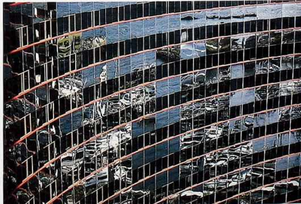
FA-31 Banded curtain wall, alternating mirror glass spandrels and windows
