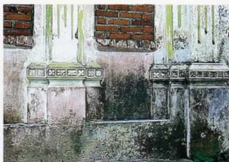
FA-85 Courtyard wall and steps: weathered pilasters with painted flutes and ornament, Indonesia
