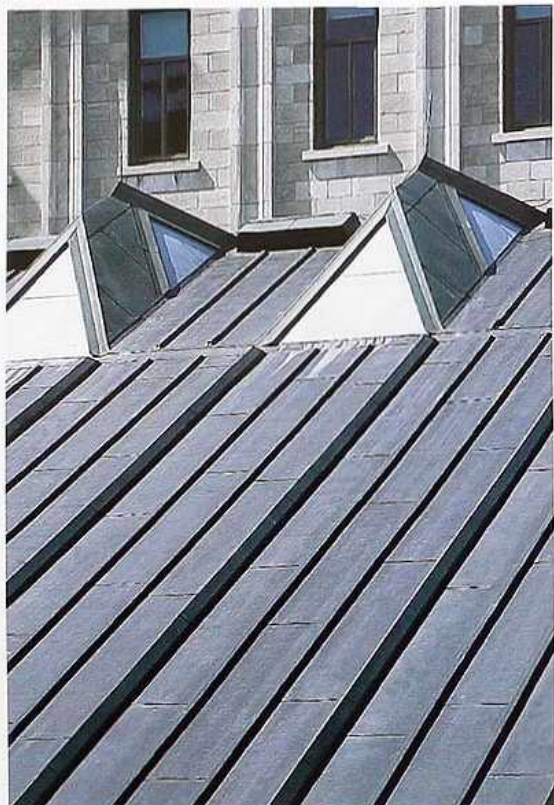
CR-21 Anodized aluminum or coated sheet steel with batten seams, modern commercial building
