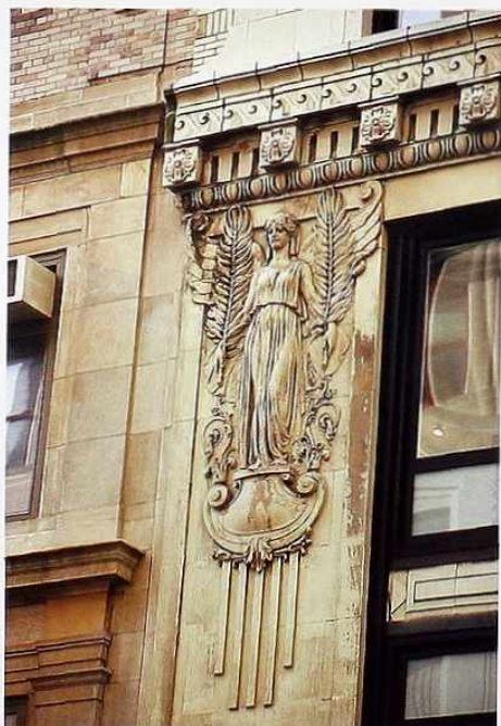
OM-42 Anta with relief winged mythological figure holding palm fronds below cornice with egg-and-dart ovolo molding and an alternating dentil and modillion band
