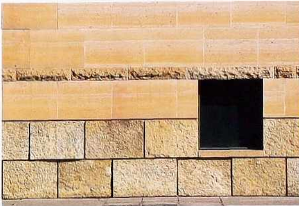
WA-68 Banded sandstone. Top: running bond, honed-finish with rock-face belt course; bottom: running bond, split-face, modern commercial building
