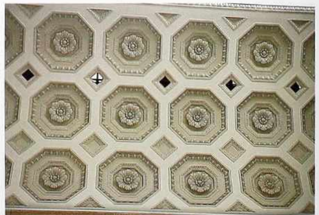
CR-15 Coffered ceiling with classically ornamented octagonal coffers
