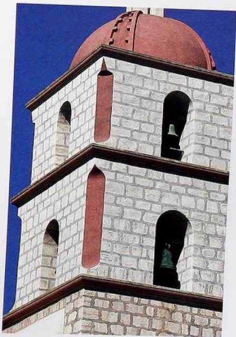
FA-91 Trompe l'oeil stucco simulating adjacent masonry on belfry, dome with chamfered corners, 19th-c. mission
