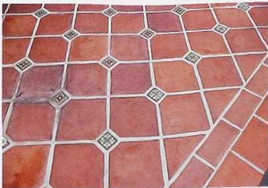
FP-99 Mexican paving tiles, straight-jointed, and inset with small decorated glazed tiles in diaper pattern, vertical-joint border (right)
