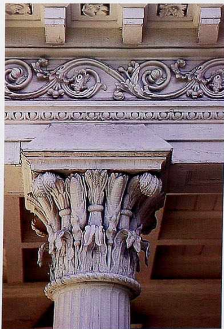
CP-24 American-order capital and entablature with egg-and-dart molding, arabesque frieze, and block modillions
