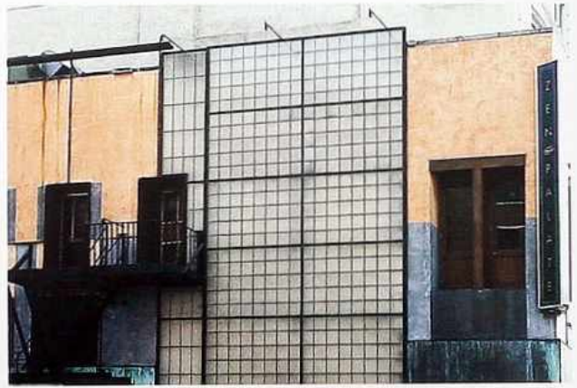
WA-298 Metal-framed glass panels with colored and patinated metal, modern commercial building
