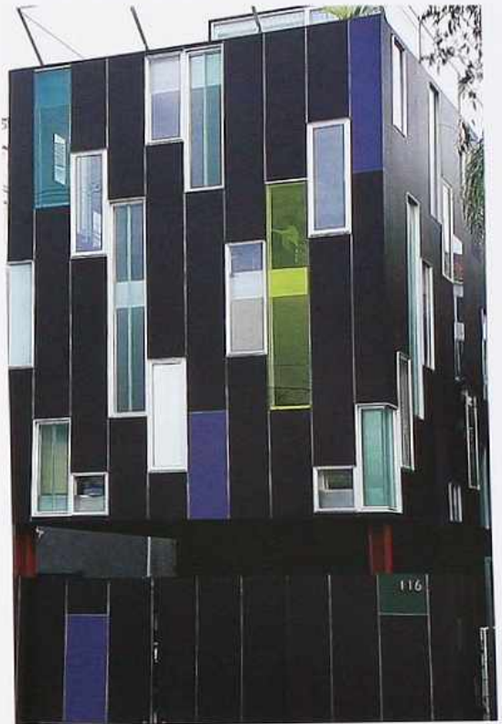
WI-16 Colored and clear fixed and casement windows (note floor plate behind the middle windows), modern house
