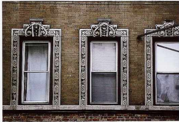
WI-130 Stone or cast concrete casings with relief ornament and ornated keystones, early 20th-c. apartment house
