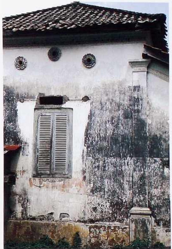
WA-261 Weathered stucco wall with pilaster
