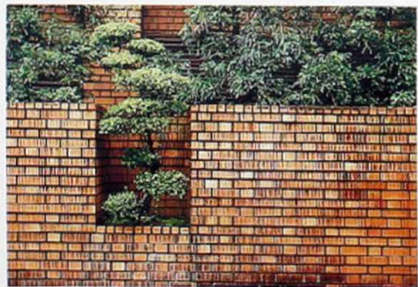
WA-157 Notched garden wall in Flemish bond with rowlock-course coping
