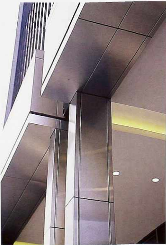
CP-124 Steel frame clad with possibly stainless steel panels, modern commercial building
