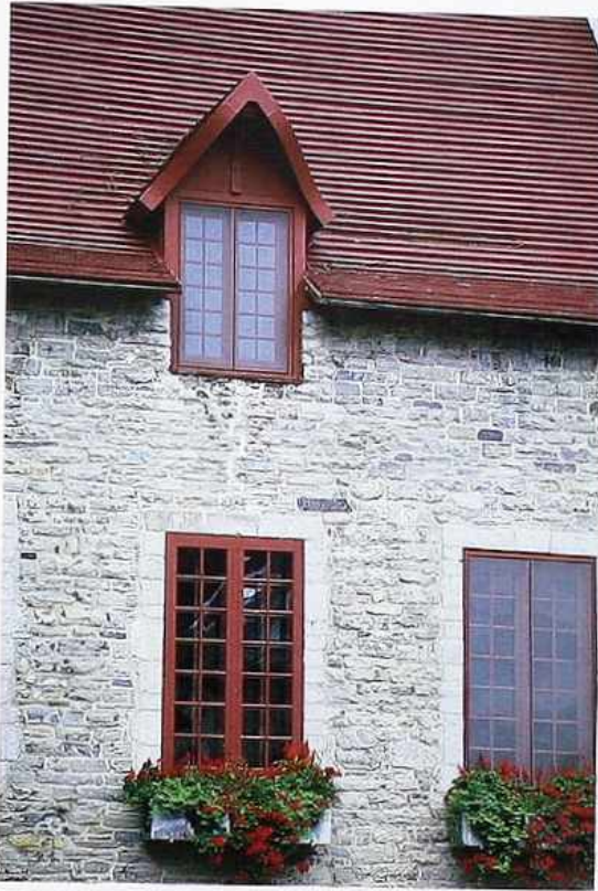
CR-89 Wall dormer on painted wood roof
