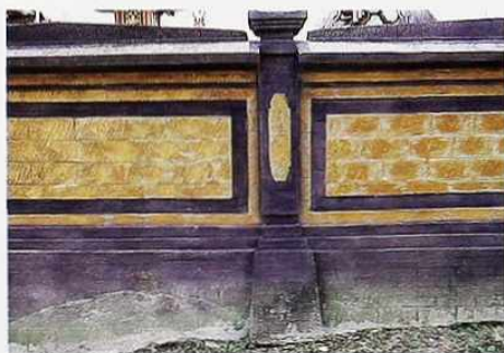
FA-84 Courtyard wall of painted stone and concrete block with scribed lines simulating masonry, Indonesia
