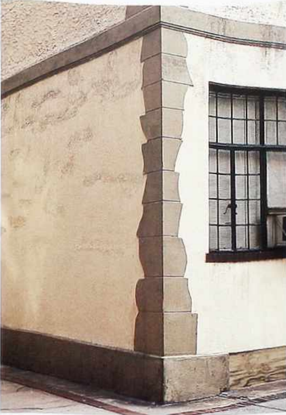
WA-234 Smooth stucco quoins and belt course on textured stucco building
