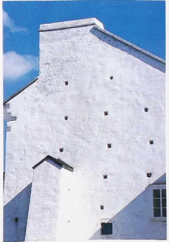
WA-235 Undulating stucco finish on gable-end wall, industrial building
