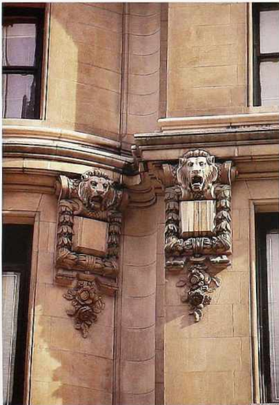
OM-11 Brackets: square panel surrounded by a garland with a lion's-head antic in front of a scroll.
