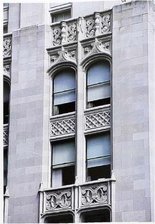
WI-141 Neo-Gothic ornament in spandrels and capping window panels, early 20th-c. commercial building
