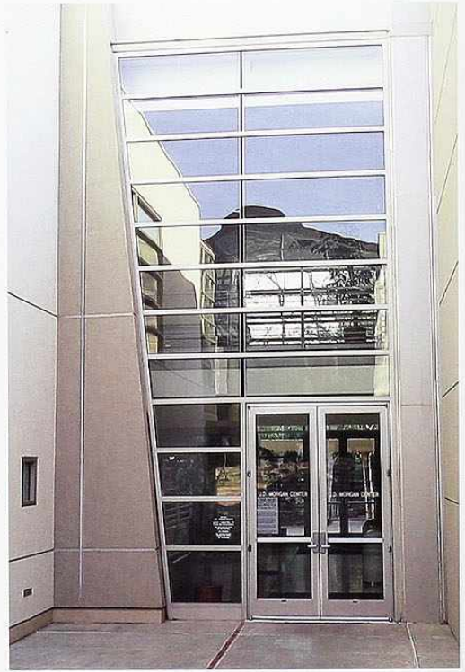
DW-102 Covered entryway: stainless steel double doors with full glass set in glass-paneled wall; masonry surround, modern commercial building
