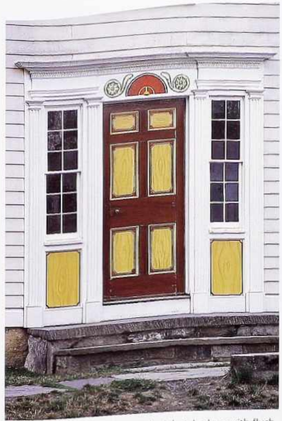
DW-38 Six-panel American Colonial-style door with flush molding, painted ornament on transom, and double-hung side lights
