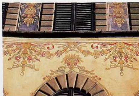
FA-86 Decorative painting of foliated ornament around rusticated arch and window on stucco Tuscan wall
