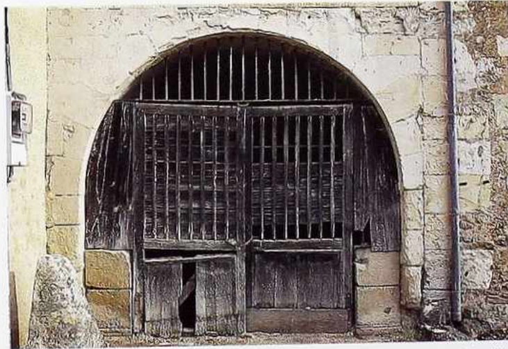
CP-160 Weathered stucco-covered stone semicircular arch with wood double doors, rustic courtyard
