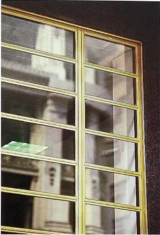
WI-5 Fixed window with brass muntins and mullion, modern commercial building
