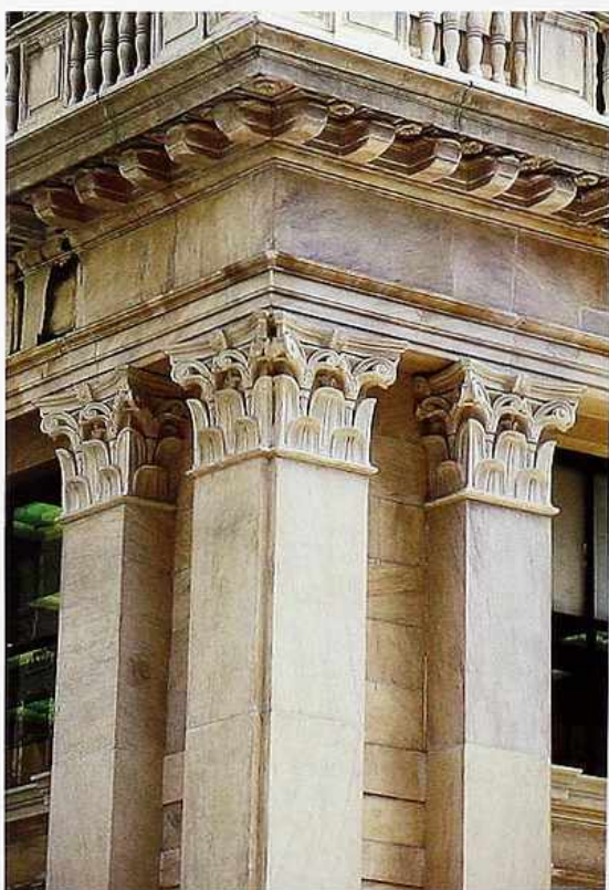
OM-103 Corinthian entablature. Top to bottom: block modillions alternating with rosettes in corona soffit; plain frieze
