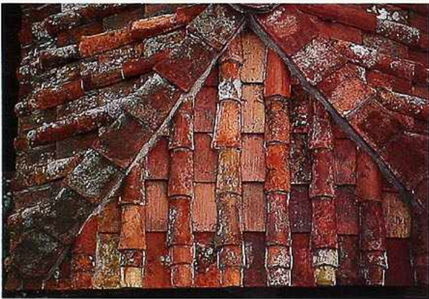
CR-46 Weathered terracotta tiles on pyramidal roof
