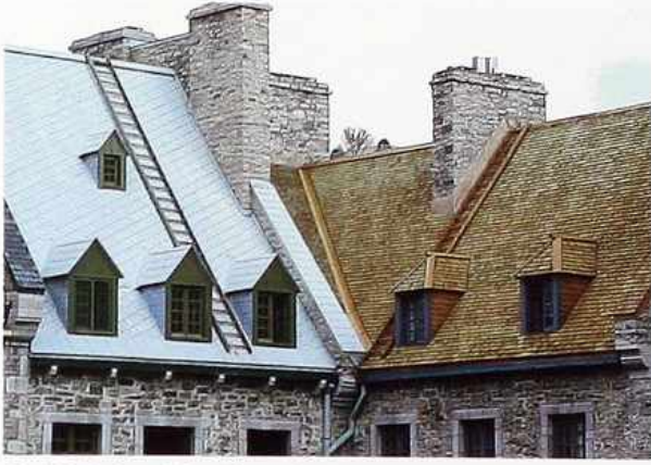
CR-120 Left: gable with roof dormers, metal with flat seam; right: gable with hipped-roof dormers, wood shingle; flashing in roof valley
