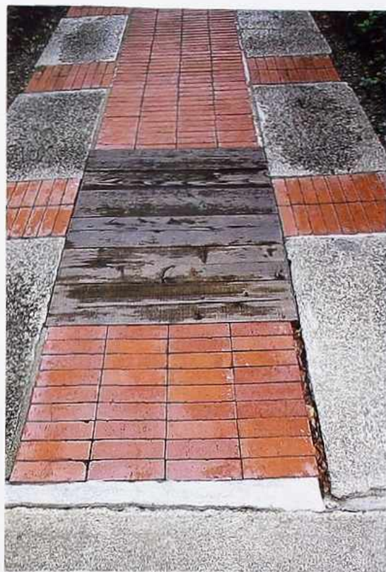
FP-62 Brick pavers in stack bond alternating with wood planks and large-aggregate concrete, urban public space
