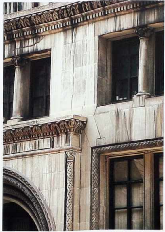
WA-115 Weathered limestone in coursed ashlar with dentil and modillion cornice; carved ornament on columns and window frames
