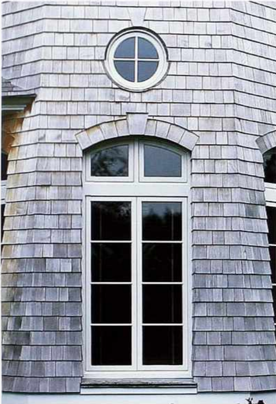
WI-94 Segmental-arch transom light with shingle "voussoirs" and "keystone" above French door, modern shingle house
