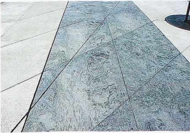
FP-23 Dark and light dimension-granite paving stone in diagonal design, urban public space
