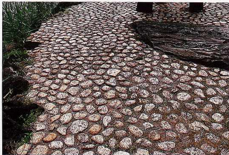
FP-39 Random round cobbles set in concrete, garden path
