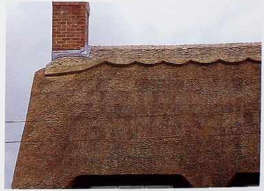
CR-73 Scalloped roof ridge on traditional English thatched house
