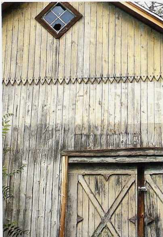
WA-30 Weathered painted flush vertical board cladding on barn gable end with diamond-shaped window and vertical scallop-edged siding
