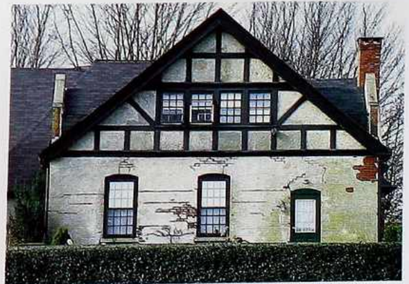
CR-125 Half-timbered gable
