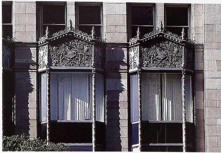
WI-83 Two-story cant-bay windows: fixed lights below ornamental cast or pressed metalwork, apartment house
