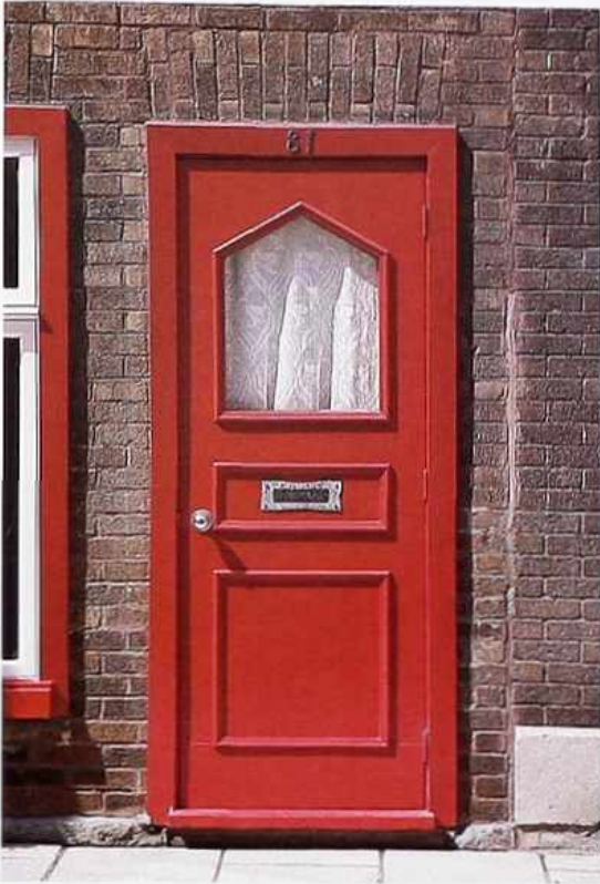
DW-41 Painted paneled door with pentagonal light in top panel, brass letter slot, in brick entry with jack arch
