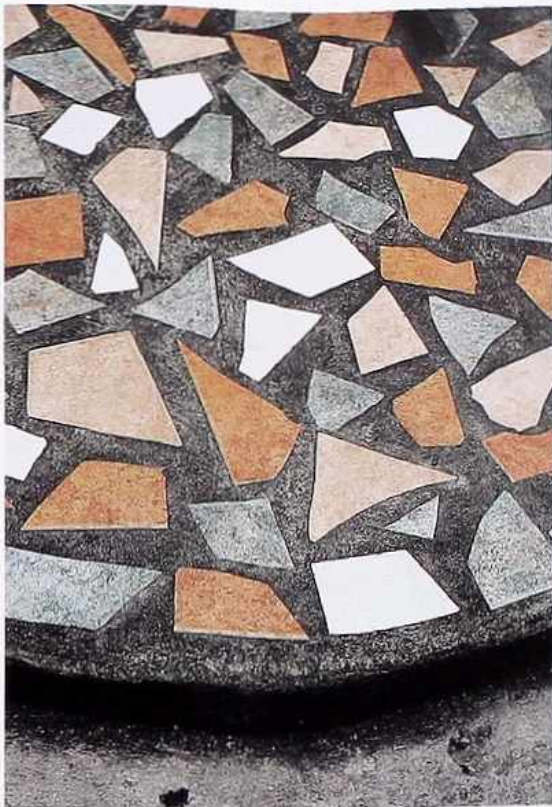
FP-97 Irregular pieces of ceramic tile set in raised concrete, patio
