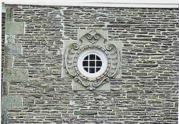
WI-63 Circular window divided by muntins, with a carved stone frame
