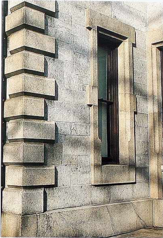
WA-93 Sawn granite in random ashlar with tooled quoins; flat granite window and base trim
