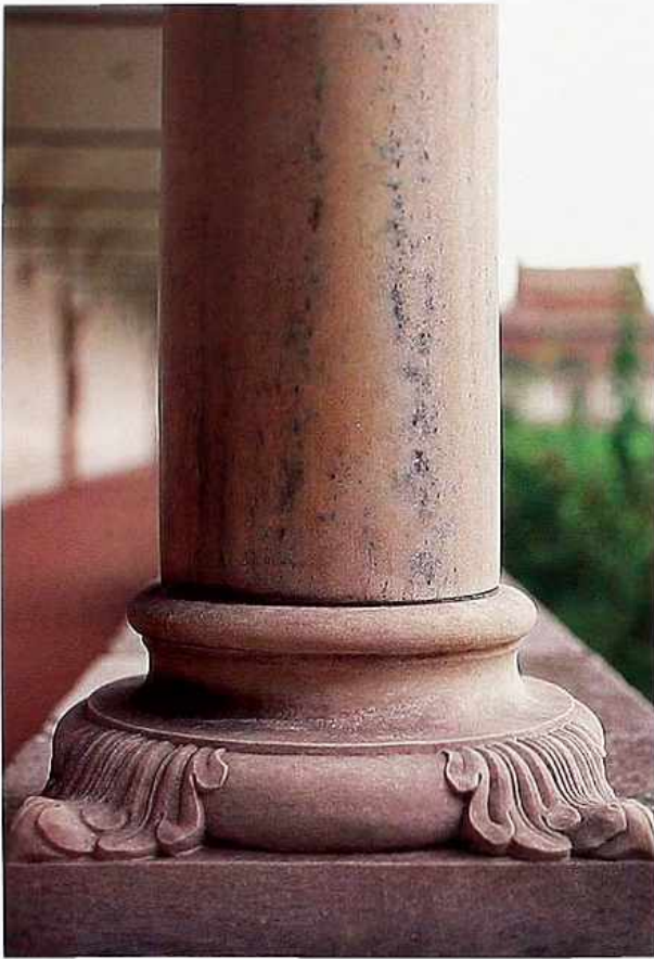
CP-31 Idiosyncratic marble Attic base with foliated ornament draped over torus on plinth
