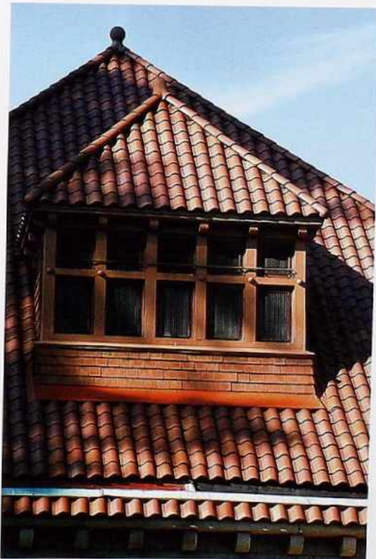
CR-91 Hipped gable roof dormer; dormer and roof clad with pantiles
