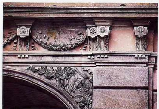
OM-52 Arch with sculpted spandrel. Entablature with frieze and festoons between consoles terminating in guttae below molding
