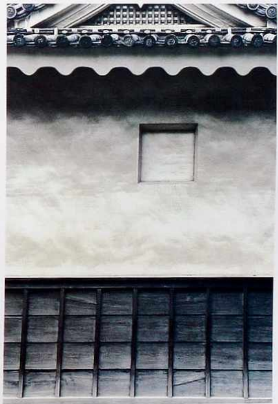
WA-281 Timber frame with infill of undulating stucco and framed planks, traditional Japanese building
