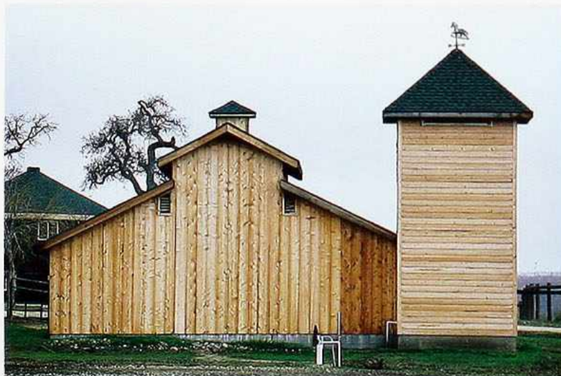
CR-119 Left: gable with gable monitor and cupola; right: pyramid roof with weather-vane
