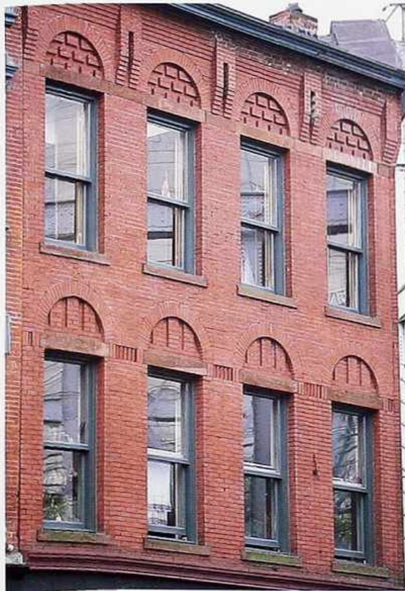
WI-57 One-over-one double-hung metal or vinyl replacement windows, 19th-c. brick apartment building
