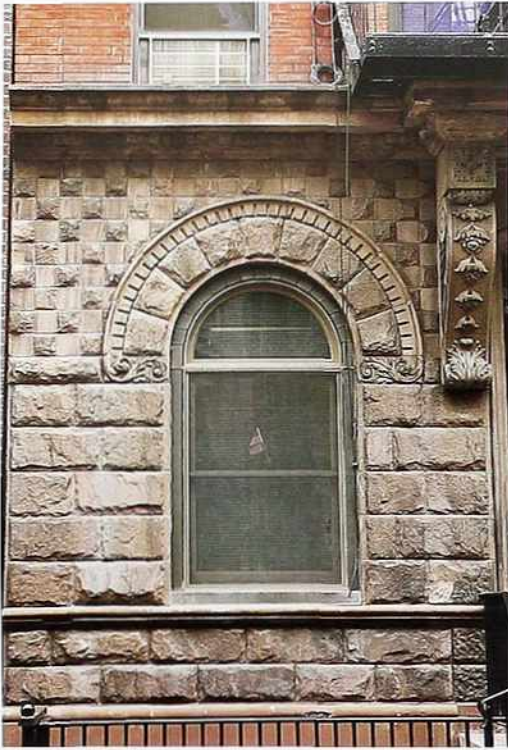
WI-140 Ornamented brownstone voussoirs around semi-circular-arch window
