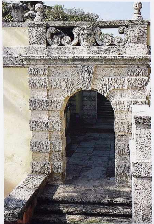
CP-168 Rusticated coquina garden portal with semicircular stepped arch, crossettes, banding, and ornamented balustrade with a mascaron
