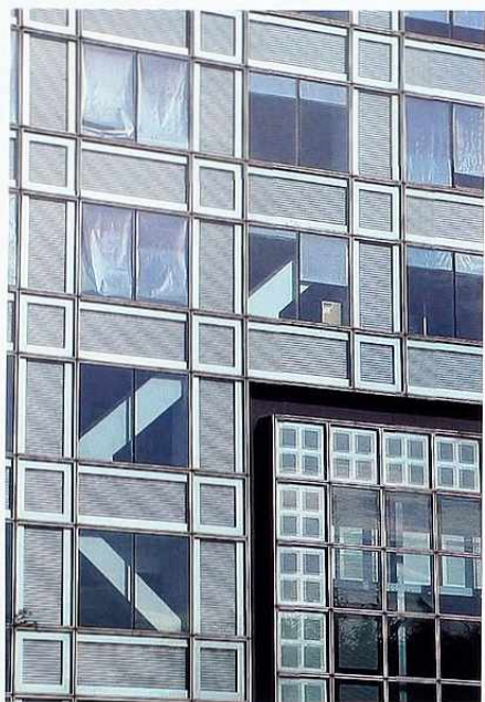
FA-128 Curtain wall with geometric design in clear and opaque glass spandrels and column covers with raised edges and mullions
