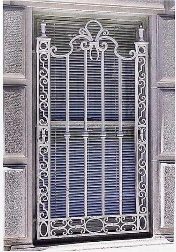
WI-168 Painted wrought-iron window grille with decorative border
