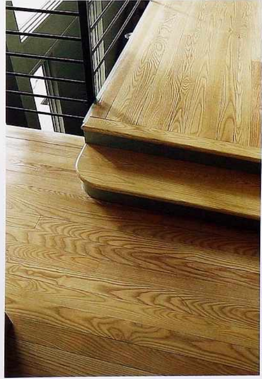
FP-7 Ash flooring and steps with rounded nosing in balcony hallway
