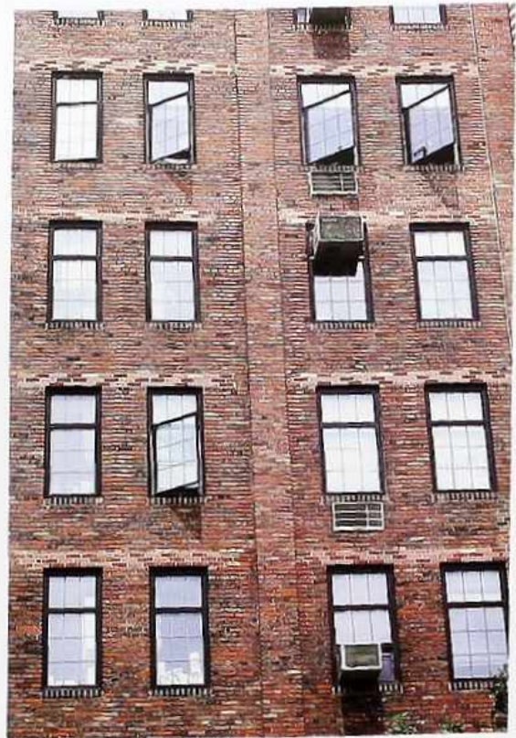
WI-31 Casement windows with internal muntins and fixed light above, modern metal replacement windows in older apartment house
