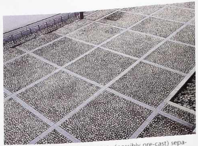
FP-73 Squares of exposed aggregate (possibly pre-cast) separated by metal or concrete grid in courtyard of modern commercial building
