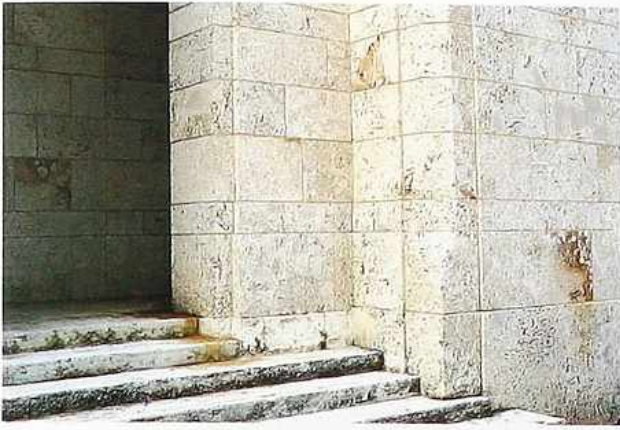
WA-126 Sawn-fossil-stone wall and staircase in coursed ashlar
