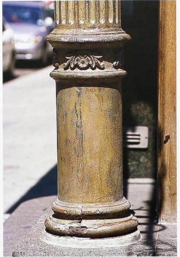
CP-59 Fluted column with Doric base on round pedestal with Attic base and floral ornament
