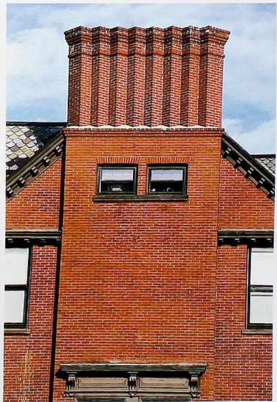
CR-146 Engaged rectangular chimney stack
