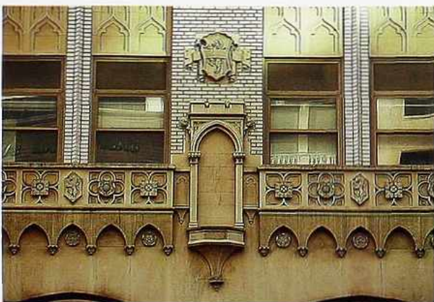
OM-61 Top to bottom: cartouche over a niche; alternating ornamental panels with quatrefoil devices with rosettes; Gothic molding
