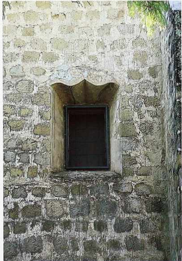
WI-121 Shaped embrasure in coursed-rubble wall, 19th-c. American Southwestern mission
