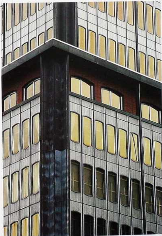
WI-17 Bronze mirror-glass windows in curtain wall, modern commercial building
