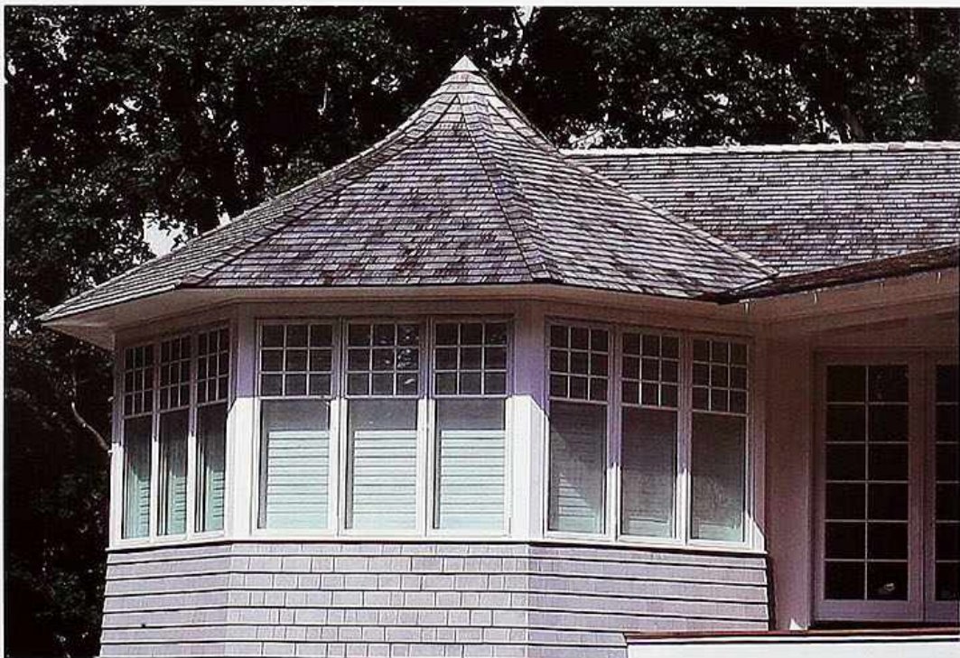
WI-82 Cant-sided bay with three windows per side, conical shingle roof, modern house
