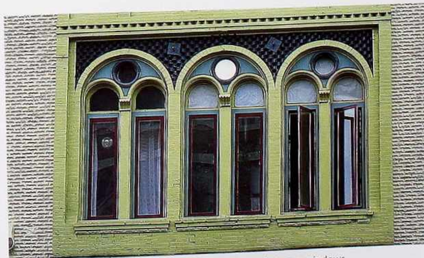
WI-29 Venetian-style casement windows with pilasters between windows
