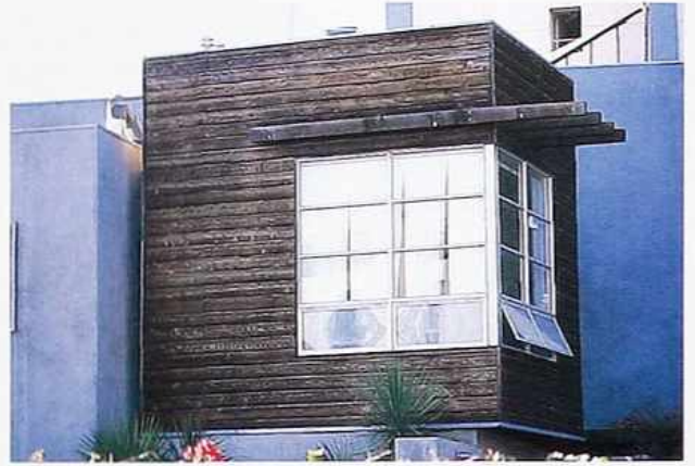
WA-52 Horizontal stained shiplap siding with corner awning windows, modern house
