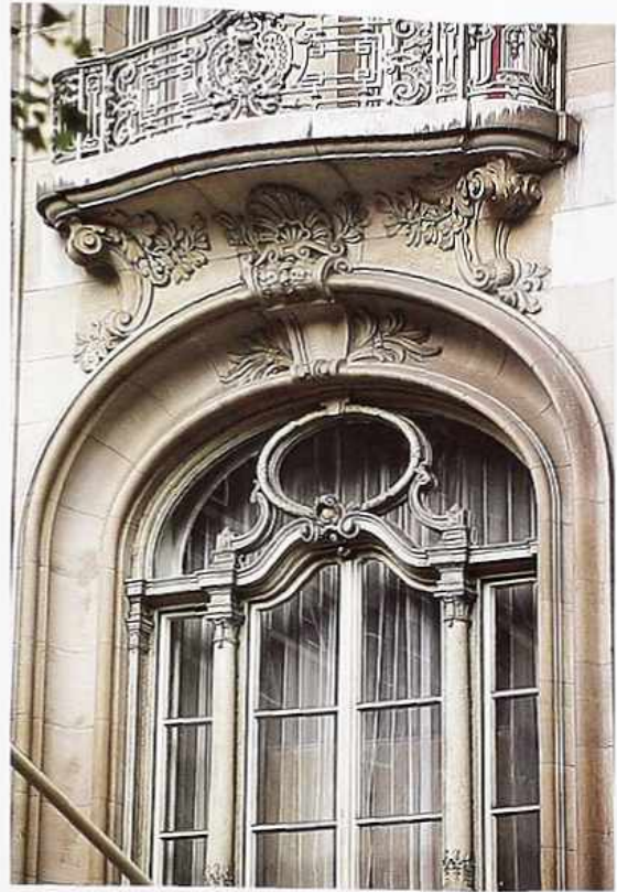
WI-95 Shaped stone transom light over French door with side lights under engaged balcony
