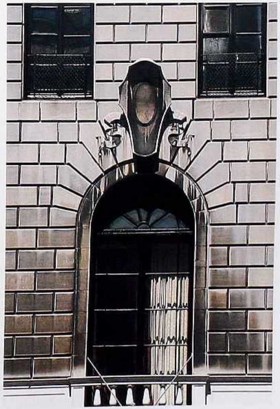
WA-113 Weathered sand-finish limestone in running bond, with cartouche keystone in stepped arch
