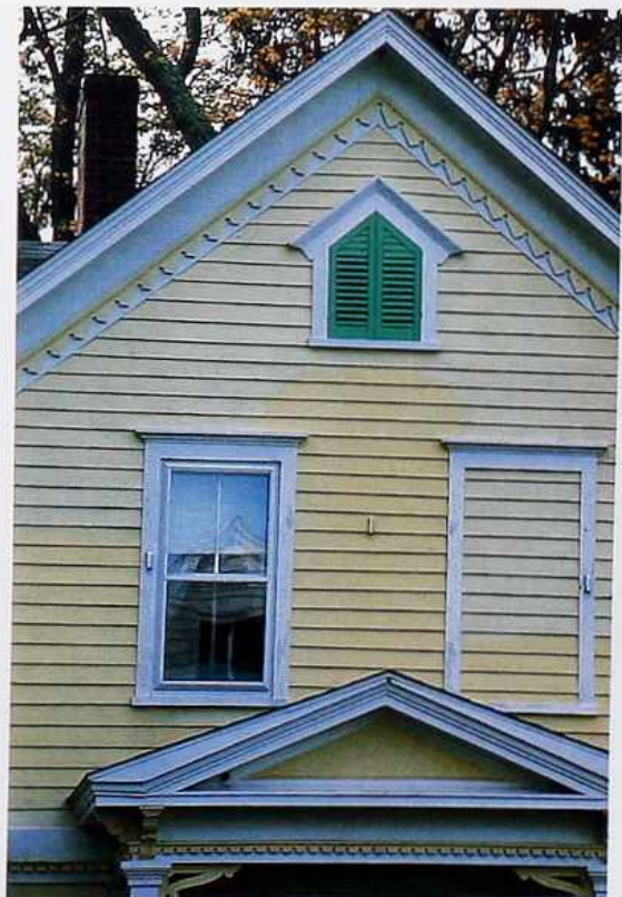
WA-35 Clapboard end-gable wall with shuttered gable window, blind window, scalloped rake trim, and pedimented porch, Greek-revival house
