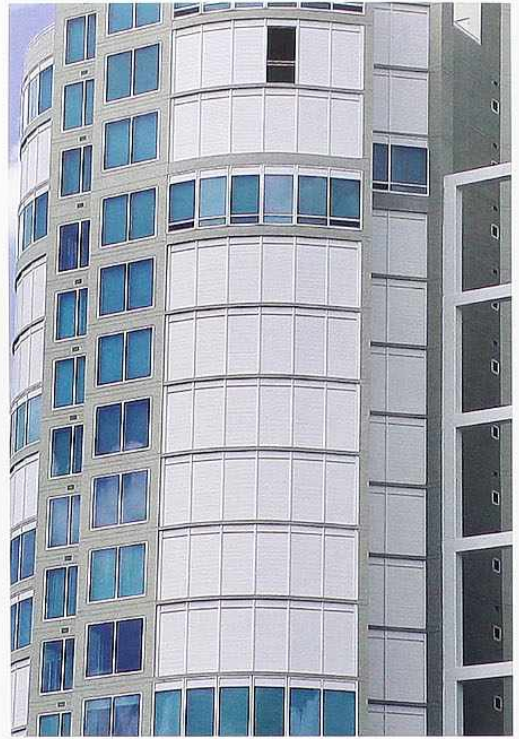
WI-203 Hurricane shutters, modern apartment house
