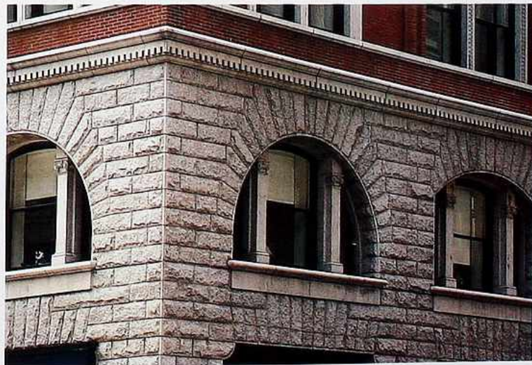
WA-105 Split-faced coursed ashlar granite wall with dentil cornice and arched windows: Florentine (left and center), segmental (right), with jack-arch entries below
