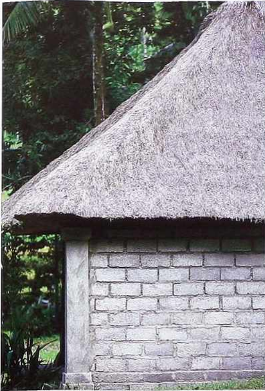
CR-70 Trimmed thatch on concrete-block building, Bali
