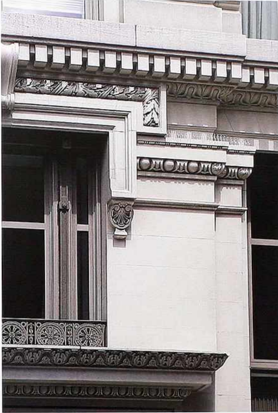
OM-82 Dentilated cornice with enriched moldings; crossette over window (left)
