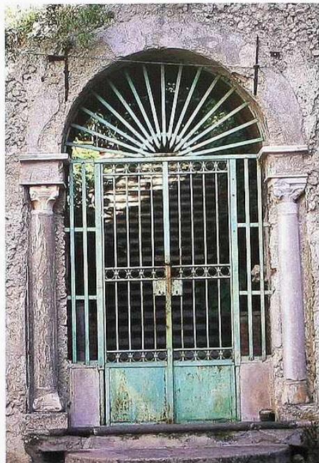
DW-115 Metal double gate with open bars and fan-shaped top panel in rustic stone arch with impostes on engaged columns
