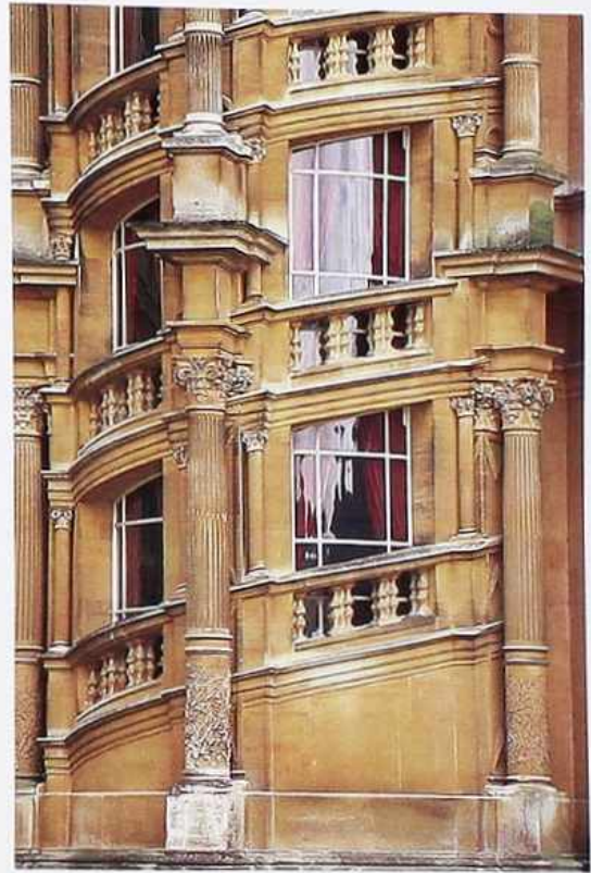
FA-109 Stair tower with engaged columns and spiral balustrade
