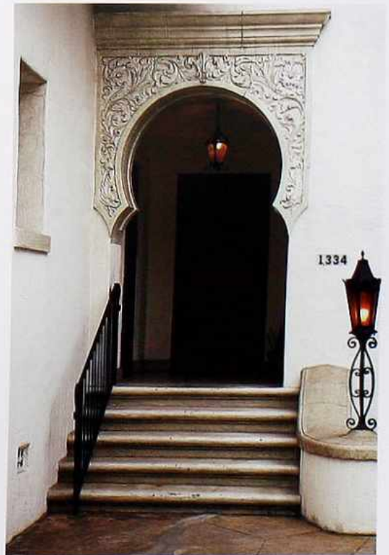
DW-93 Recessed entry with ornate horseshoe arch and steps
