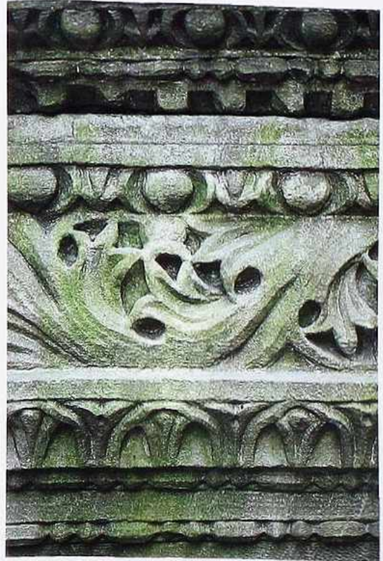
OM-64 Stone molding. Top to bottom: egg-and-dart, dentil band, fascia, egg-and-dart ovolo, foliated band, leaf- or heart-and-dart, fascia between two bead-and-reel moldings
