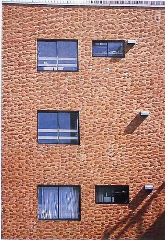
WA-179 Mottled effect in polychrome toned brick, modern residential building
