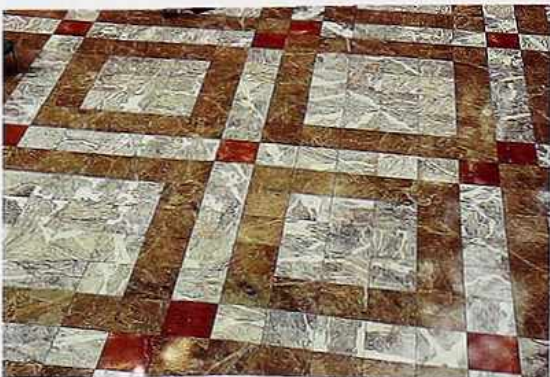
FP-17 Marble parquet in polychrome geometric pattern, interior of modern commercial building
