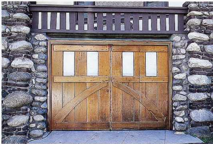
DW-31 Wood double garage doors with lights and curved Z-braces in field-stone wall, Arts and Crafts house
