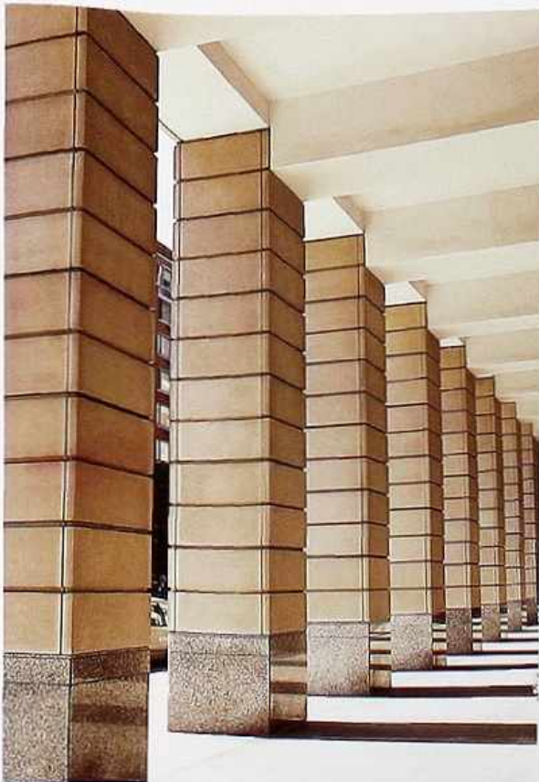
CP-136 Polished rusticated granite-veneer piers with adjoining boxed beams in arcade, modern commercial building
