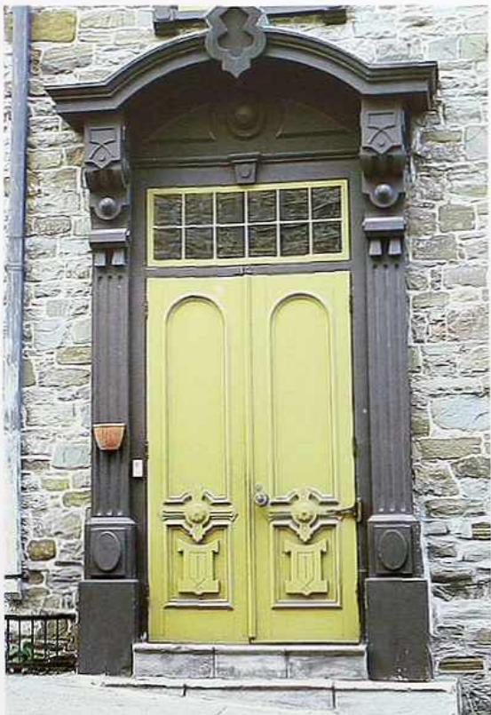
DW-80 Door hood: arch with ornate pilasters, carved paneled doors, twelve-light transom panel; 19th-c. building
