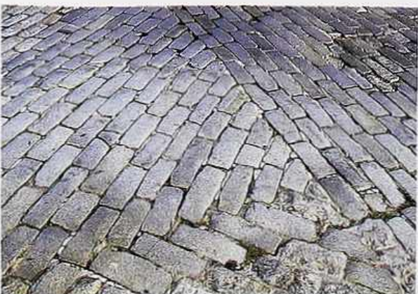
FP-35 Jumbo cobblestones in intersecting running bonds on an ancient street
