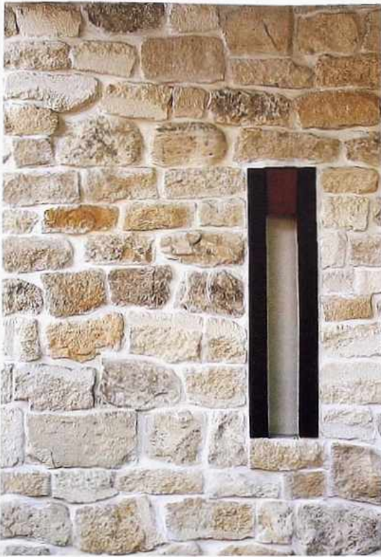
WA-56 Split-faced roughly squared sandstone in coursed rubble with ventilation slit
