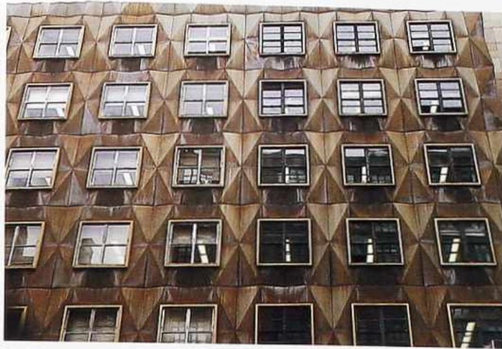
FA-23 Weathered panelized wall system with stamped diamond pattern, modern apartment house
