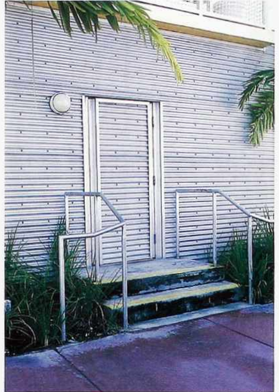
FA-20 Corrugated galvanized steel panels with visible fasteners, modern commercial building
