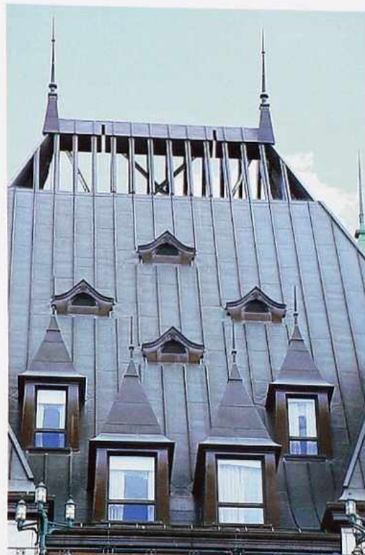
CR-100 Four flared-gable roof dormers above flared pyramidal roof dormers on metal hipped roof
