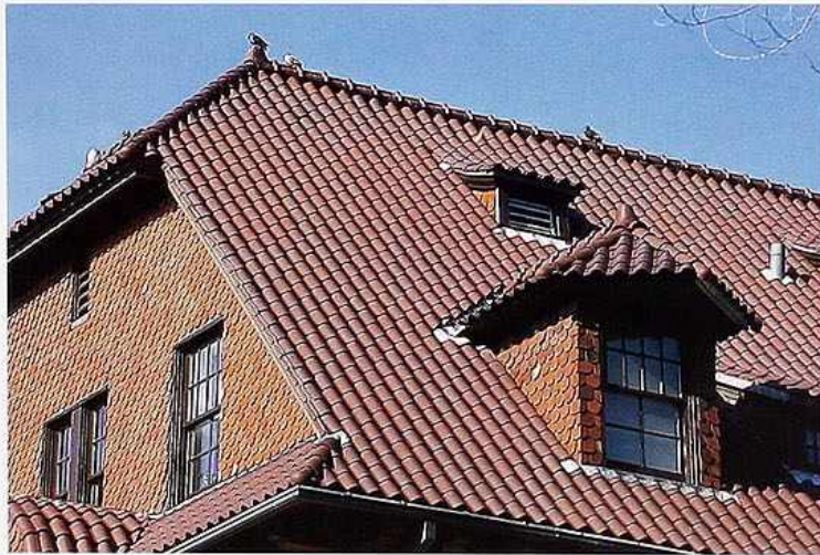
CR-87 Dormer with hipped roof on jerkinhead tile roof with scalloped terra-cotta tiles, gable-end wall
