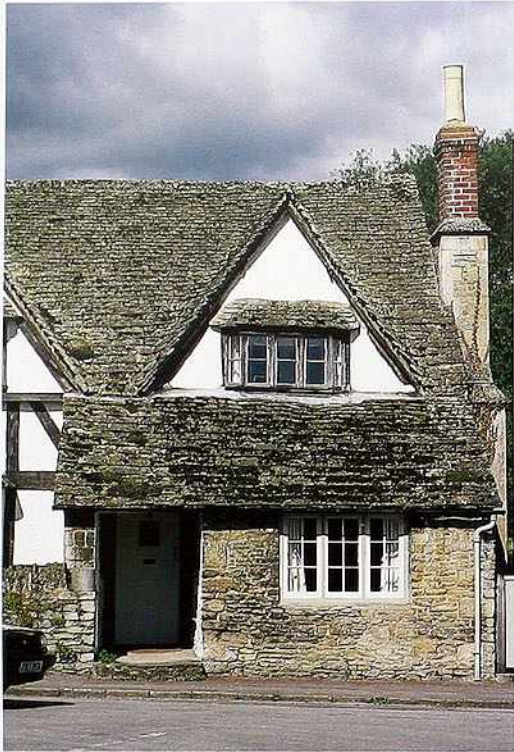
CR-126 Slate gable roof and gabled roof dormer with bay
