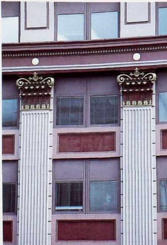
CP-82 Flush fluted pilasters with Corinthian-style capitals
