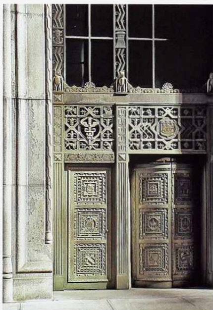
DW-48 Cast-bronze paneled hinged and revolving doors; pierced transom grille
