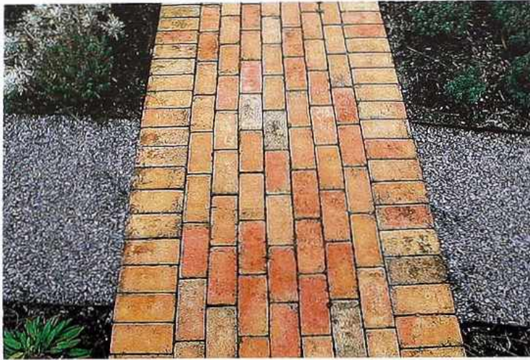
FP-58 Brick pavers in running bond bordered by soldier courses intersecting pebble path; flexible paving, garden walk
