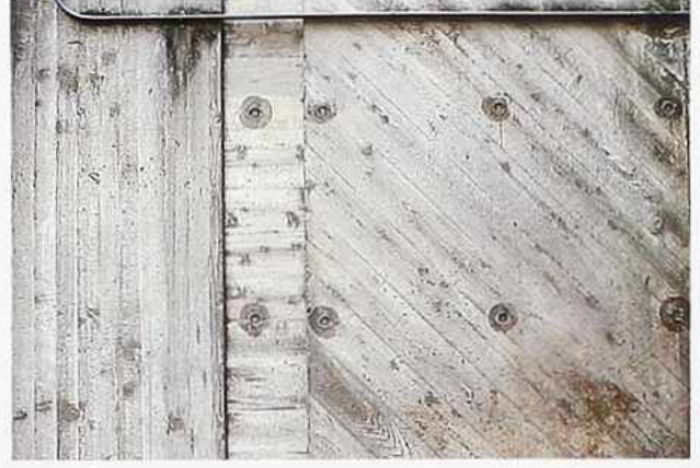
WA-213 Board-formed concrete with textured finish from wood formwork
