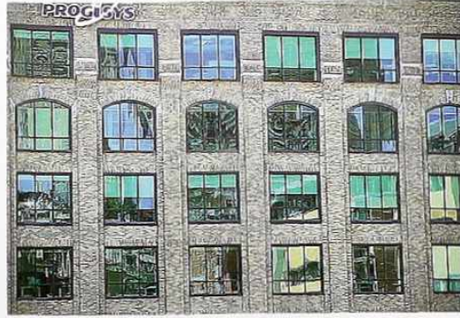
WI-159 Banded fenestration: row of arched windows and rows of square windows; metal replacement windows, 19th-c. industrial building
