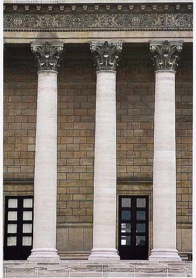
CP-74 Corinthian columns supporting portico
