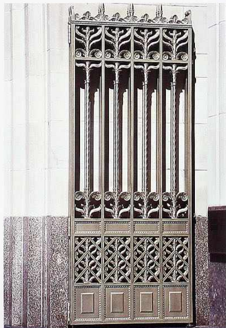
DW-117 Cast-bronze gate coated with sealant to prevent patination, commercial building
