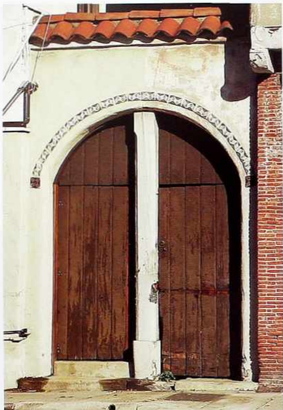
DW-23 Arch-shaped wood double doors with center pilaster; stucco surround, American Southwestern mission style
