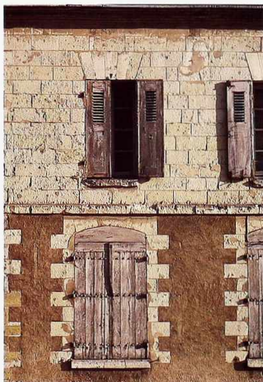
WI-197 Weathered painted wood paneled shutters
