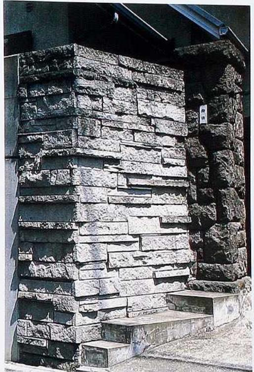
WA-94 Split-faced granite wall in shelf, random ashlar with roughly squared rubble pillar (right)
