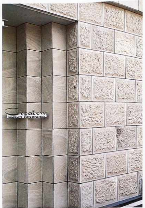
WA-132 Corner of rusticated running bond with reveal; sand-finish pilaster strips in stack bond on entry, modern commercial building
