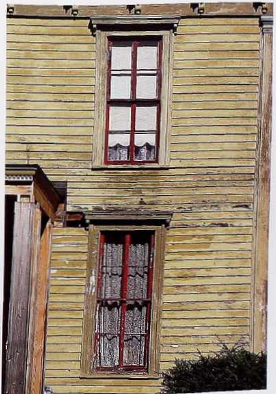
WI-47 Four-over-four double-hung windows with crown molding, 19th-c. American clapboard house
