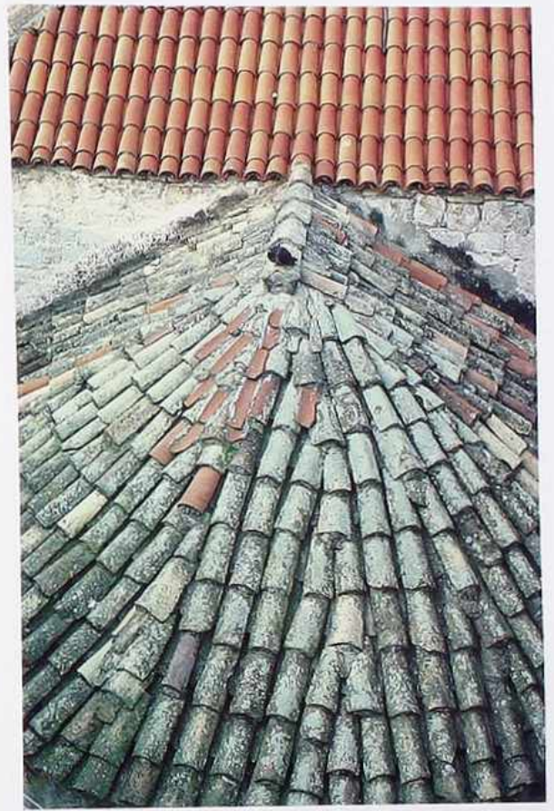
CR-41 New and weathered terracotta mission tiles. Top to bottom: shed roof; gable roof, half-cone roof
