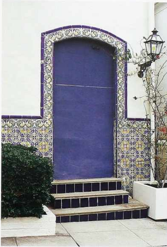
DW-90 Spanish-colonial-style recessed door in segmental arch framed with decorated glazed tiles on stucco wall; Mexican tile steps
