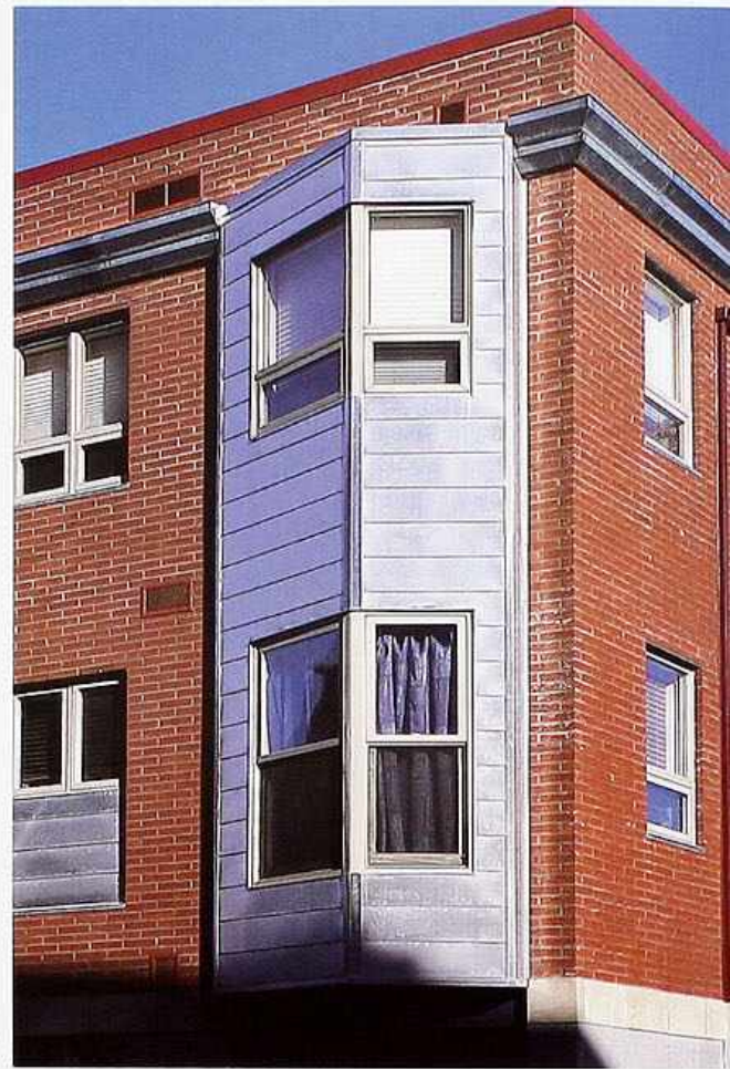
WI-81 Metal-clad two-story angled bay. Top: fixed windows with awning lights; bottom: one-over-one double-hung sashes, modern apartment house
