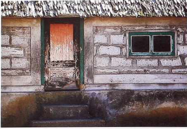
WA-221 Weathered handmade concrete block with mortar in irregular running bond on house
