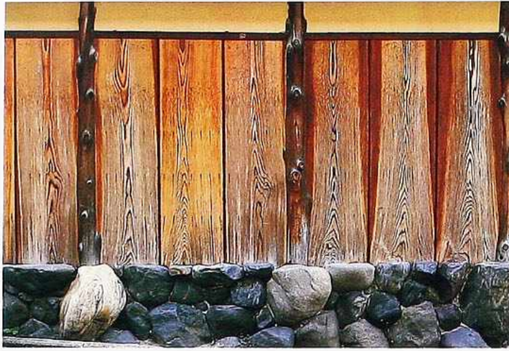
WA-44 Weathered unfinished plain-sawn planks with vertical undressed timbers on rubble foundation
