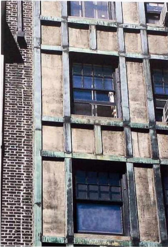
WA-278 Decorative half-timbered facade with concrete infill and copper "timbers," 20th-c. residential building
