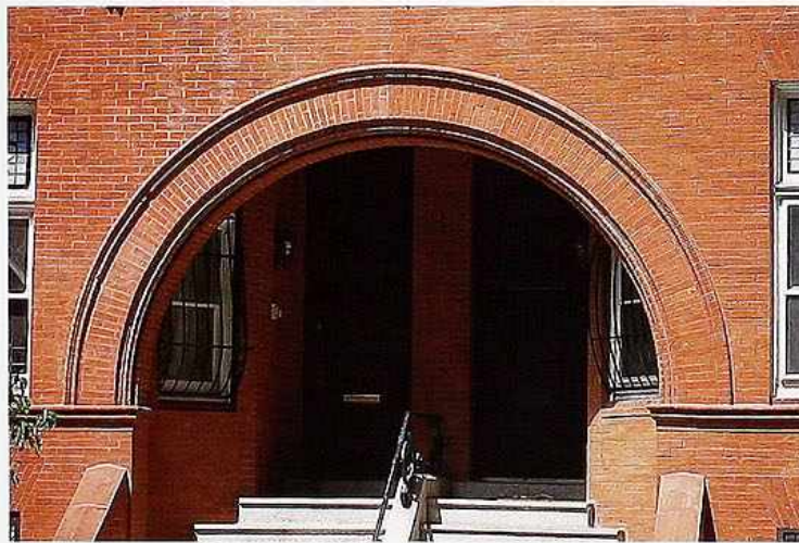
CP-157 Semicircular gauged-brick arch over entryway
