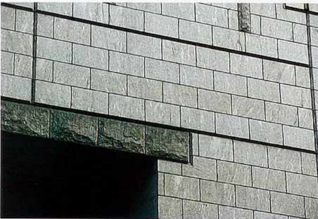
WA-128 Rock-face granite doorway lintel with contrasting sawn-granite panels in running bond with wide V-shaped joints
