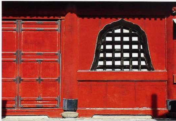
FA-73 Traditional red painted wood-infill post-and-beam facade and paneled door, Japanese entry gate
