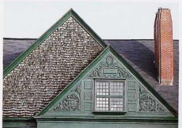
CR-83 Wall dormers. Left: shingle-clad; right: wood with carved ornament, American house
