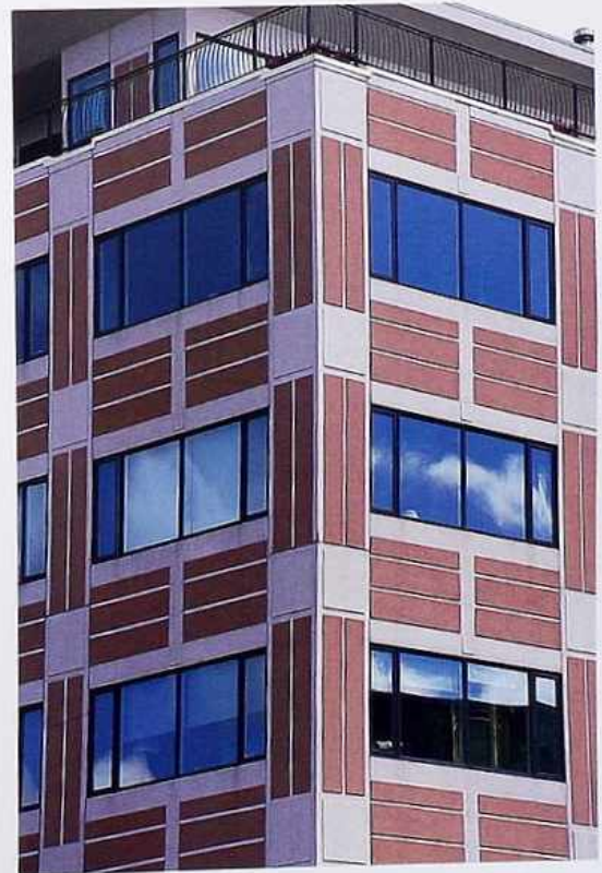
FA-127 Trabeated facade finished in colors suggesting post-and-lintel construction, modern mixed-use building
