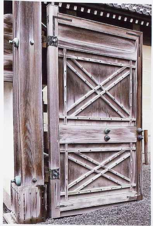
DW-13 Weathered two-panel wood with double cross-braces, brass hardware, and doorknob in center stile, Japanese courtyard gate
