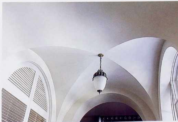
CR-9 Plaster vaulted ceiling, traditional house
