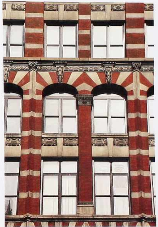
WA-287 Banded brick-and-stone arches with carved ornament in keystones and spandrels
