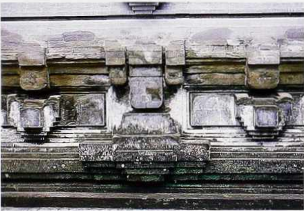
OM-69 Stepped fascia moldings, inset panels, corbelled block, and modillion-like elements
