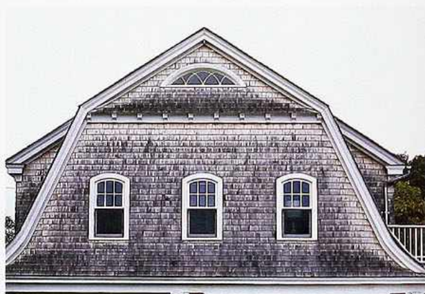
CR-96 Gable-end wall of flared gambrel roof with white cedar shingles; corbelled tie spanning gable
