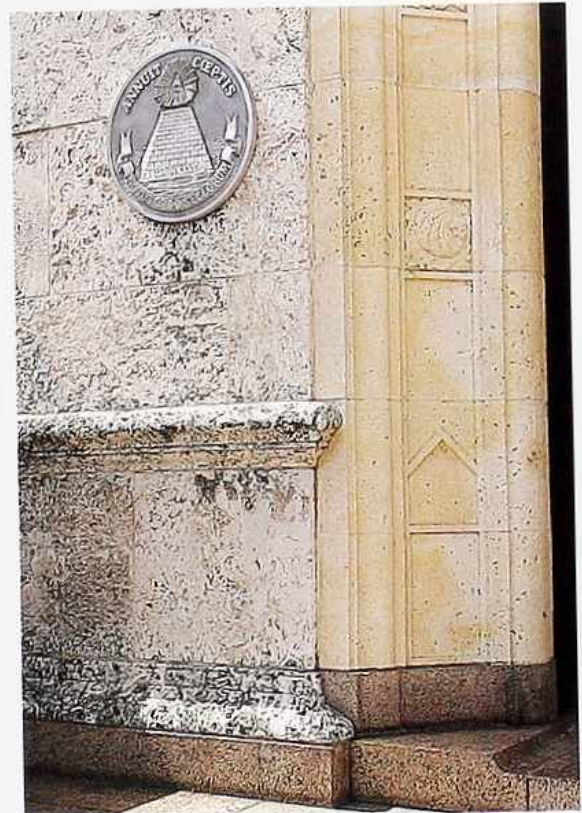
WA-100 Partially honed fossil-stone doorway with water-table course and base molding
