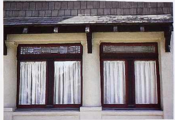
WI-101 Leaded rectangular transom lights over casement windows; hood supported by brackets, Arts and Crafts house
