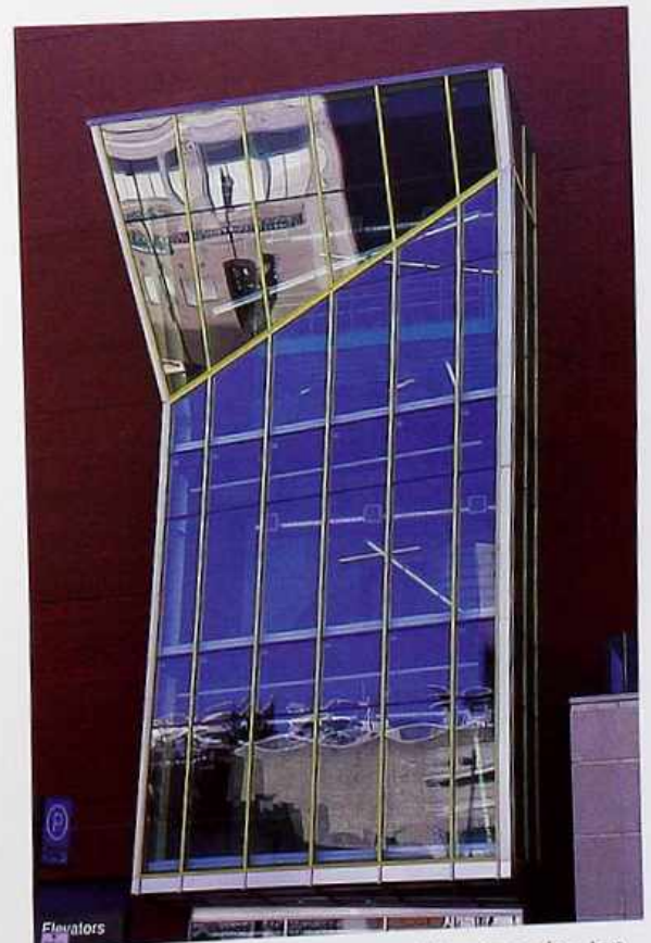
WI-93 Idiosyncratic fixed-light bay with mirror-glass top section, modern commercial building
