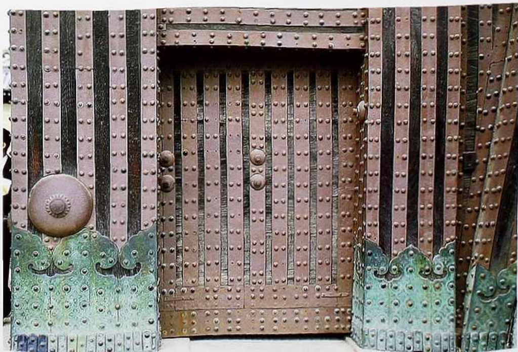
DW-57 Iron door inset in gate wall; bases of adjacent reveals clad in decorative metal work; 16th-c. Japanese castle
