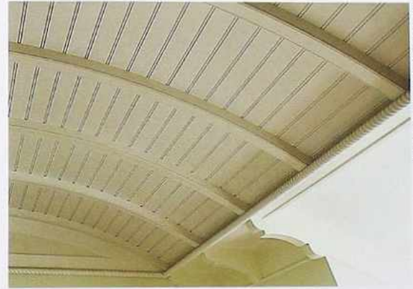
CR-8 Painted barrel ceiling with tongue-and-groove between exposed ribs, modern house
