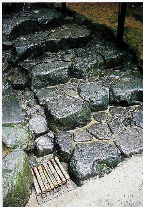
FP-46 Steps made from roughly squared split, polished fieldstone set in concrete. Bottom left: bamboo drain cover
