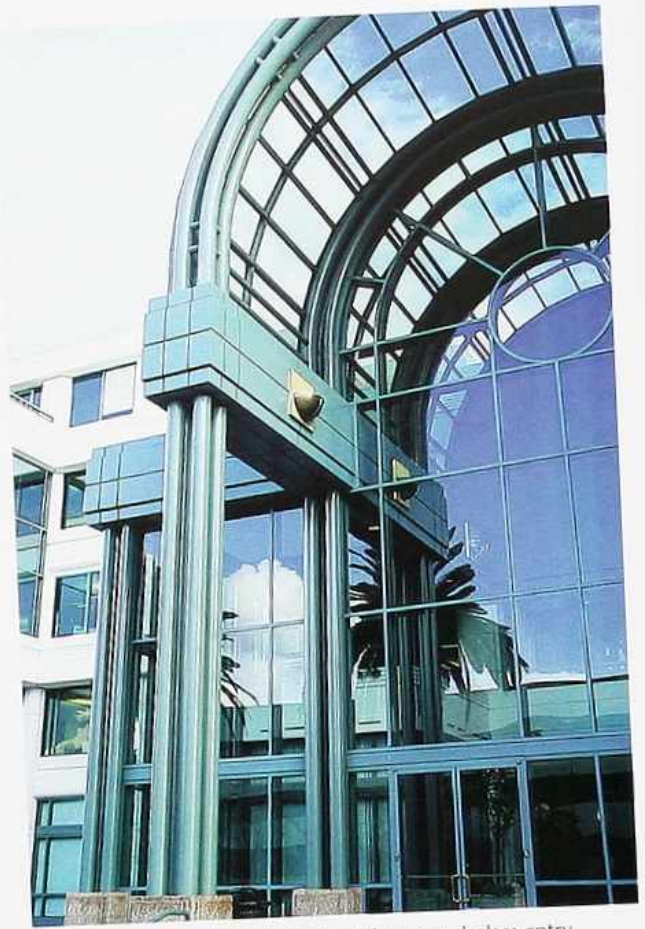
CP-177 Barrel-vaulted tubular-steel-frame-and-glass entry, modern commercial building
