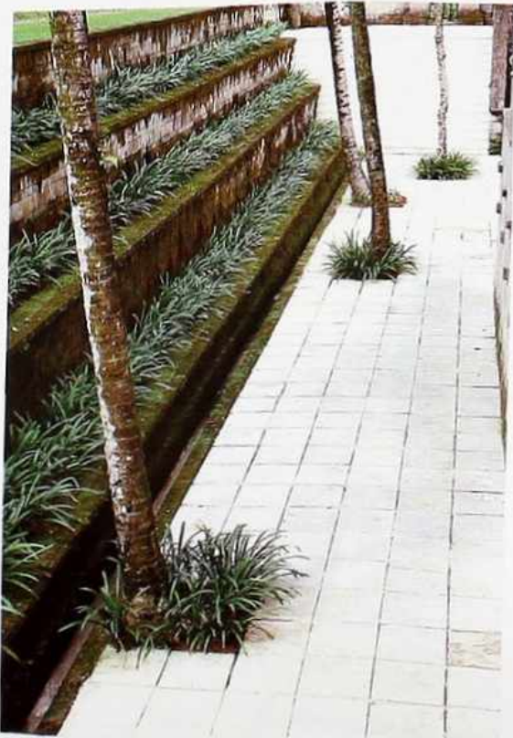
FP-53 Paving stone made from river stone and cement, Indonesian courtyard
