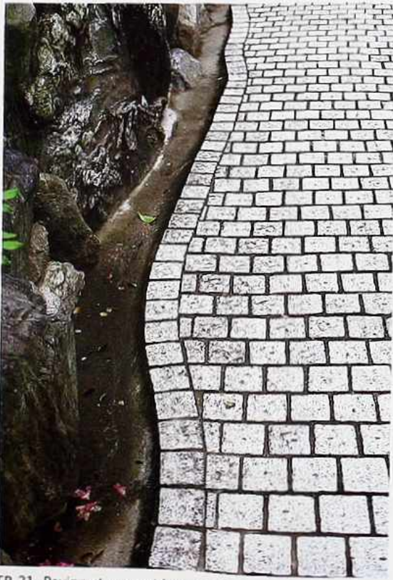
FP-21 Paving stones set in concrete in running bond with soldier-course border adjacent to natural rock wall, garden path
