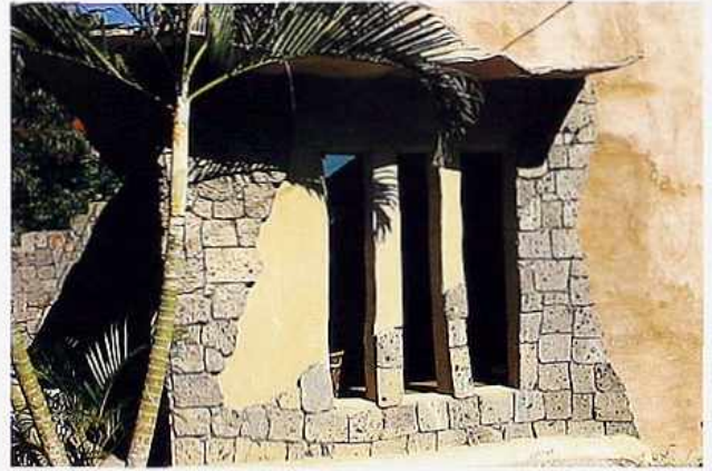
WA-241 Stucco over random ashlar stone
