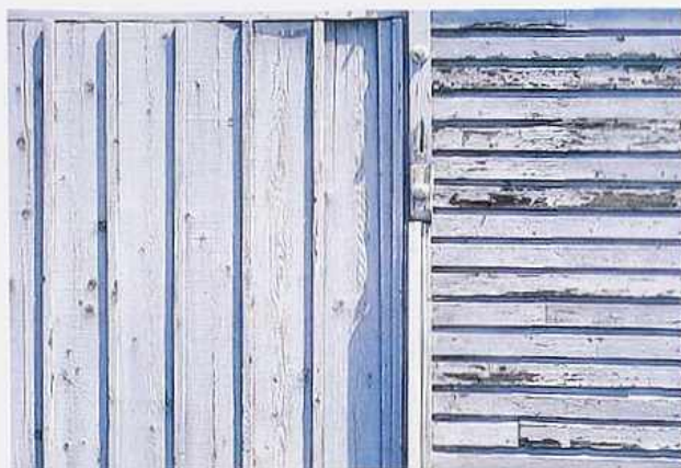
WA-11 Weathered painted wood siding. Left: board-and-batten; right: clapboard
