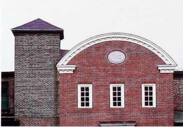
CR-122 Compass roof, fascia with modillions
