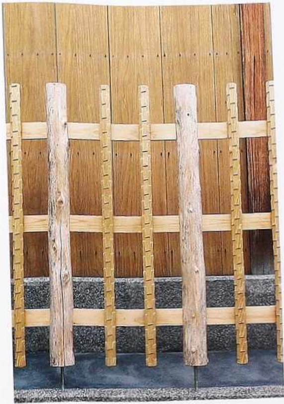
DW-110 Unfinished-wood entry gate of alternating notched square stock and roughly dressed timber posts attached to horizontal battens
