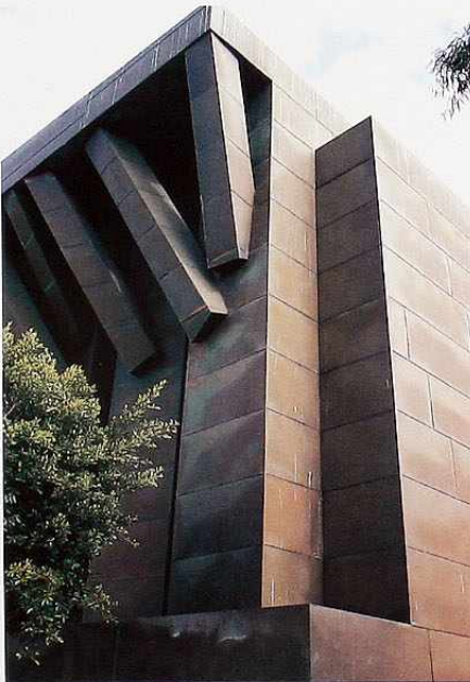
FA-13 Copper cladding, modern commercial building
