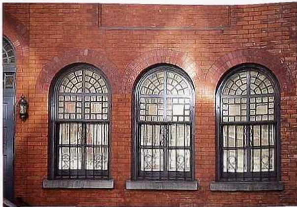
WI-100 Semicircular-arch fanlights over square fixed lights, with one-over-one double-hung sashes and window gates, 19th-c. townhouse
