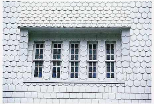
FA-48 Painted sawn shingles in fish-scale pattern on shed dormer
