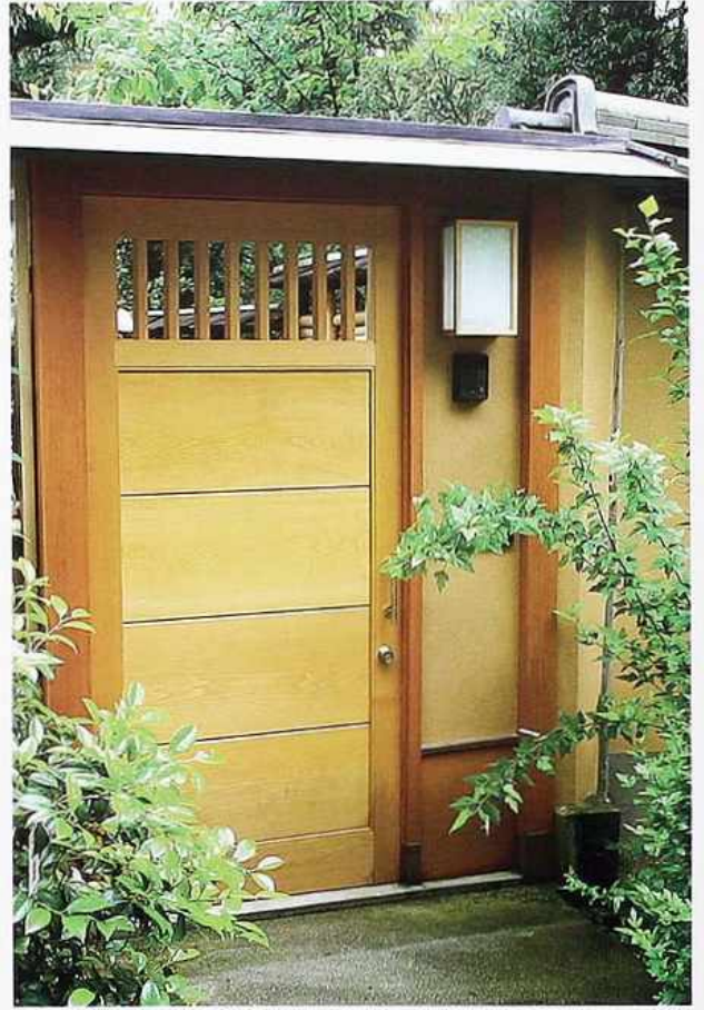
DW-95 Courtyard entry to modern house: door hood over natural wood paneled door with wood grille
