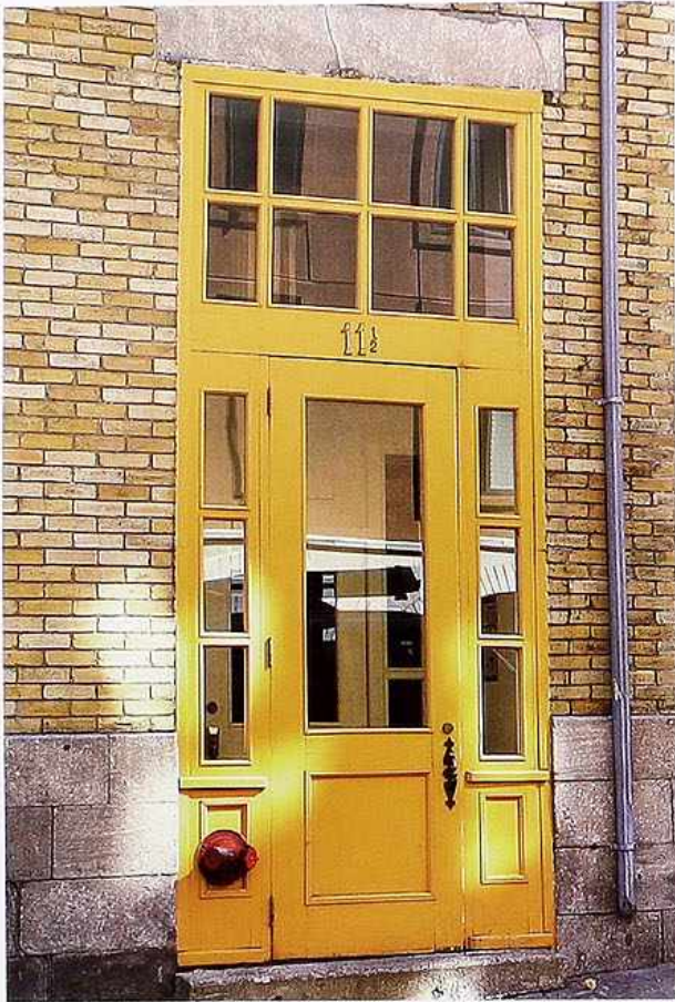
DW-66 Painted wood doorway with eight-light transom panel over three-light side lights and single-light paneled door, commercial building
