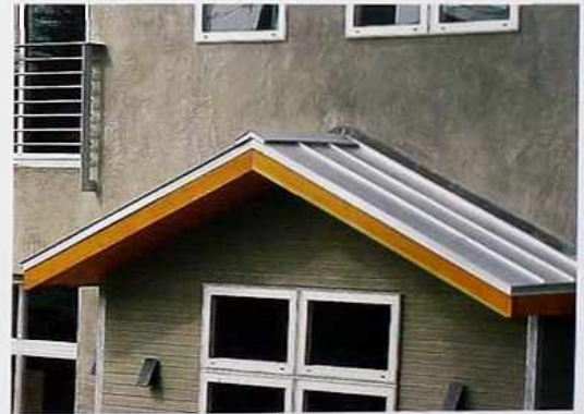
CR-112 Metal and wood gable with eave acting as door hood, modern beach house
