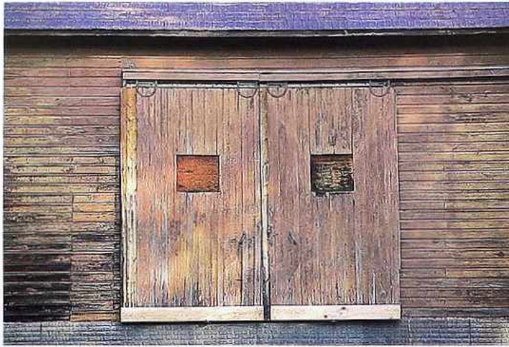
DW-30 Painted wood siding and hanging double doors on weathered barn
