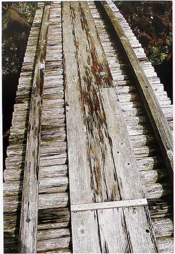
FP-2 Dressed logs with center-sawn planks and wood-peg construction, rustic garden bridge
