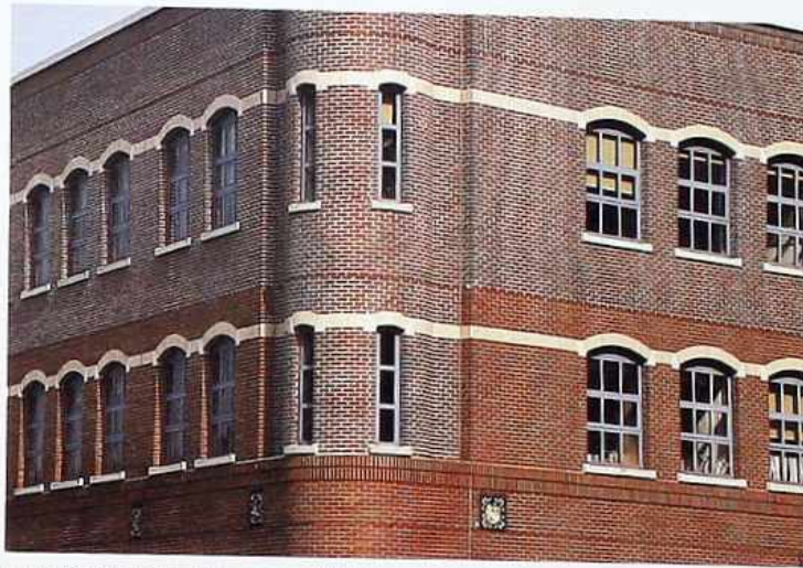
WA-186 Radial brick corner with banding in contrasting colors and masonry; segmental-arch windows, modern commercial building
