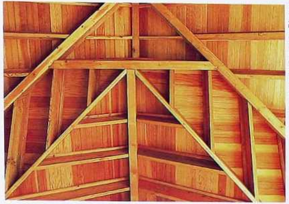
CR-6 Exposed select-fir framing in residential common room
