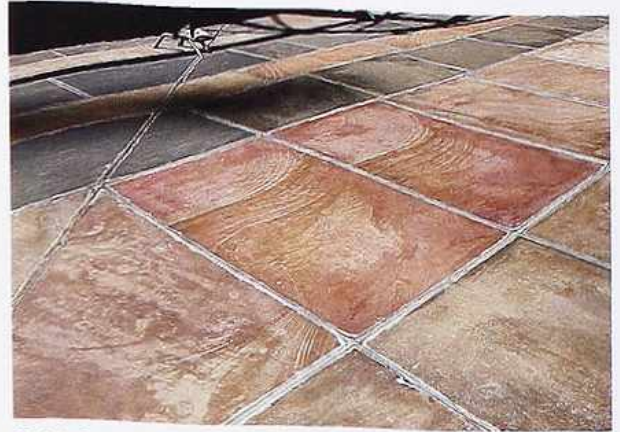
FP-24 Grouted squared bluestone in various colors, sidewalk
