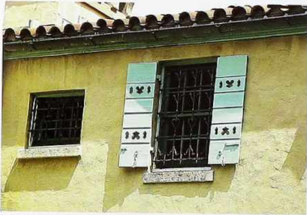
WI-191 Horizontal-board shutters with pierced design
