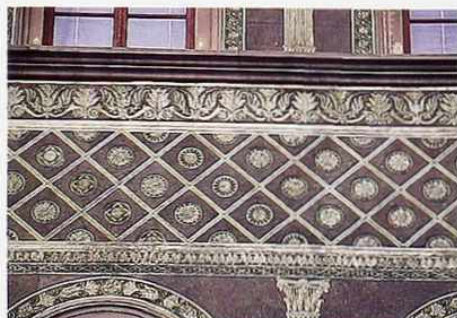
FA-87 Sgraffito depicting pilasters, enriched archivolts, classical moldings, reticulated band with paterae on wall, Italy
