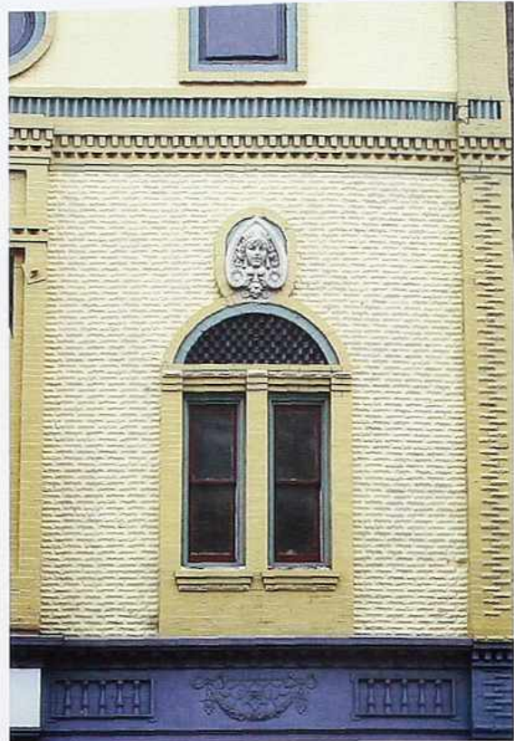
WA-176 Painted rock-face brick with dentil molding, pilasters, and double window under arch in recessed panel with cartouche
