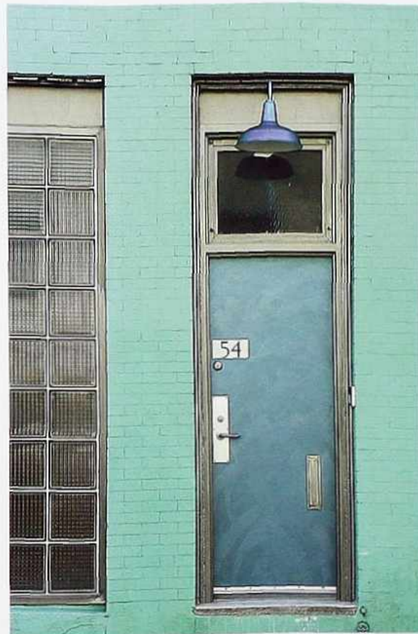
DW-56 Painted metal door with stainless steel hardware; brushed stainless steel doorframe with transom light
