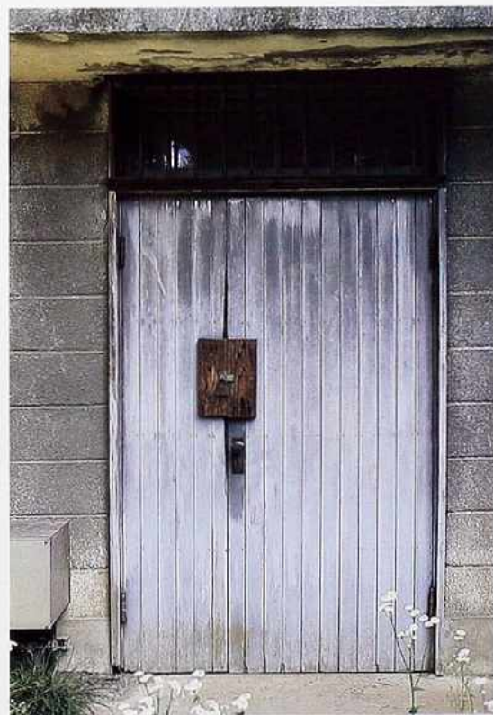
DW-35 Weathered whitewashed wood-plank double doors, concrete-block shed
