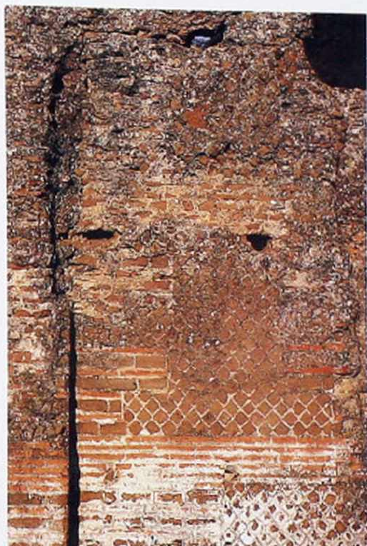
WA-160 Ancient Roman wall with exposed rubble, running and diagonal bonds
