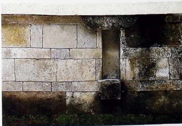
WA-80 Stone in coursed ashlar with bracket, niche, and perpendicular under niche, Bali
