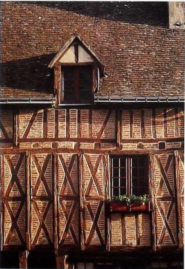
WA-284 Half-timber with brick infill, 15th- or 16th-c. French house
