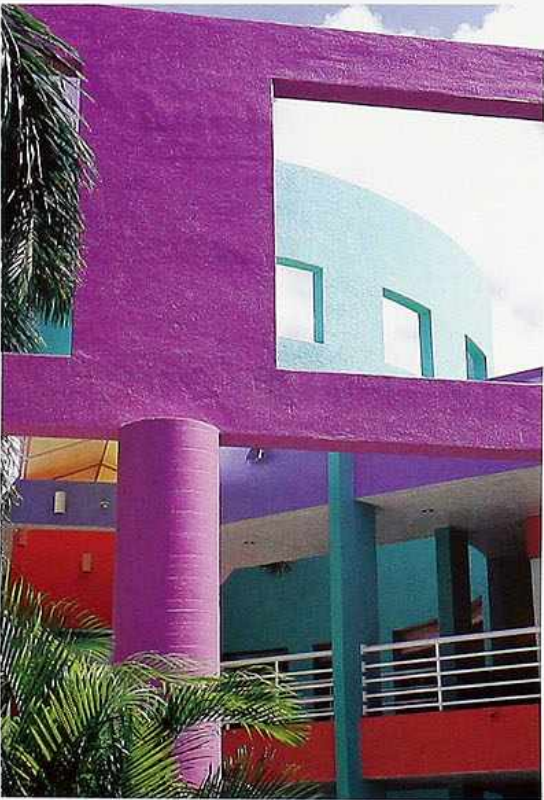
CP-114 Painted poured-in-place concrete pier supporting a steel frame with cladding finished with spray-on stucco
