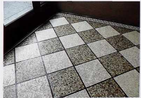
FP-100 Squares of pre-grouted stone mosaic tiles in checker design with dark mosaic grid outline squares, commercial entry
