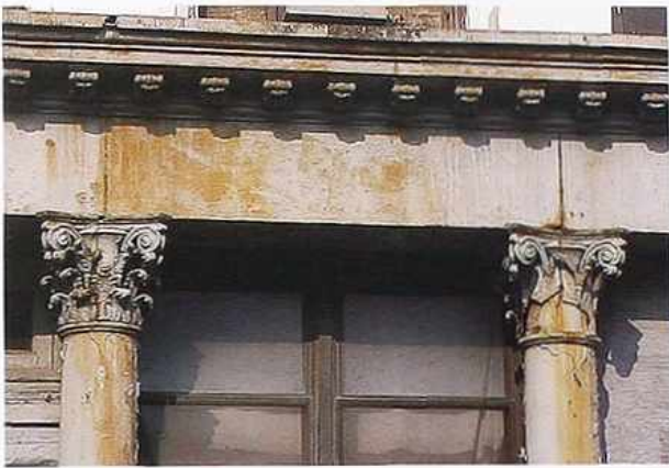
OM-92 Classical entablature: plain architrave, no frieze, modillion band on cornice on weathered tin facade. Weathered tin Corinthian capitals
