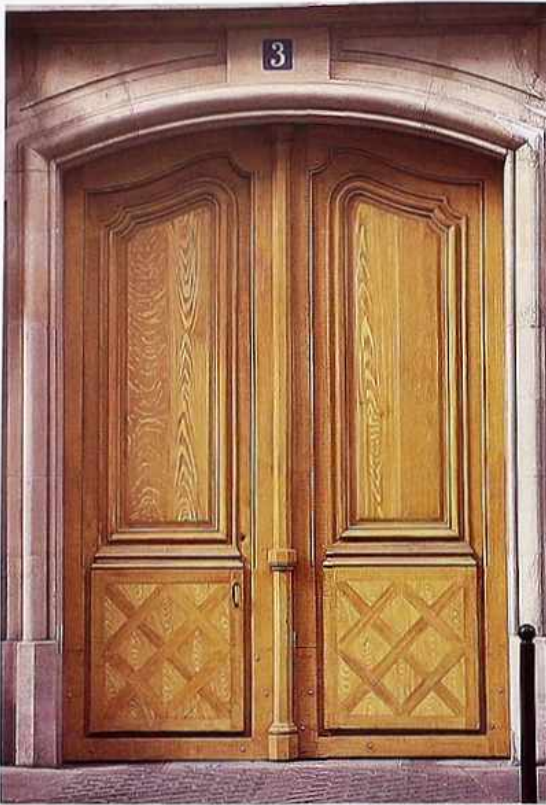
DW-37 Trompe l'oeil wood-grained two-paneled double doors, dimensional flush molding; segmental arch
