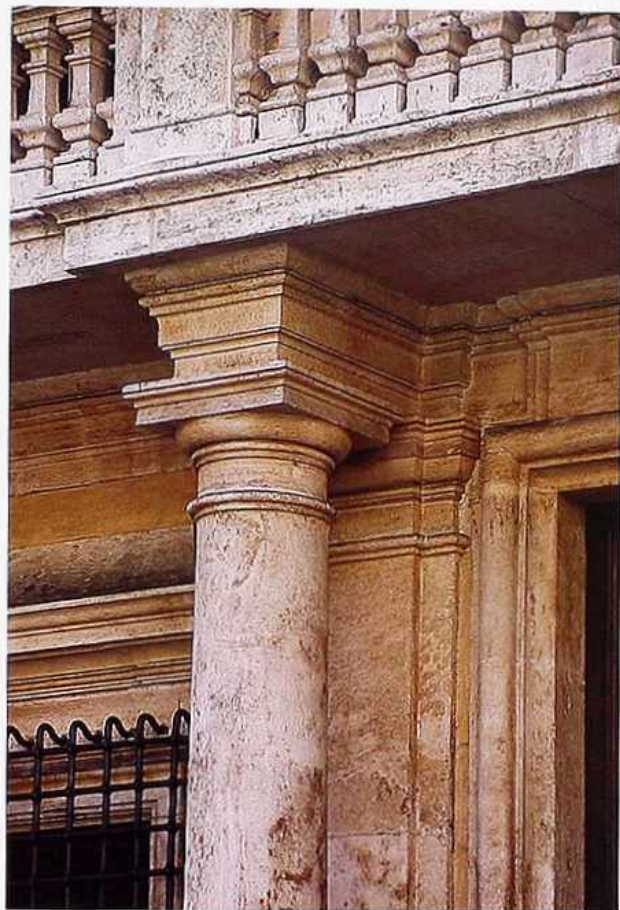
CP-12 Tuscan capital under an overhang with balustrade
