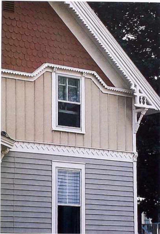
WA-32 Painted siding divided by molding. Top to bottom: scalloped wood shingles; board-and-batten; clapboard. Bargeboard with saw-tooth motif
