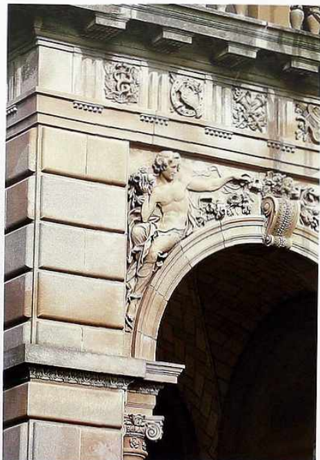
OM-40 Portal with sculpted spandrel, ancon keystone below Doric-style entablature with sculpted metopes and triglyphs
