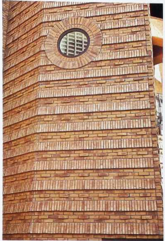
WA-202 Bands of decorative brickwork: running bond alternating with projecting soldier rows; rowlock and soldiers around roundel, modern commercial building
