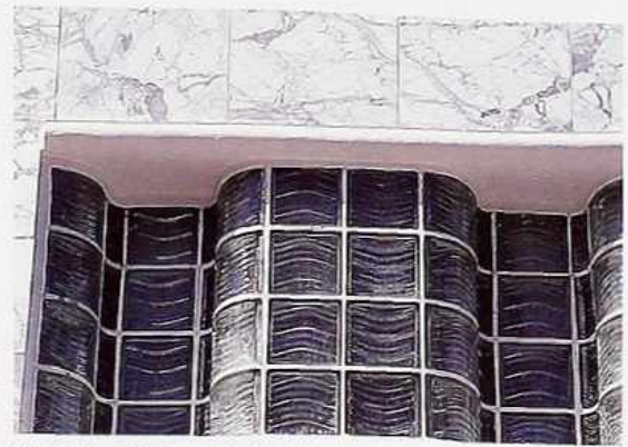
WI-22 Undulating window: flat and curved glass block with wavy texture, Art Deco apartment building
