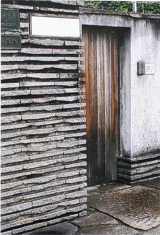
WA-110 Entry wall with flagstones in staggered shelf courses
