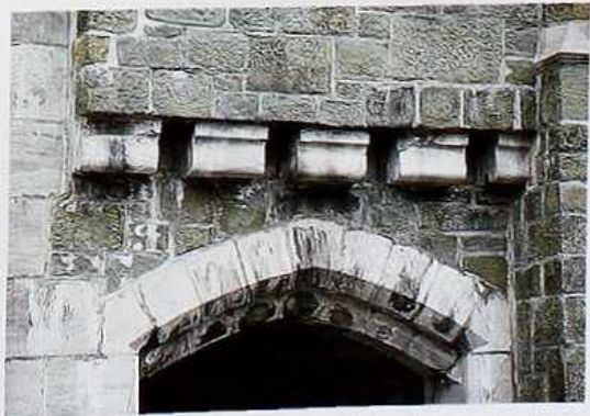
CP-155 Two-centered surbased arch (arch rising less than half its span) in castle entry under corbelled jetty
