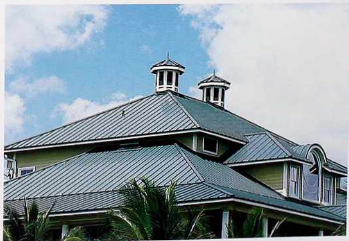
CR-139 Hipped roof with octagonal cupolas, metal with standing seams
