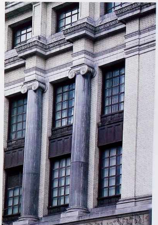
CP-95 Ionic engaged columns with polished granite shafts
