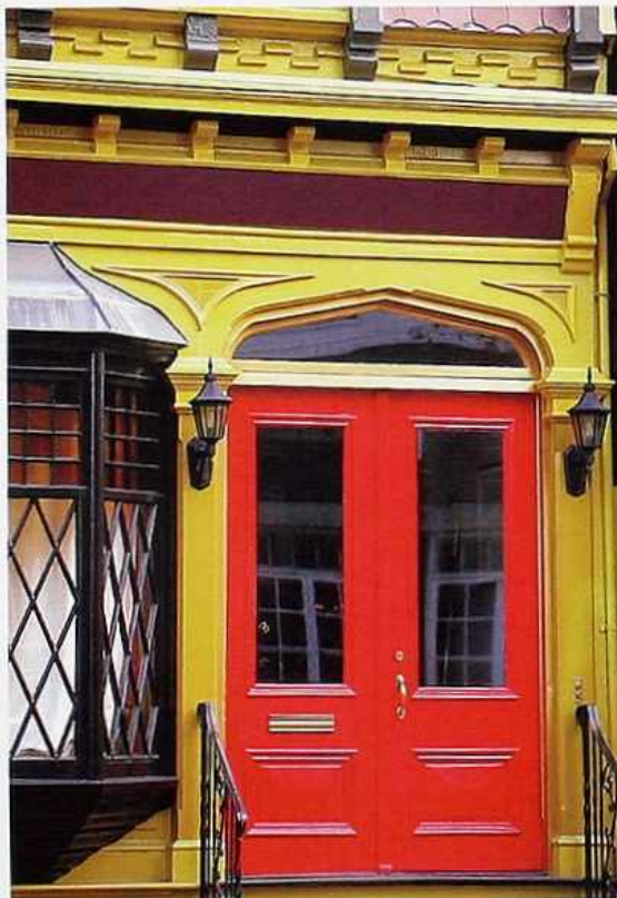
FA-77 Tudor-arch doorway and adjacent oriel painted with exterior gloss colors, 19th-c. storefront
