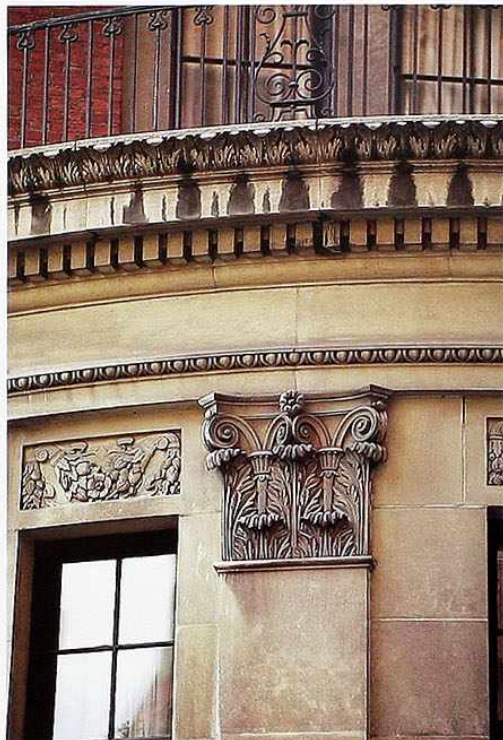
CP-19 Corinthian capital on flat pilaster below weathered entablature with egg-and-dart and dentilated moldings
