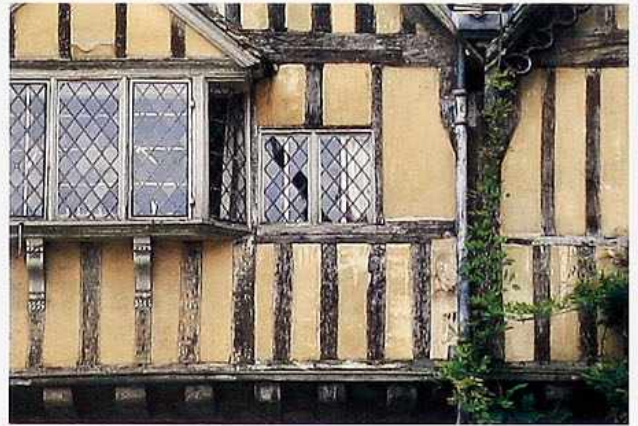
WA-276 Half-timber construction with corbels under jetty; leaded windows, and console supports under oriel, 16th- or 17th-c. English house
