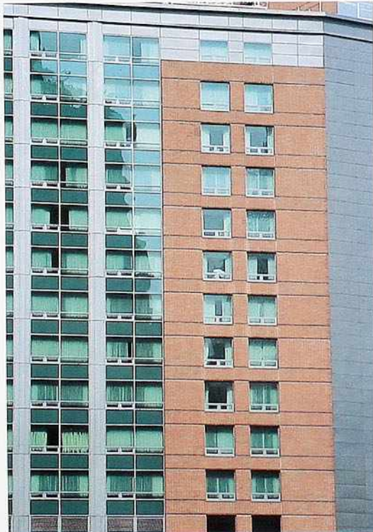
WA-308 Glass, stone, and brick modern commercial building
