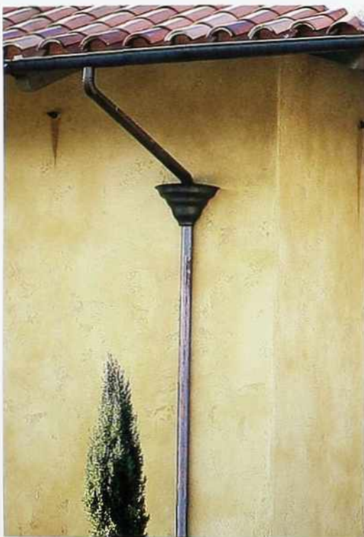
CR-157 Metal gutter, drainpipe, and rainwater head
