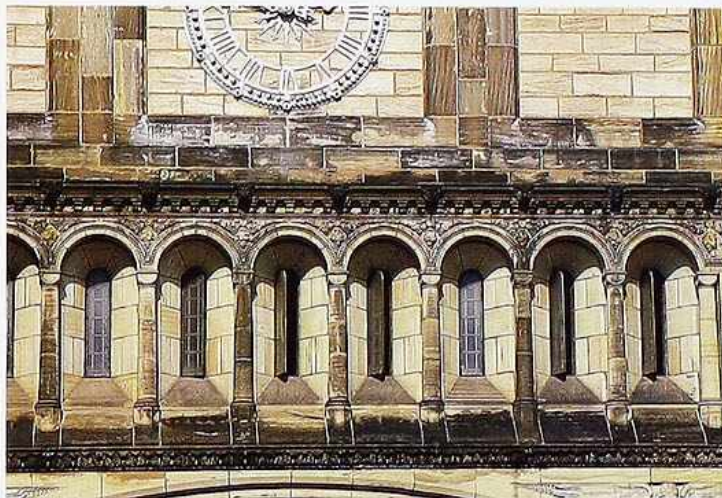
CP-174 Fenestrated arcade of semicircular arches framing embrasure windows
