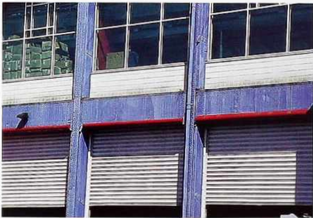
CP-118 Painted metal beam with welded and riveted connections; painted corrugated metal walls
