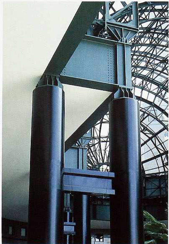
CP-115 Poured-in-place concrete piers supporting deep steel plate girders
