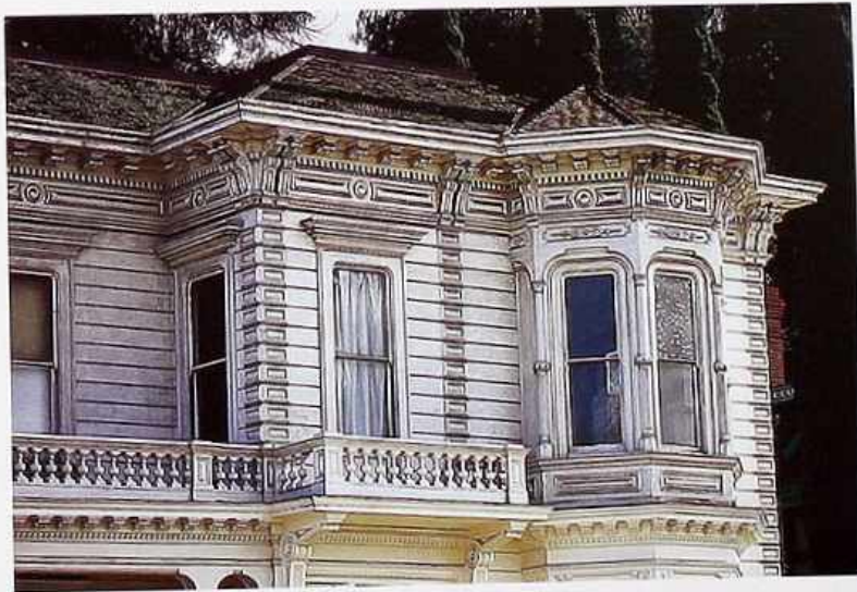
WI-116 Ornament, molding, and balustrade around double-hung windows in cant-bay and wall windows; 19th-c. American clapboard house
