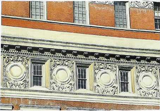
FA-119 Brick facade with decorative masonry frieze of sculpted spandrels between windows
