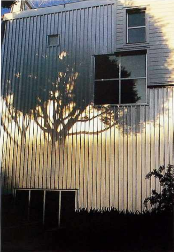
FA-19 Possibly galvanized steel, batten-seam vertical panels
