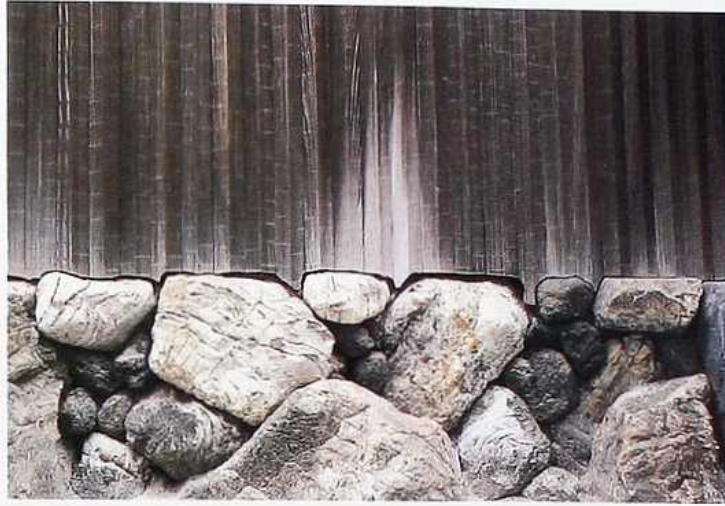
WA-270 Vertical planks of weathered cedar shaped to fit profile of fieldstone base
