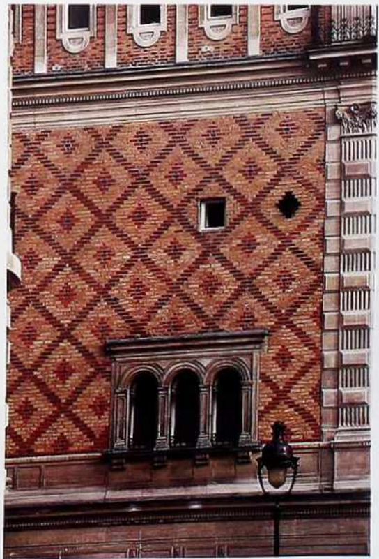
FA-111 Diamond-patterned brick facade with window arcade, framed by a rusticated corner pilaster and cornice
