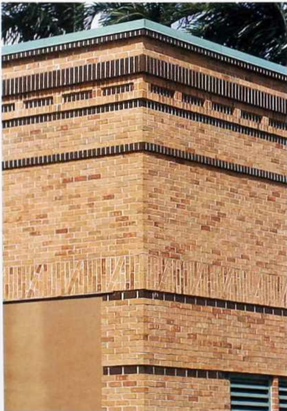
WA-191 Corner detail of bands of running bond, rowlock and soldier courses in contrasting colors, modern commercial building
