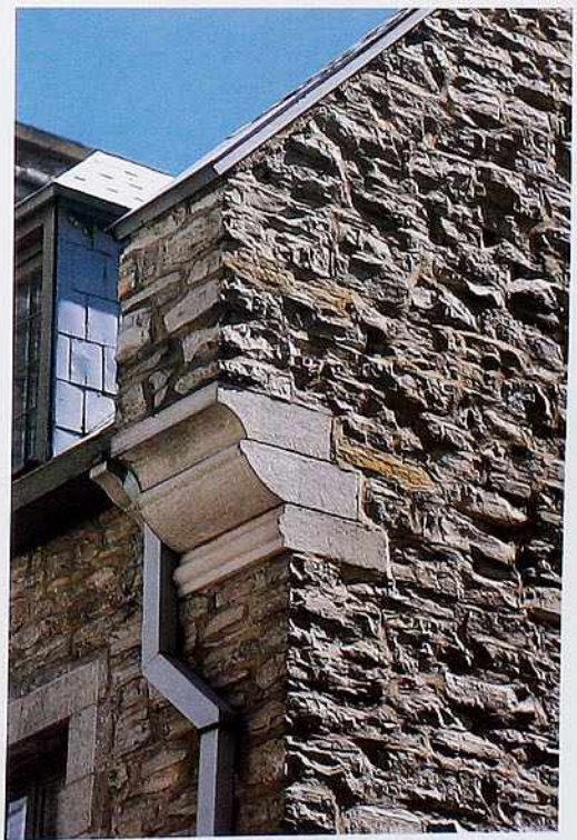
WA-96 Split-faced coursed roughly squared rubble with sand-finished corbel
