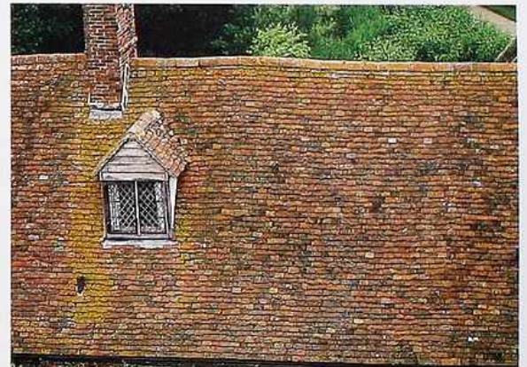
CR-52 Weathered flat shingle tiles with gabled roof dormer
