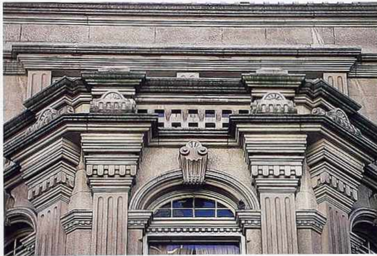
OM-99 Two cornices, the lower supported by flat pilasters with molded imposts with scalloped dentil motif; balustrade in the frieze position
