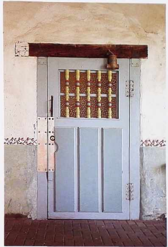
DW-42 Door with painted panels and grille of turned spindles; stucco adobe doorway with exposed timber lintel, American Southwestern mission
