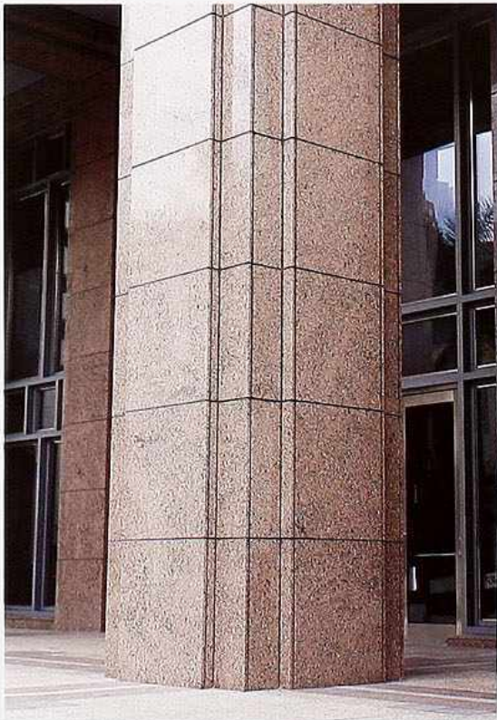
CP-128 Rectangular stone-veneer pier with articulated corners supporting portico, modern commercial building
