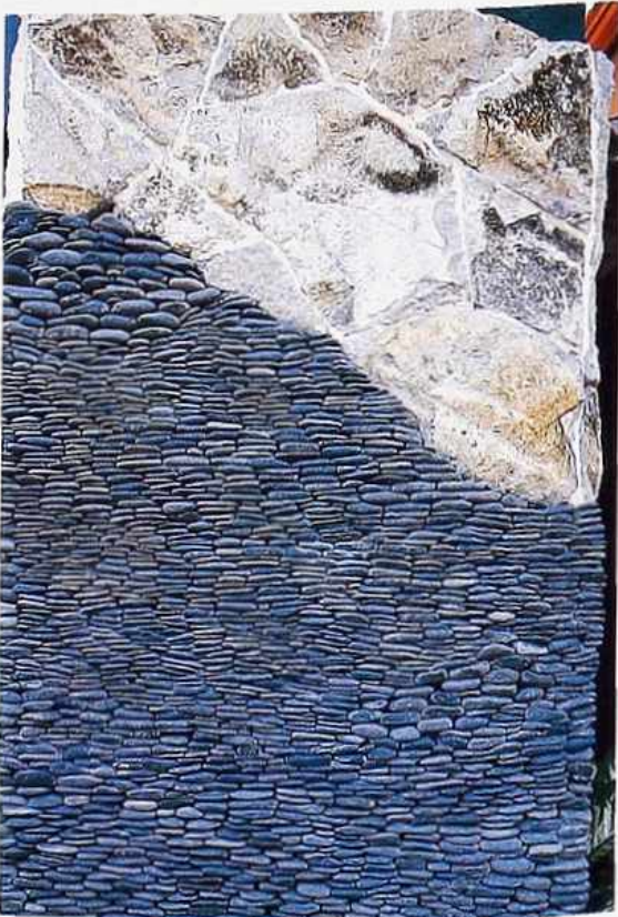
WA-74 Top: fieldstone rubble in mosaic bond; bottom: coursed rubble of beach pebbles
