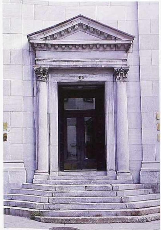
DW-73 Classical-style marble entry with steps, Corinthian columns and entablature, and pediment with block modillions
