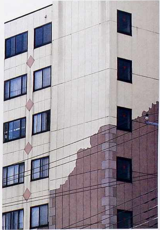
WA-247 Colored smooth stucco supergraphic with stucco quoins in lower section, modern apartment house
