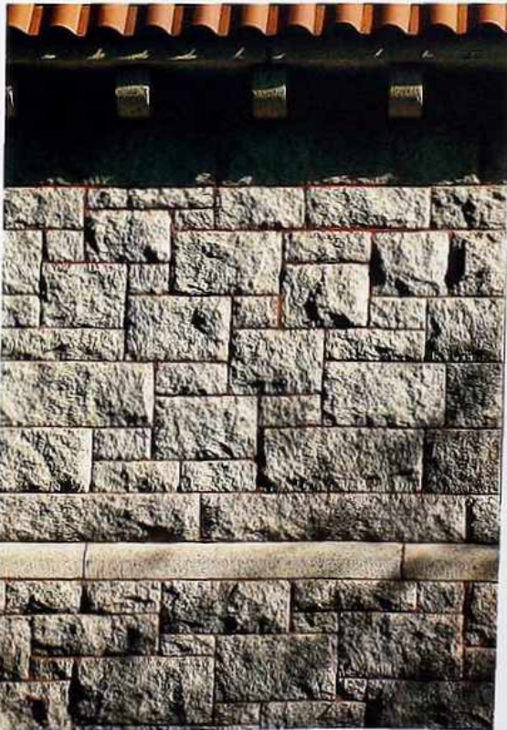
WA-58 Split-faced granite in random ashlar with smooth-faced water-table course, tinted mortar
