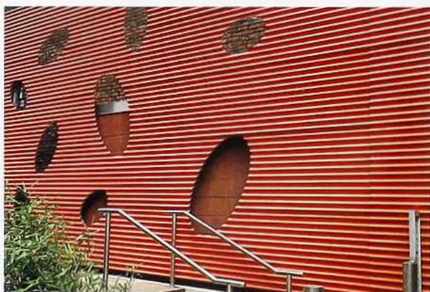
FA-4 Painted corrugated metal screen wall with elliptical cutouts, urban park
