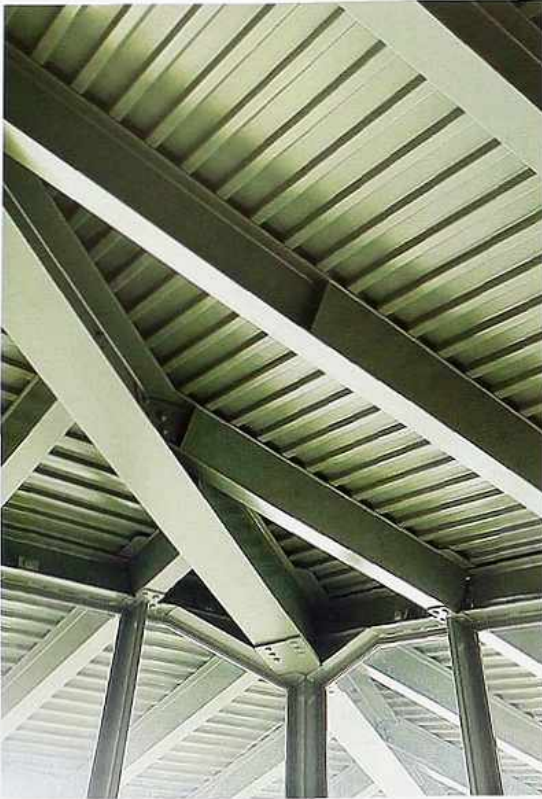
CP-122 Painted steel frame with wide-flange beams and riveted connections, supporting corrugated steel decking, ceiling of modern house
