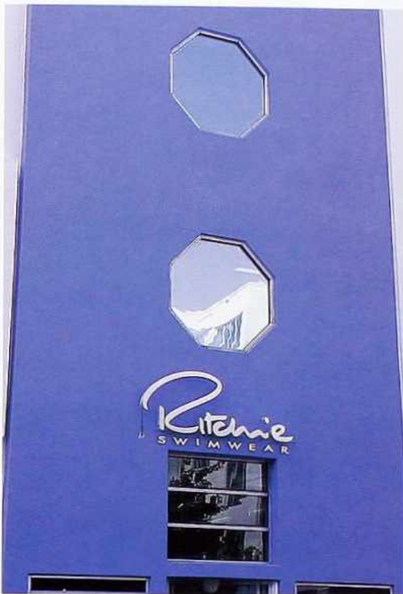
WI-59 Fixed hexagonal windows, modern commercial building
