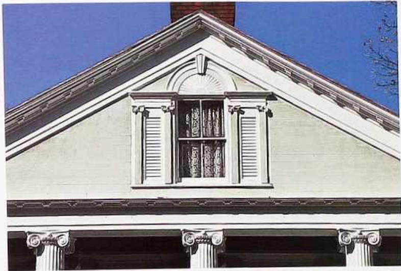
WI-115 Round pediment over gable double-hung dormer window flanked by pairs of attached columns
