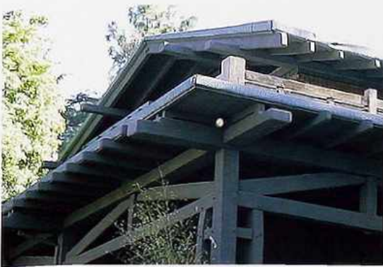
CR-111 Eaves of hipped roof on notched cross-beams, Arts and Crafts house
