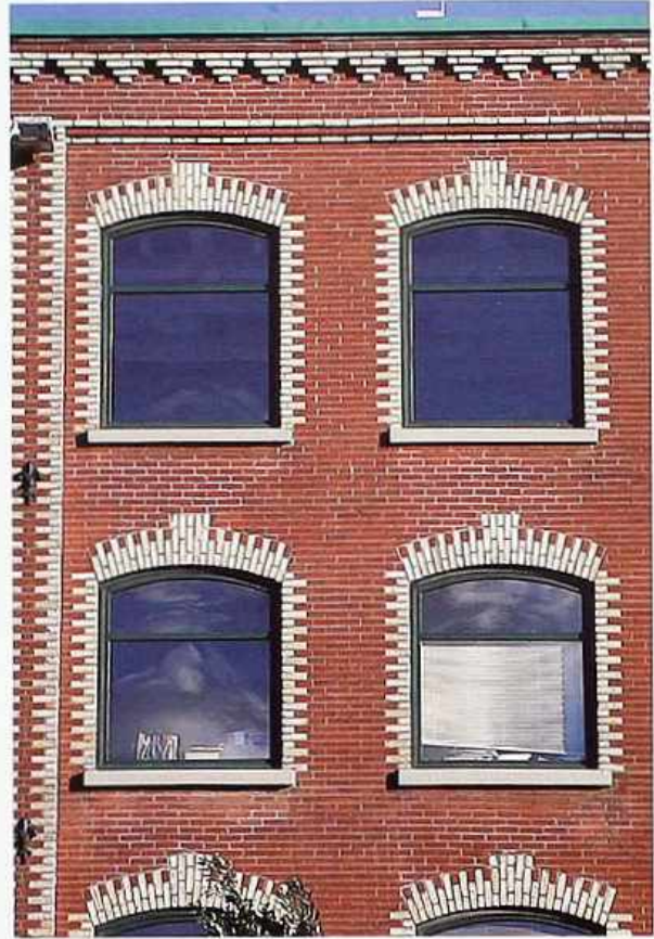
WI-119 Gauged-brick segmental-arch windows with brick quoins and "keystones" in contrasting color
