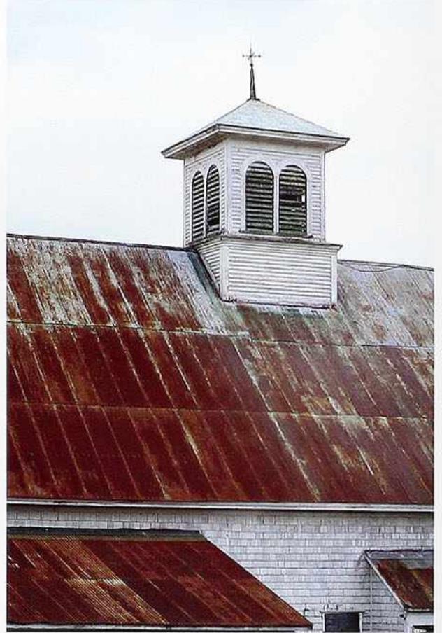
CR-38 Weathered corrugated metal barn roof with pyramidal roof on monitor
