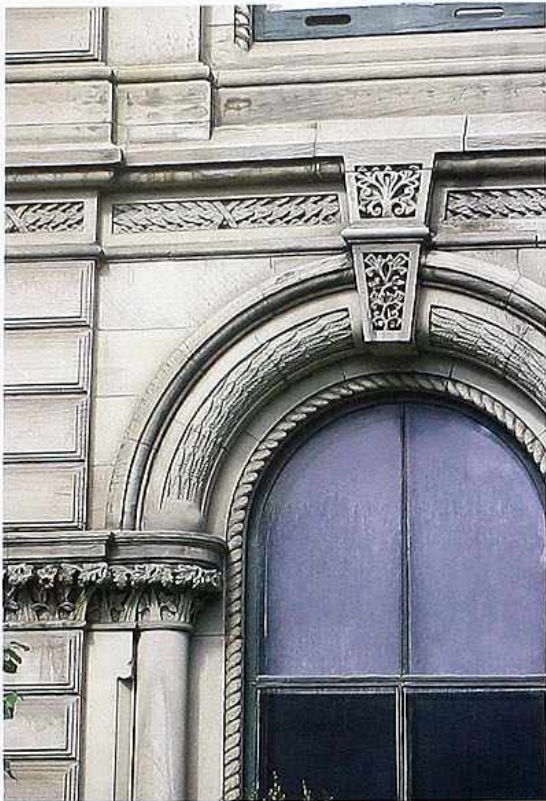
CP-146 Semicircular arch around window with ornamented keystone, rope and foliated moldings
