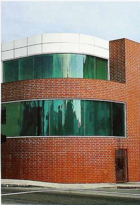
WI-88 Curved corner strip windows, modern commercial building
