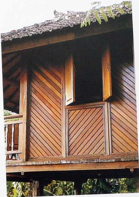
WA-40 Tongue-and-groove panels in alternating diagonal patterns, Indonesian house on stilts
