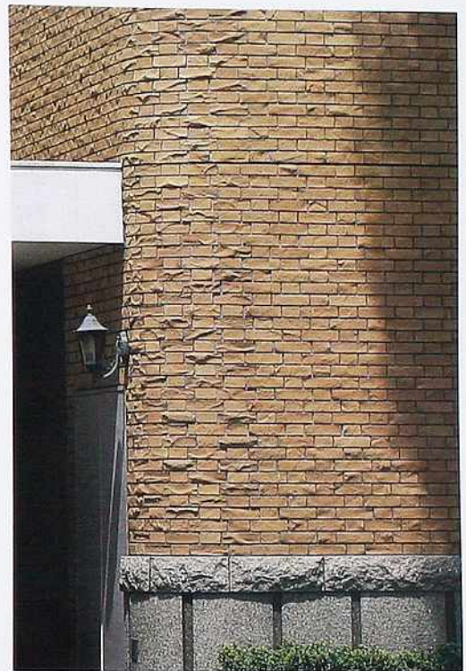
WA-150 Rusticated brick in Flemish bond, shelf angle, with curved corner above granite rock-face belt course and honed base
