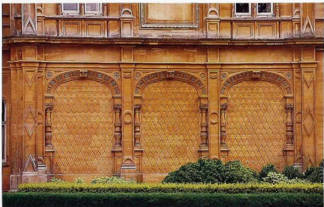
CP-172 Blind arcade: basket-handle (three-centered arch) stone arches with ornament, late-18th-c. courtyard
