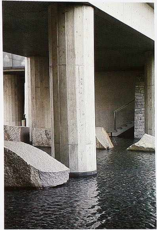
CP-127 Polygonal concrete pier supporting overhang, reflecting pool in modern commercial building
