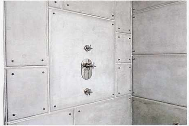
WA-215 Cast concrete, shower room
