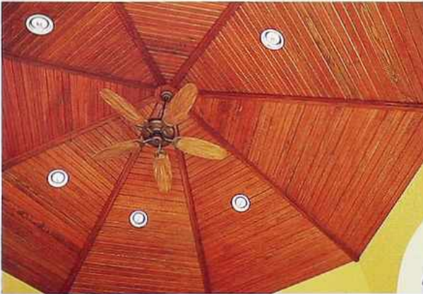
CR-7 Octagonal tongue-and-groove pool-house ceiling, modern house
