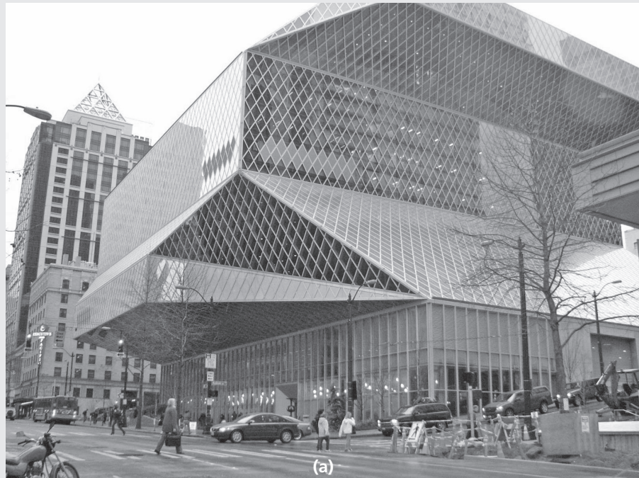
Figure 4.7 Rem Koolhaas OMA: Seattle Public Library (a); CCTV Tower, Beijing (b). OMA's theory of "Bigness" conceives of a global cyber-contextual siting of buildings rather than simply responding to localized physical sites. This results in buildings that are essentially interchangeable with regard to locale: the form in (a) can be in Beijing, and vice versa. Photographs courtesy of David Wang.
