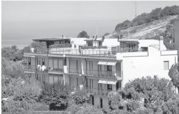
Figure 9.19 View of the building. Courtesy of Elsevier.
