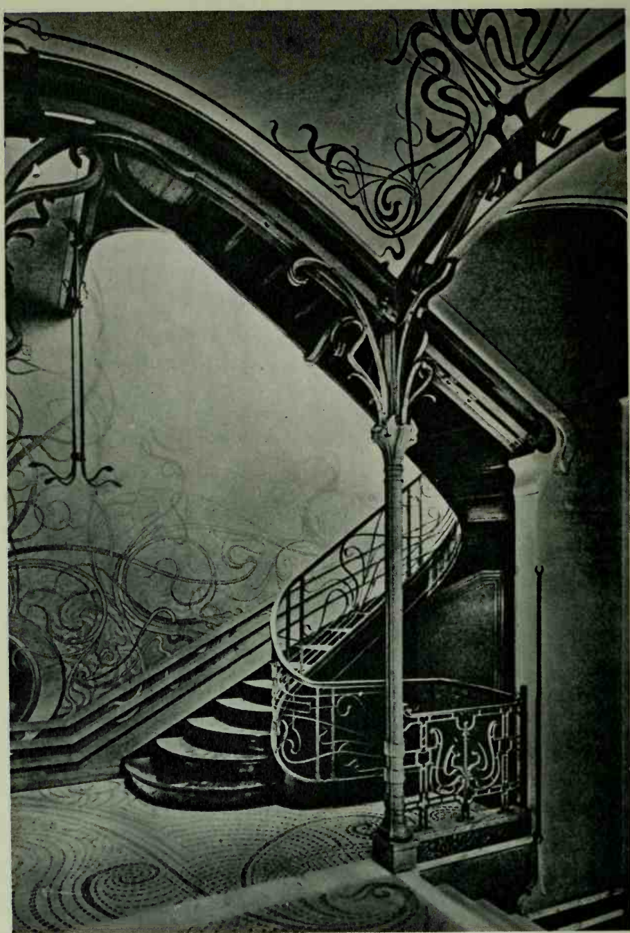
1893. An Art Nouveau interior: the staircase hall of a house in the Rue Turin. Brussels, by Victor Horta.
