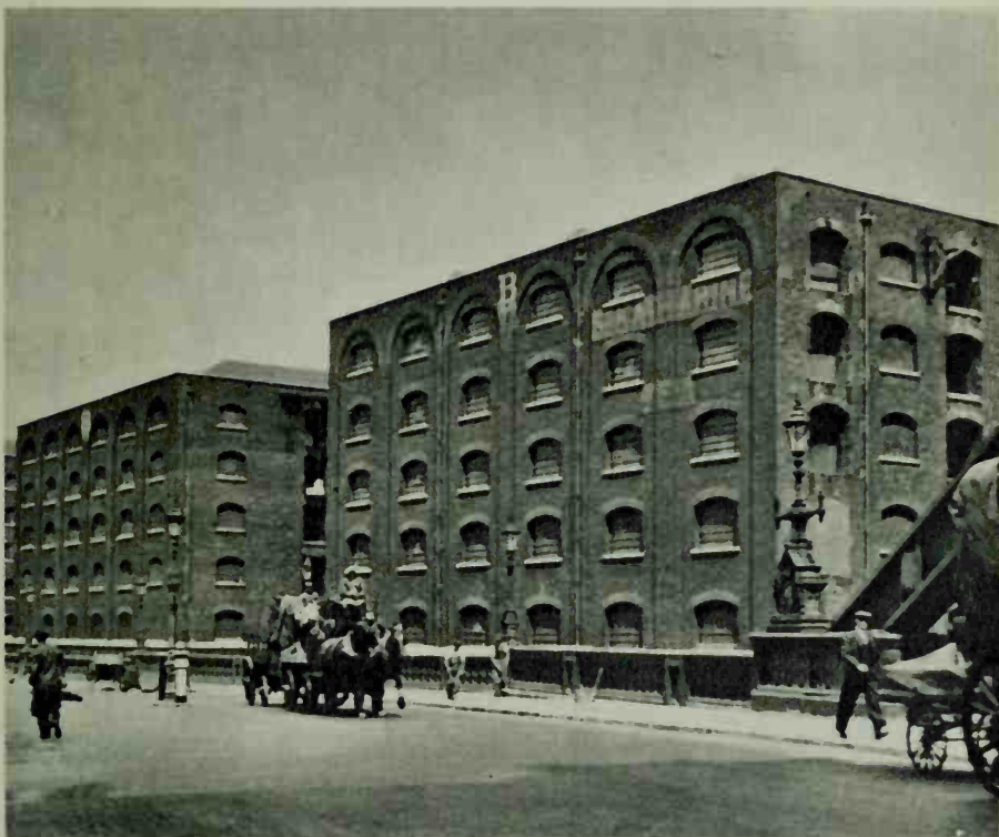
1824–1828. St Katharine's Docks, London, by Thomas Telford. Typical of the simple but noble engineer's architecture of this time.
