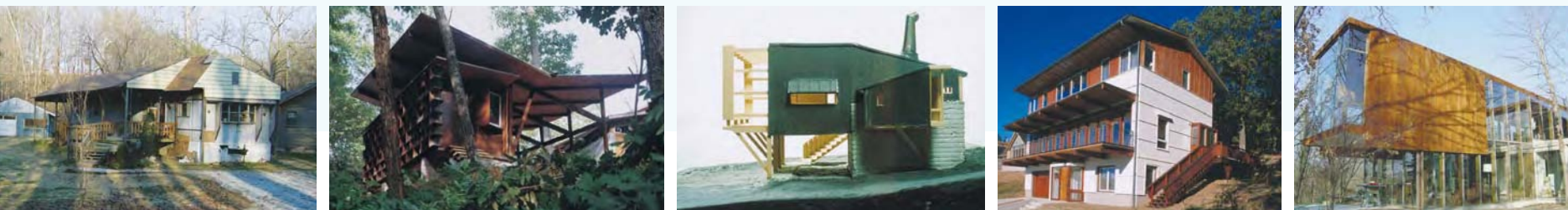
FROM LEFT 4 trailer home with addition, Johnson, Arkansas; 5 Moore HoneyHouse, Cashiers, North Carolina, 1998; 6 BullFrog House prototype, 1992; 7 2Square House, Fayetteville, Arkansas, 1998; 8 Arkansas House, northwest Arkansas, 2004
