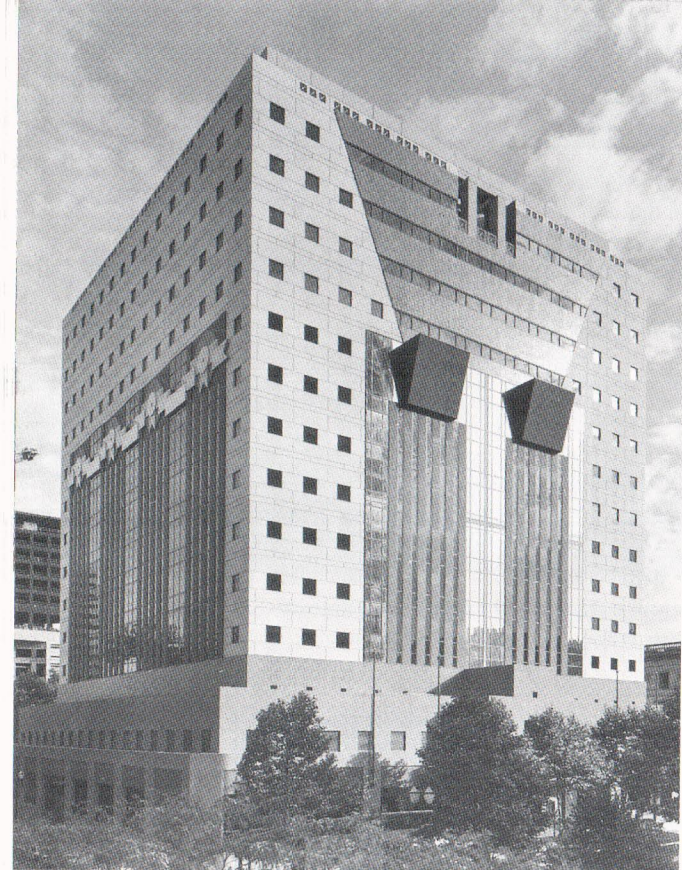
252 Michael Graves, Portland Public Service Administration Building, Portland, Oregon, 1981-82.
