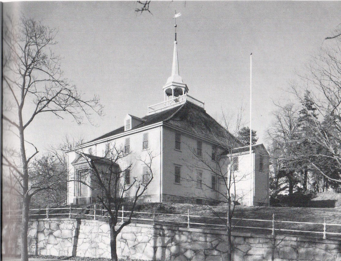
14, 15 Old Ship Meeting House, Hingham, Massachusetts, 1681; additions 1731, 1755.
