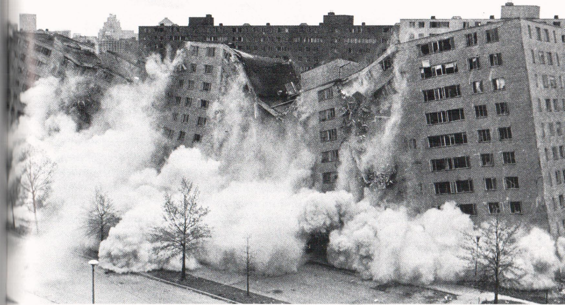
211 Demolition of part of Minoru Yamasaki's Pruitt-Igoe public housing project, St. Louis, Missouri, 1972.
