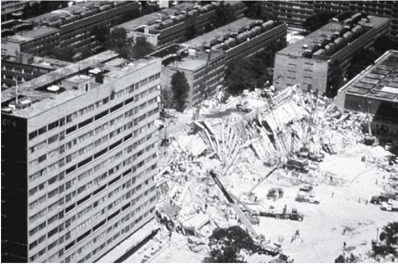
Figure 2. Typical Mexican residential reinforced concrete construction
