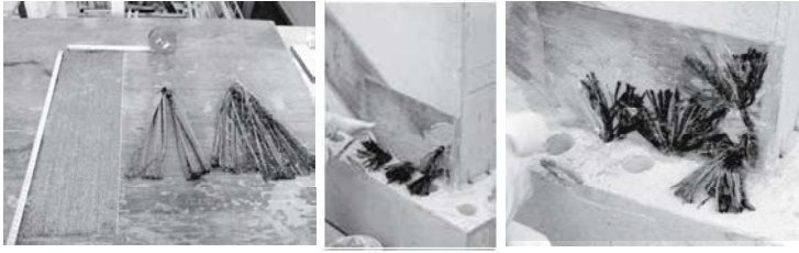
Figure 4. Preparation of CFRP anchors
