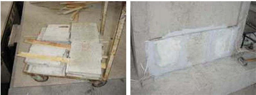
Figure 8. Panels with different geometry (left); glued panels (right)
