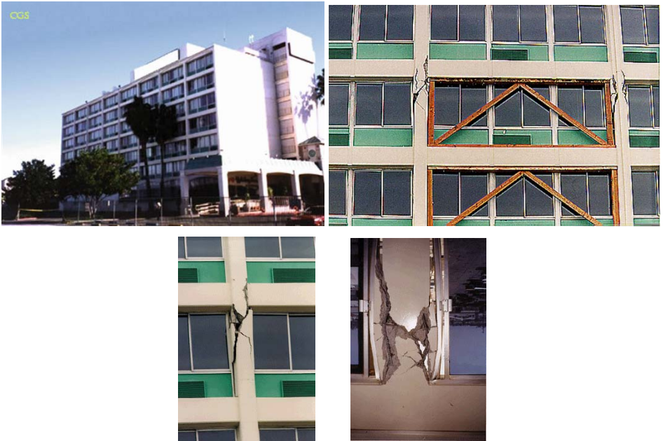
Figure 15. The Van Nuys 7-Story Hotel and damage to its fourth floor columns during the 1994 Northridge earthquake
