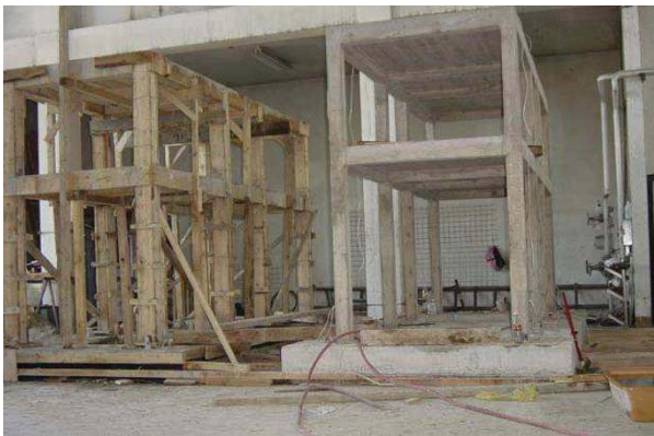
Figure 1. Display of the test specimens during construction
