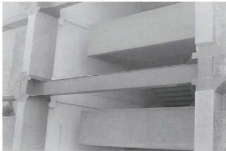
Figure 13. Added beams in stairway areas for continuity between braced bays
