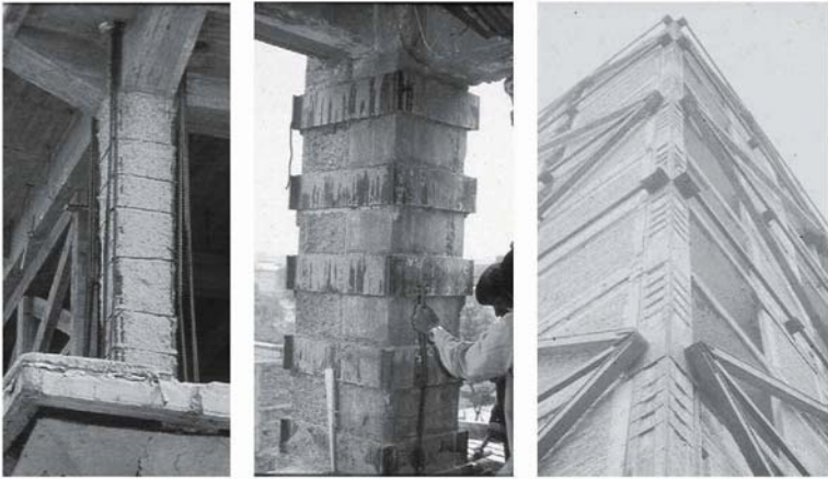
Figure 5. Examples of column jacketing
