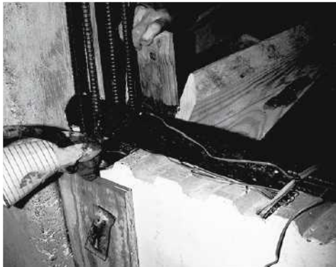
Figure 9. Grouting of Column Shear Lugs
