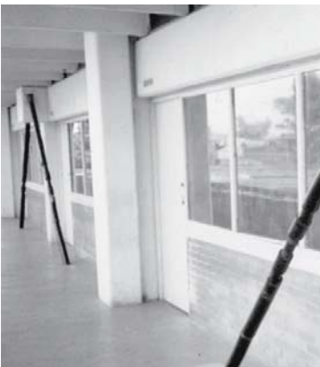
Figure 17. Cable-braced school buildings
