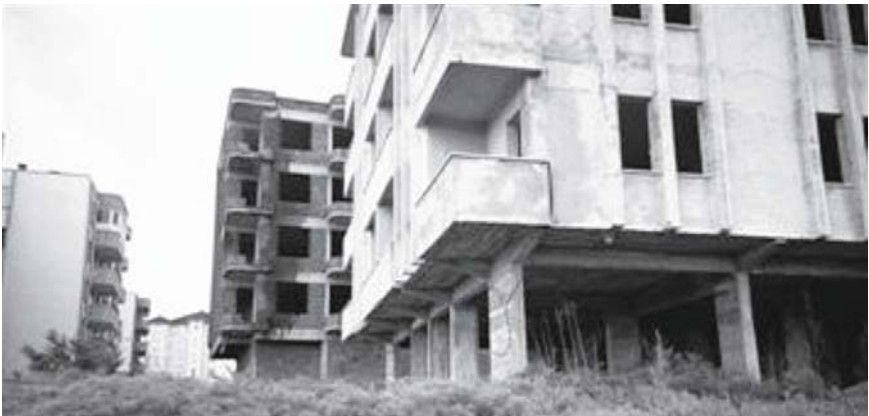
Figure 1. Typical Turkish residential reinforced concrete construction
