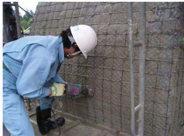
Full scale Mock up after pouring
