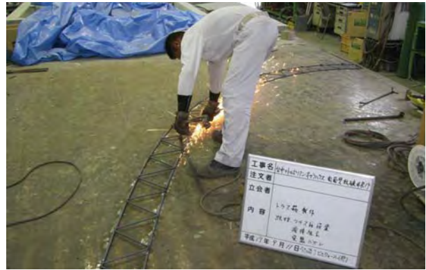
Welding of reinforcement truss
