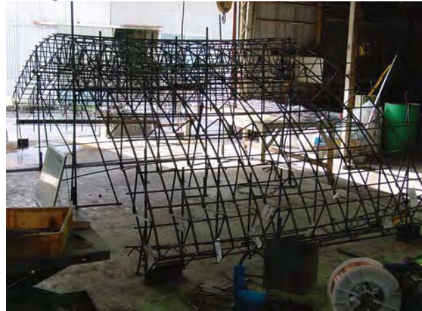
Pre assembled Truss wall
