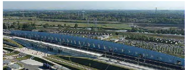
Fig. 4 - Avignon High Speed Train Station
