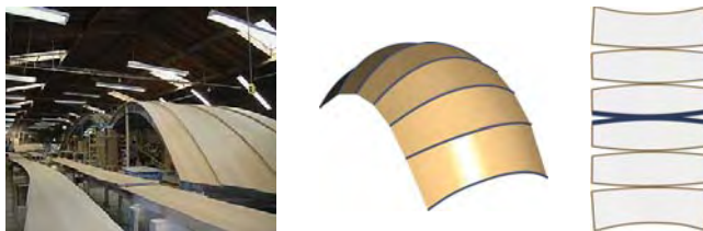
Figure 4: Left: Assembly of wooden strips onto the framing for the interior of the Disney Concert Hall (courtesy Gehry Technologies). Center and Right: Example of a simple geodesic strip model and its development. An edge curve of the geodesic model leads to oppositely congruent curves in the development (blue curve pair).
