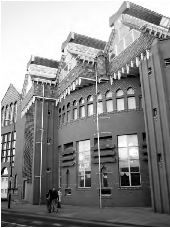
Figure 26.3 Inlet louvres leading to plenum below seating rake
