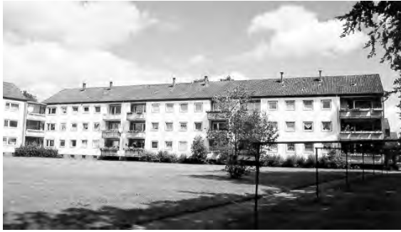
Figure 11.2 Garden view of monitored building
