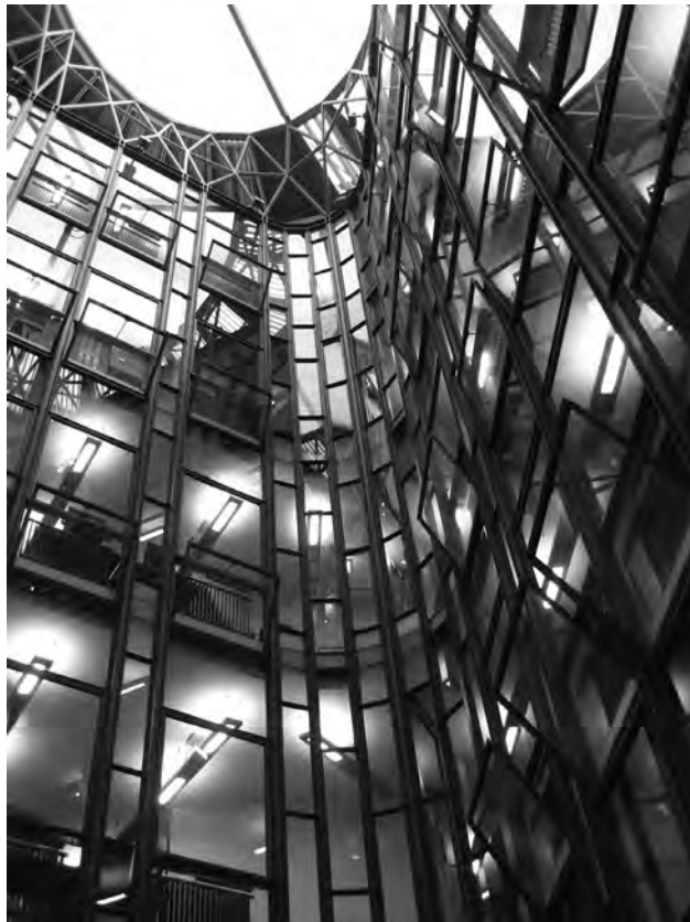
Figure 20.16 The central light well at the heart of the building with the bottom-hung windows
