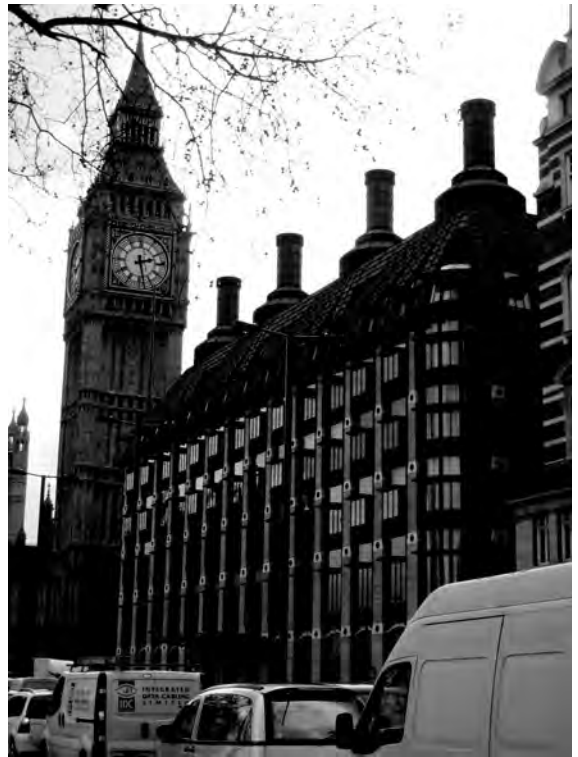
Figure 17.14 Portcullis House, London
