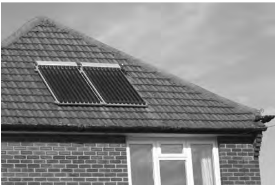
Figure 12.4 Solar panels
