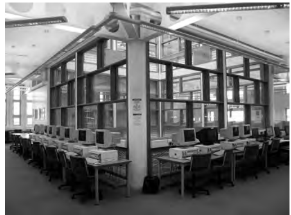
Figure 27.8 Supply lightwell with low-level air inlet dampers and trench heating
