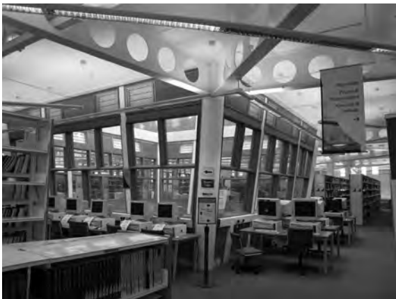
Figure 27.5 Central lightwell, tapered to account for increased airflows higher up the building and to maximize daylight provision across the deep-plan floors
