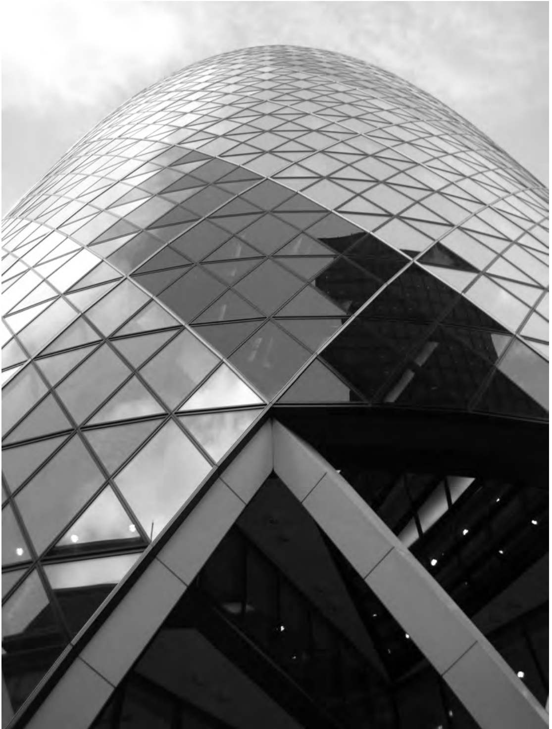
Figure 20.21 Atriums creating spirals of darker glass at the elevation
