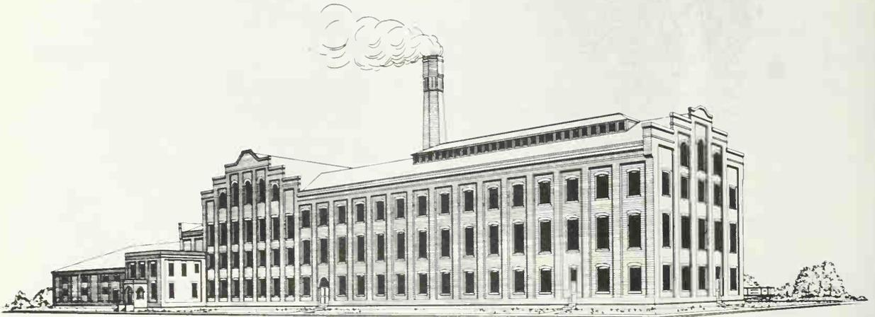
440 Garland Beet Sugar Refinery. Garland, Utah. 1903. Part of an integrated agricultural production system, incorporating an irrigation canal, a hydroelectric generating system, a sugar-beet demonstration farm, and a railroad spur.
