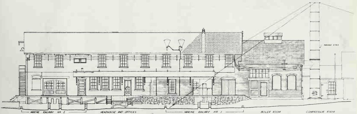
**432** Thames Tow Boat Company, Thames Shipyard, New London, Connecticut. 1900–1903. This was a construction and repair facility for wooden tugs and barges used to transport coal from Virginia to southern New England. It included a steam-powered sawmill, blacksmith shop, joiner shop, storage buildings, sail loft, boiler, and machine shops. Steam-powered marine railways hauled ships to dry ground.
