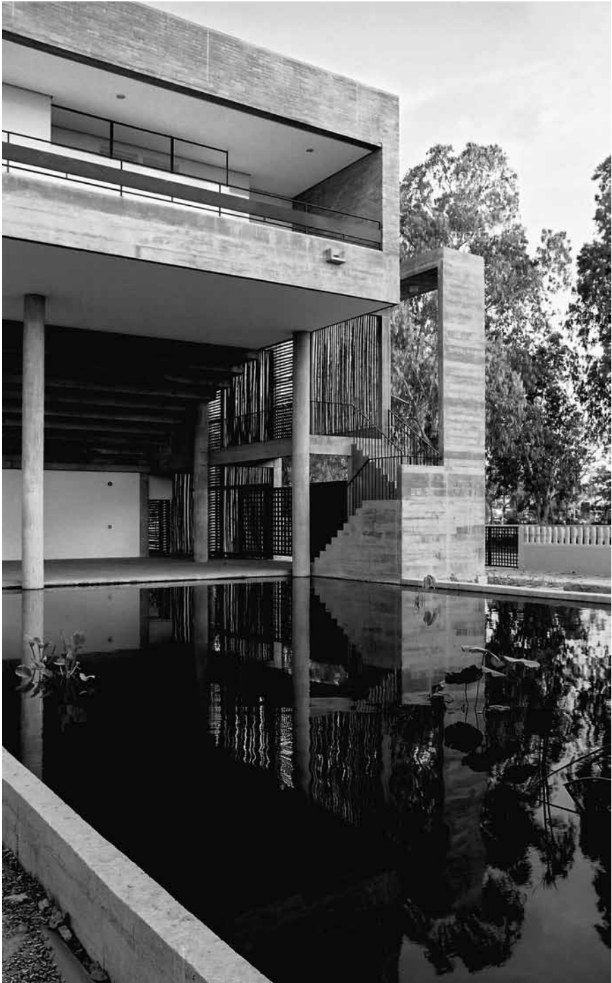
18.7 Local material married with modern expression of the external courtyard. Asma Architects, Kantha Bopha Conference Center, Siem Reap, Cambodia, 2001
