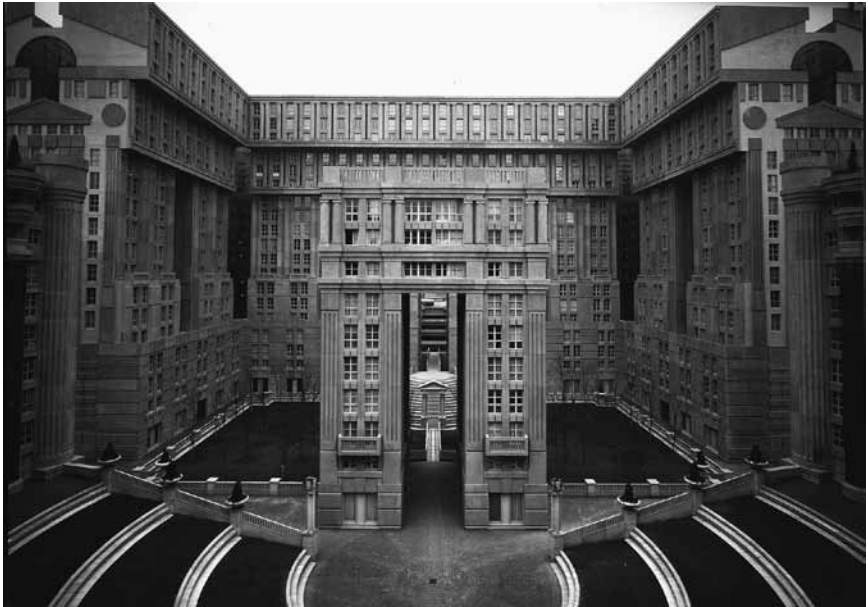
2.9 Taller Ricardo Bofill, Les Espaces d'AbraXas, "L'Arc" and "Le Palacio," Marne la Vallée (France), 1982
