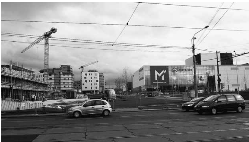
13.12 Construction of Forum Nová Karolina by Multi Corporation, Ostrava, Czech Republic, 2011
