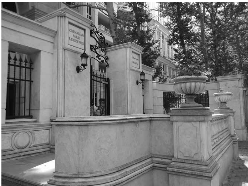
17.11 Chenaran Park Residential Complex by Farzad Daliri. Tehran, Iran, 2008. Left to right: General view; entrance to the complex; details of façade
