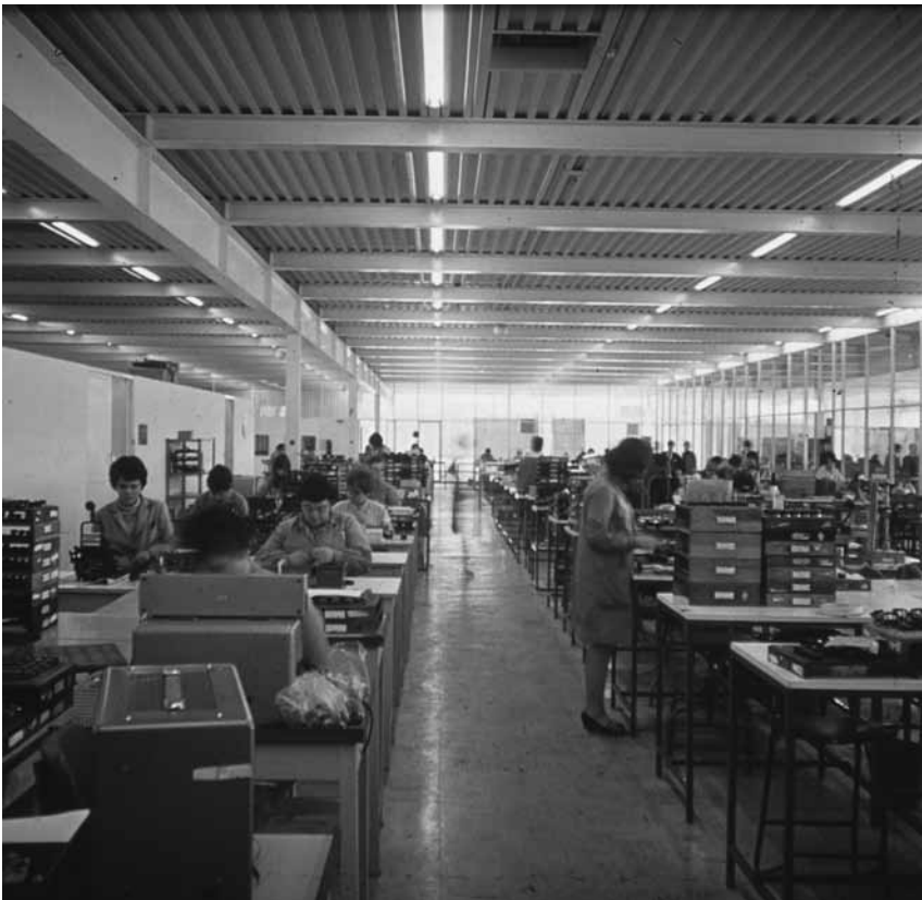
3.4 Team 4, Reliance Controls Factory, interior
