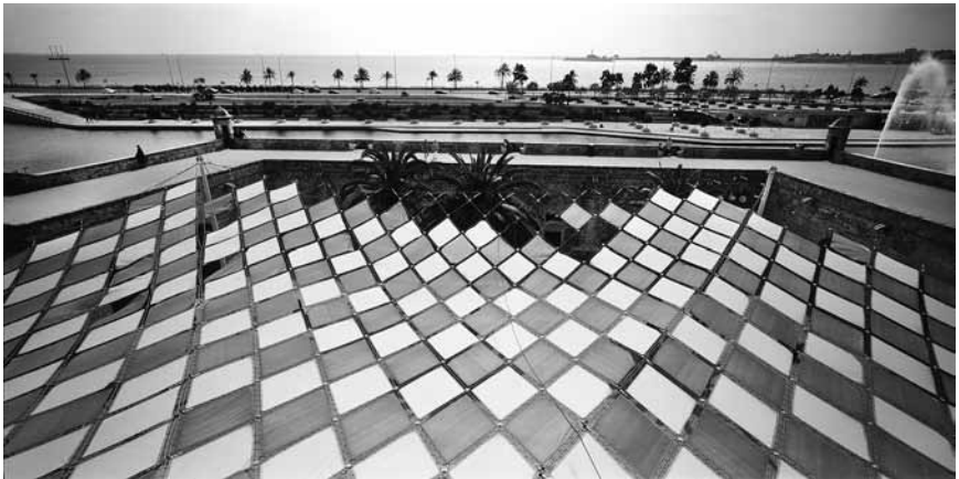
11.8 Elias Torres and Martínez Lapeña. Restoration of City Walls. Palma de Mallorca, 1983–1992
