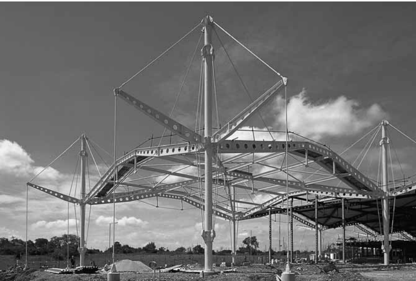
3.11 Foster + Partners, Renault Distribution Centre, Swindon, England, 1980–82. Left: Axonometric of a structural module. Exterior view of the building under construction
