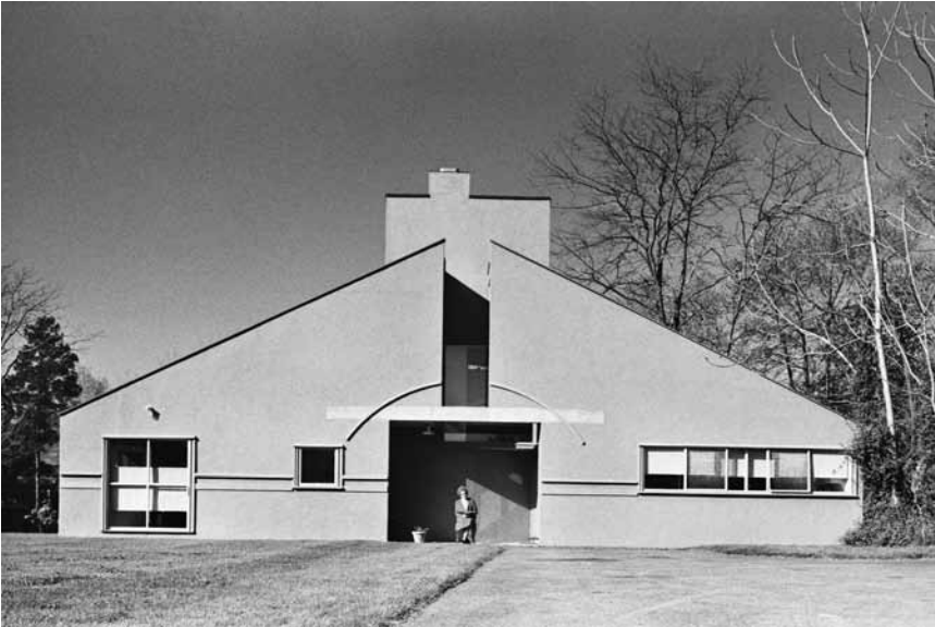
2.1 Robert Venturi, Vanna Venturi House, Philadelphia, 1964
