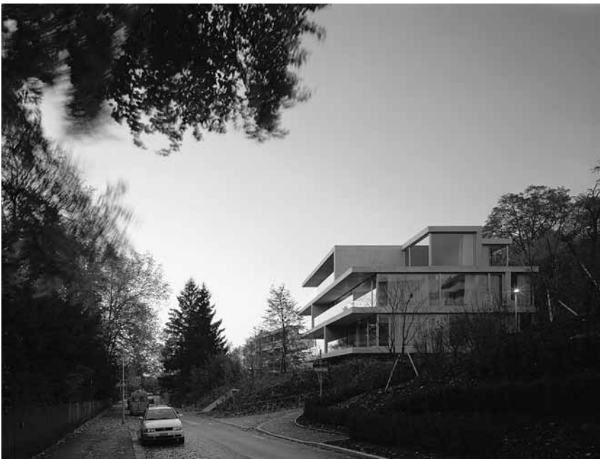
12.8 Christian Kerez: Apartment Building, Forsterstrasse, 1998–2003
