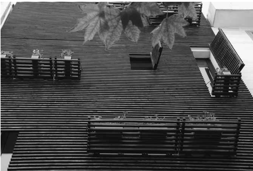
17.4 Dowlat II Residential Complex, 2007. View of the façade with opened wooden panels
