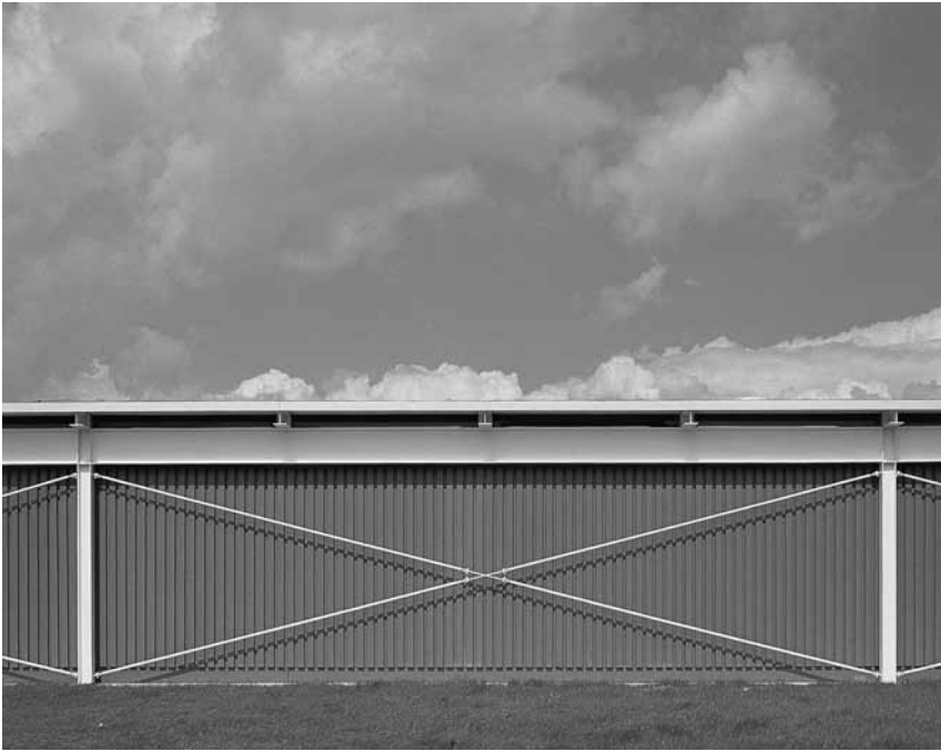
3.3 Team 4, Reliance Controls Factory, Swindon, England, 1965–66, exterior
