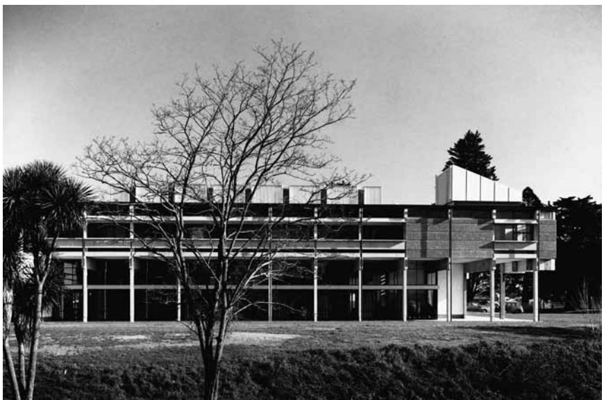
22.2 Warren & Mahoney, Student Union Building, University of Canterbury, Ilam Campus, Christchurch, New Zealand, 1964–67
