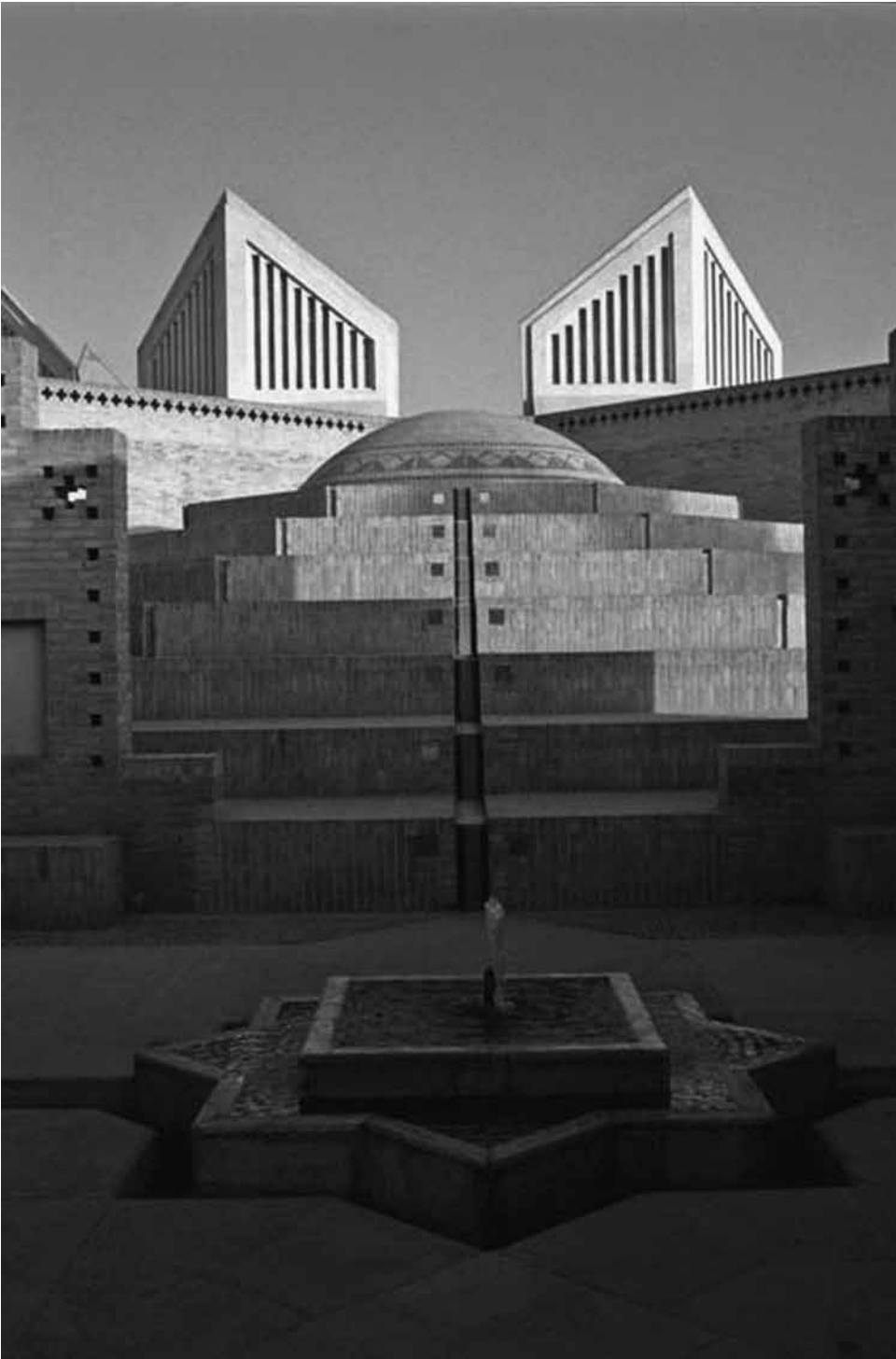
17.3 Dezful Cultural Center, 1995. View across the courtyard fountain
