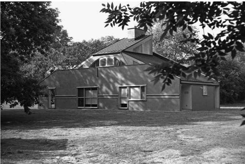
2.2 Robert Venturi, Vanna Venturi House, Philadelphia, 1964
