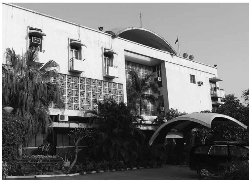
19.3 The curved bangle roof form of the Azad Bhawan building, designed for the Indian Council for Cultural Relations by Achyut Kanvinde (1958–61), is an early example of experimentation with regionally associated forms by an established modernist architect
