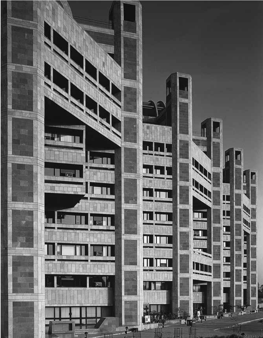
19.7 The SCOPE government office complex, New Delhi (1980–89) by architect Raj Rewal employed sandstone polychromy and undisguised references to the chattris and ramparts of historic Rajput fortresses to ennoble the labour of the army of humble civil servants employed within
