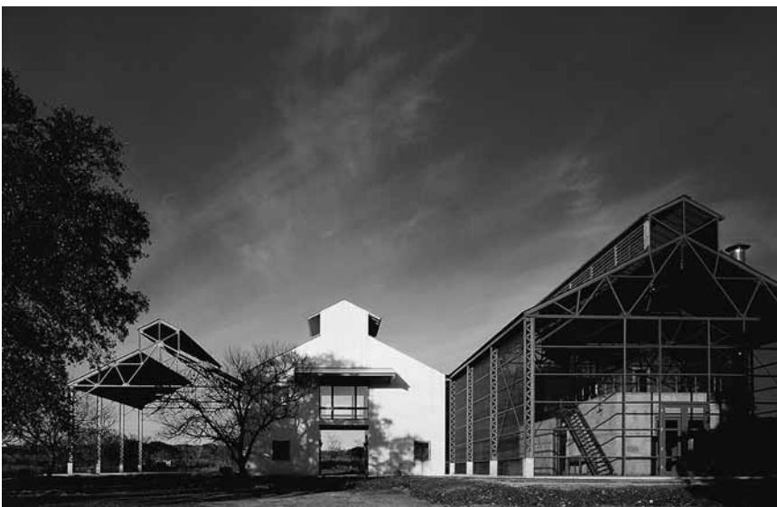
5.8 Lake Flato Architects, Carraro Residence, Kyle, Texas
