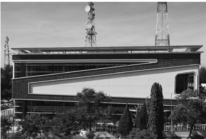
18.5 Advanced technology is combined with soft engineering to create eco-infrastructure. T.R. Hamzah & Yeang Architects, DIGI Technology Operation Center in the Subang High Tech Park, Malaysia, 2012
