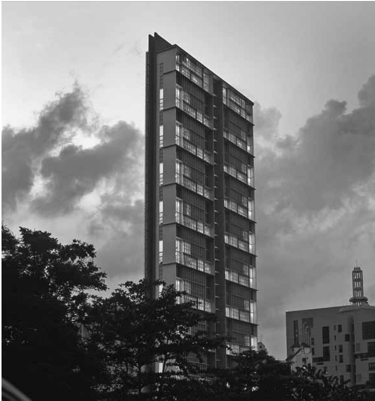
18.10 Interlocking units are visible in the façade. SCDA, Lincoln Modern Tower, Singapore, 2003
