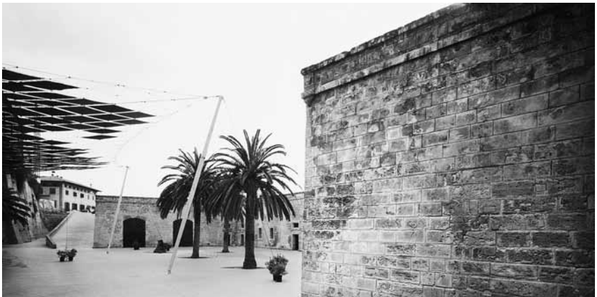
11.9 Elias Torres and Martínez Lapeña. Restoration of City Walls. Palma de Mallorca, 1983–1992
