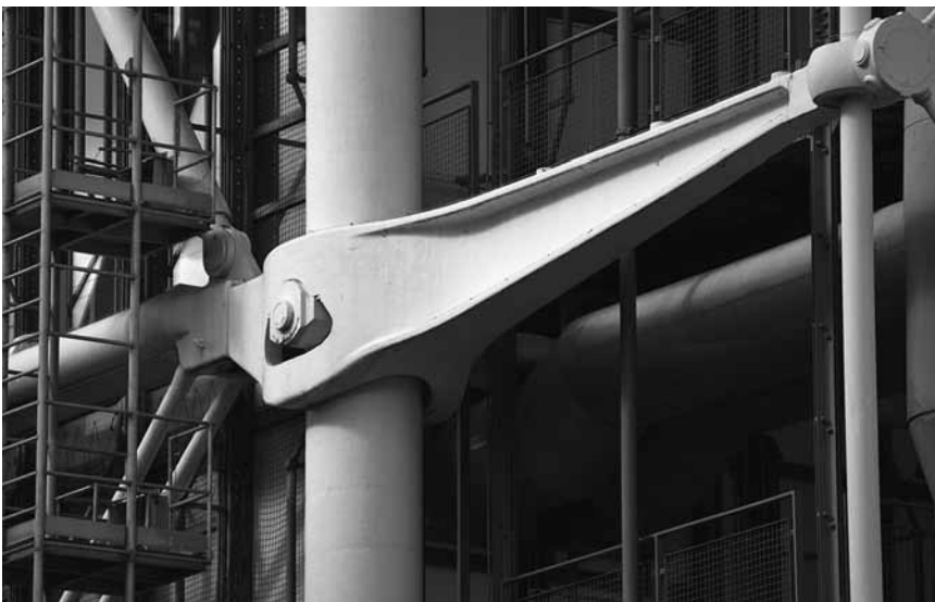
3.1 Detail of the "gerberette" designed by Peter Rice for the Pompidou Center, Paris, France, 1971–77
