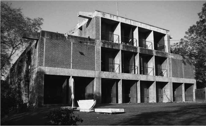
19.1 The School of Architecture at Ahmedabad was a direct outcome of the conjunction of entrepreneurial institution-builders and foreign technical and cultural aid that made Ahmedabad a nexus of international exchange in the 1960s. Built incrementally beginning in 1966 to designs by founding director, B.V. Doshi, the campus and its buildings embodied a dialogue between Doshi, Le Corbusier, and Kahn, with both of whom the architect had enjoyed a close working relationship
