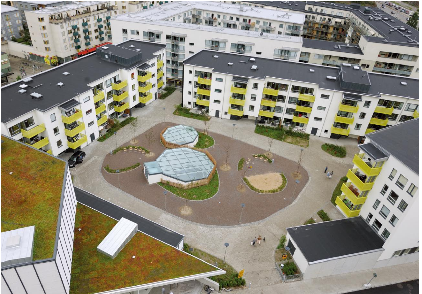
Top left: View from the highway
