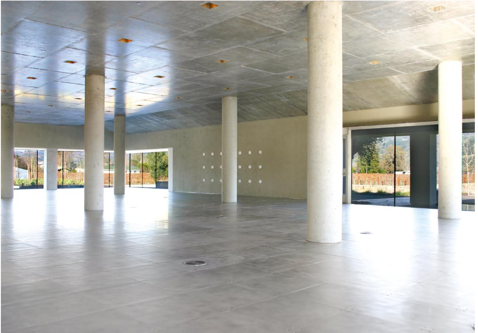
Right: Mirror-like exposed concrete obtained with the use of plastic form liners
