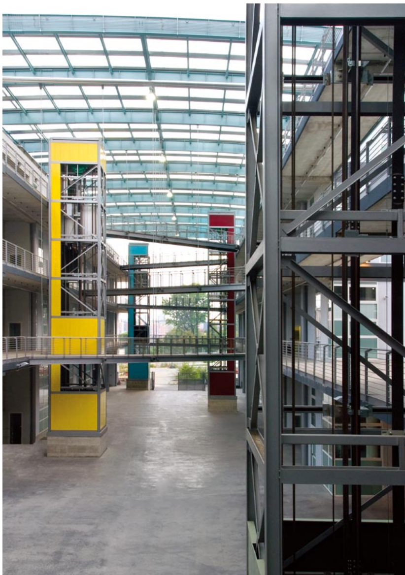
Left: The loading lifts are covered with transparent polycarbonate elements Right: Transparent roofing
