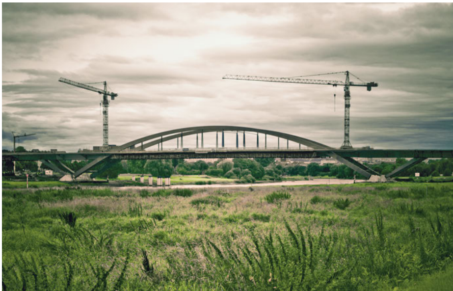
Fig. 3.8: View impaired by Dresden's Waldschlösschenbrücke
