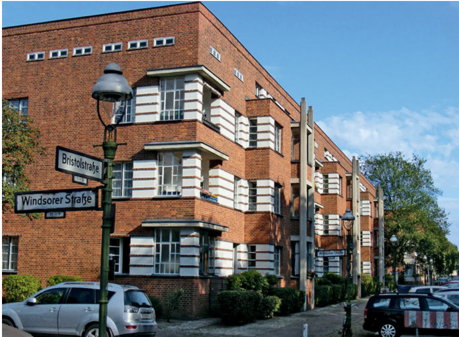
Fig. 2.5: Schiller Park Housing Estate in Berlin (Germany)
