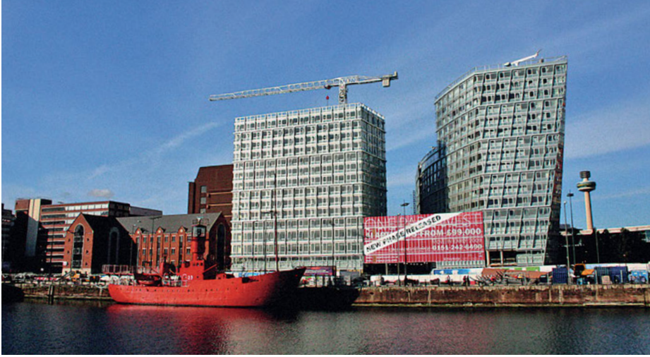
Fig. 4.10: Newly constructed office buildings at Liverpool Docks (United Kingdom)
